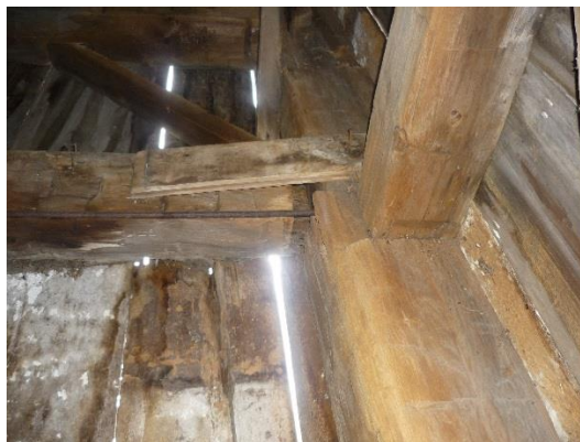
Plate 53: Beam pulling away from post
