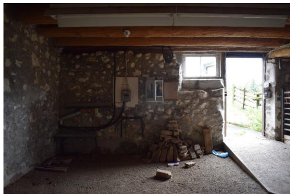
Plate 59: East entrance to stables looking east
