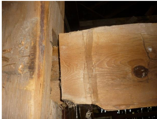
Plate 51: Beam pulling away from post
