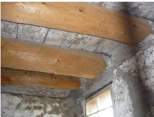
Plate 52: Beam pulling away from post
