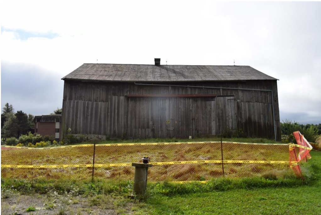
Plate 20: North elevation of barn looking south
