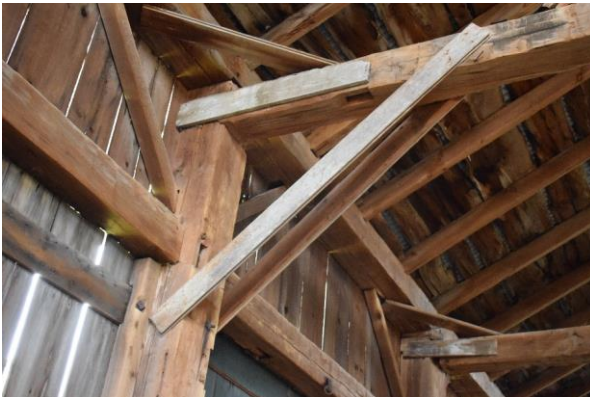
Plate 47: Wood brace on post and bent looking southwest
