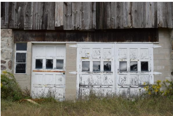
Plate 31: Double doors and man door on south elevation
