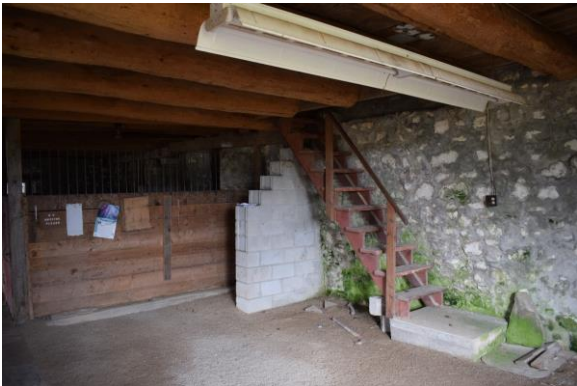
Plate 61: Wooden stairs leading to threshing floor looking northwest
