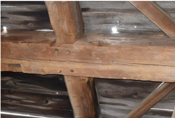
Plate 45: Pins in roof post
