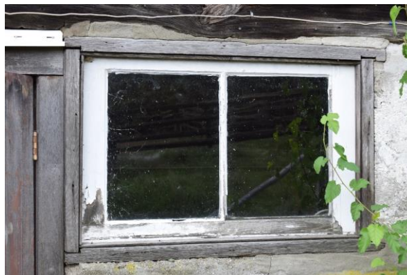
Plate 27: Fixed wood window on east elevation
