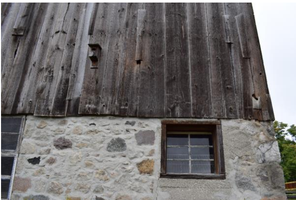
Plate 35: Smaller six-pane wood fixed window on south elevation
