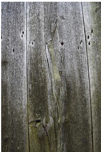
Plate 18: Close-up of vertical wood planks on north elevation
