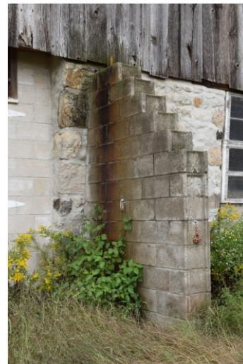
Plate 36: Concrete support wall on south elevation
