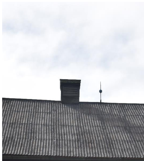
Plate 19: Ventilator and lightning rod on roof looking south
