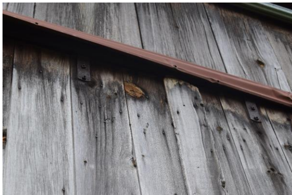
Plate 22: North elevation door track and original hangers
