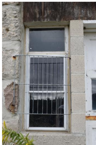
Plate 32: Window adjacent to doorway on south elevation
