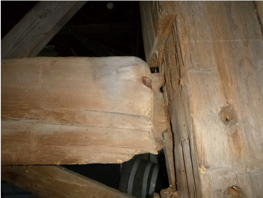
Photograph No. 5: Beam post connection failed.
