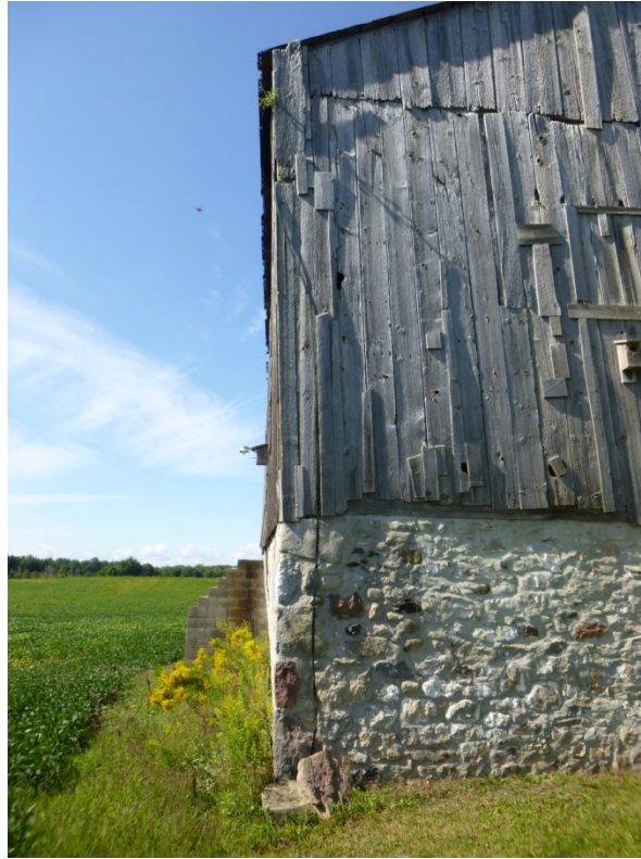
Photograph No. 3: Southeast corner of barn looking west. Foundation wall leans at mid width of barn; block buttress added.
