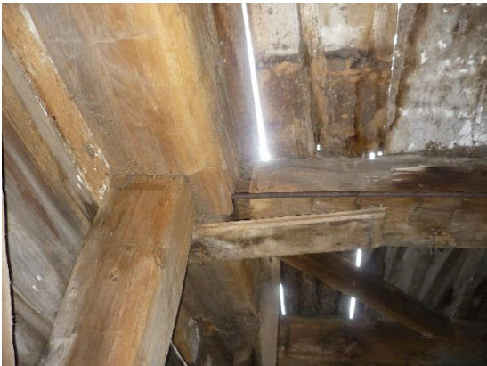
Plate 50: Beam pulling away from post
