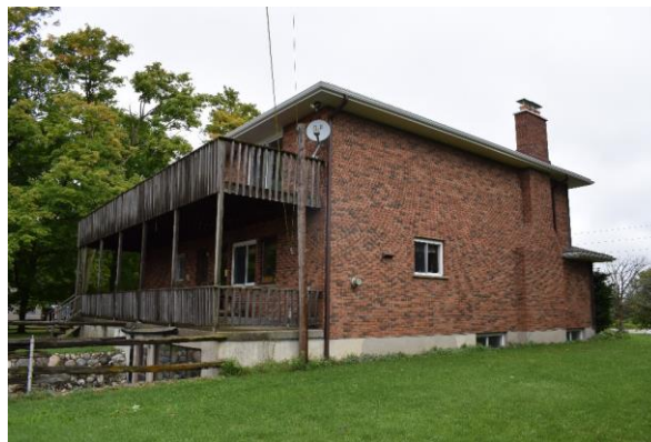
Plate 13: Southwest elevation of residence looking northeast
