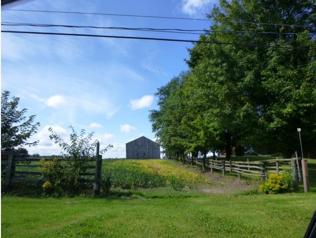
Photograph No. 1: Barn noticeably leaning southward.
