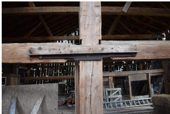
Plate 44: Close-up view of post with metal plate
