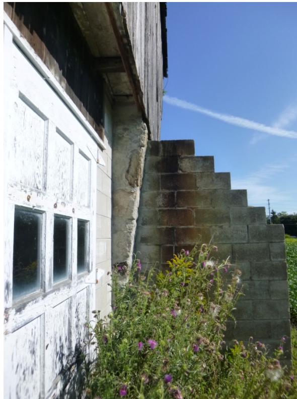
Photograph No. 4: Block buttress at leaning south foundation wall.
