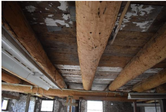
Plate 62: Wood beams looking south
