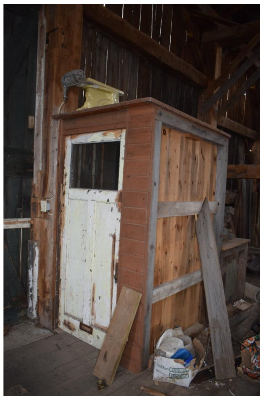
Plate 40: Vestibule wood entrance door
