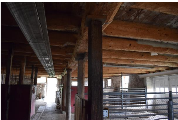
Plate 63: Wood beam extending the length of the barn looking southeast
