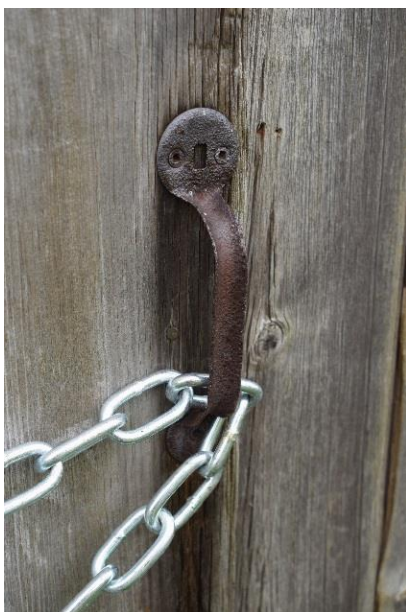
Plate 23: Original metal handle on north elevation doors
