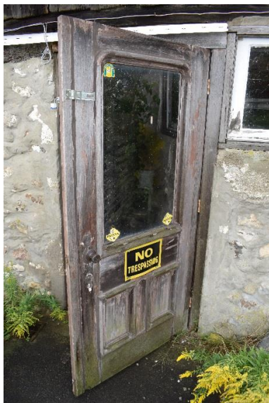
Plate 26: Wood half glass entrance door on east elevation
