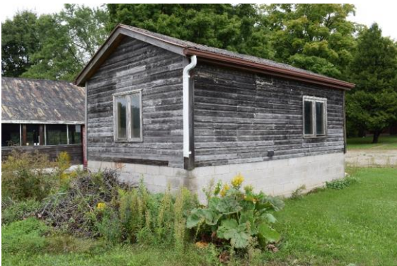
Plate 16: Small outbuilding looking northeast
