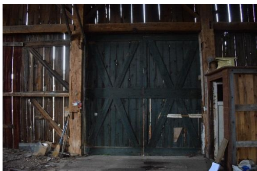
Plate 39: Wood entrance doors to threshing floor looking north
