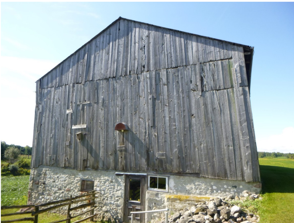
Photograph No. 2: East wall wood structure leaning south. Foundation wall stable (not leaning).
