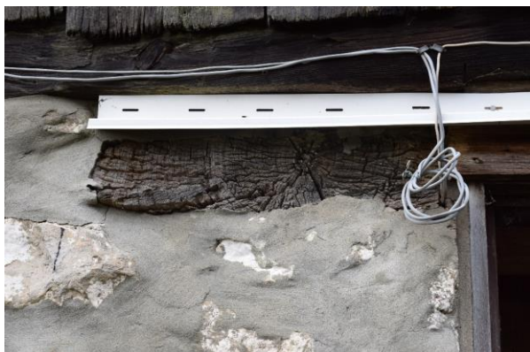
Plate 28: Timber beam end on east elevation
