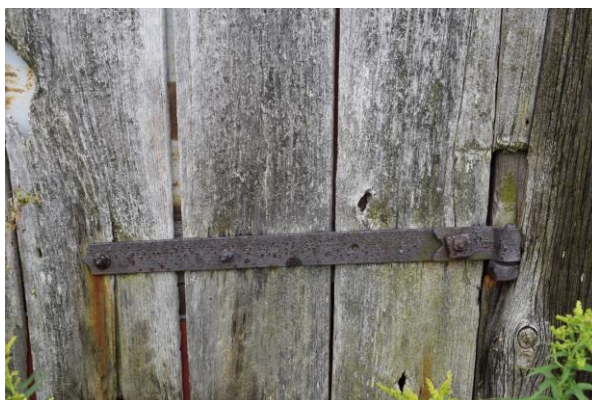
Plate 24: Original metal hinge on north elevation door
