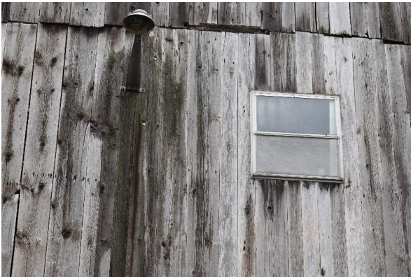
Plate 33: Window and light fixture above doorway on south elevation
