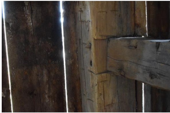
Plate 46: Mortise and pinned wood bent looking west
