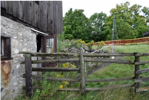
Plate 9: Cedar spilt-rail fencing on east elevation of barn
