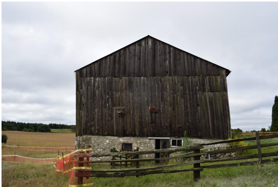
Plate 25: East elevation of barn looking west
