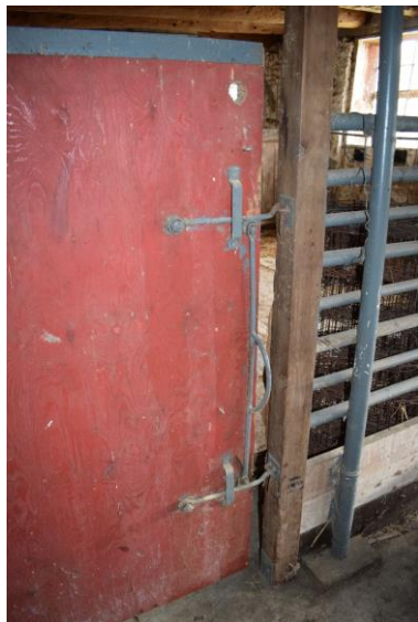
Plate 69: Horse stall door on south side looking southeast, with original lock
