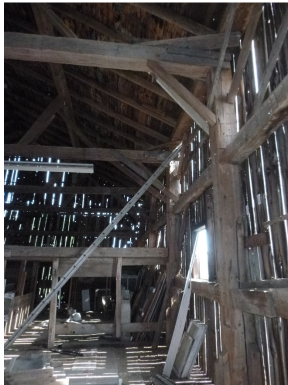
Photograph No. 6: Looking east. Note worst lean is evident at southeast post (18").
