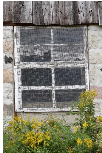
Plate 34: Six-pane fixed wood window on south elevation
