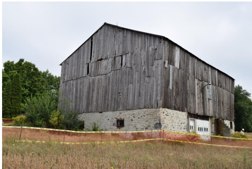
Plate 17: Southwest corner of barn looking northeast
