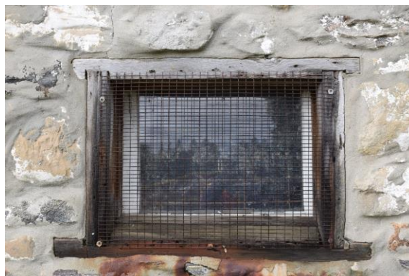
Plate 29: Fixed wood window on east elevation
