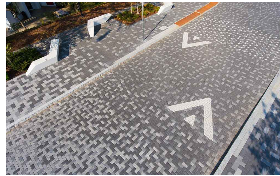
UNIT PAVING IN A GRADIENT PATTERN
