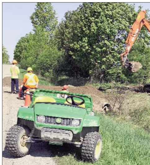
Students from Conestoga College build the road access, parking lot and school bus turning circle for the new Guelph Lake Nature Centre.
