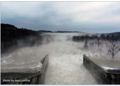
Extremely high river flows due to melting snow and rainfall in mid-April brought some flooding-0in low lying areas. This is the view from the Conestogo Dam when flows were around 170 cubic metres per second. They did get as high as 250 cms, compared to 4.5 cms during the summer. The fog was created by the cold lake water being discharged into 20-C air tempemperatures.
