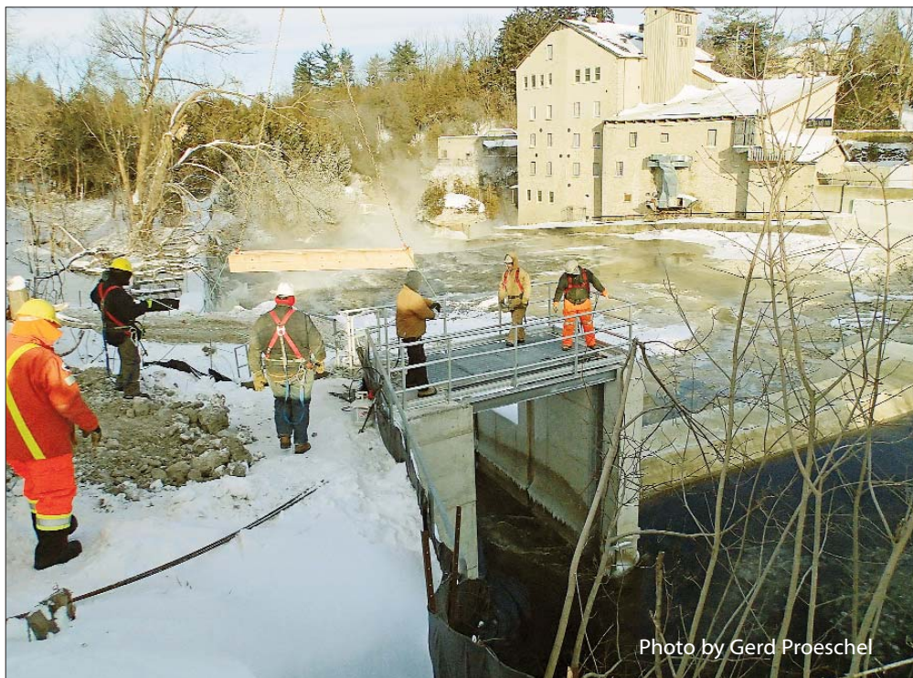
The stop logs were put in place on the new Drimmie Dam in Elora in January on a very cold day. Construction has been underway throughout the winter.
