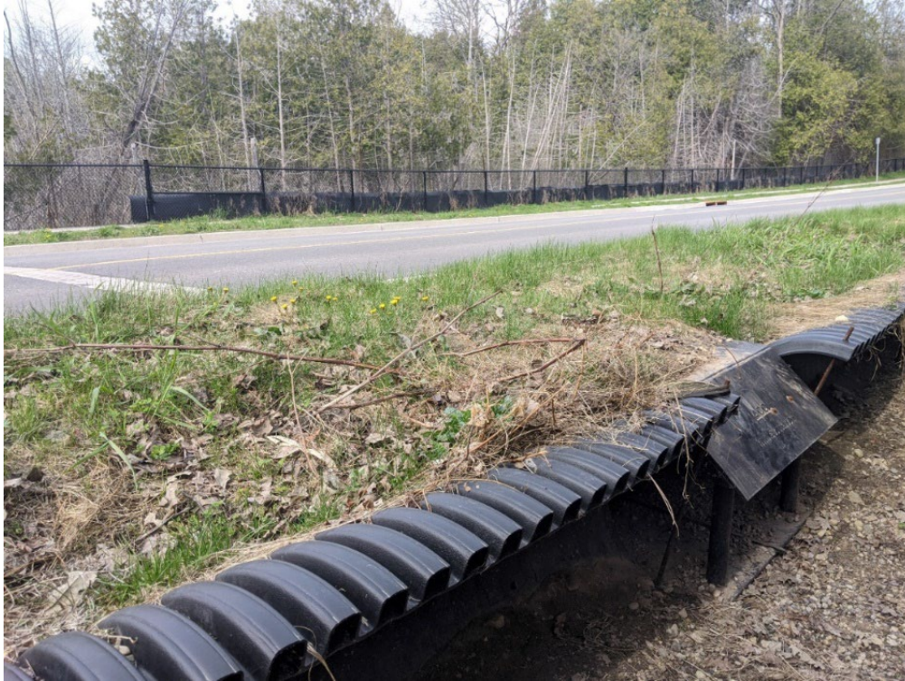
Figure 3 ACO climate tunnel at Niska Road, Guelph with HDPE half-pipe exclusion fencing in foreground and ANIMEX fencing in background (Photo credit: Pauline Catling, North-South Environmental Inc.)
