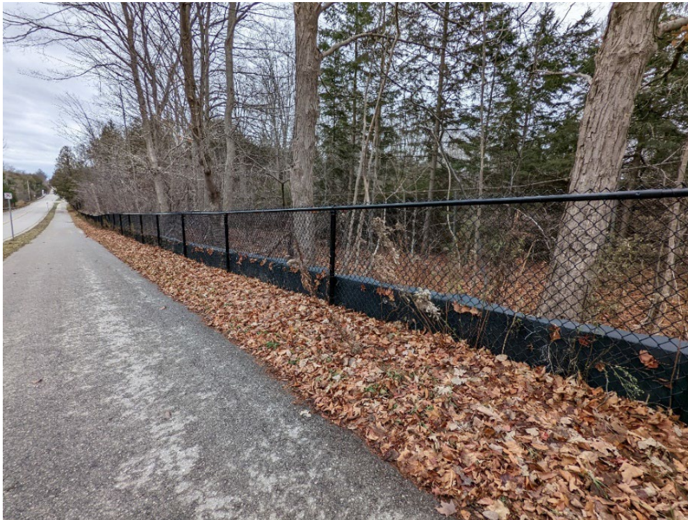
Figure 4 ANIMEX fencing installed on chain link at Niska Road, Guelph (Photo credit: Devin Bettencourt, North-South Environmental Inc.)
