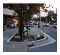
Figure 8.1: Left to Right: Bioswale part of a surface Light Rail Transit; Bioretention Planters as are part of a surface Light Rail Transit; and bioretention bump outs as part of bus lay-bys
