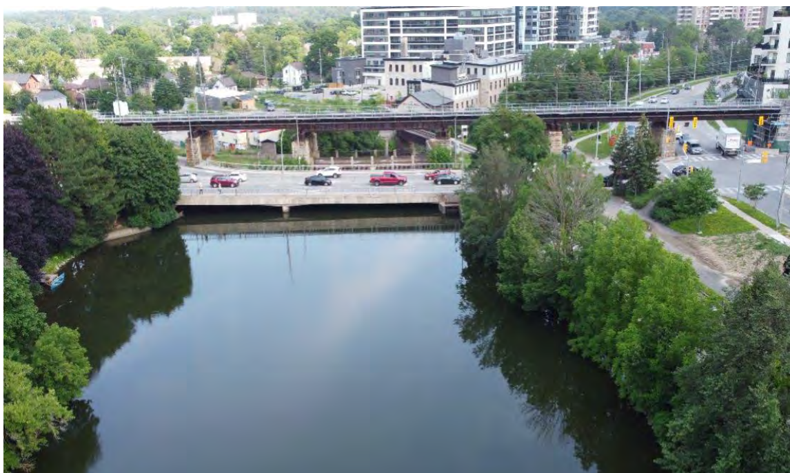
Exhibit 3-1: Macdonell Bridge Aerial View
