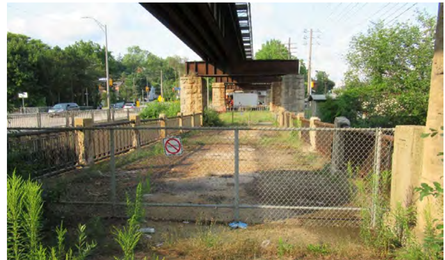
3b) Allans Dam Bridge Closure
