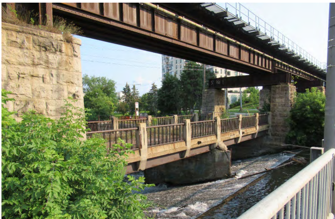
Exhibit 4-1: Allans Dam Bridge
