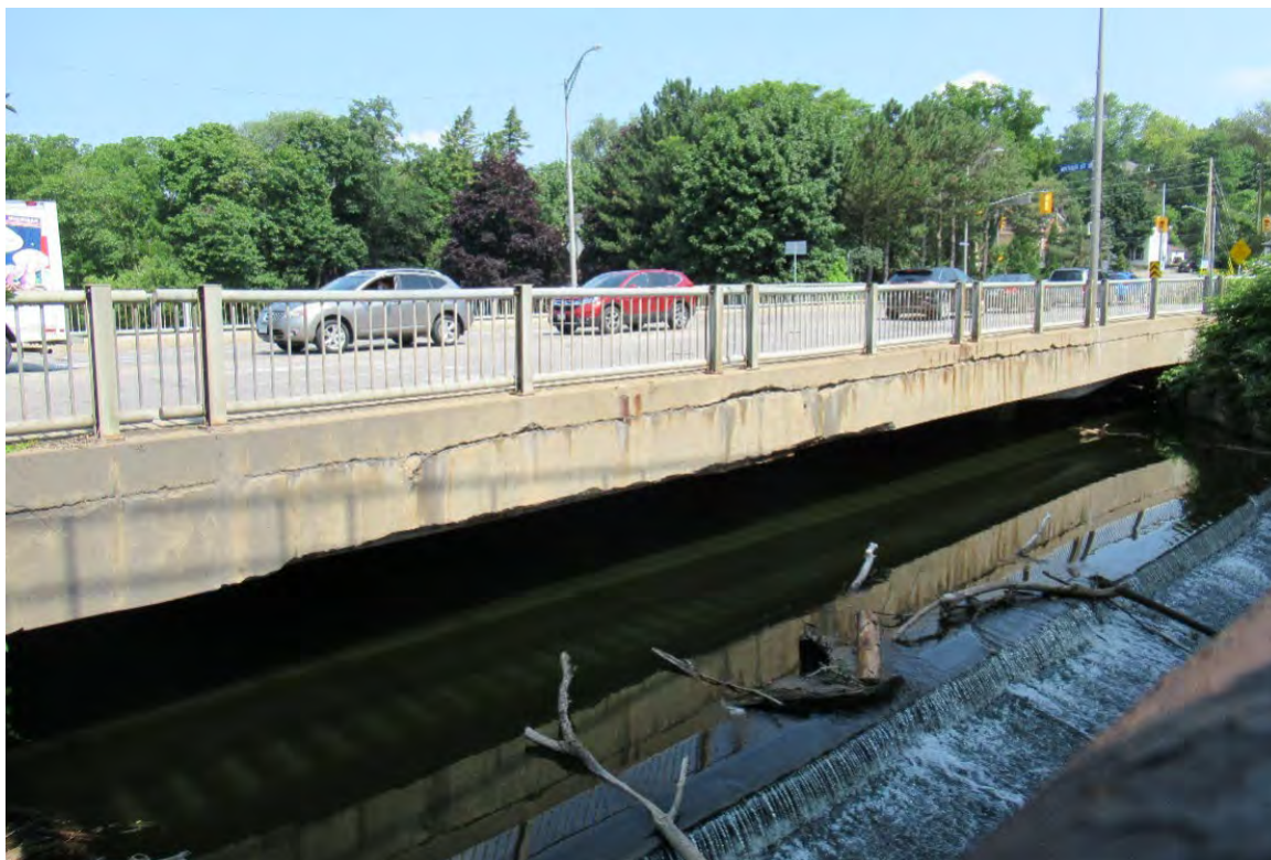
Exhibit3-2: Macdonell Bridge Aerial View
