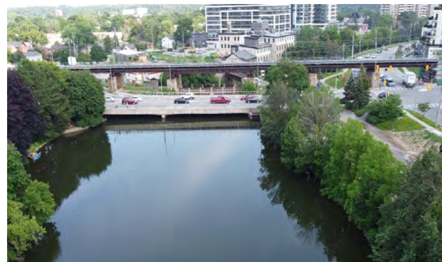
2a) Macdonell Bridge Aerial View
