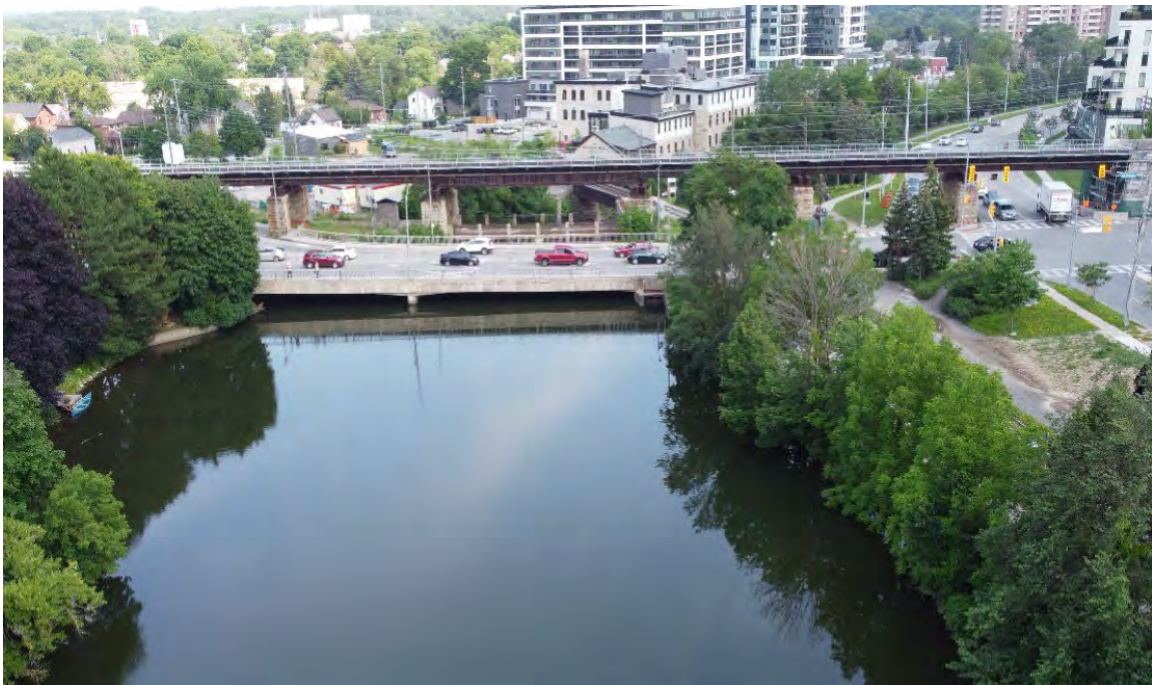
Exhibit 3-1: Macdonell Bridge Aerial View
