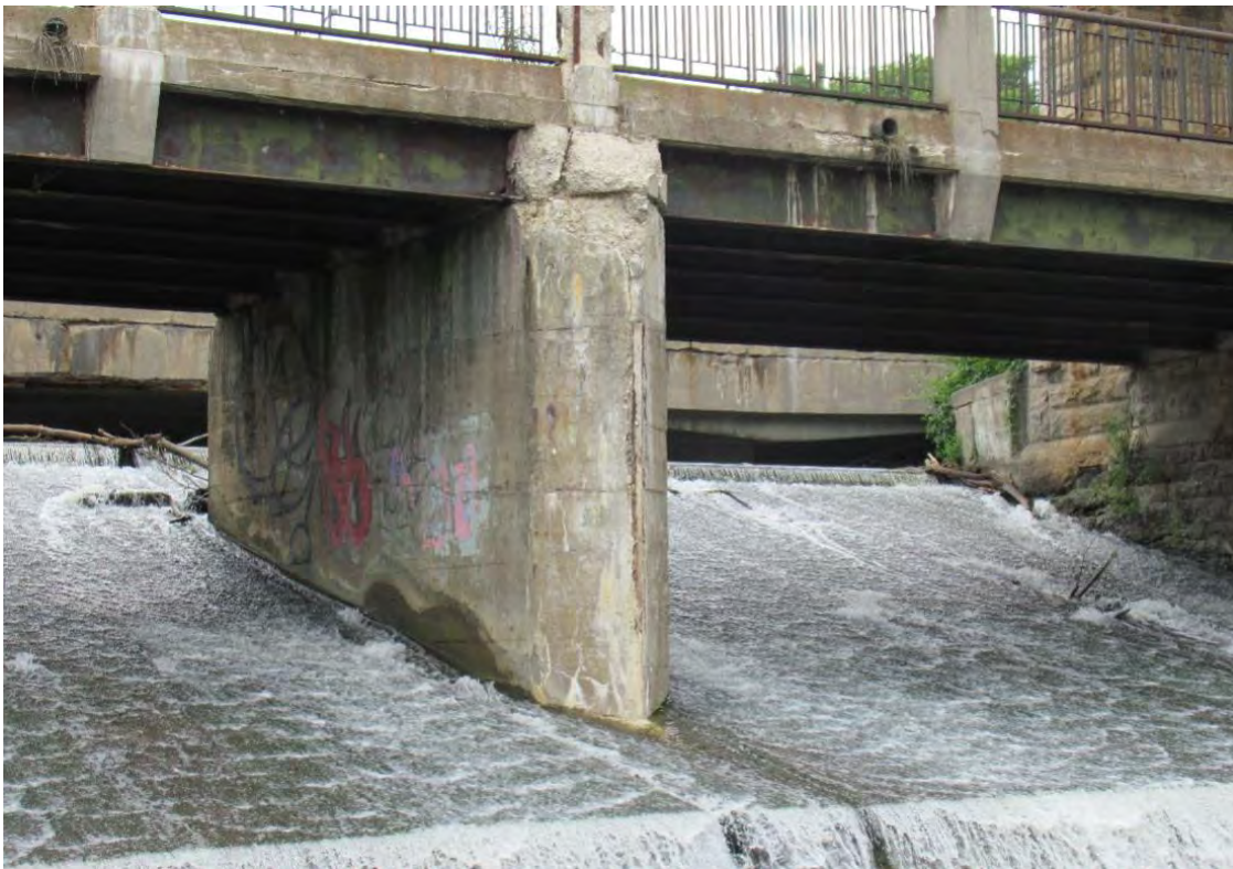
Exhibit 5-2: The spillway forms a weir to control the Speed River elevation, previously used for the now-removed Allan's Mill
