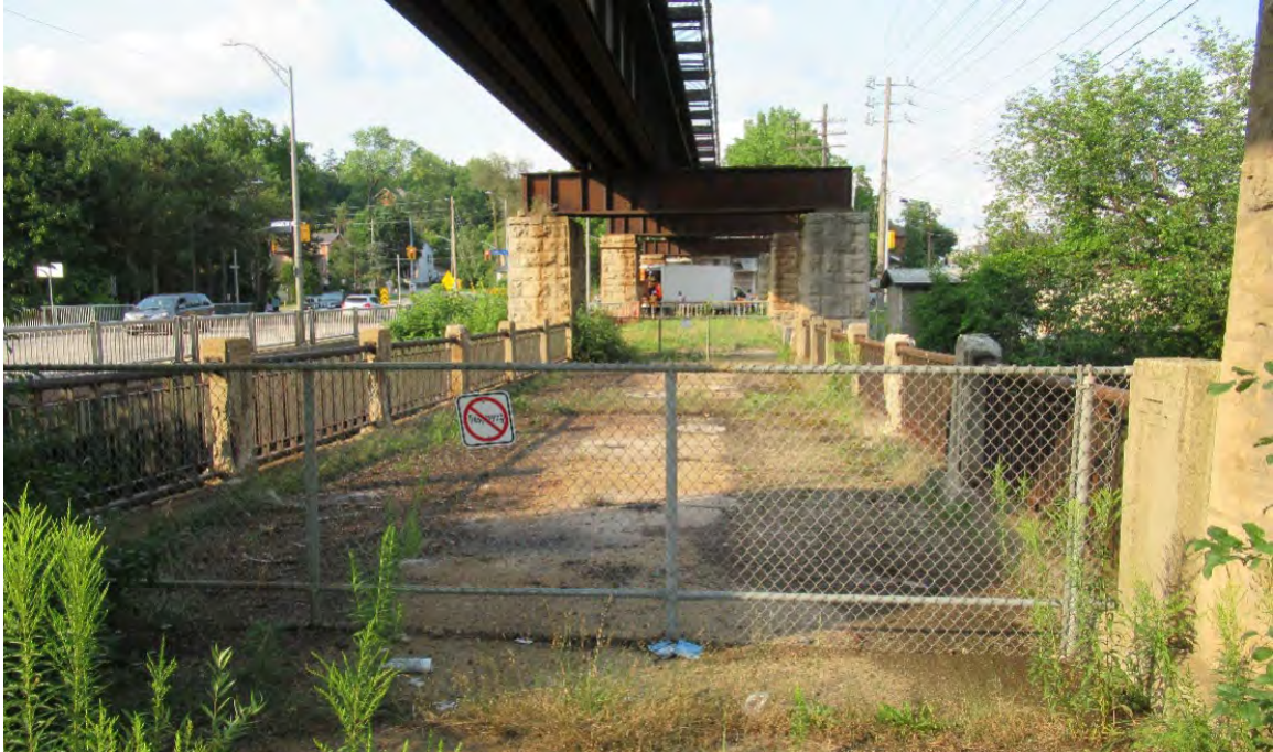
Exhibit 4-2: Allans Dam Bridge Closure
