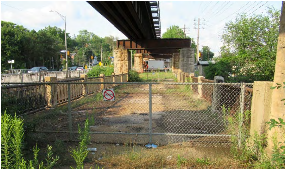
Exhibit 4-2: Allans Dam Bridge Closure
