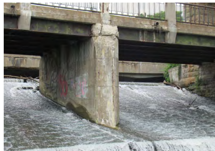
4b) The spillway forms a weir to control the Speed River elevation, previously used for the now-removed Allan's Mill.
