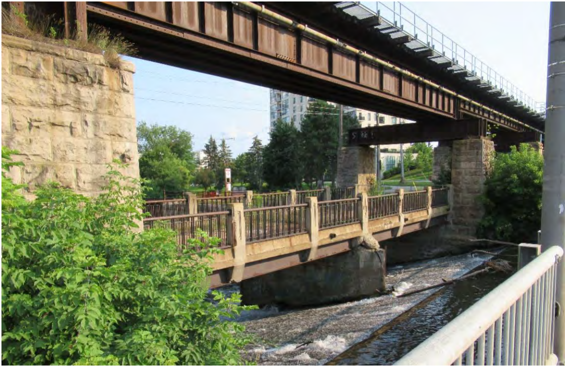
Exhibit 4-1: Allans Dam Bridge
