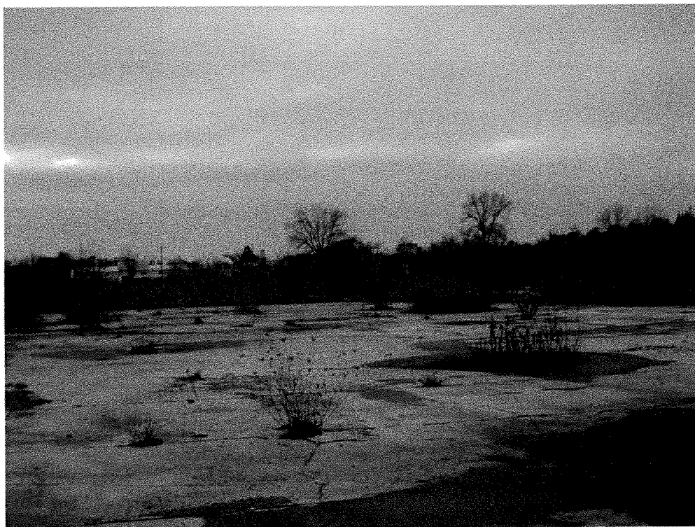
Photograph N° 1: Looking west from near east fence line. Note concrete floors left in place.
