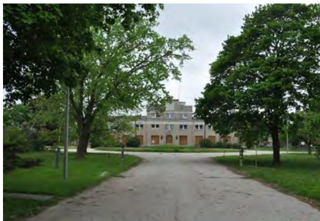
Image 41: View from drive to Administration Building
