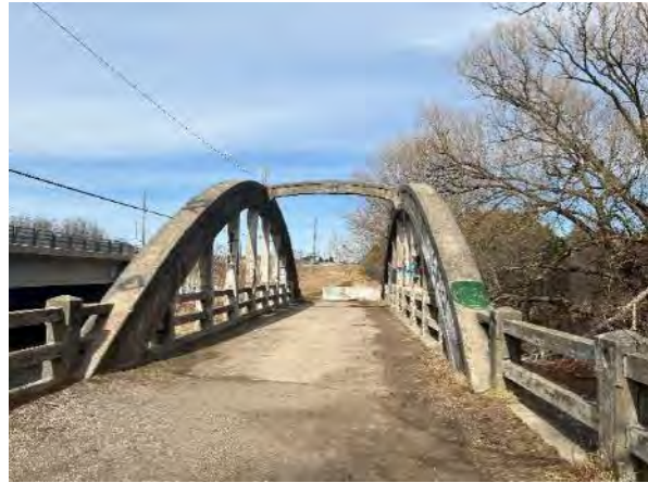
Image 101: McQuillan's Bridge, 1916 date of construction engraved on the cross brace
