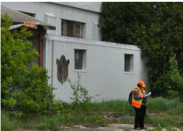
Image 70: Oil and Cement Shed
