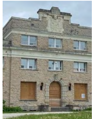
Image 44: Detail of the Administration Building
