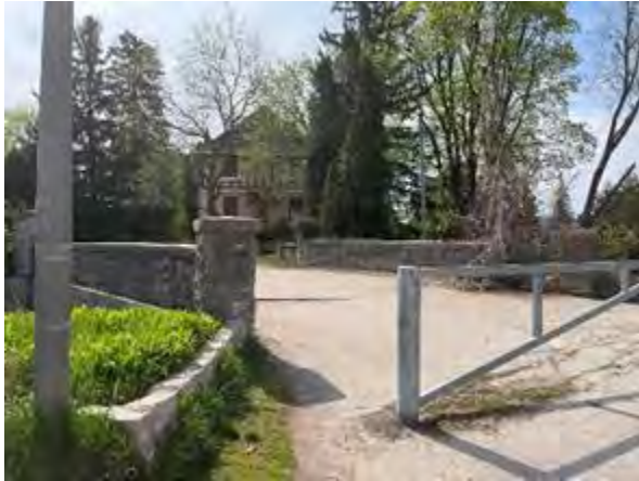
Image 31: Main Entry stone walls and bridge
