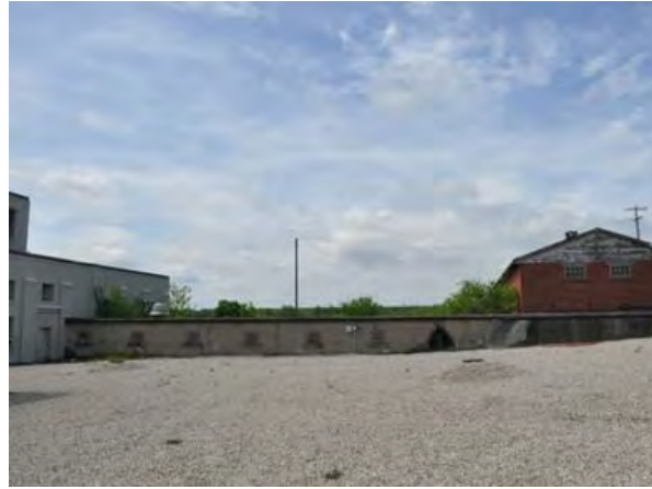
Image 67: Portion of the Powerhouse (left) connected by Tunnel to Cannery Storage (right)
