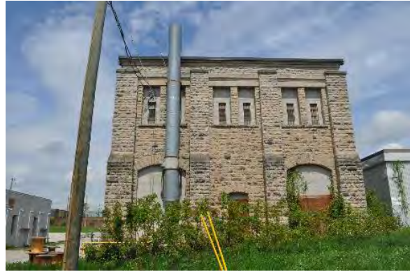
Image 61: Machine Shop south elevation
