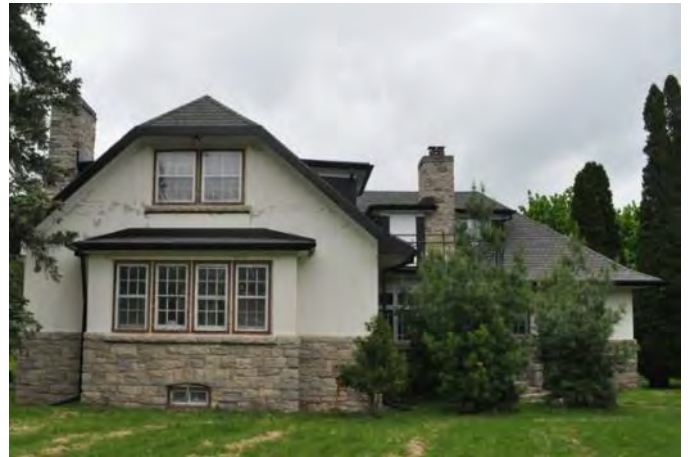
Image 38: Façade of former Superintendent's Residence
