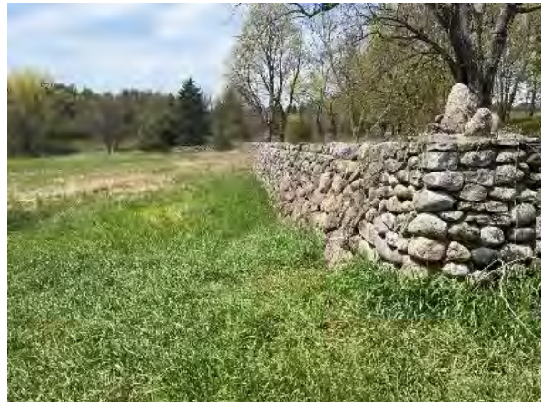
Image 85: Fieldstone retaining wall
