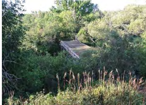
Image 103: View of CPR wood trestle bridge deck
