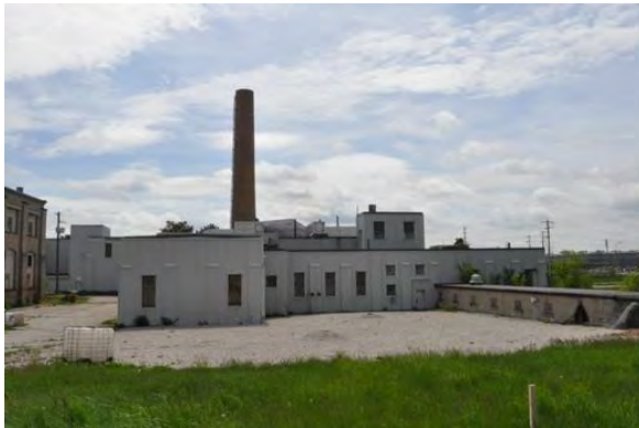
Image 62: Powerhouse and Chimney
