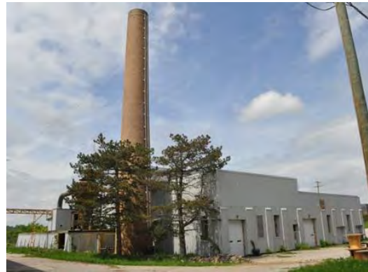
Image 63: Powerhouse and Chimney
