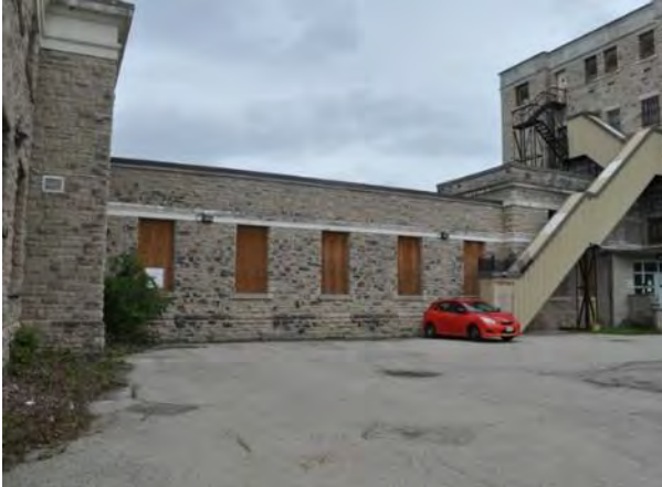
Image 47: Administration Building Corridor
