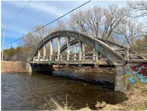
Image 100: McQuillan's Bridge, reinforced concrete bowstring arch truss construction
