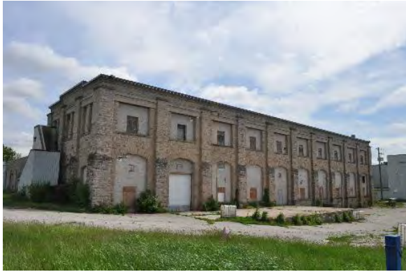
Image 60: Machine Shop façade (west elevation)
