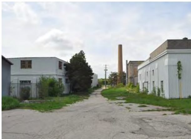
Image 64: Character Area C industrial buildings, road and Powerhouse Chimney Stack
