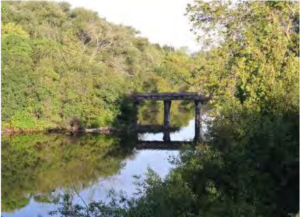
Image 102: CPR wood trestle bridge over the Eramosa River
