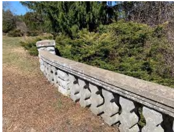
Image 35: Entry drive a (detail of concrete balustrade)
