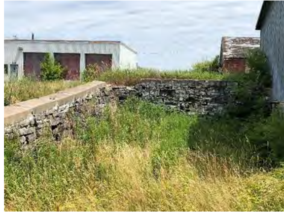
Image 59: Stone wall enclosure
