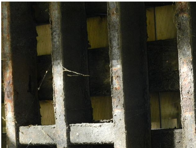
Underside Surface. Showing isolated medium corrosion.
