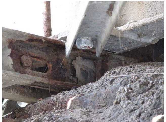
Underside Surface. Showing isolated severe corrosion.
