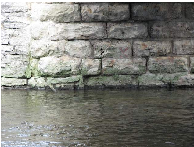
East Side. Showing isolated severe spalling.
