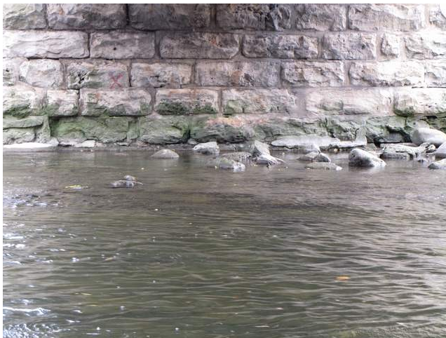
East Surface. Showing isolated severe deterioration.
