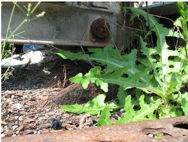
Bottom Surface. Showing extensive severe corrosion.
