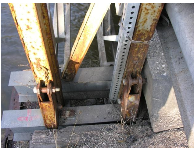
West End. Showing isolated severe corrosion.
