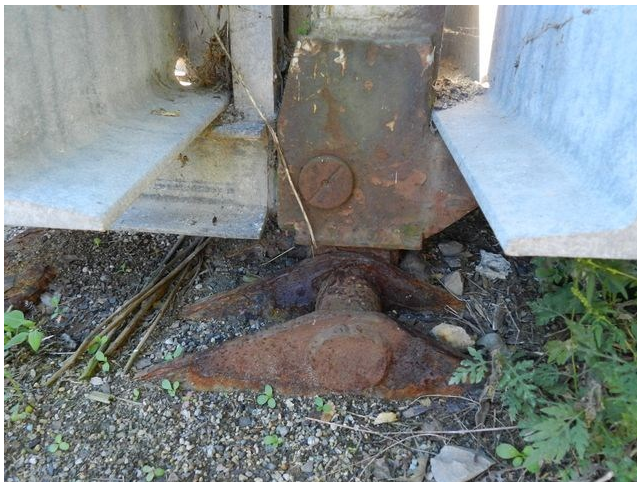
Overall View . Showing severe corrosion.
