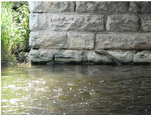
Bottom Surface. Showing isolated severe deterioration.
