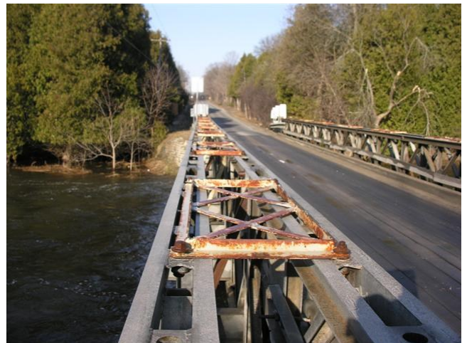
South Surface. Showing widespread medium corrosion
