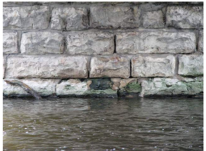
West Surface. Showing isolated severe deterioration.
