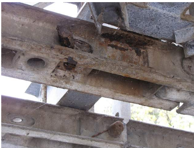
Underside View . Showing isolated severe corrosion.
