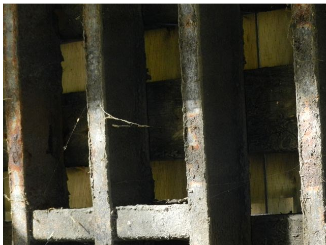
Underside Surface. Showing isolated medium corrosion.
