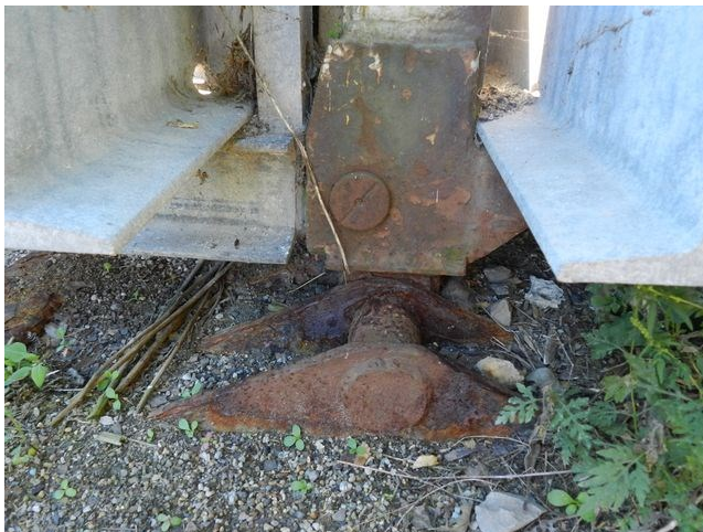
Overall View. Showing severe corrosion.
