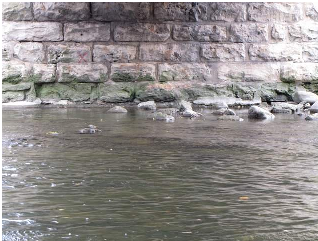
East Side. Showing isolated severe spalling.
