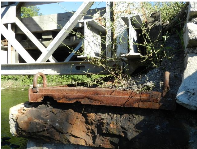
East Side. Showing severe corrosion.
