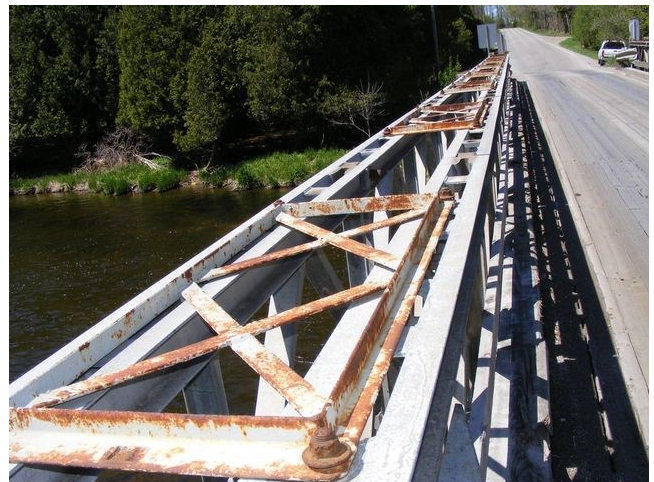
South Surface. Showing widespread medium corrosion
