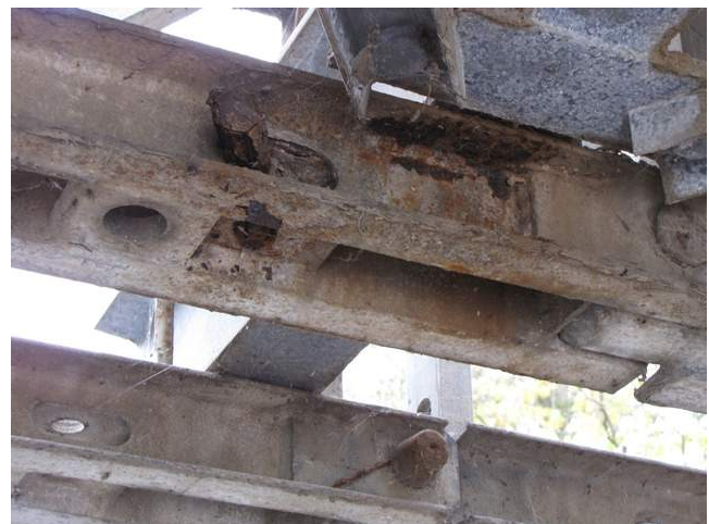
Underside View. Showing isolated severe corrosion.
