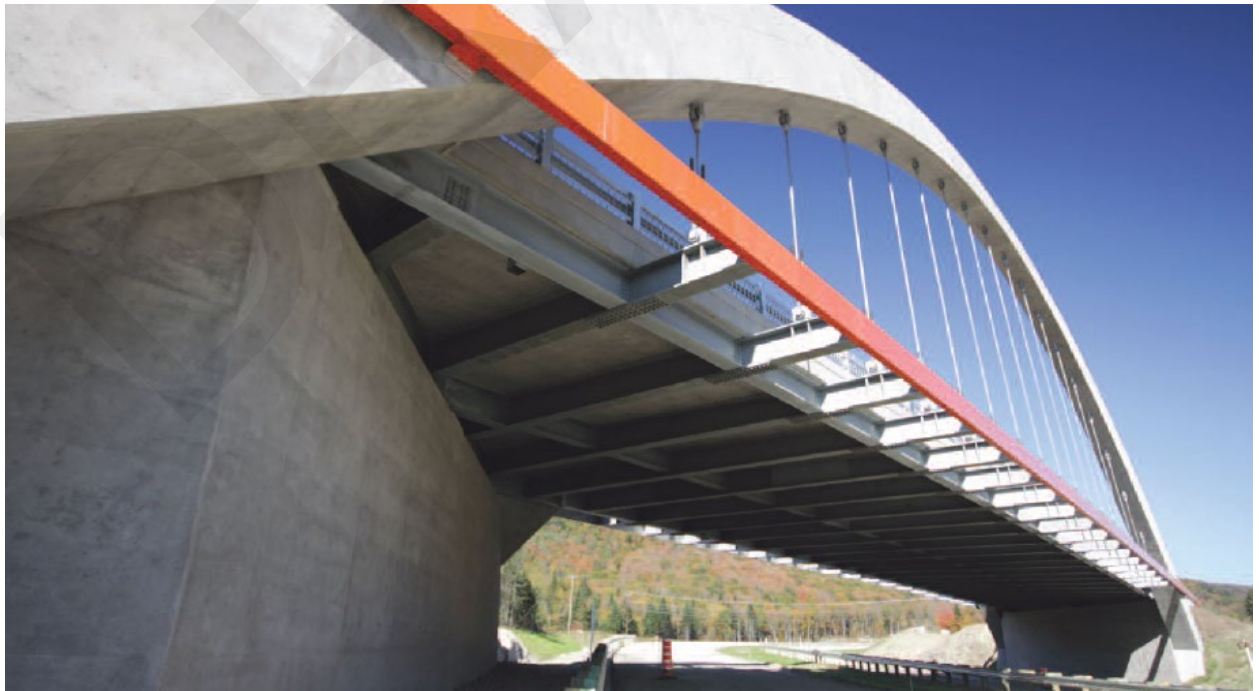
Figure 6.3: Arch Bridge in Stoneham Quebec (Photo from "2012 Consulting Engineering Awards")
