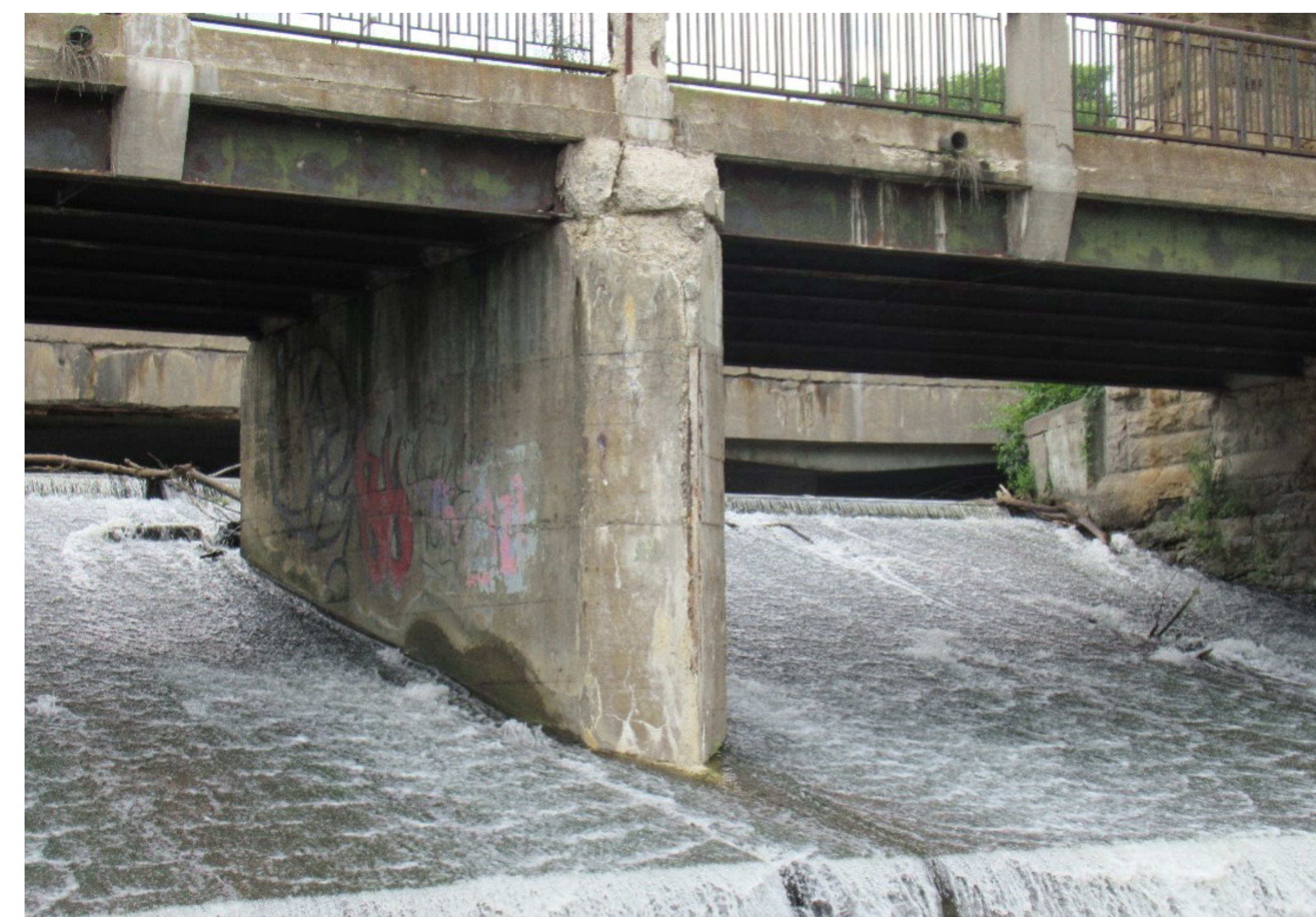
23b) The spillway forms a weir to control the Speed River elevation, previously used for the now-removed Allan's Mill.
