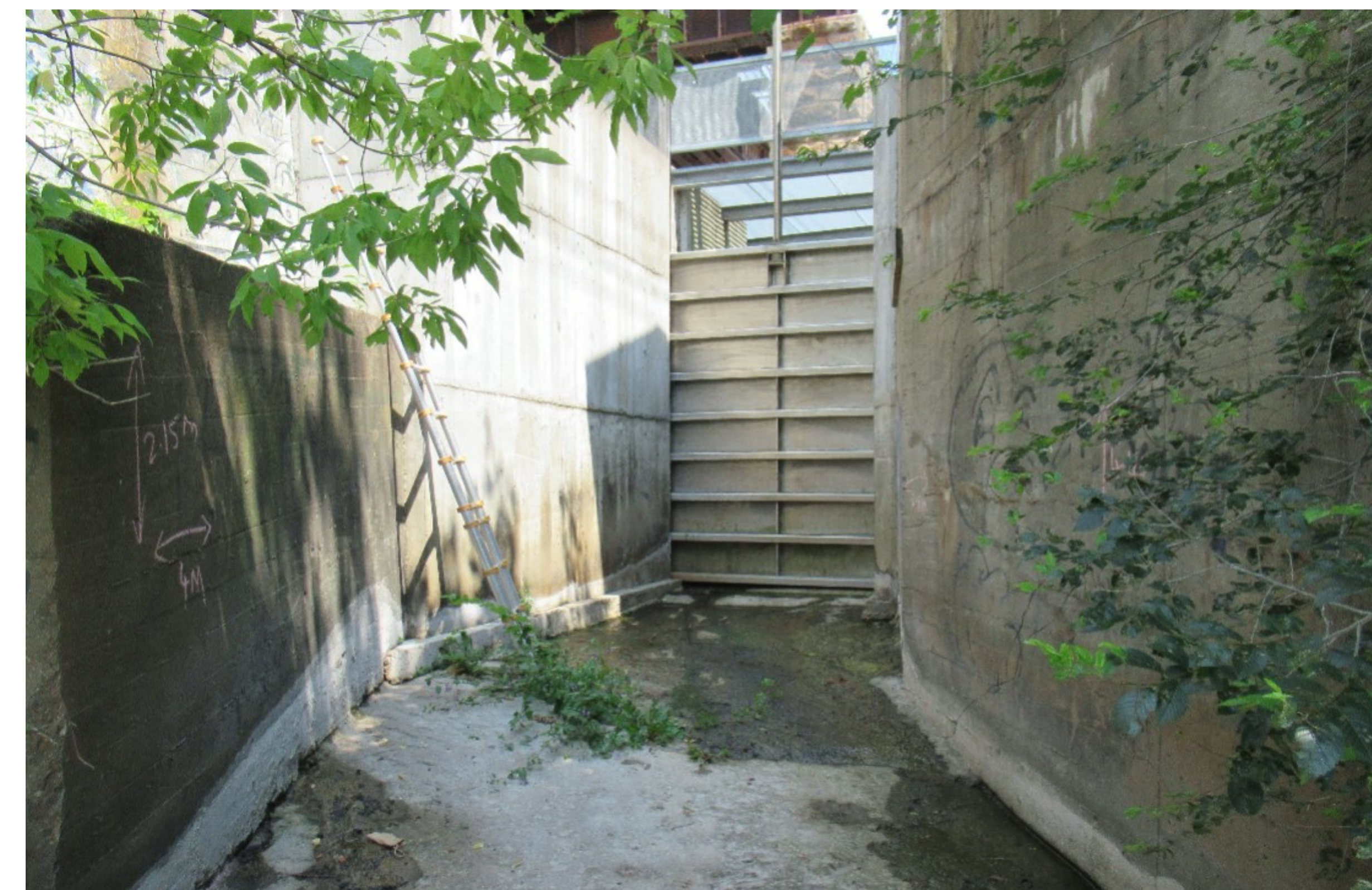
23a) The sluiceway is a concrete channel with a metal gate to carry excess water.
