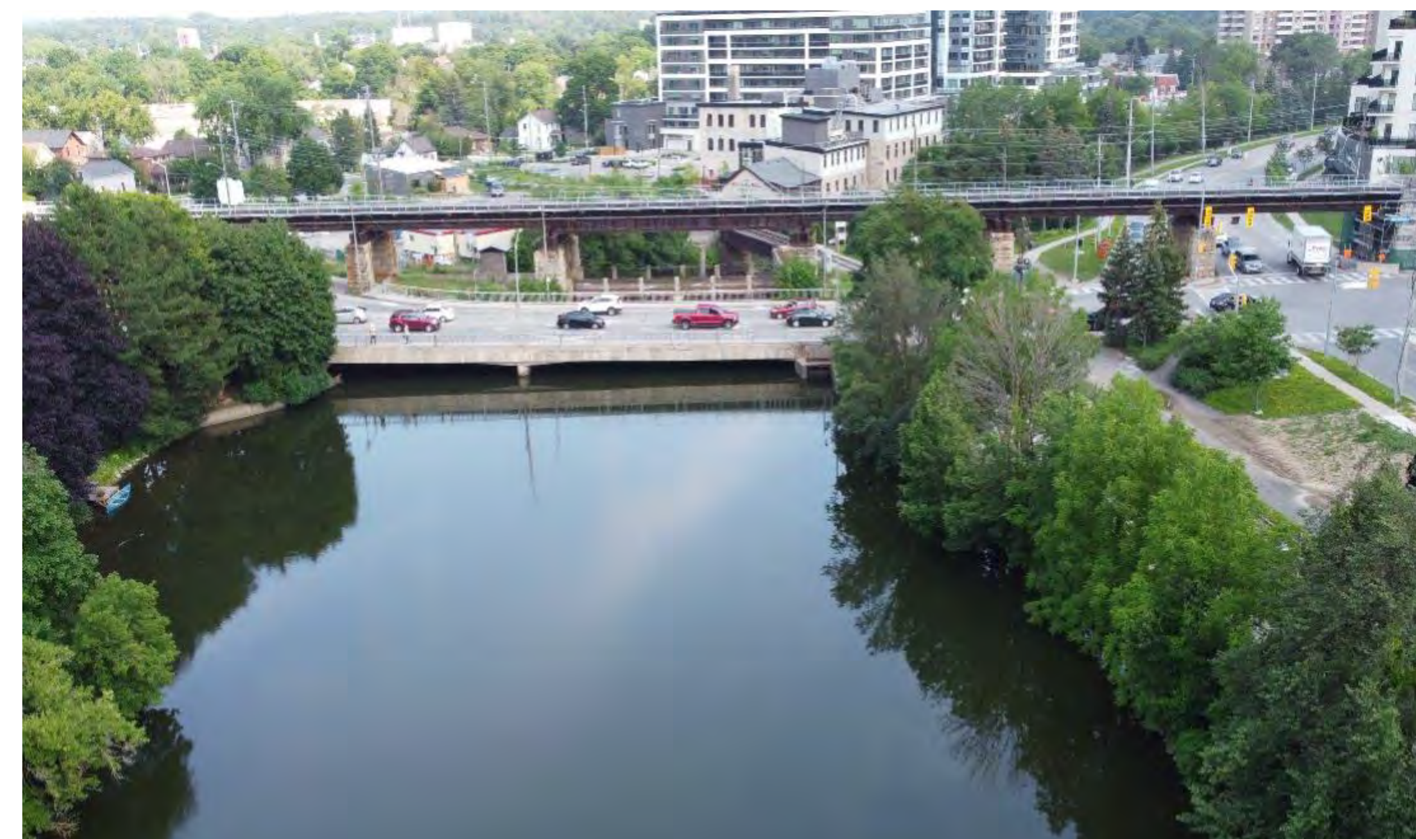
21a) Macdonell Bridge Aerial View
