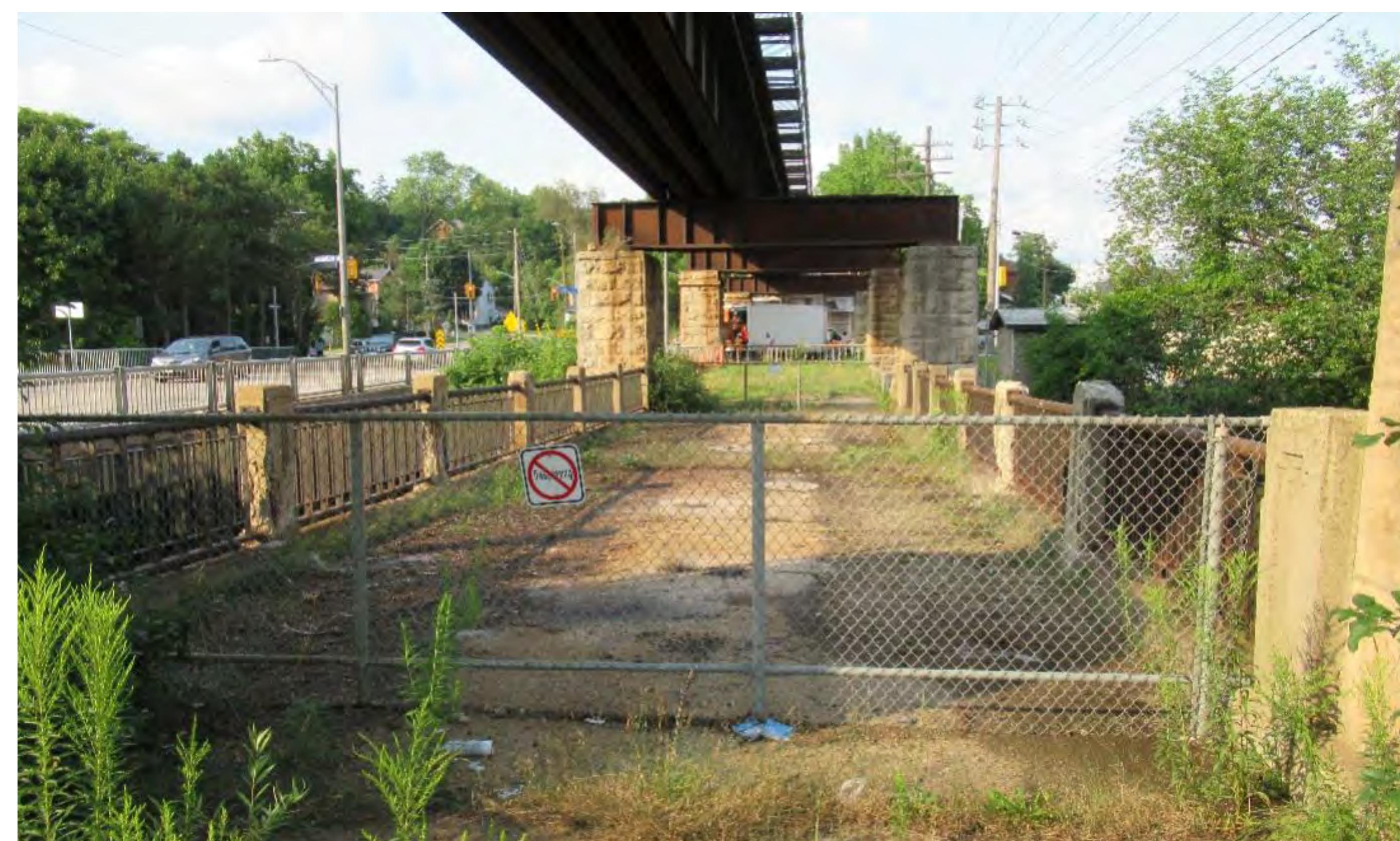
22b) Allans Dam Bridge Closure
