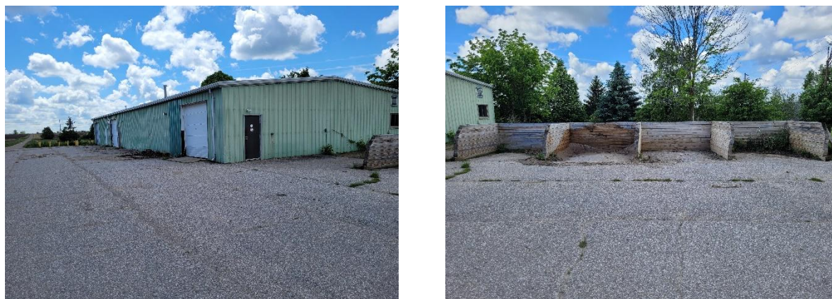
Figures 43 & 44: (left) View of contemporary steel accessory structure, (right) View of compost and soil sorting area, (MHBC, 2022)
