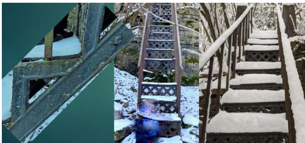
Figure 36: Photographs of iron stairs which were identified by the Heritage Guelph Designation Working Group. (Source: Heritage Guelph, n.d.)
