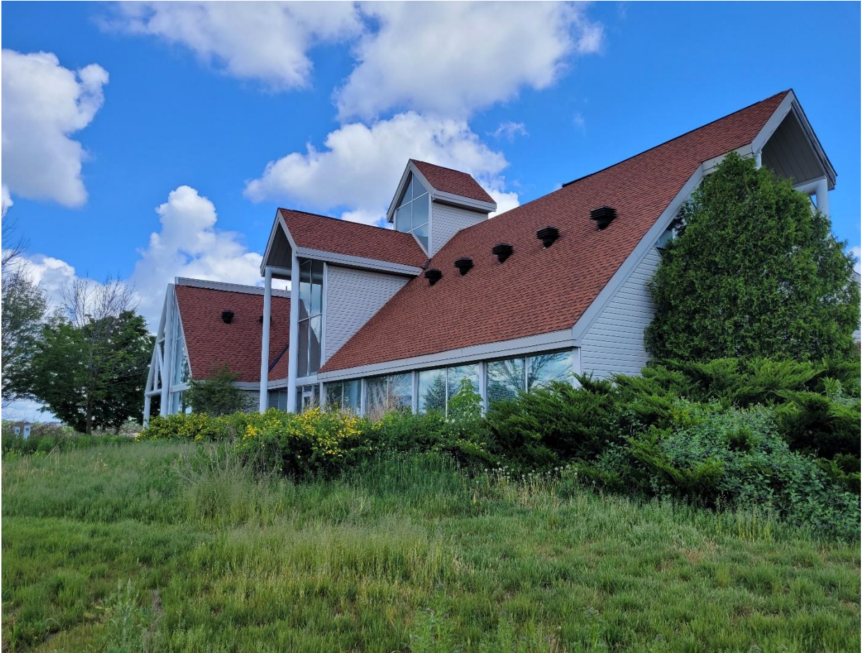
Figure 24: View of Guelph Turfgrass Institute former G.M. Frost building (south and west elevations). (Source: MHBC, 2022)
