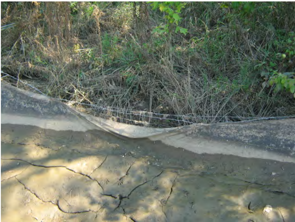
Photo 3: Fencing along south edge of stockpile area failing as a result of excess topsoil
