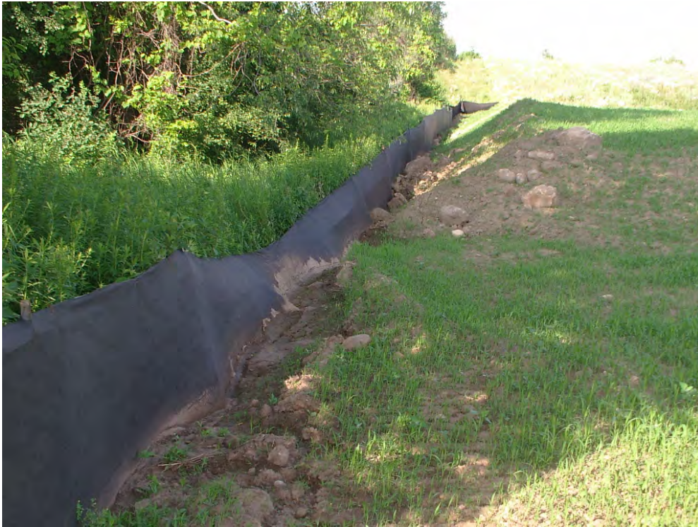
Photo 3: Accumulation of topsoil against southern edge of silt fence in stockpile area
