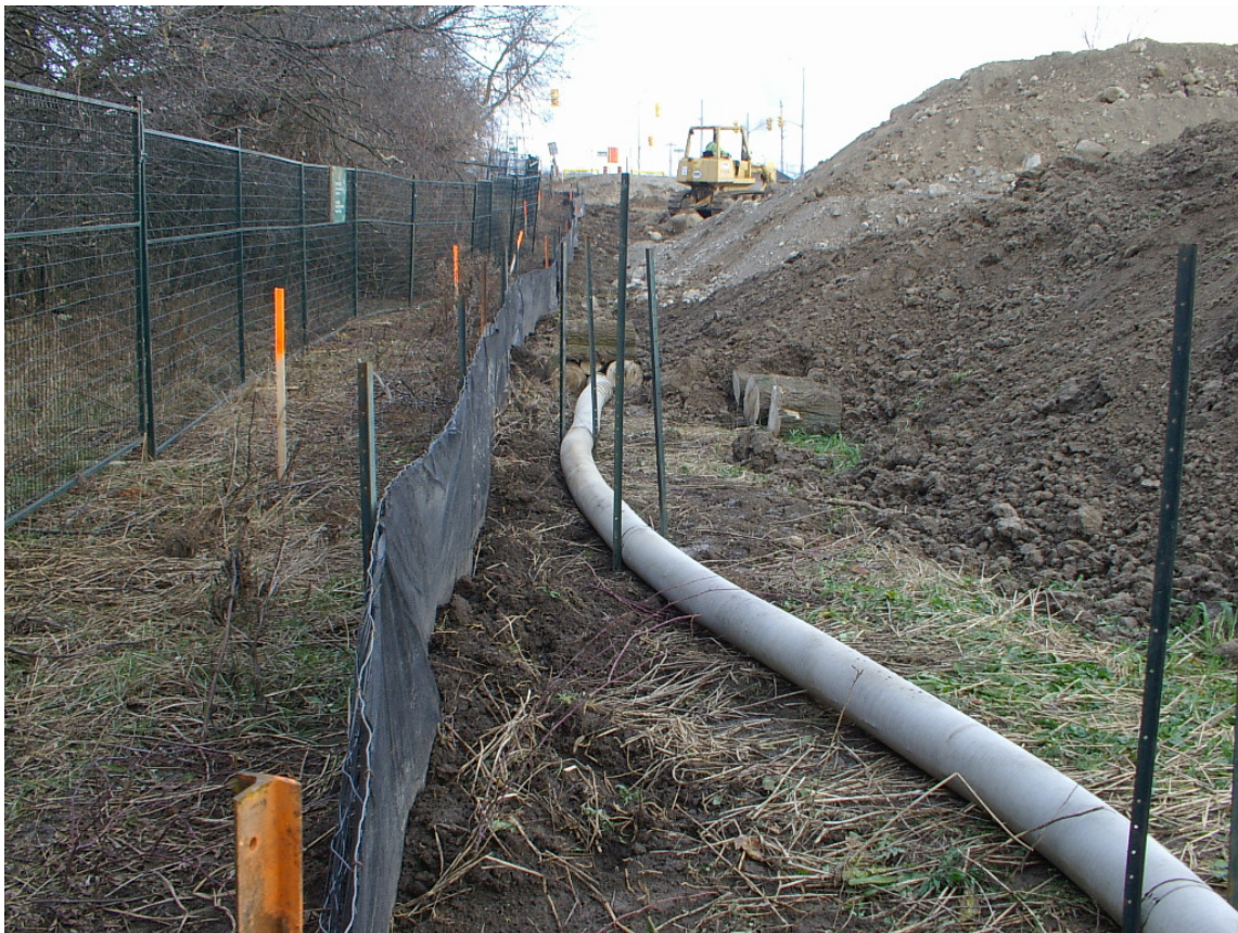
Photo 2: Heavy-duty silt fencing along north edge of work area
