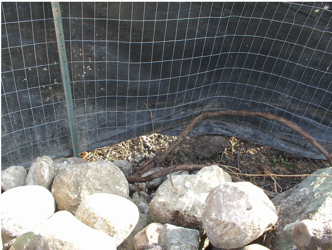
Photo 4: Small section of heavy-duty silt fencing in northeast corner not keyed in
