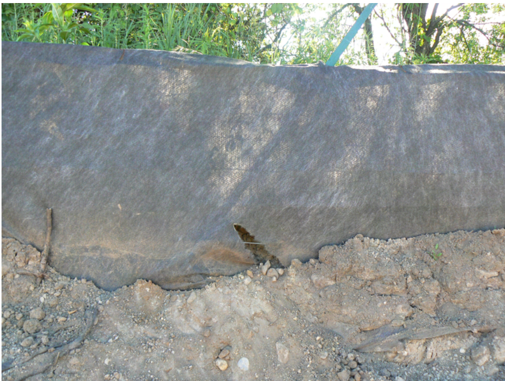
Photo 1: Small tear in ESC fence along west edge of fill borrow area
