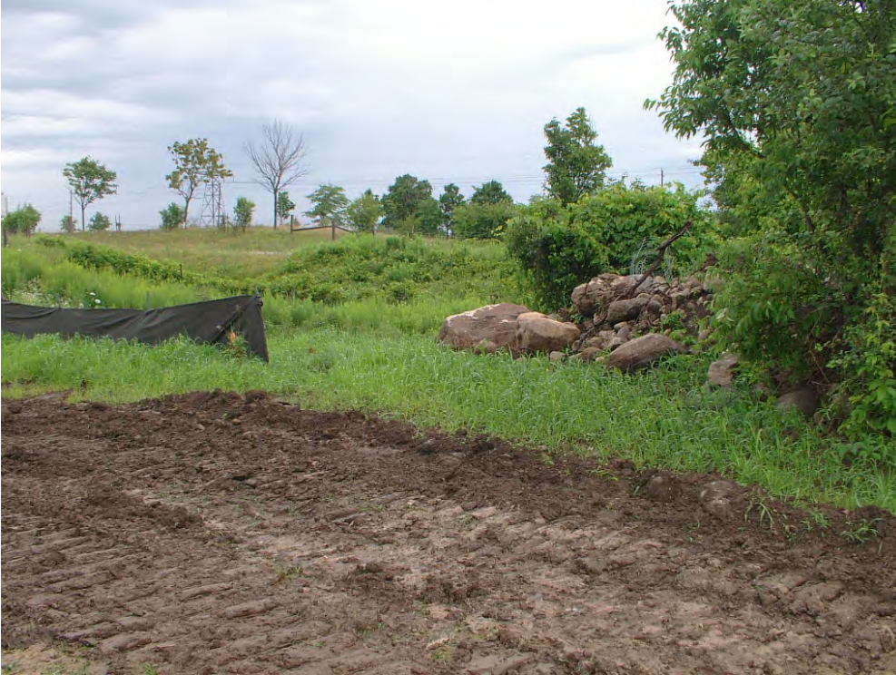
Photo 1: East side of access to stockpile along hedgerow missing silt fencing
