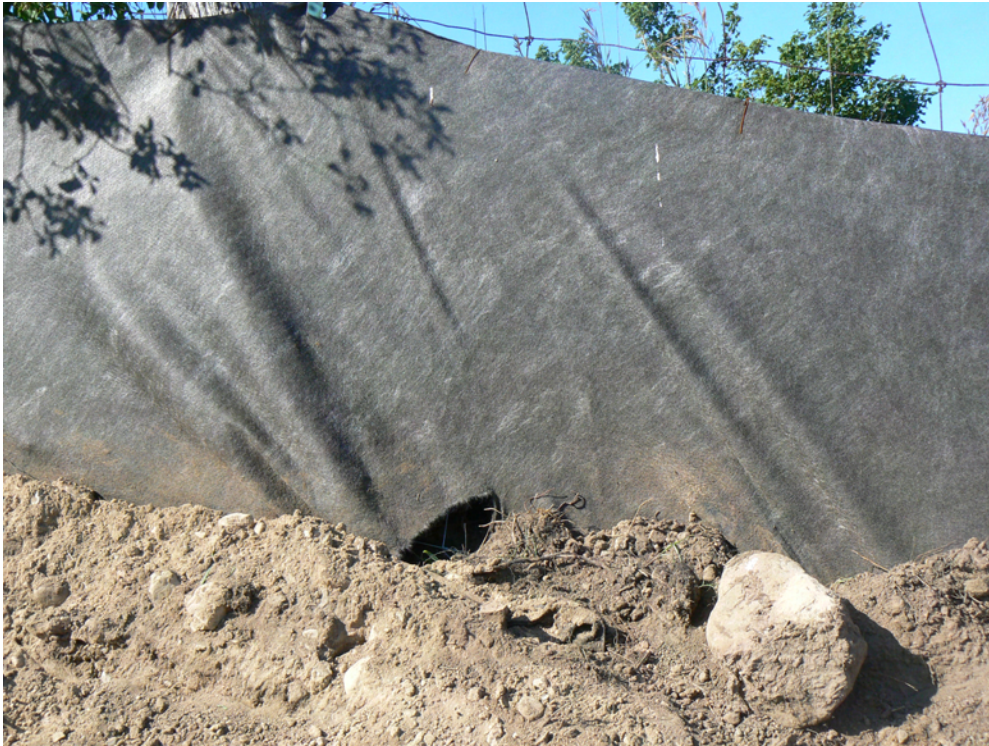
Photo 3: Tear in ESC fence in northeast corner of fill borrow area
