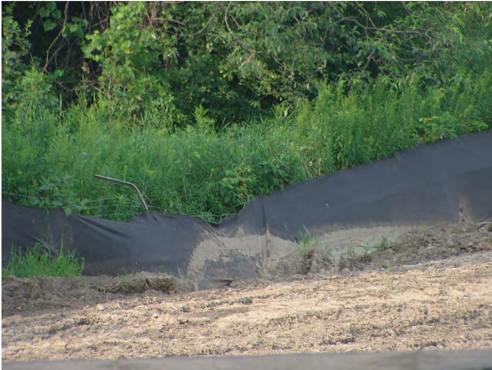
Photo 5: Slumping in fence along southern edge of stockpile area
