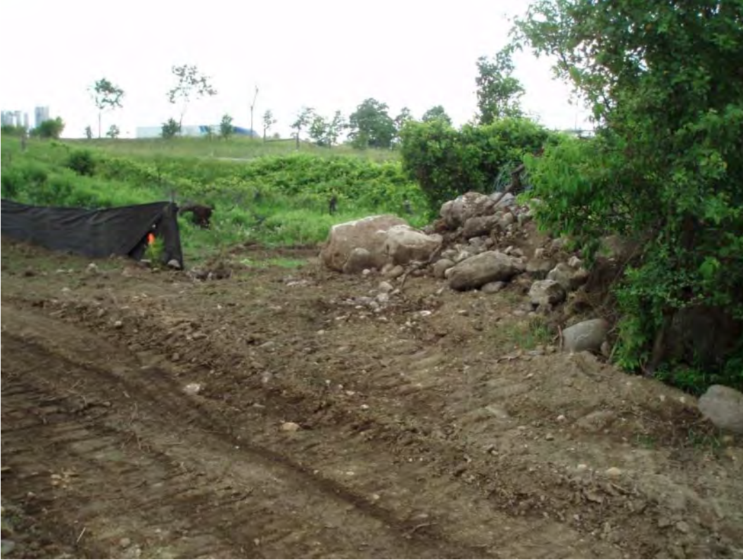
Photo 3: West side of access in hedge row missing silt fence
