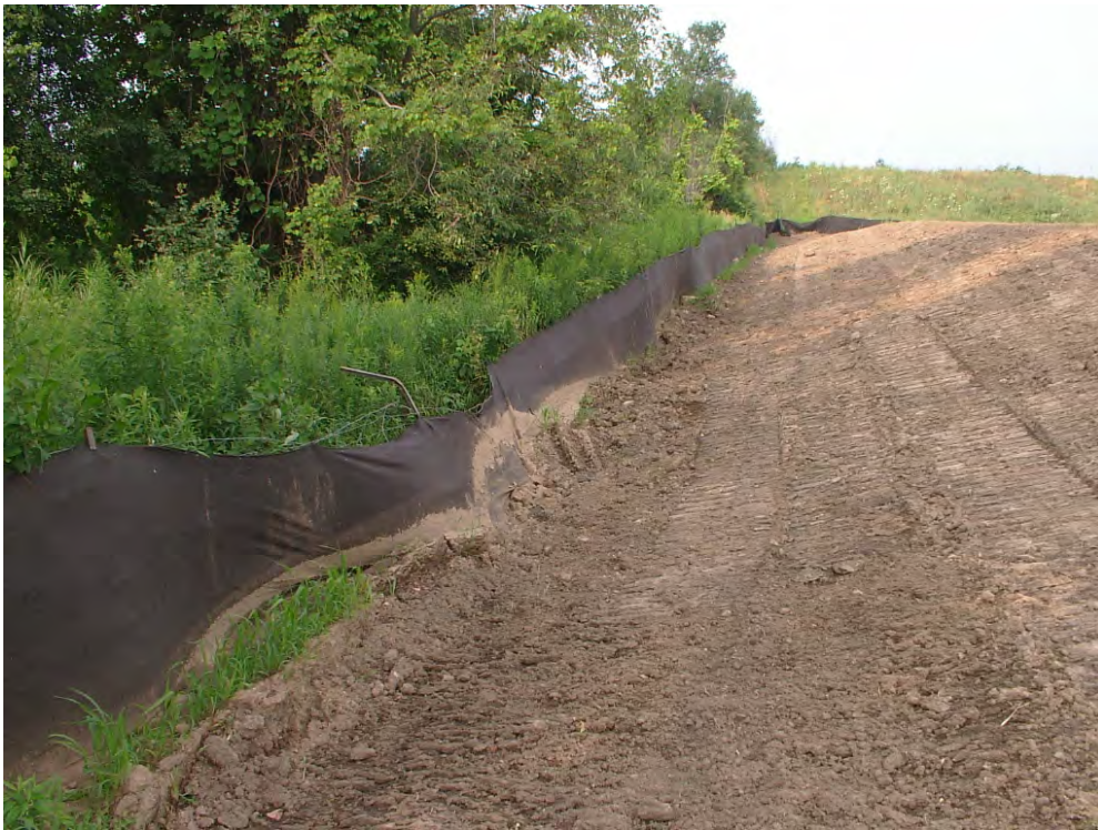
Photo 4: Southern edge of stockpile area that experienced accumulation of topsoil
