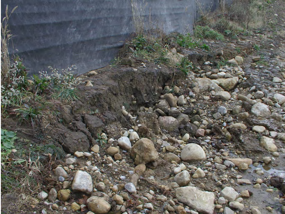
Photo 3: Erosion along slope due to Phelan Drive culvert
