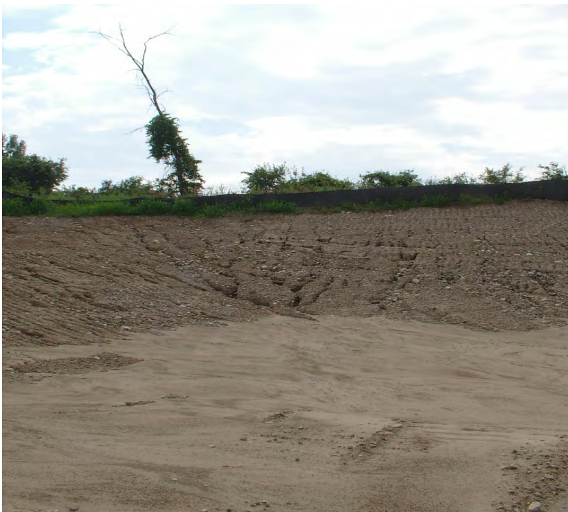
Photo 2: Gullying in southwest corner of fill borrow area
