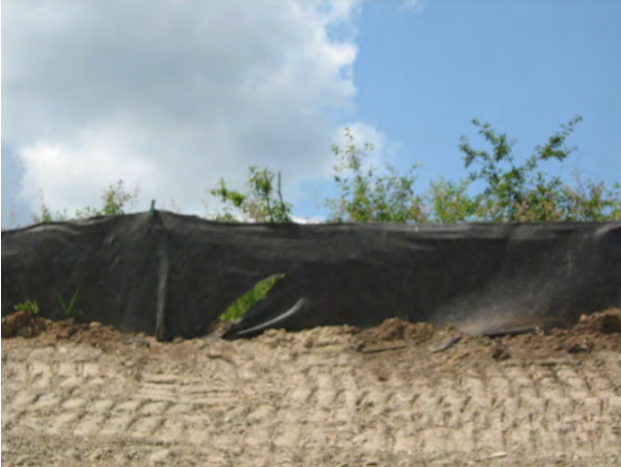
Photo 1. 1 of 2 tears in silt-fencing along western edge of borrow pit
