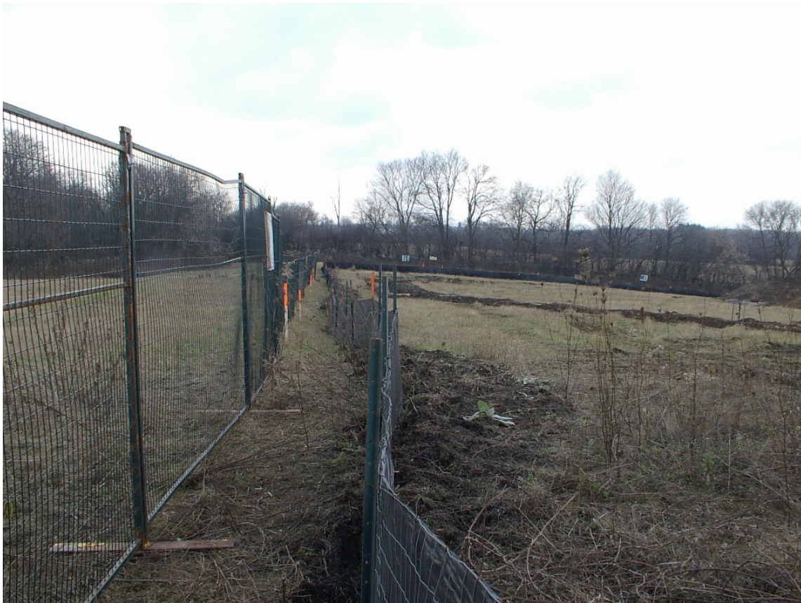
Photo 1: Heavy-duty silt fencing along south edge of work area
