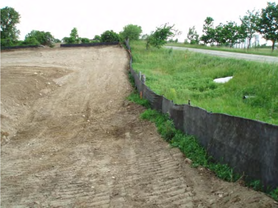
Photo 1: Heavy duty silt fencing keyed in and installed as per design
