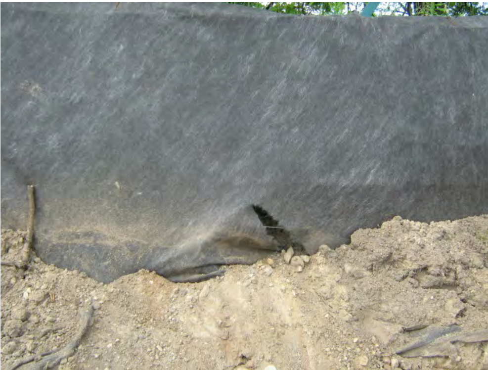
Photo 2: Second tear in silt fence along west edge of fill borrow area
