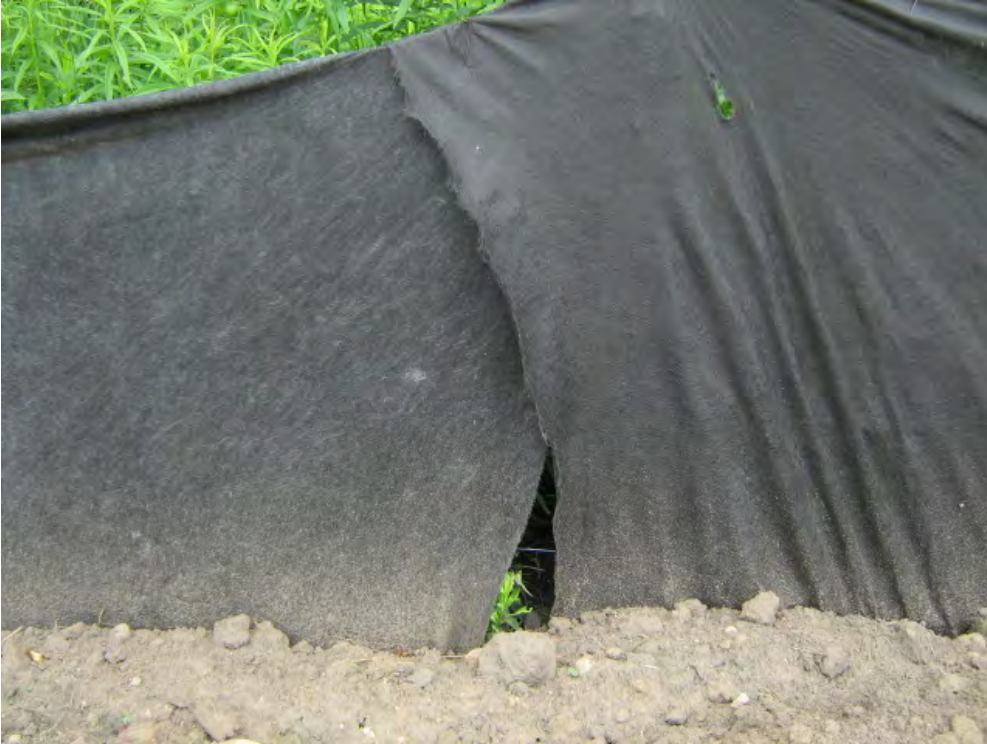
Photo 3: Separation in silt fence along north edge of fill borrow area
