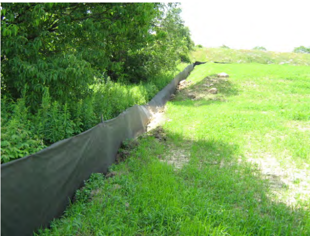
Photo 3. Accumulation of topsoil against southern edge of silt fence in stockpile area
