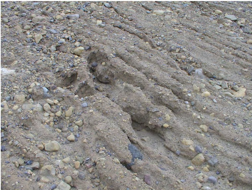
Photo 2: Gully along fill borrow side slopes
