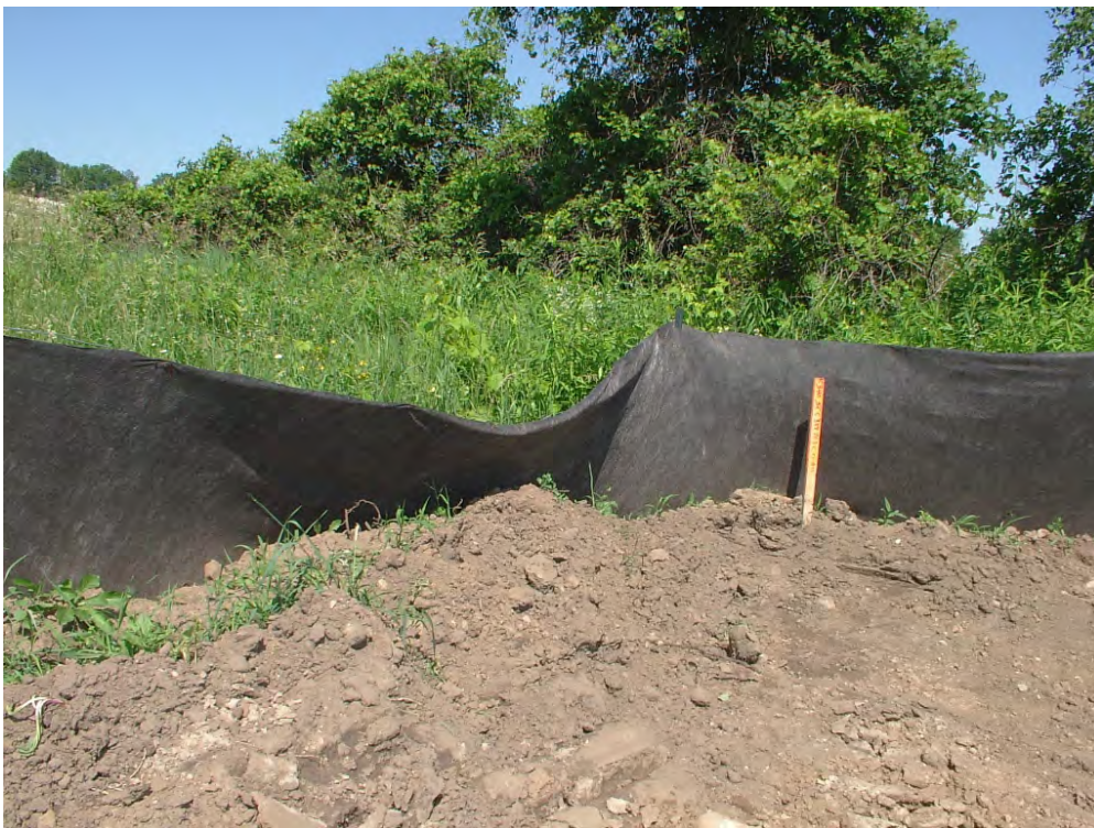
Photo 4: Slight slumping in silt fence in northwest corner of fill borrow area
