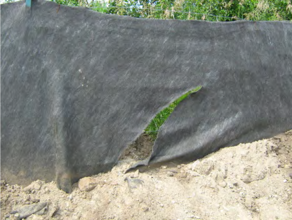
Photo 1: Tear in silt fence along west edge of fill borrow area
