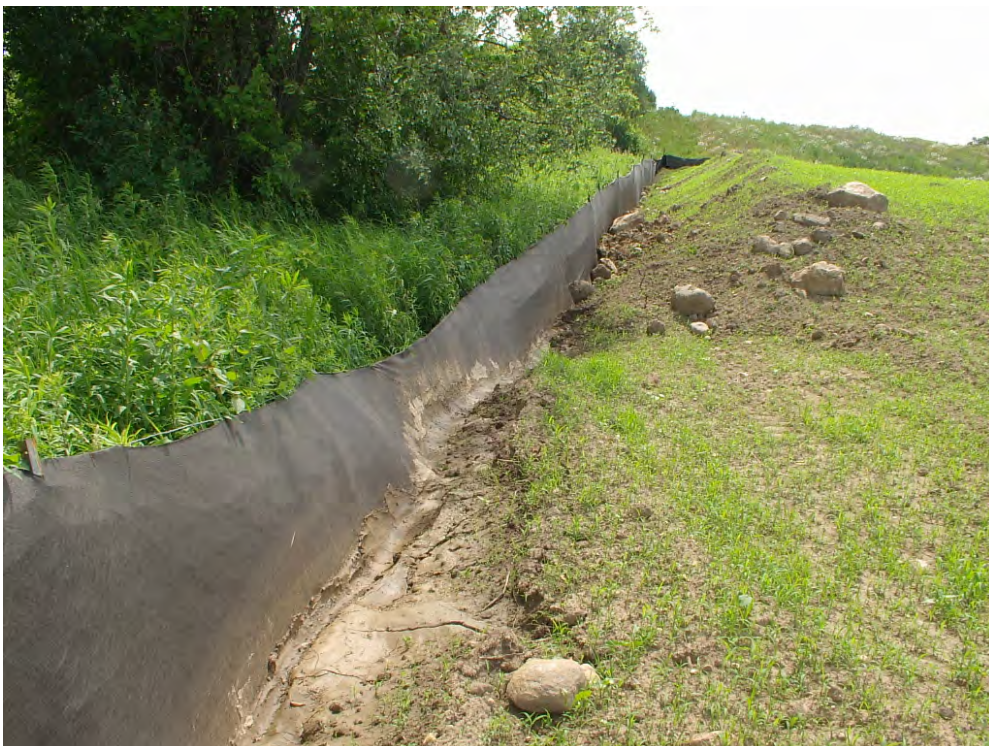
Photo 4: Accumulation of topsoil against southern edge of silt fence in stockpile area
