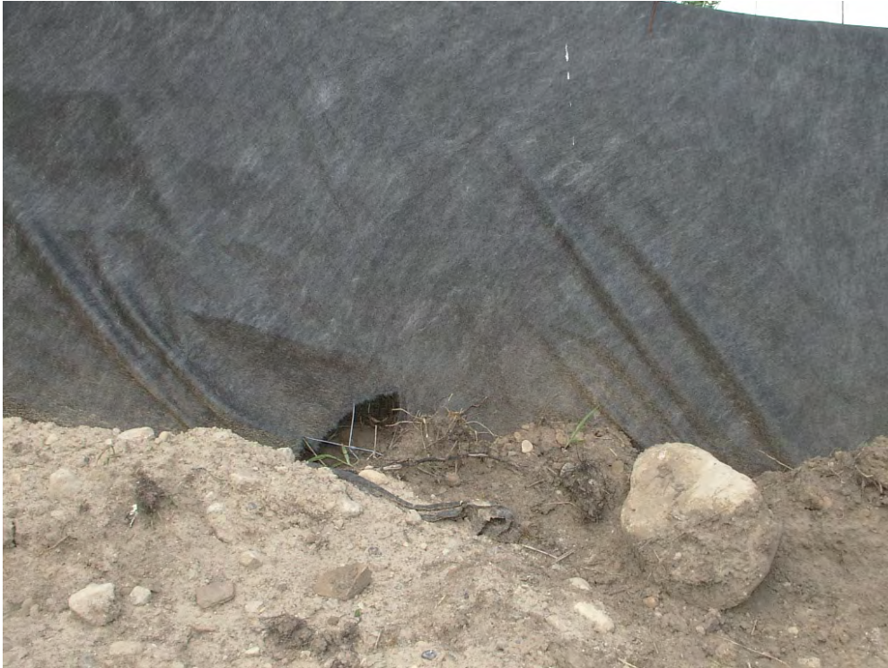
Photo 1: Small tear in ESC fence along east edge of fill borrow area
