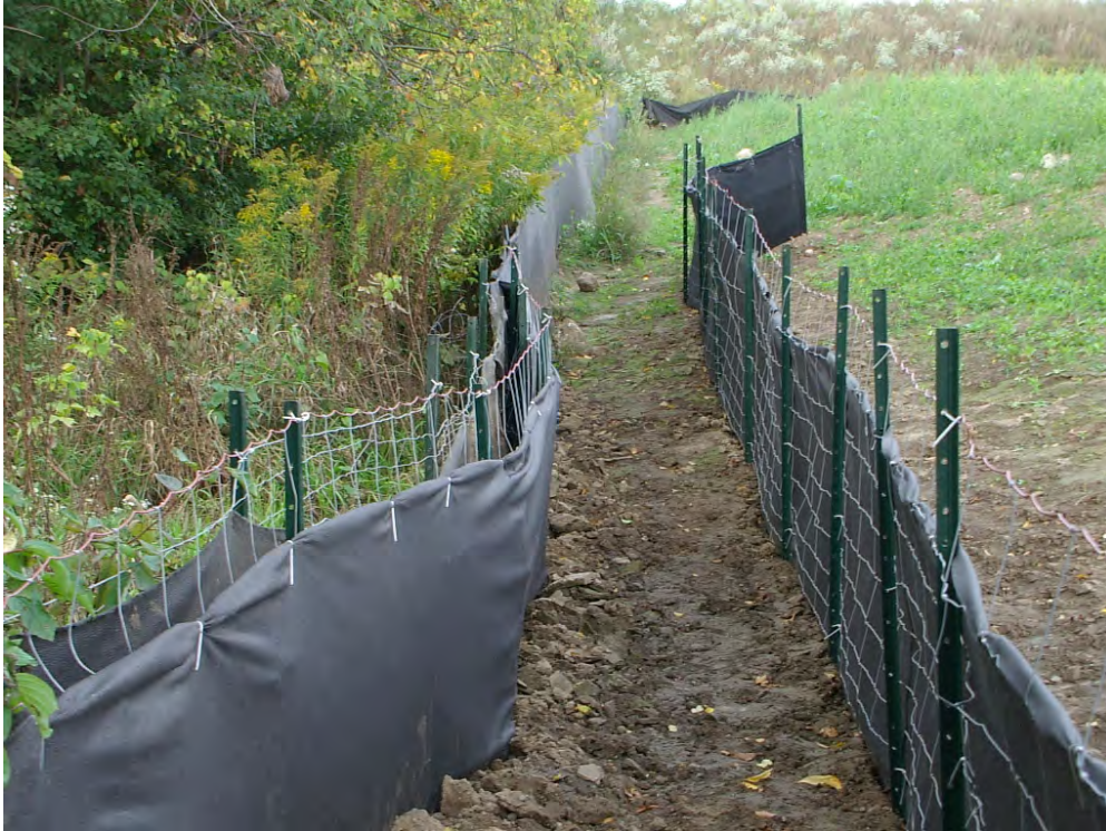
Photo 3: Reinforced fencing along south edge of stockpile area
