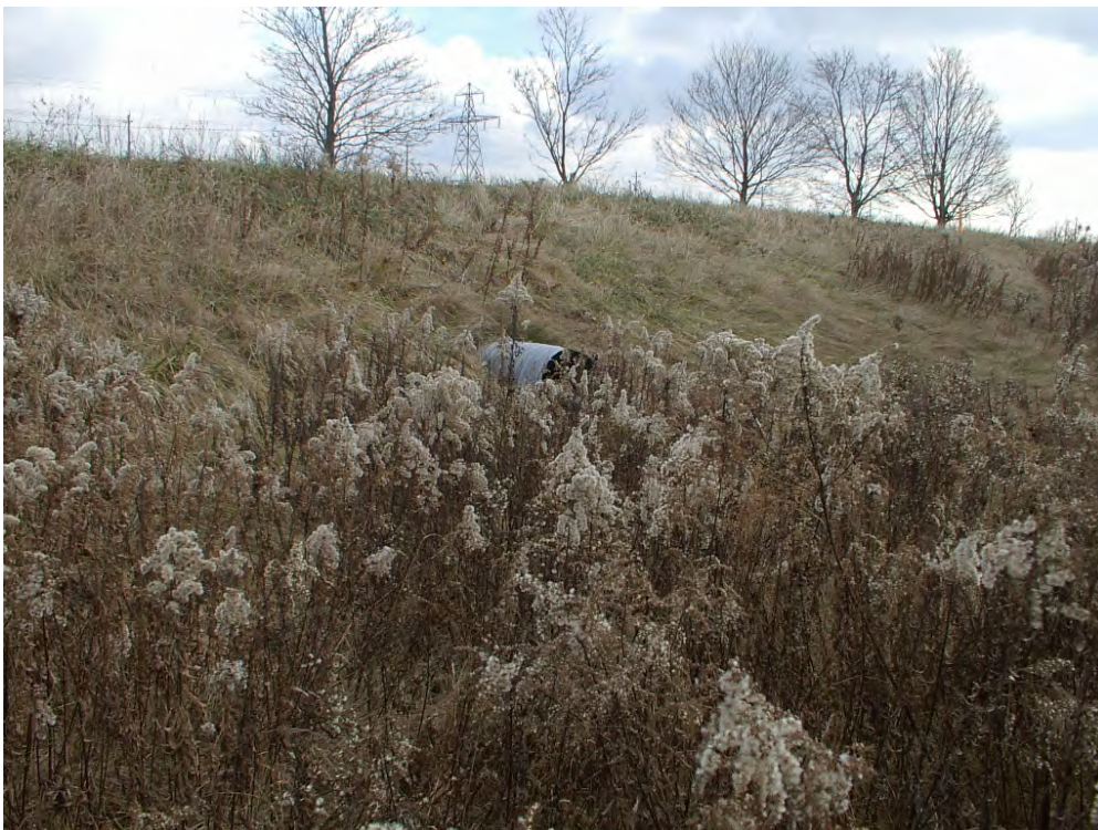
Photo 2: Culvert adjacent to Phelan Drive that is draining into fill borrow area
