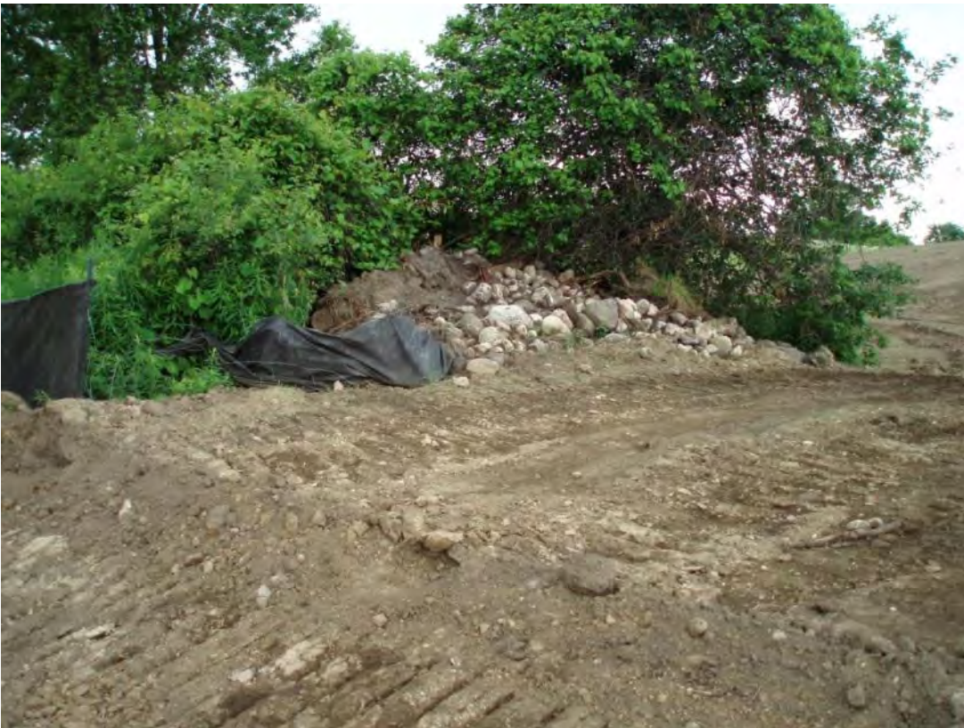
Photo 4: East side of access to stockpile along hedgerow missing silt fencing
