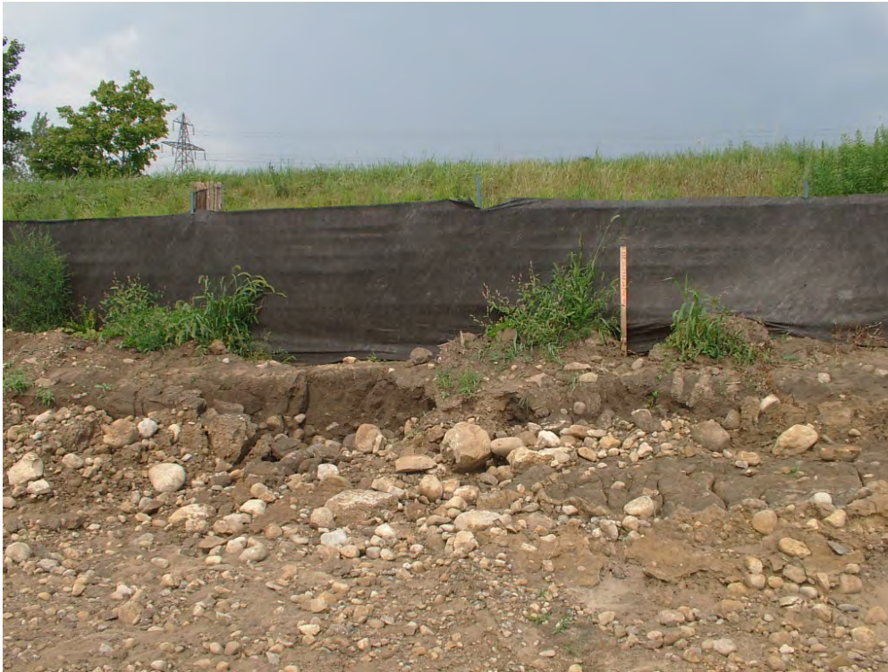
Photo 3: Un-keyed silt fence along east side of fill borrow area
