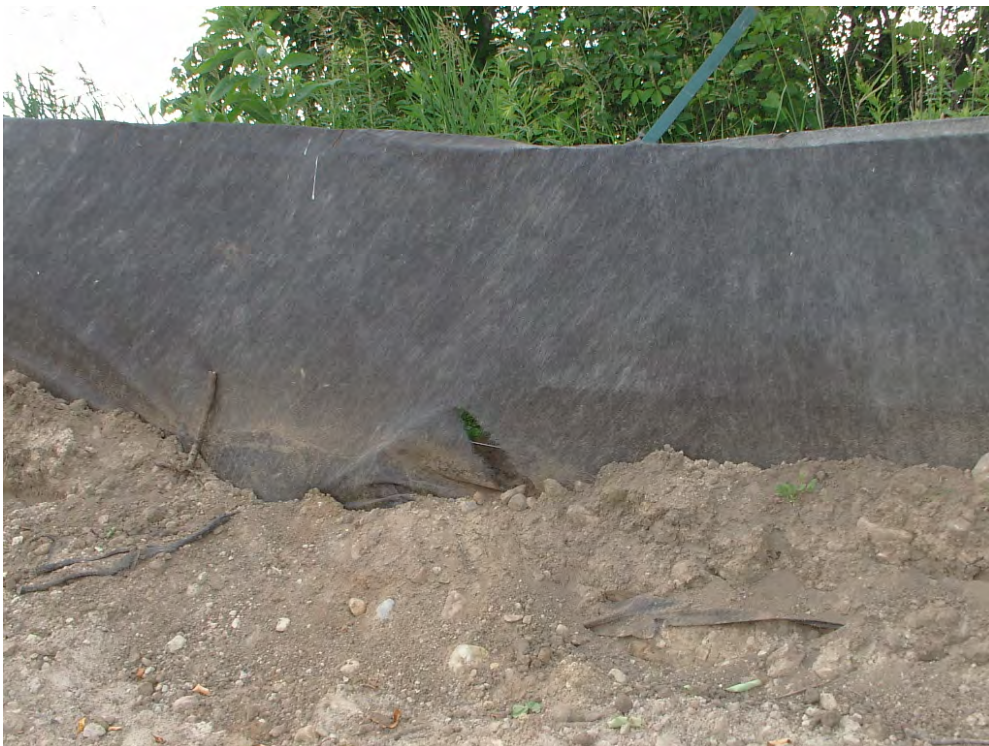
Photo 2: Small tear in ESC fence along west edge of fill borrow area
