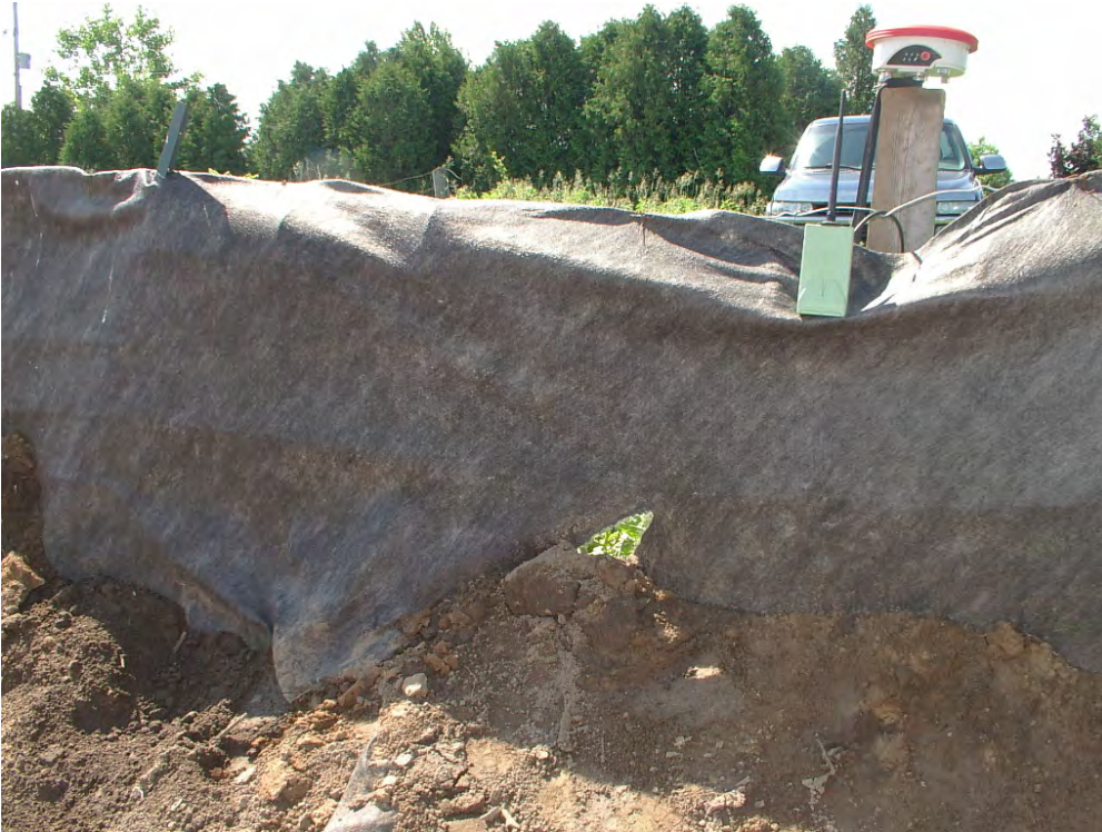
Photo 1: Tear in silt fence along south edge of fill borrow area
