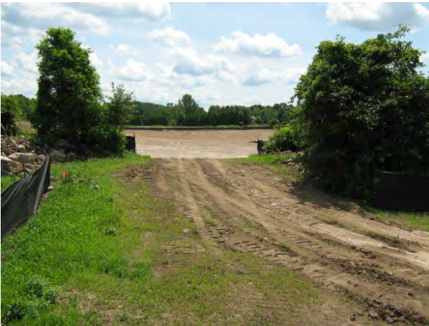
Photo 2. Access lane between borrow pit and topsoil missing silt fence
