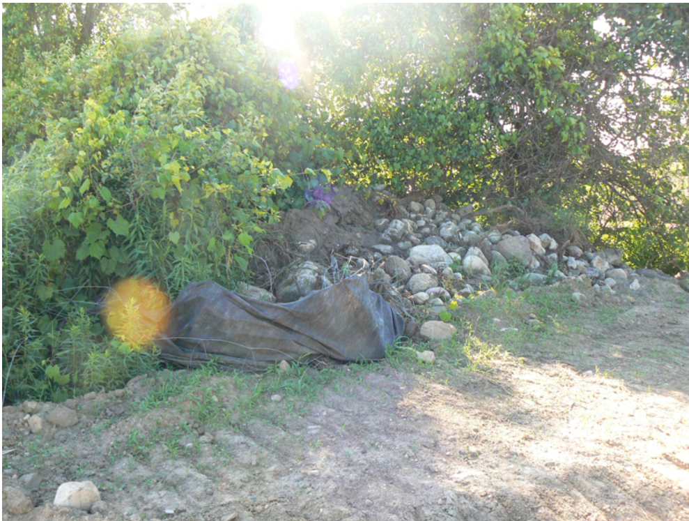
Photo 4: West side of access in hedge row missing silt fence
