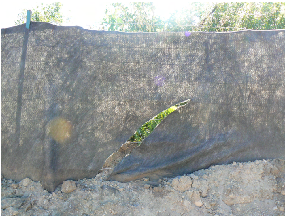
Photo 2: Tear in ESC fence along west edge of fill borrow area
