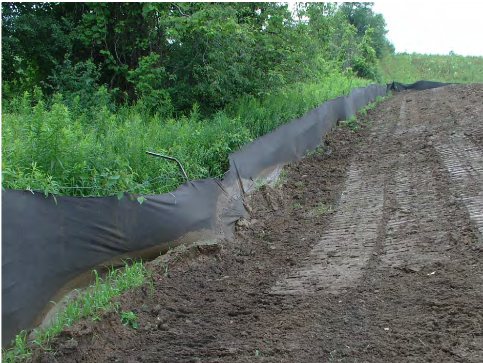
Photo 4: Accumulation of topsoil against southern edge of silt fence in stockpile area and grading change to alleviate pressure on silt fence
