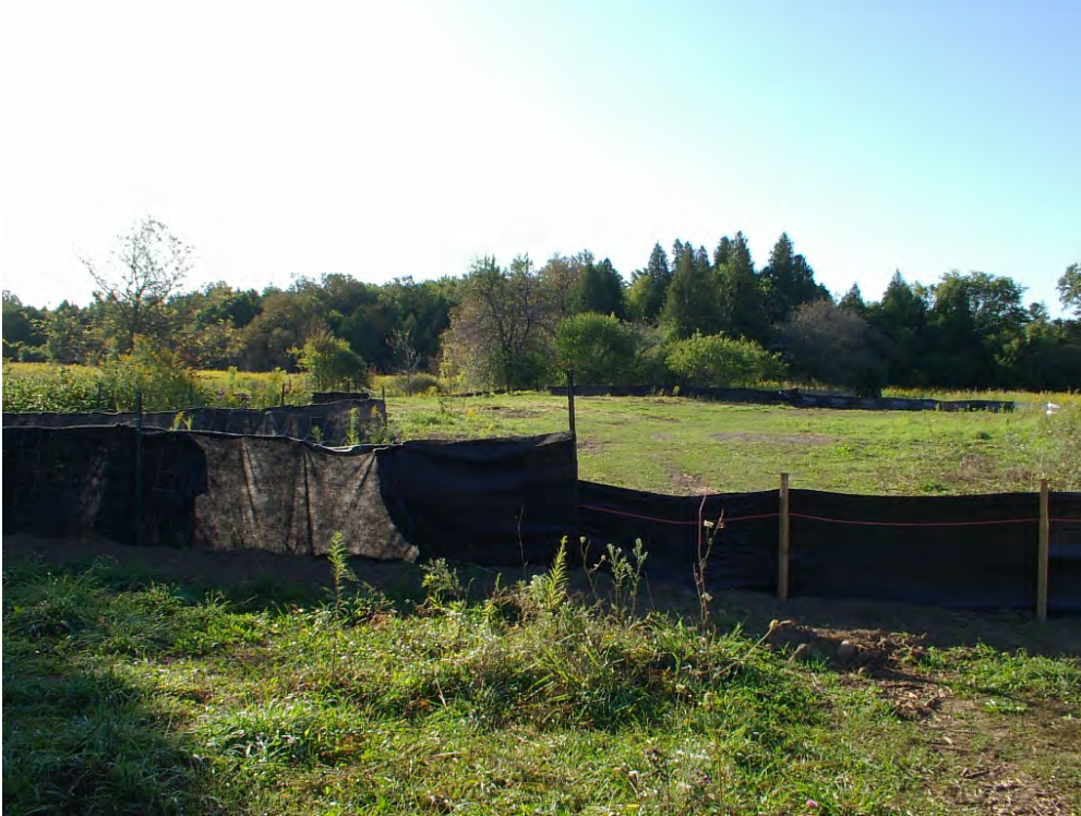
Photo 1: Heavy duty silt fence and Terrafix fencing
