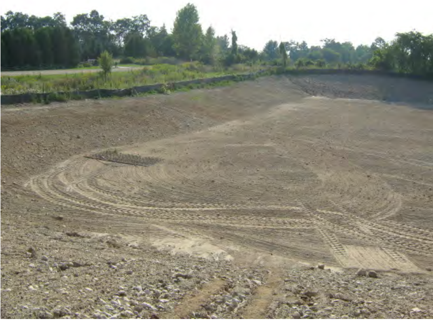
Photo 3: Recent scarification of soil in preparation for seeding.
