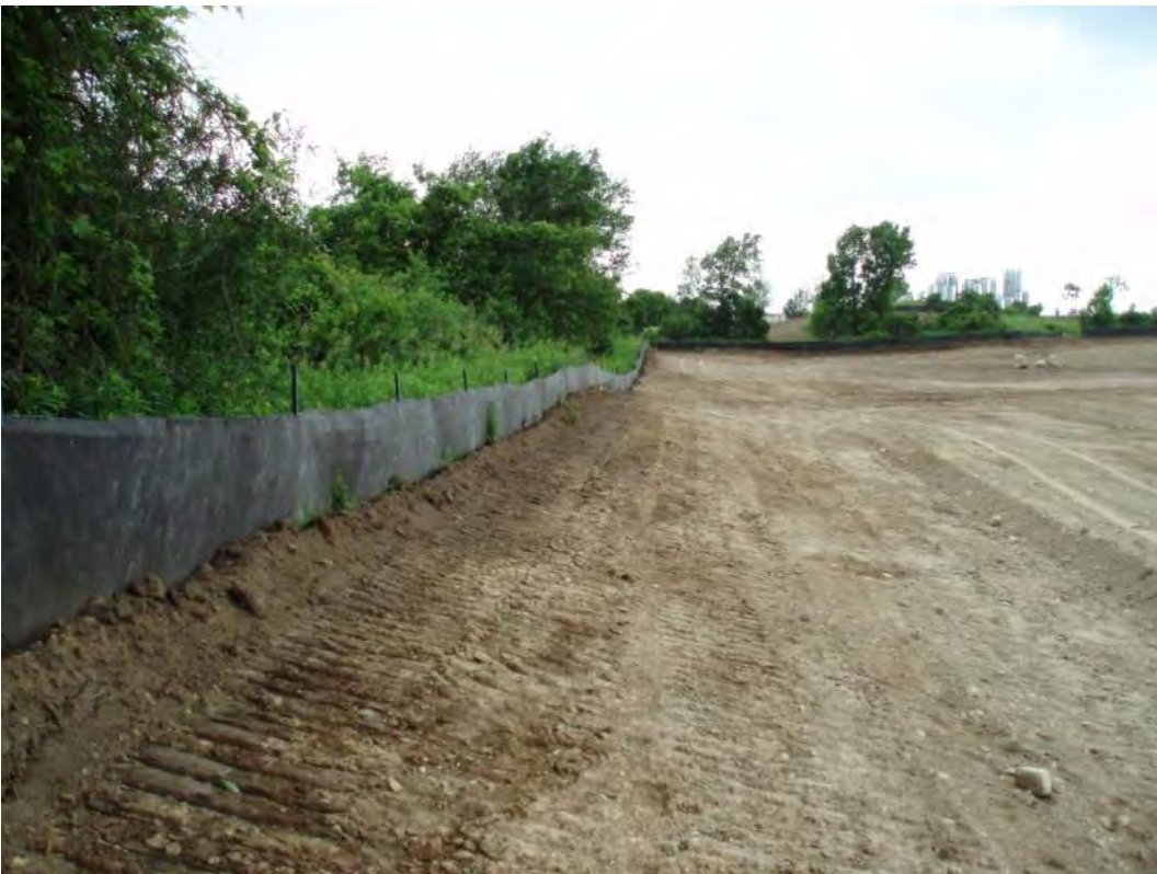
Photo 2: Small earth berm created along inside of silt fencing
