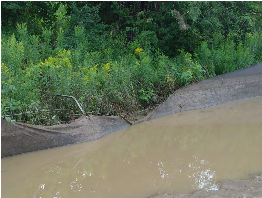
Photo 4: Fencing along south edge of stockpile area that has failed as a result of heavy rains and excess topsoil
