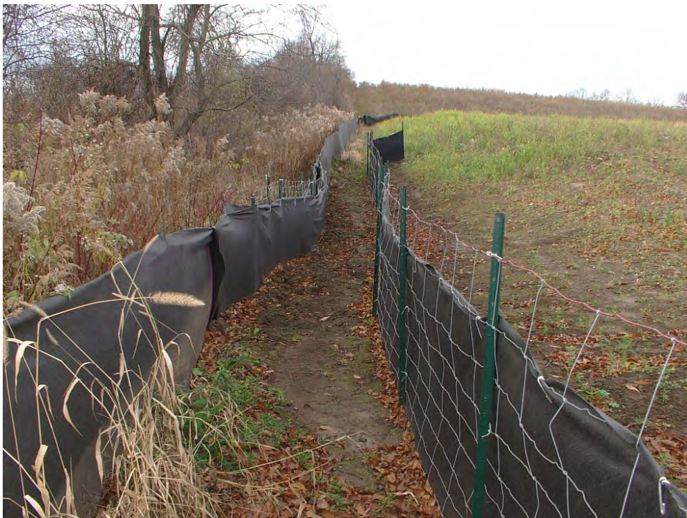
Photo 4: Reinforced heavy-duty silt fence along south portion of stockpile area
