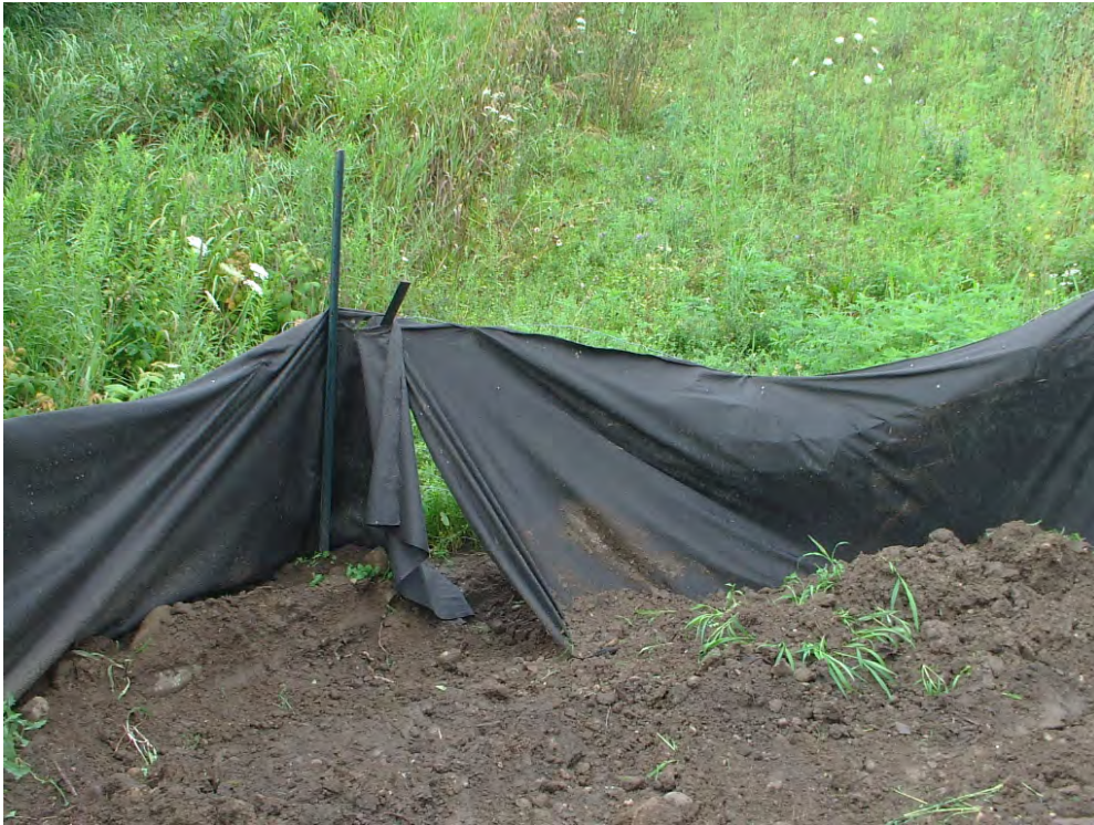
Photo 3: Gap and slumping in silt fence in southwest corner of stockpile area
