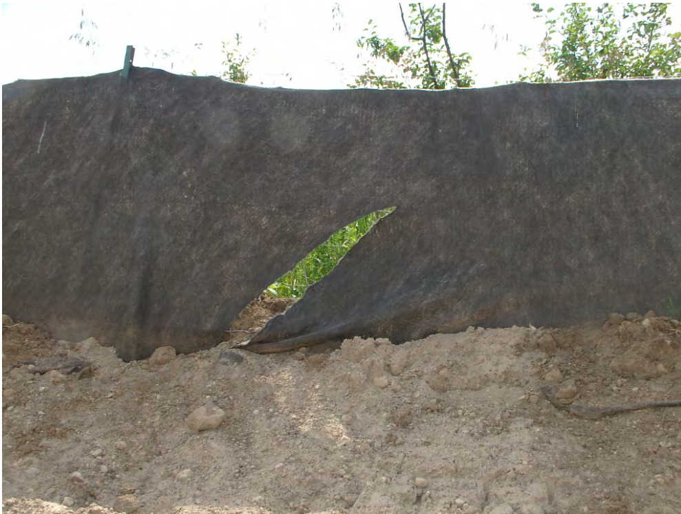
Photo 3: Second tear in ESC fence along west edge of fill borrow area
