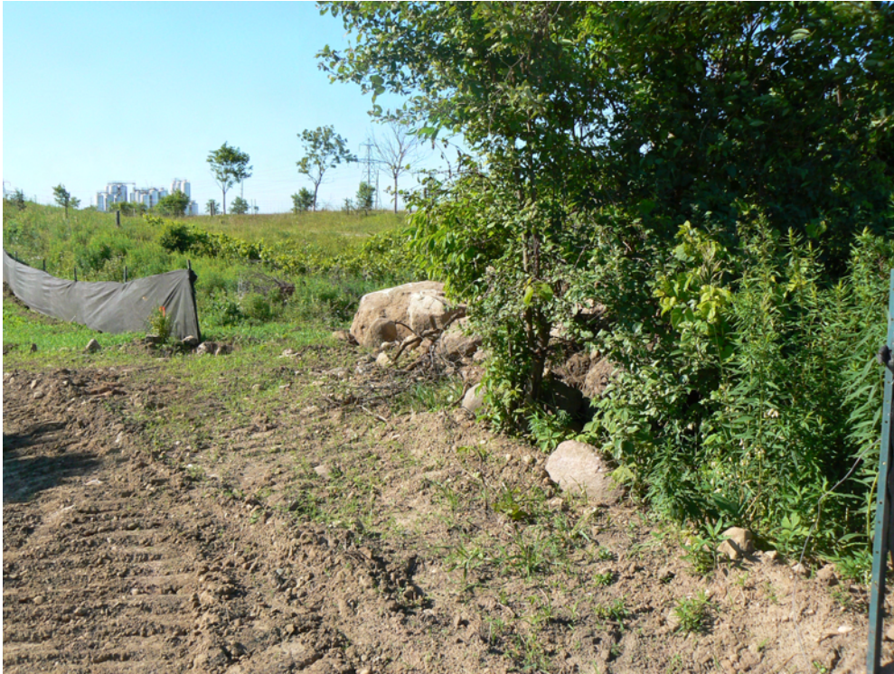
Photo 5: East side of access to stockpile along hedgerow missing silt fencing
