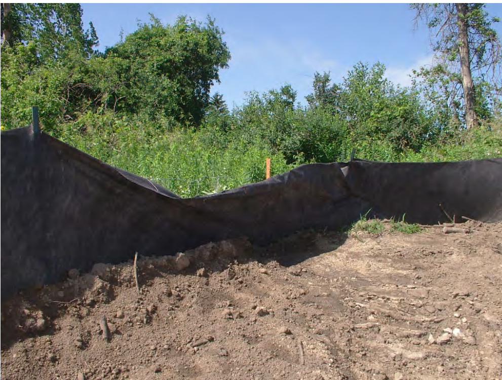
Photo 2: Slumping in silt fence in southwest corner of fill borrow area
