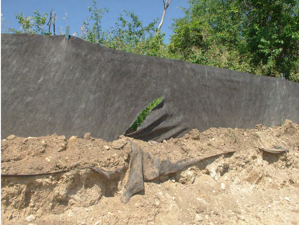
Photo 3: Tear in silt fence along west edge of fill borrow area
