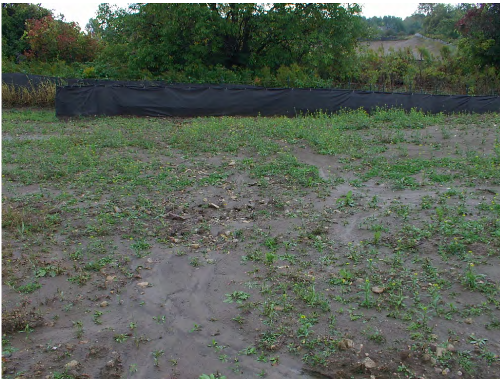
Photo 3: Signs of run-off due to lack of seed establishment within stockpile area
