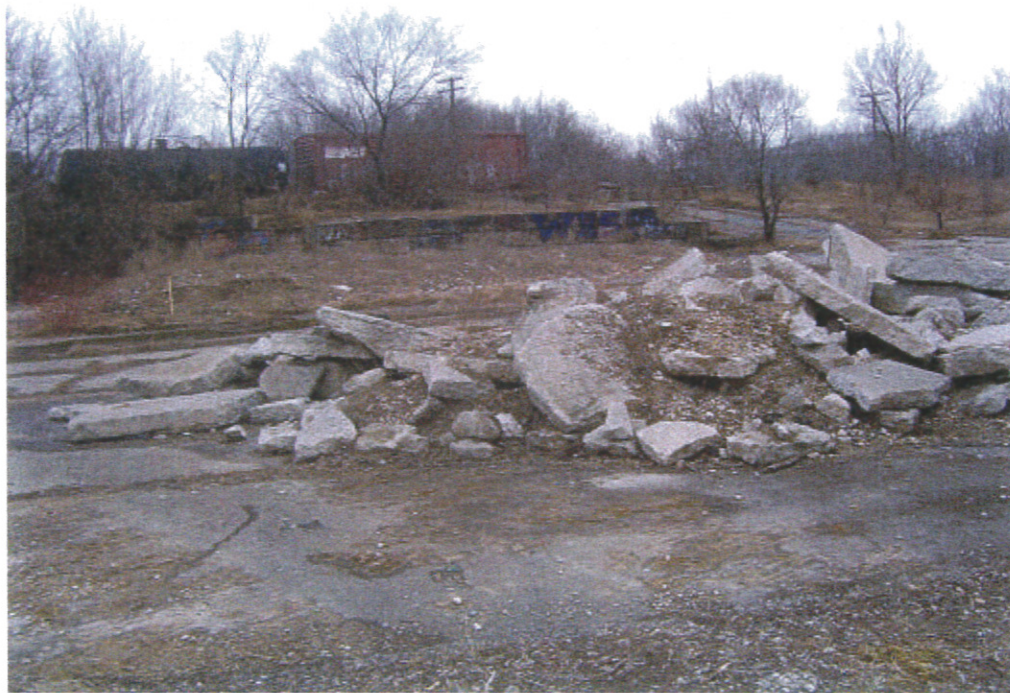
Photograph 10: A view of the concrete pieces observed near the former asphalt plant.
