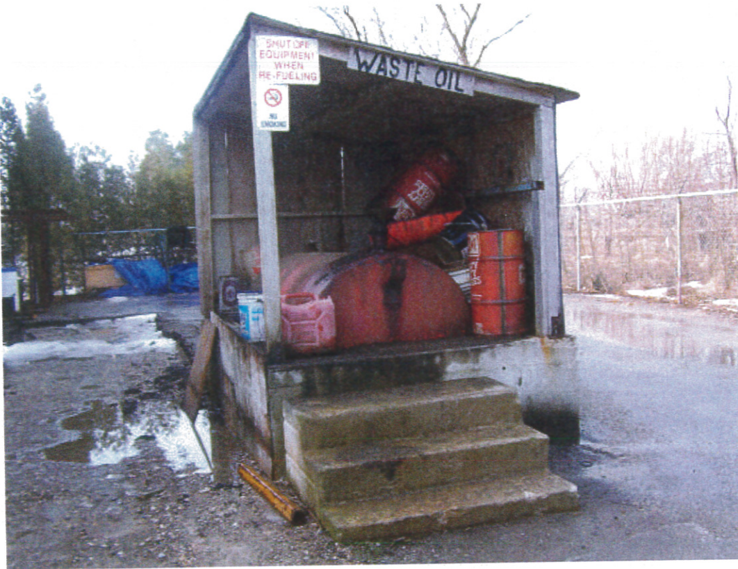
Photograph 7: A view of the waste oil AST located on the north side of the building.
