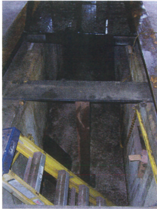
Photograph 1: A general view of the concrete pit located in the workshop.
