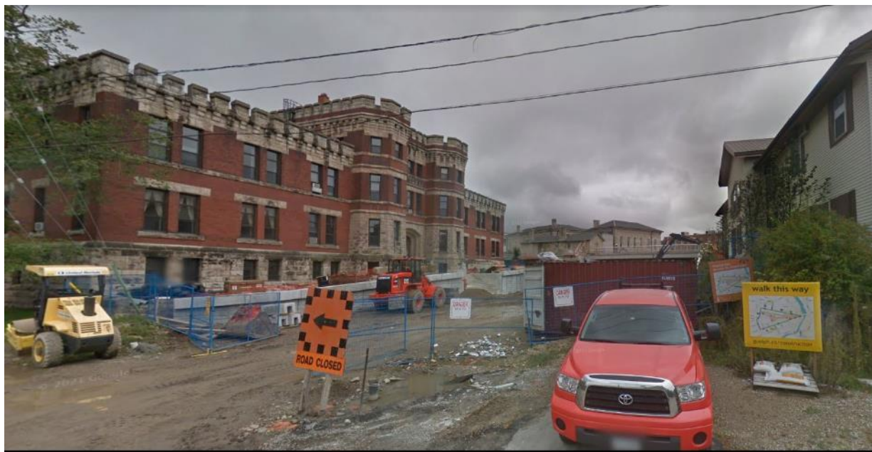
Image 49: 2011 construction on Wyndham Street South and within the Armory grounds.
