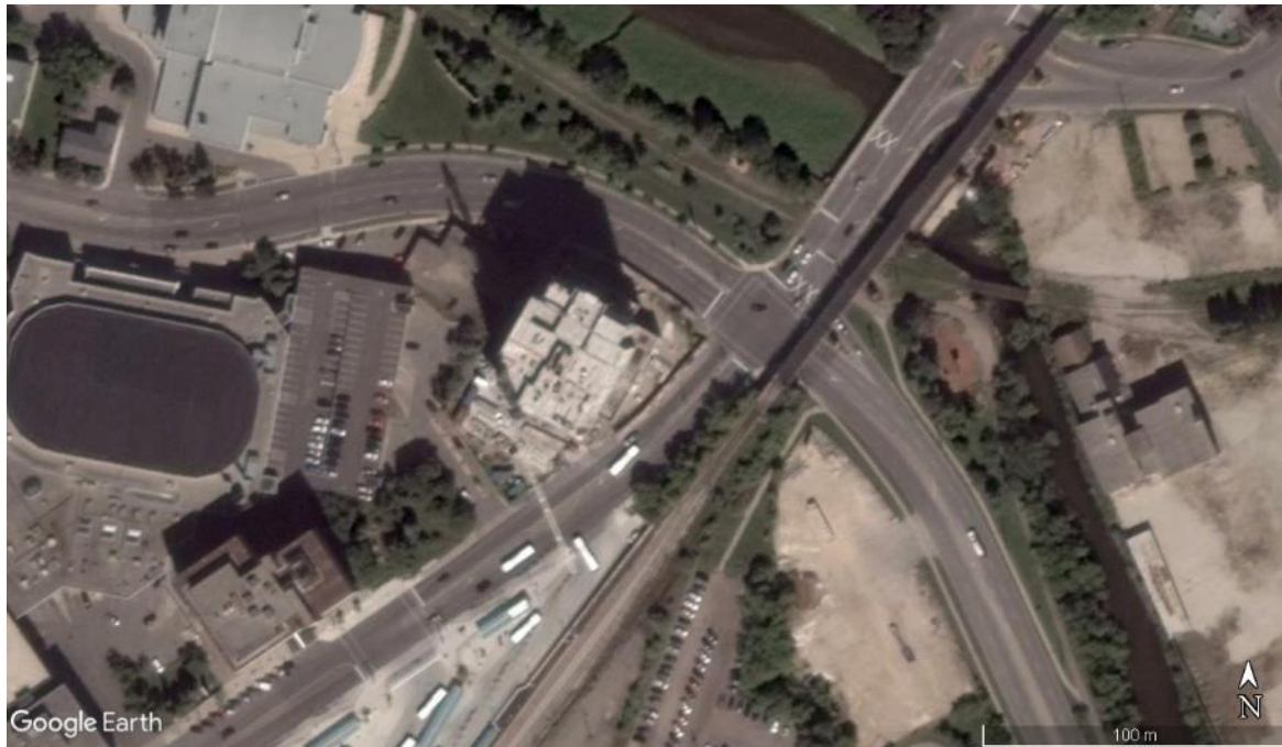
Image 54: 2013 construction of 160 Macdonell Street
