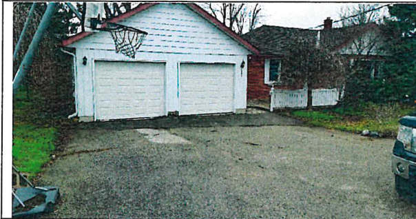
IMAGE 1 1871 GORDON STREET, WITH DRIVEWAY AND STONE PATIO
