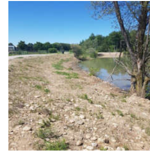
Side slope missing vegetation
