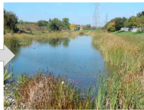
Side slope missing vegetation
