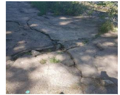
Cracking concrete spillway structure
