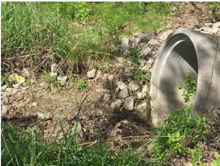
E. Early sediment accumulating at mouth of 1050mm pipe inlet
