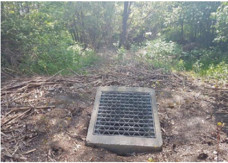
G. Ditch inlet catchbasin to infiltration trench in good condition
