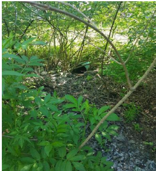
F. 375mm PVC inlet is est. 30% buried by rip rap, sediment and vegetation
