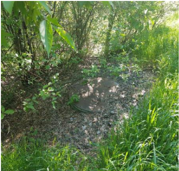
A. Perforated riser outlet with dense vegetation nearby and sediment deposition around 50mm clear stone jacket
