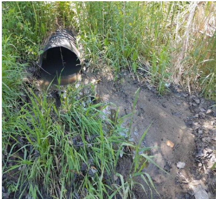
C. 450mm CSP Inlet 20% submerged and sediment deposition near mouth
