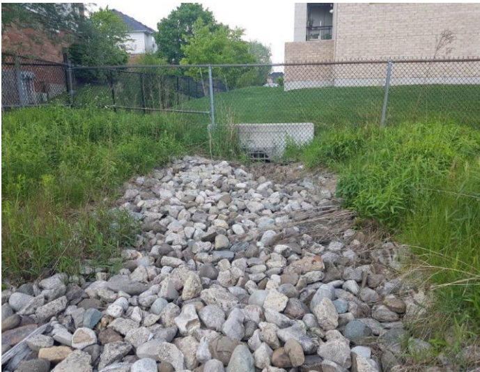
G. Downstream end of second pipe with 15% blockage from riprap
