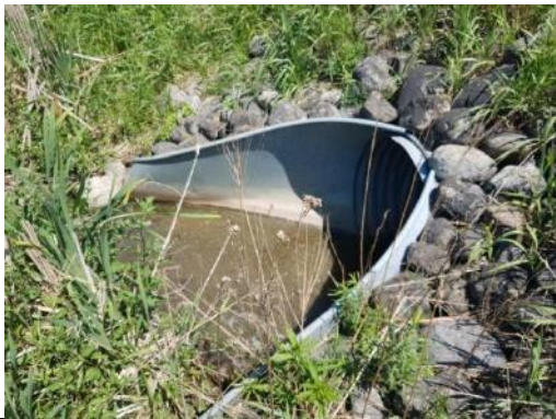
G. Outlet pipe with vegetation immediately downstream
