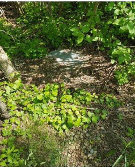
B. Perforated riser outlet with sediment accumulation covering clear stone jacket.
