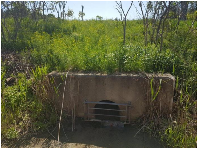
G. Inlet from East 10% filled with sediment
