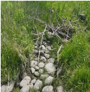
C. Riprap channel from inlet filled with dead fall and trash debris
