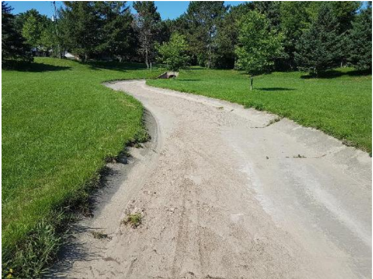
J. Concrete drainage channel going towards outlet structure. Note sediment accumulated at bottom of channel.
