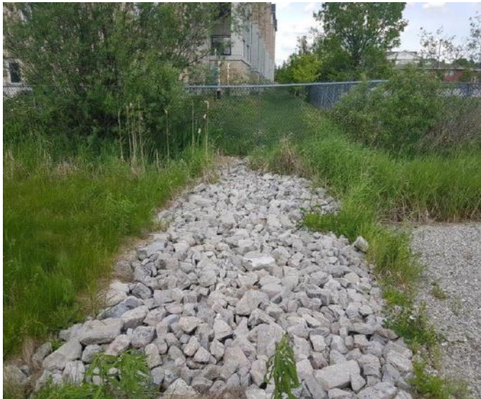
D. Rip-rap inlet channel looking upstream
