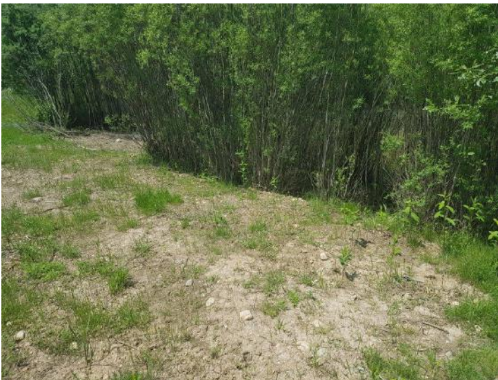
E. Berm from dry pond to west outlet pond with poor vegetation cover
