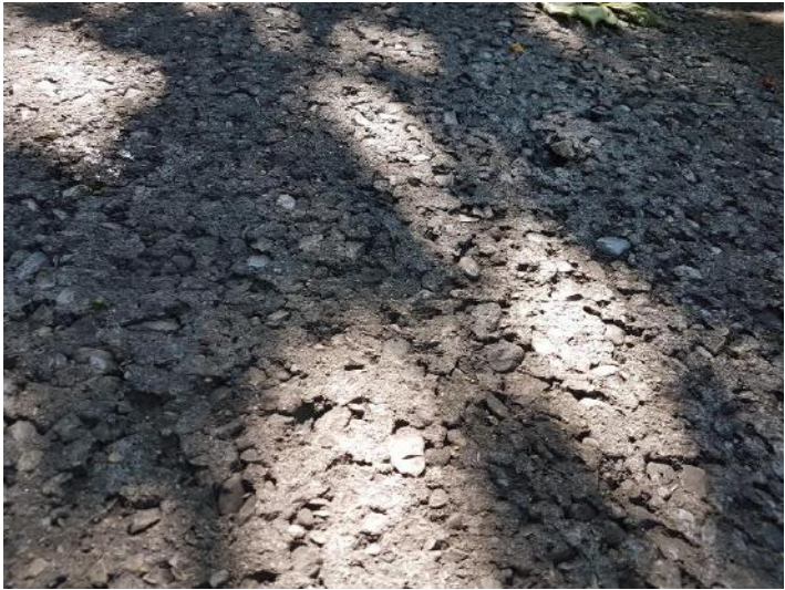
I. South inlet pipe concrete outfall channel showing early signs of erosion.
