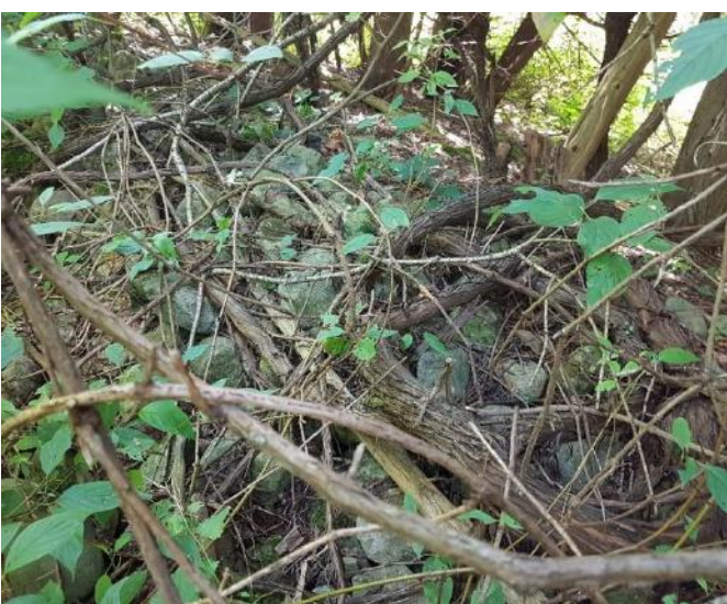
C. Overflow weir with rip-rap and dense brush vegetation causing minor flow restriction
