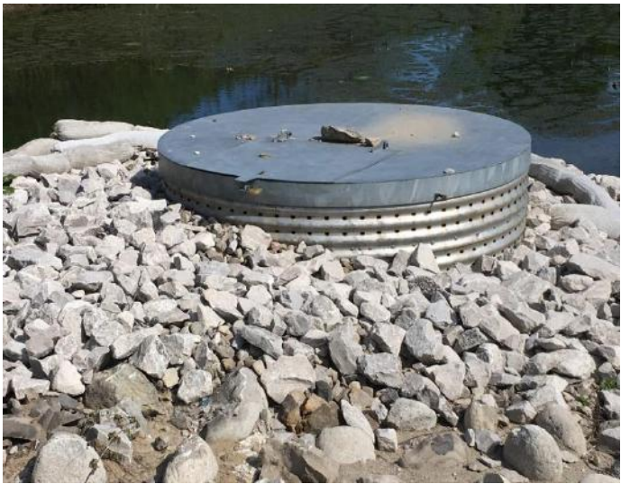
C. Hickenbottom structure with riprap base in good condition
