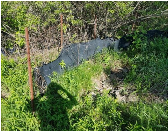
H. Silt fence at outlet channel
