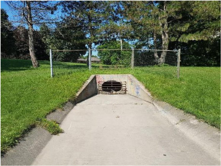
K. Concrete outlet pipe and headwall structure with protective fence. Note graffiti on
