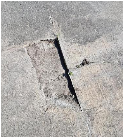
M. Crack in concrete drainage channel near outlet structure. Allows water to infiltrate and may expand with freeze thaw cycles.
