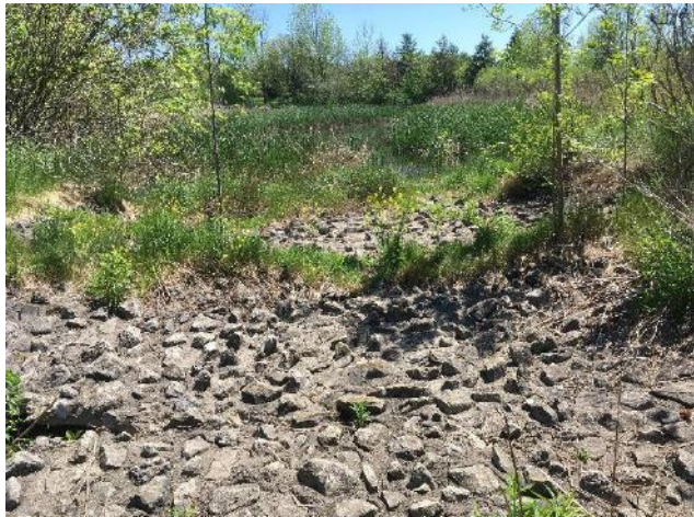
E. Overflow weir from forebay to dry pond
