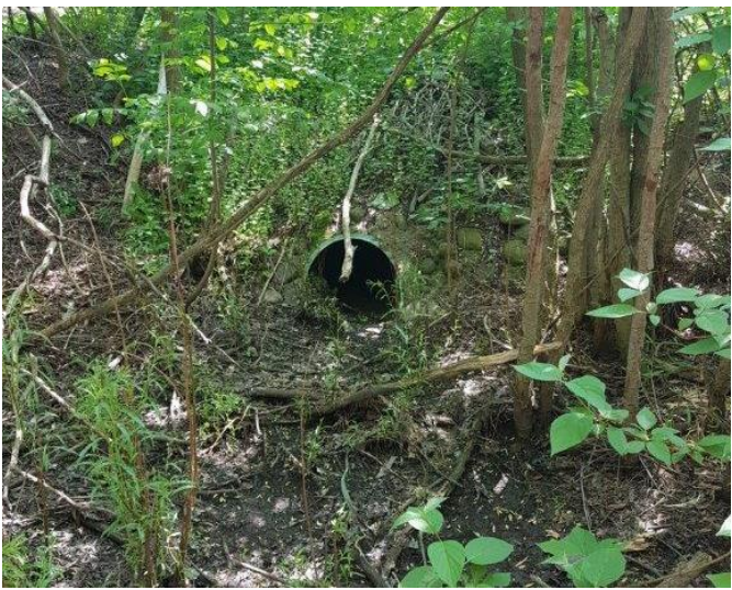
E. Inlet pipe an estimated 15% clogged
