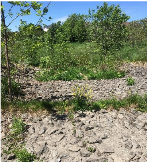
G. Overflow weir from forebay to dry pond
