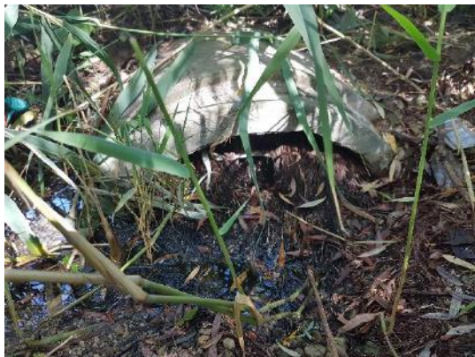
J. 600mm concrete inlet pipe from Valleyhaven Lane 95% blocked with sediment
