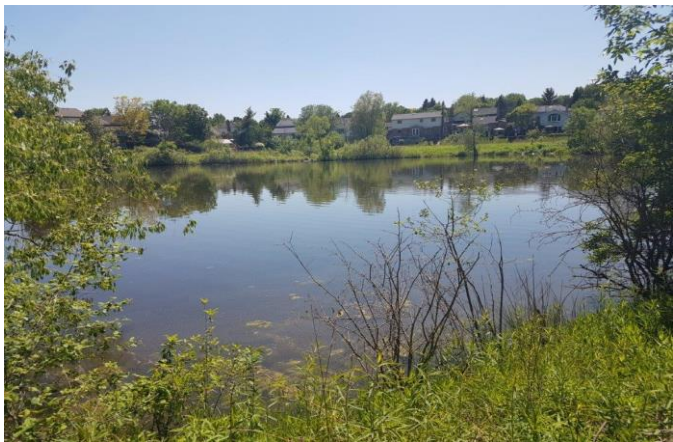
E. Recharge basin with high permanent water level
