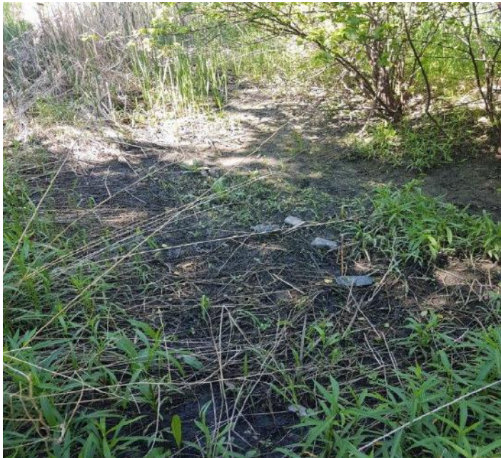
B. Ditch with sediment deposition overtop sand filter layer
