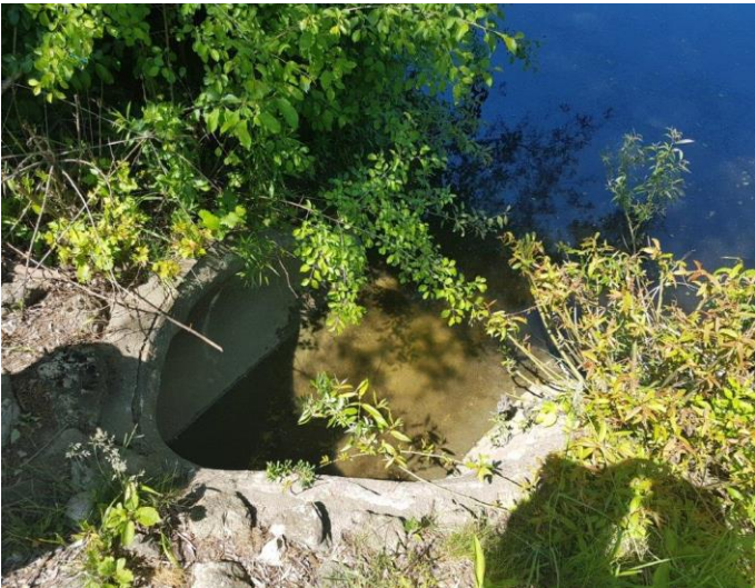
A. Concrete inlet pipe and outfall into forebay basin
