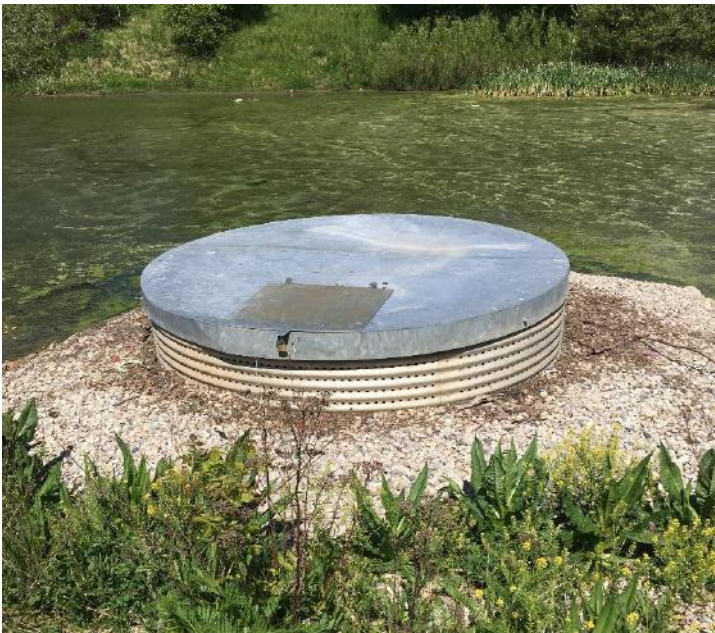
B. Hickenbottom riser with early signs of sediment accumulation
