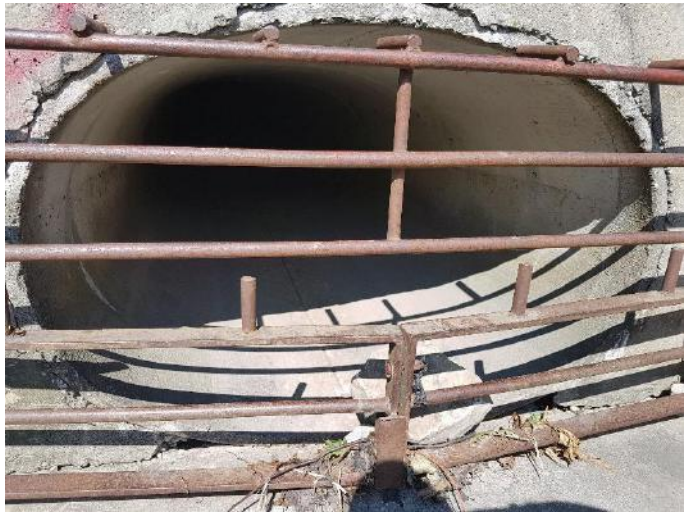
L. Concrete outlet pipe and trash grate.
