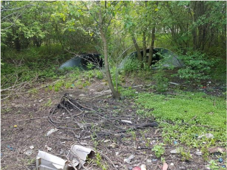
B. Outlet structures with garbage and trees growing in front of pipes
