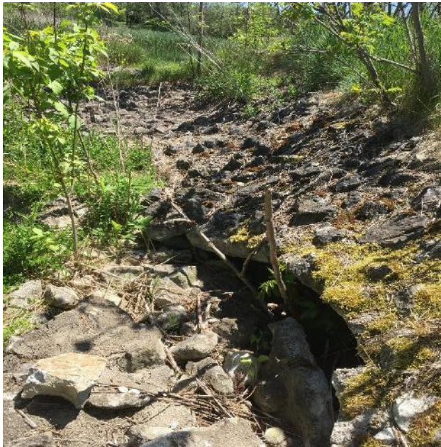
C. Riprap channel between ponds (damaged)
