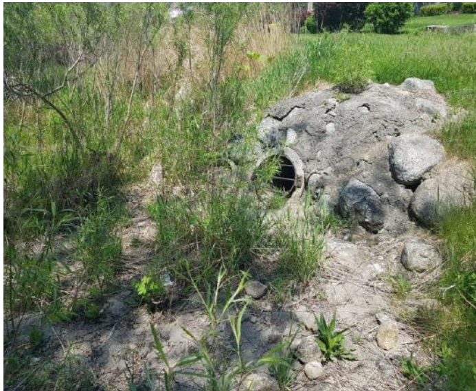
D. Concrete inlet pipe, East Pond
