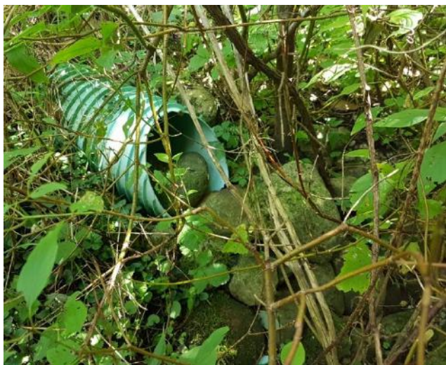
G. 300mm PVC outlet pipe from hickenbottom riser structure with rip-rap around outfall creating a 30% blockage in flow capacity
