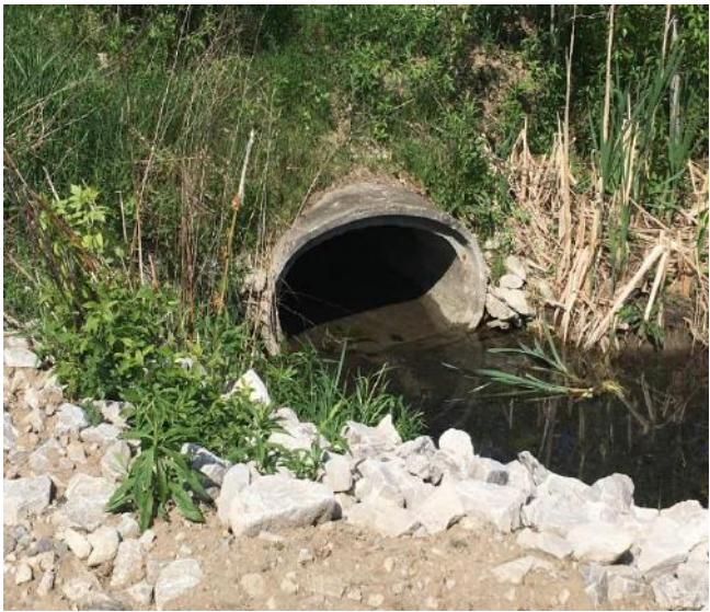
A. Inlet to forebay pond approximately 15% submerged
