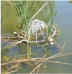
E. Submerged trash rack from sediment clogging on up or downstream end of outlet pipe
