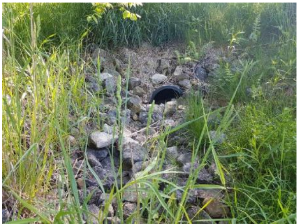
I. Pond outlet pipe 50% blocked by rip-rap
