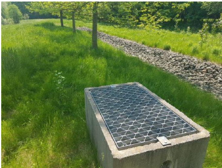
F. Overflow inlet grate structure with rip-rap
