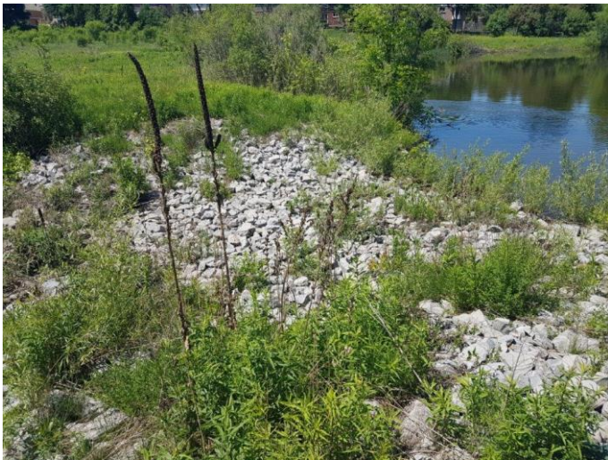
D. Spillway between forebay and main cell with minor vegetative overgrowth (replaced in 20__)
