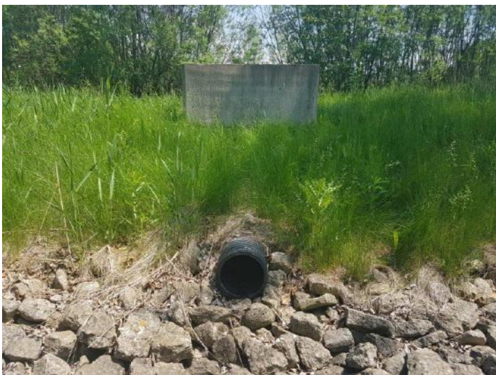
G. Downstream end of pipe with rip-rap (East)
