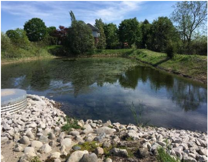
B. Forebay with algae growth and high standing water level
