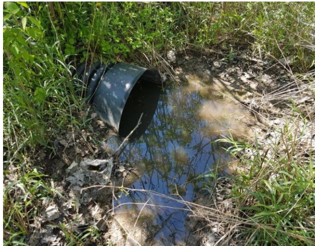
F. 500mm inlet pipe that is 30% submerged
