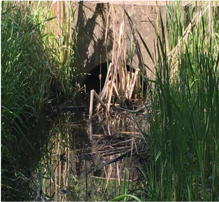
A. Inlet pipe 30% submerged
