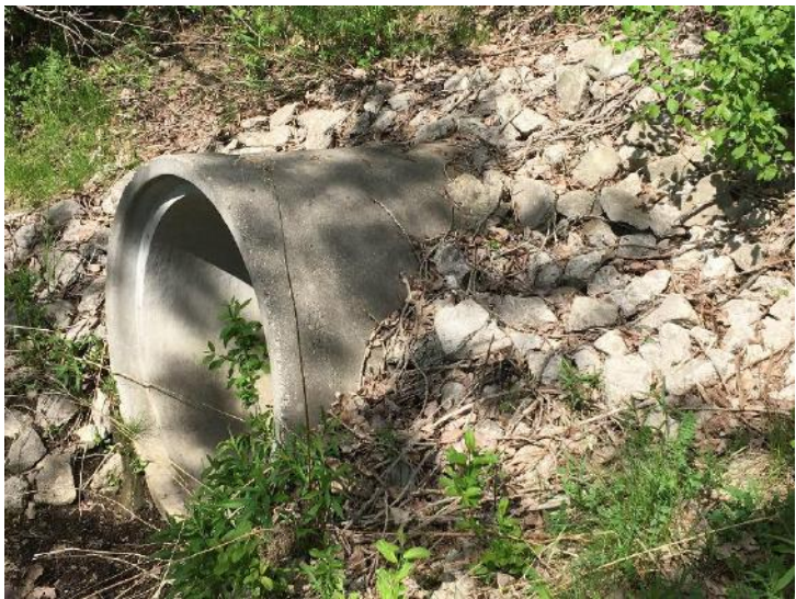
F. Riprap around 1050mm pipe
