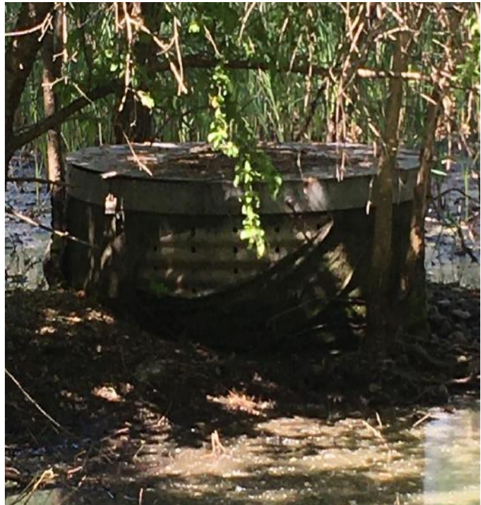
C. Perforated riser outlet structure with torn sediment cloth and missing 50mm clear stone jacket as noted in design drawings
