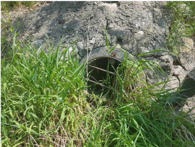
C. Inlet to dry pond 15% blocked by vegetation
