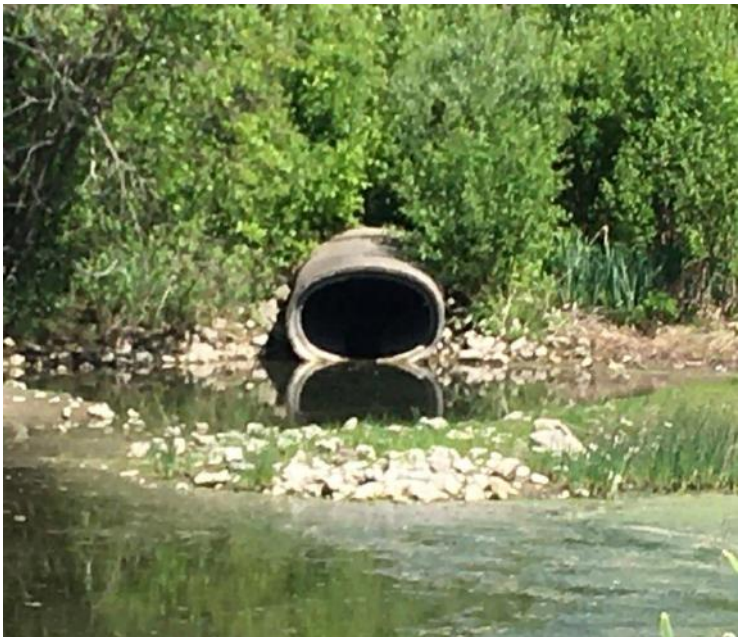
C. Inlet wet pond and forebay
