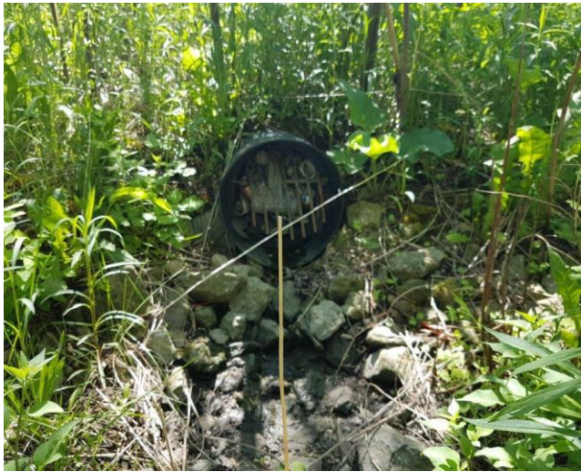
E. 300mm inlet pipe with damaged grate and 40% clogged with trash
