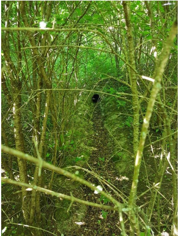
A. Riprap channel and inlet pipe with vegetation and debris in outfall
