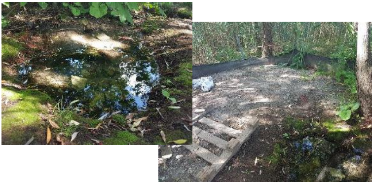
K. 600mm concrete inlet pipe from Henry Court 80% blocked and submerged in small pool. Outfall area filled with sediment and trash present
