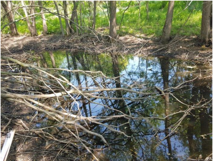
D. Dry pond basin with less than 300mm of standing water and accumulated sediment preventing water from leaving via riser outlet structure
