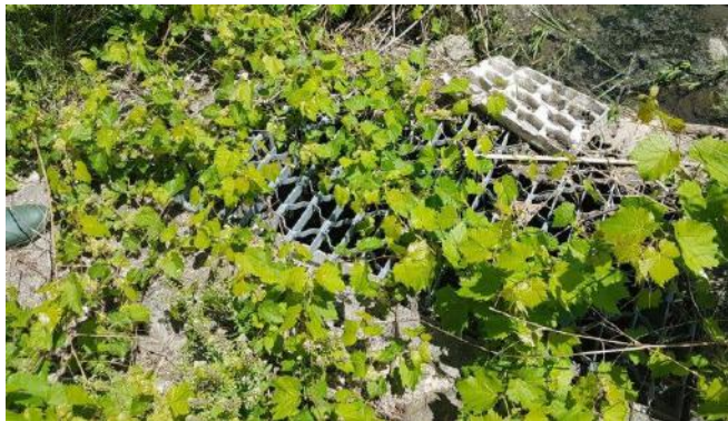
H. Outlet grate structure covered in vegetation
