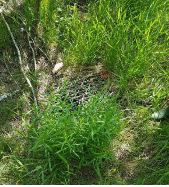
A. Ditch inlet blocked by vegetation and debris
