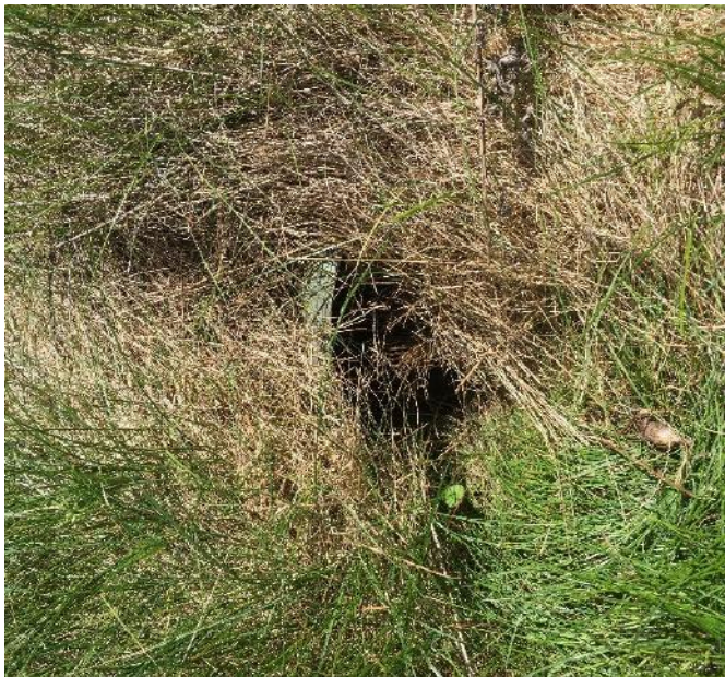
A. Outlet pipe from dry basin perforated riser 30% buried in earth and grass
