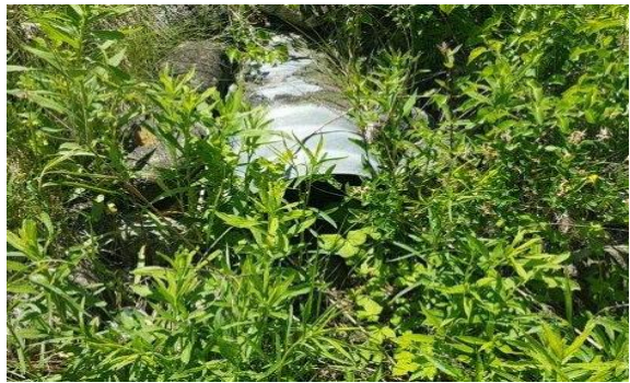
E. CMP 50% buried in vegetation and debris
