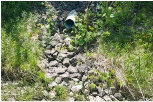
D. 200mm Inlet pipe off channel
