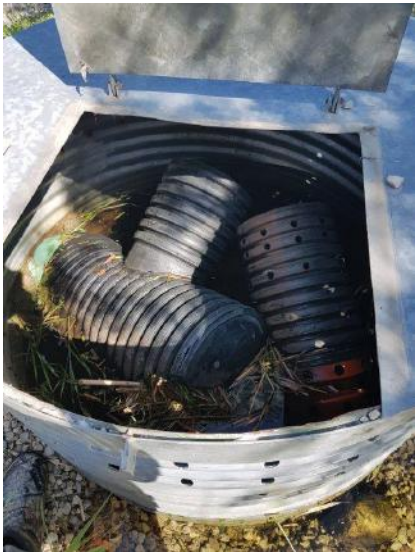
B. Inside Hickenbottom with multi-perforate riser outlet system
