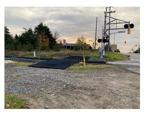
FIGURE 3-5: RUBBER SPIKE MAT AT WATSON ROAD LRC
