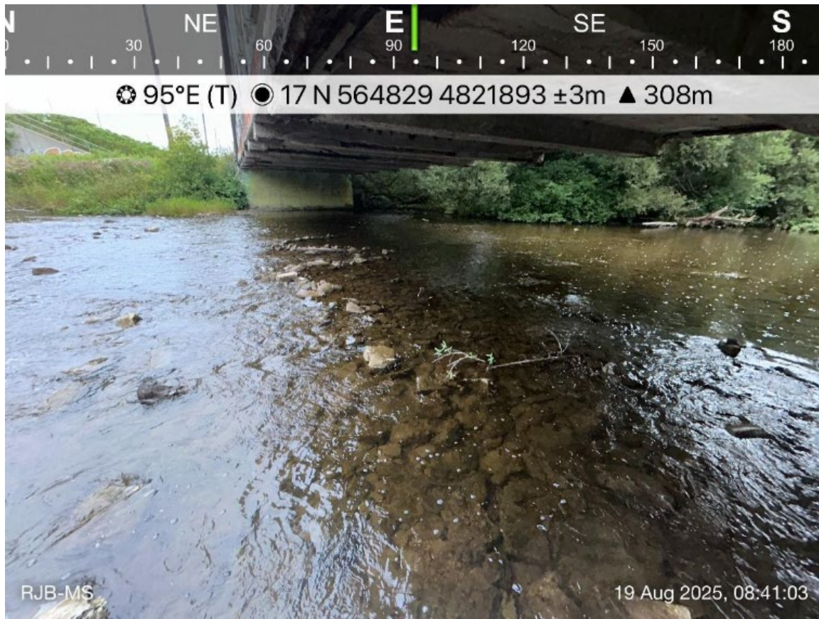
Photo 4: Underneath McQuillan's Bridge (Structure 116), downstream area of the pool.
