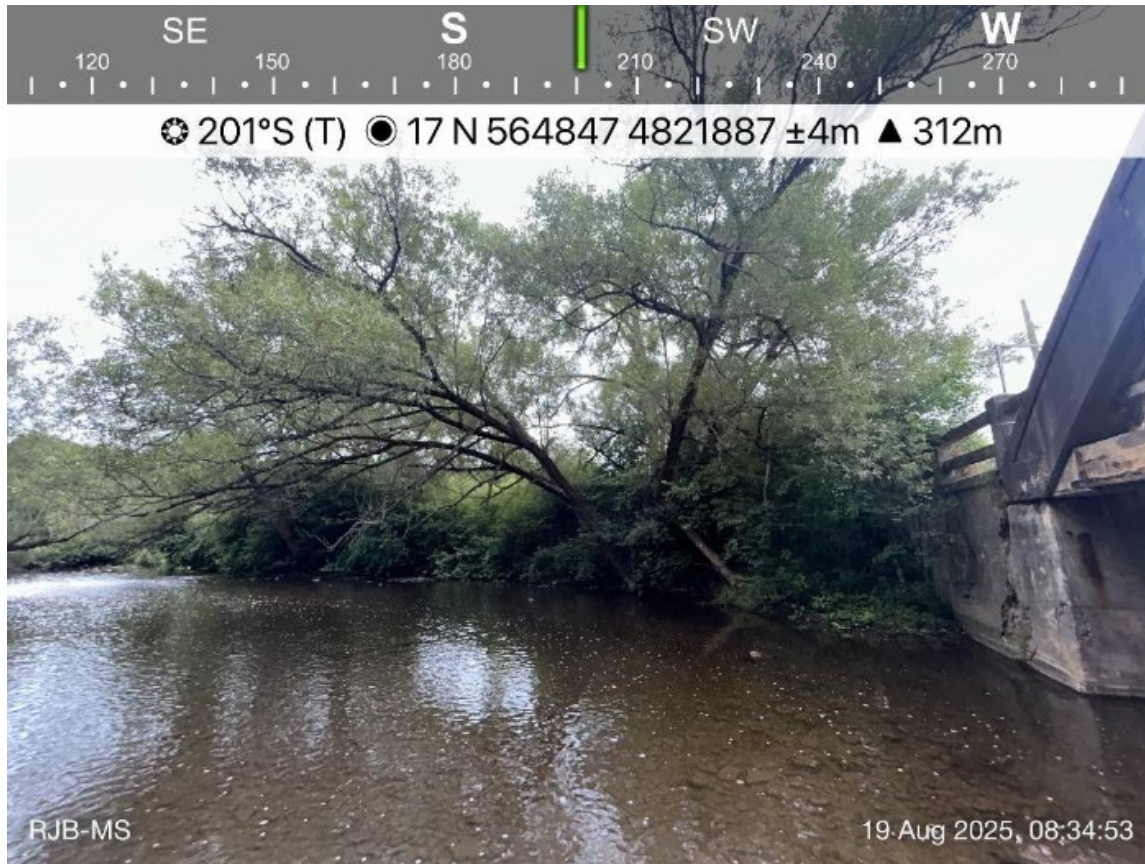
Photo 2: Looking upstream of McQuillan's Bridge (Structure 116)'s run.
