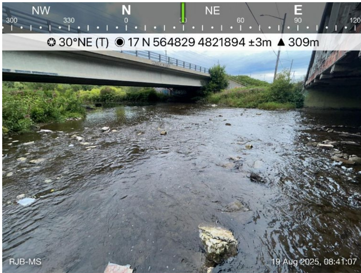
Photo 5: Area between McQuillan's Bridge (Structure 116) and Stone Road Bridge.
