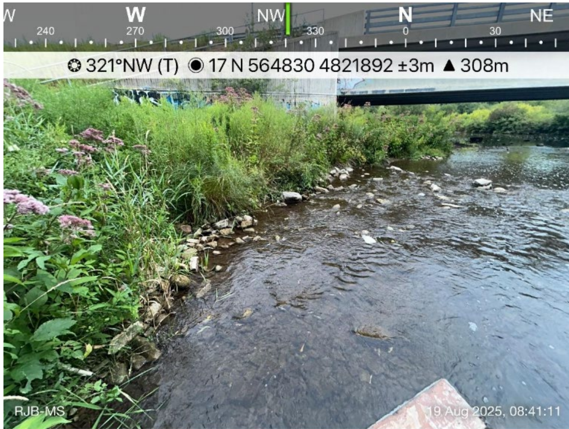
Photo 6: Riverbank of the area downstream of the bridge on Stone Road.
