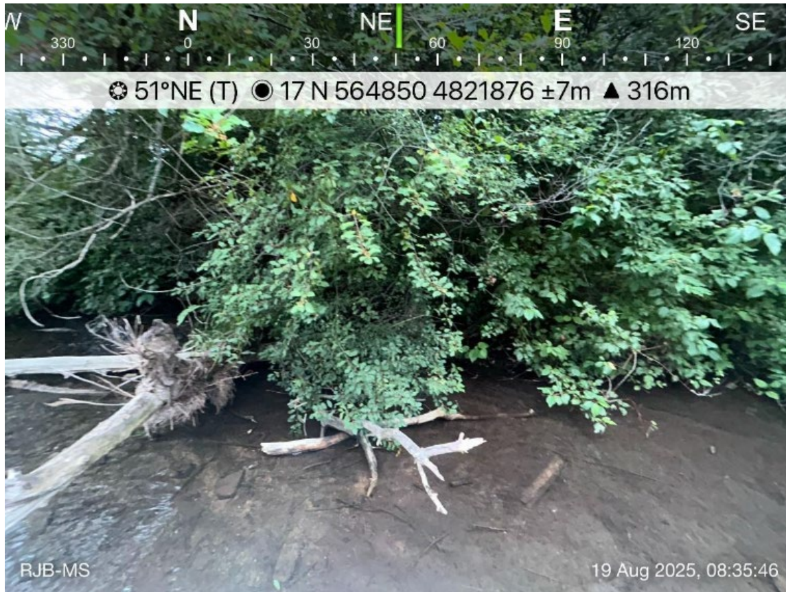
Photo 3: Looking toward the upstream McQuillan's Bridge (Structure 116)'s pool.
