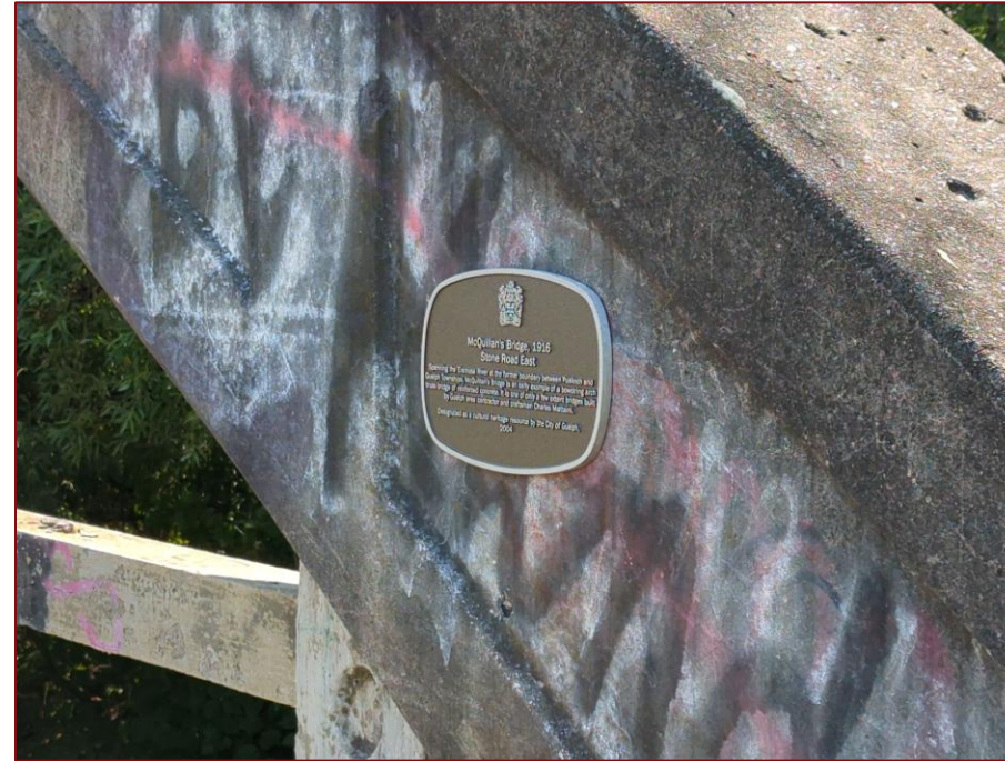
Image 16: Concrete Cross-Tie with Date Inscription
