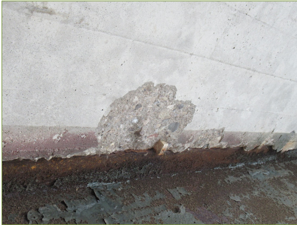
Photo P15 Soffit at West Abutment, north edge (spall) and Girder (light corrosion)
