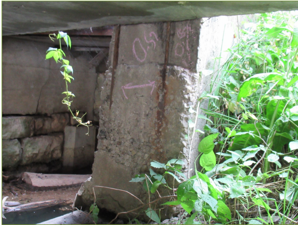
Photo P3 Inlet – North Elevation, West Wall (spall, and delamination) note, exposed rebar
