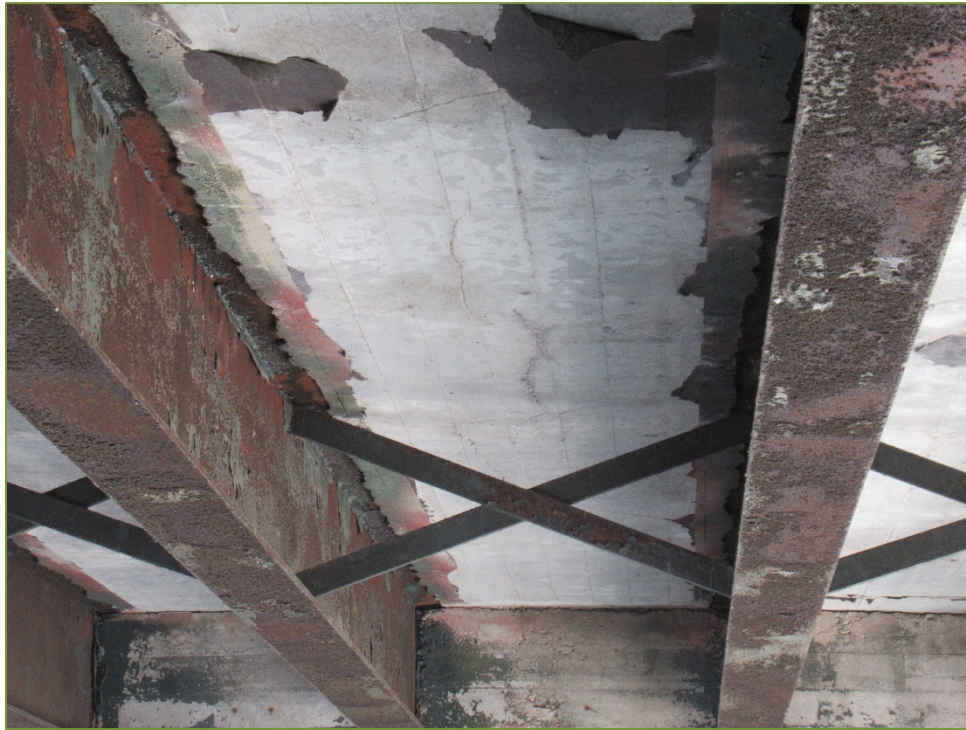
Photo P17 Soffit between West Abutment and Pier between 3 rd and 4 th Girder from North (cracks and light scaling) and Girders (light corrosion)
