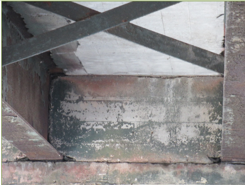
Photo P38 Typical Diaphragm at Pier – East Face
