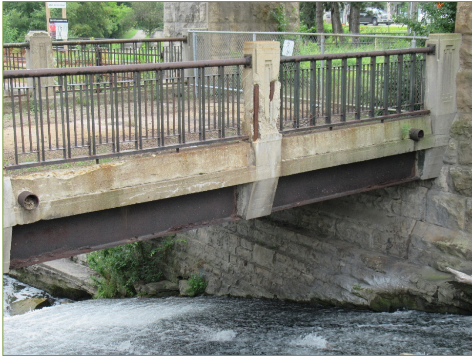
Photo P41 North Elevation – Fascia (cracks, spall, delamination, and light scaling)
