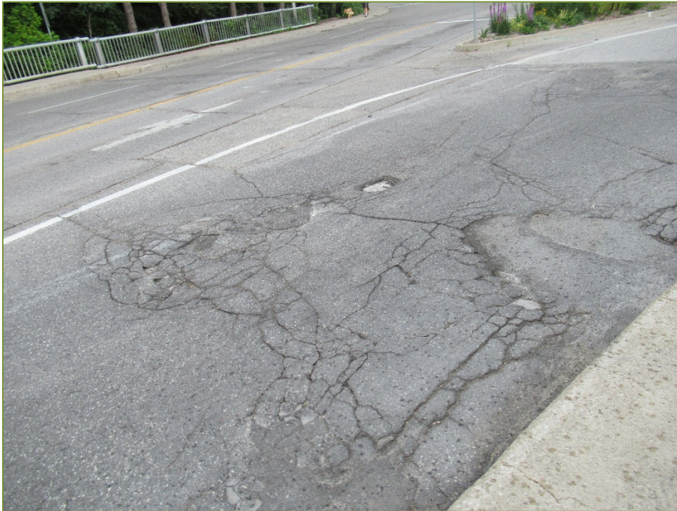
Photo P8 Deck Wearing Surface (unsealed cracks, alligator cracks and pot holes and rutting)
