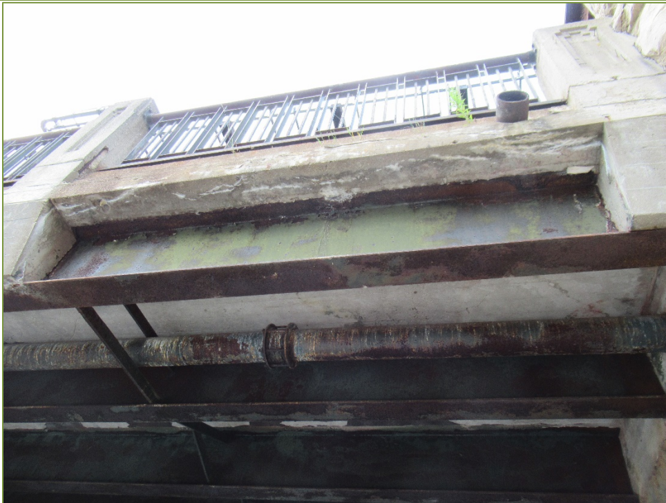
Photo P30 Soffit between at East Abutment, south edge (cracks) and Girders (light corrosion)
