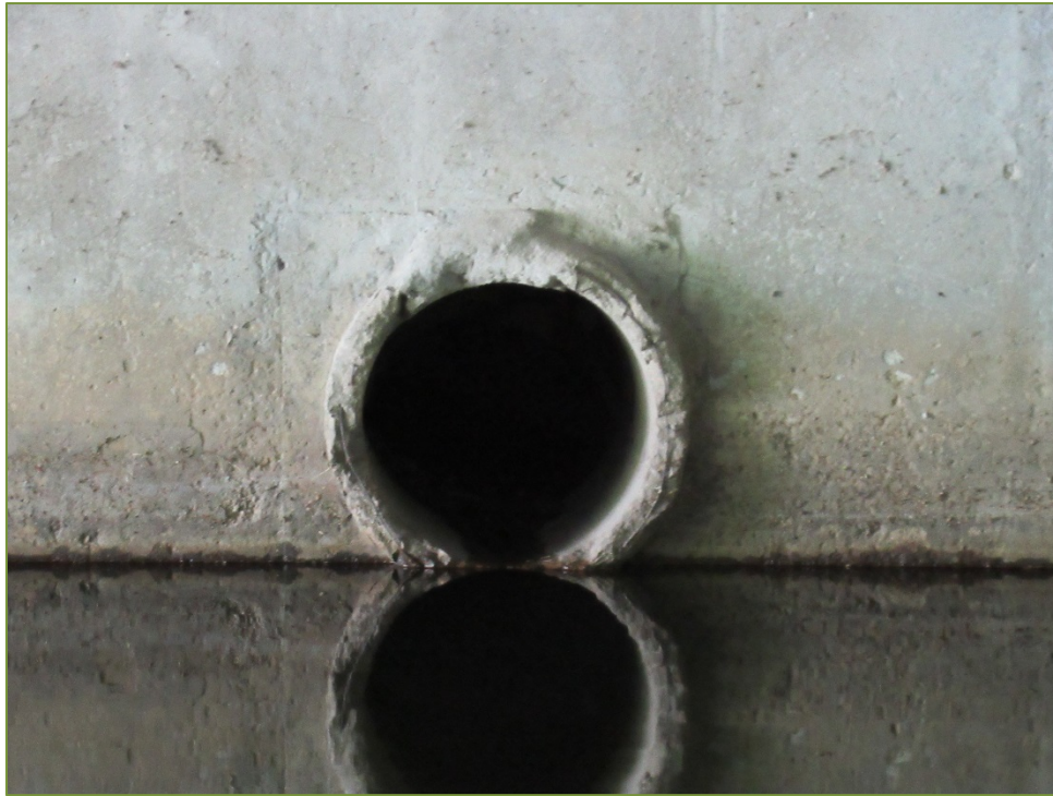
Photo P49 East Abutment (cracks, and medium scaling) note, drain
