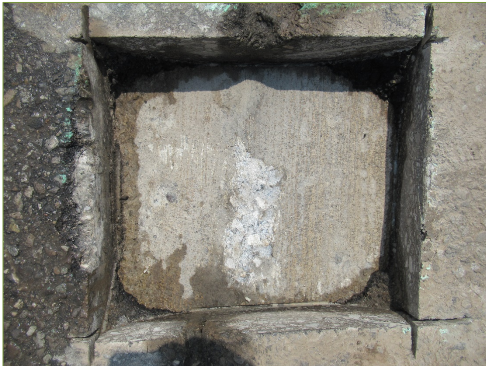
Photo S12 – Sawn Sample SS12 (light scaling)
