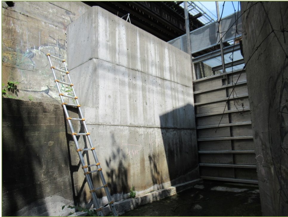
Photo P13 Outlet – North Wall, new structure (cracks, and light scaling)
