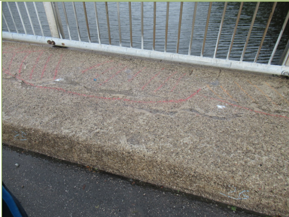
Photo P40 North Sidewalk (cracks, spall, delamination, and severe scaling) and Handrail (light corrosion)
