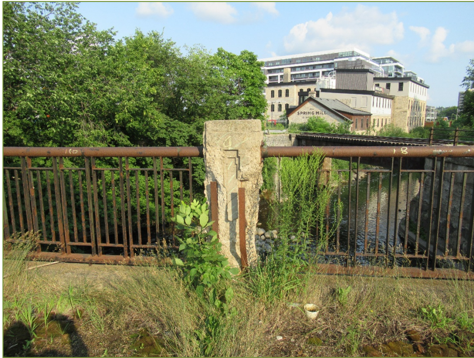
Photo P53 South Curb (medium scaling) Concrete Posts (cracks, spall, delamination, and light scaling) and Handrail (light corrosion)
