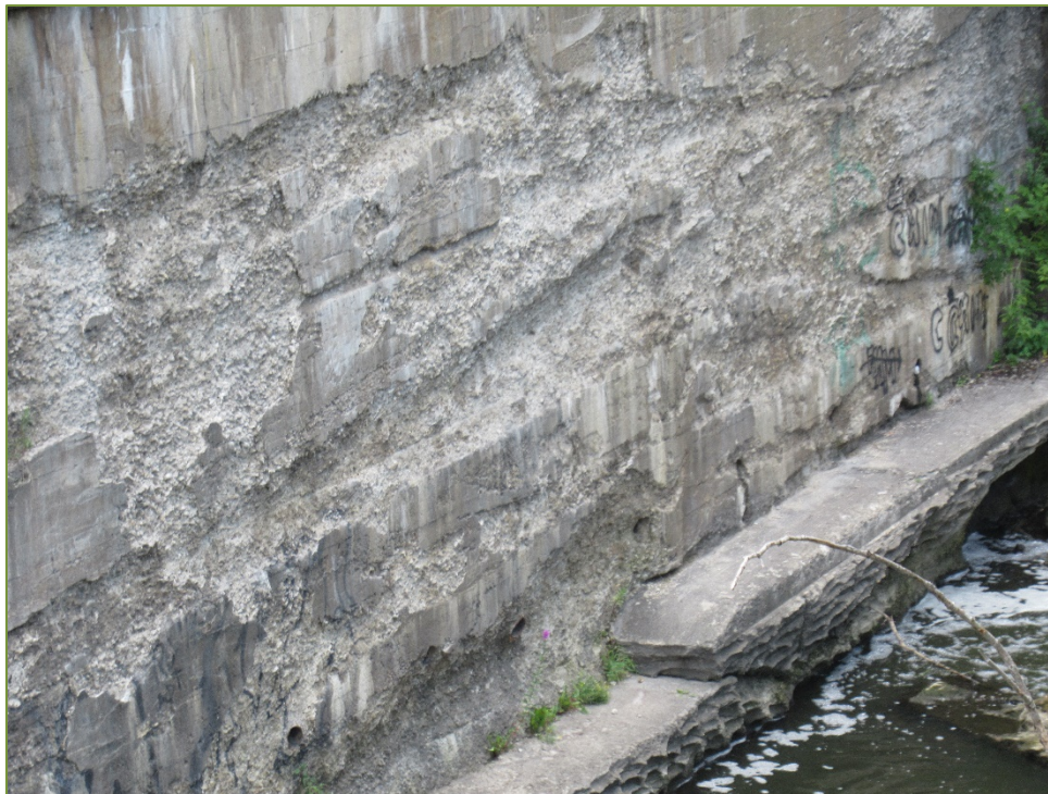
Photo P69 Southwest Retaining Wall (spall and severe scaling)
