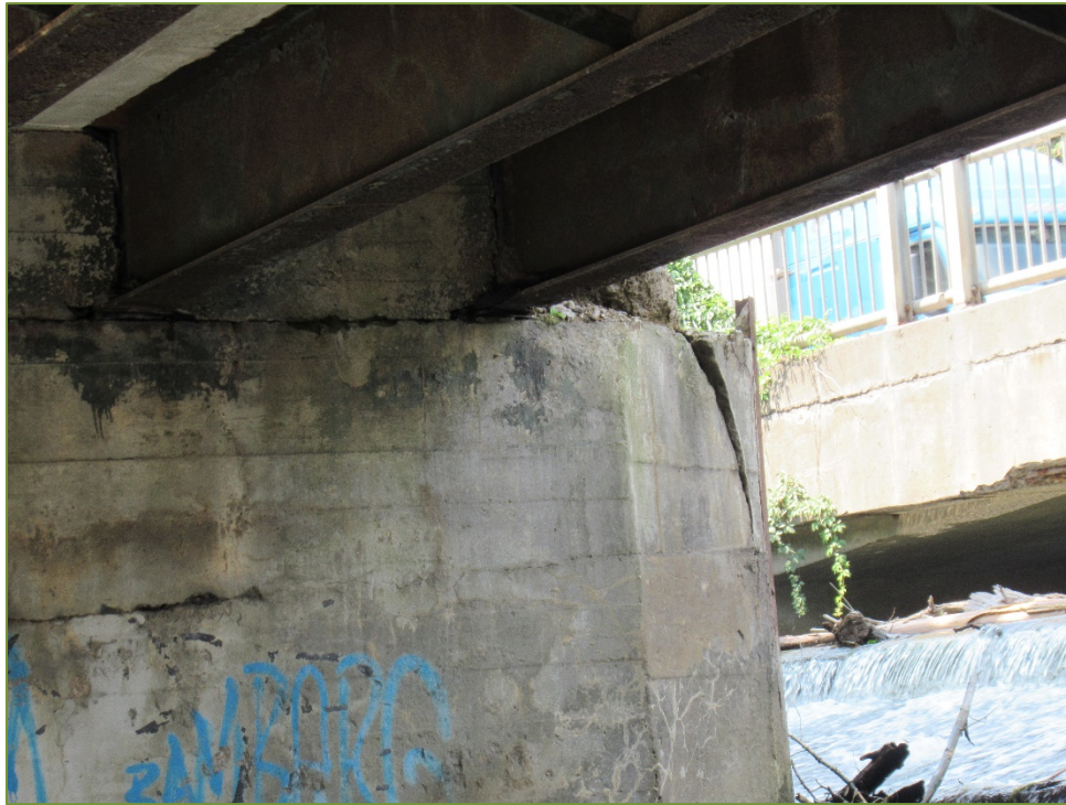
Photo P71 Pier - East Face, north side (cracks, spall, delamination, light to medium scaling, and wet area)
