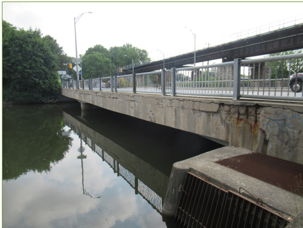
Photo P22 North Elevation – Fascia (wide cracks, spall and delamination) note, exposed rebar
