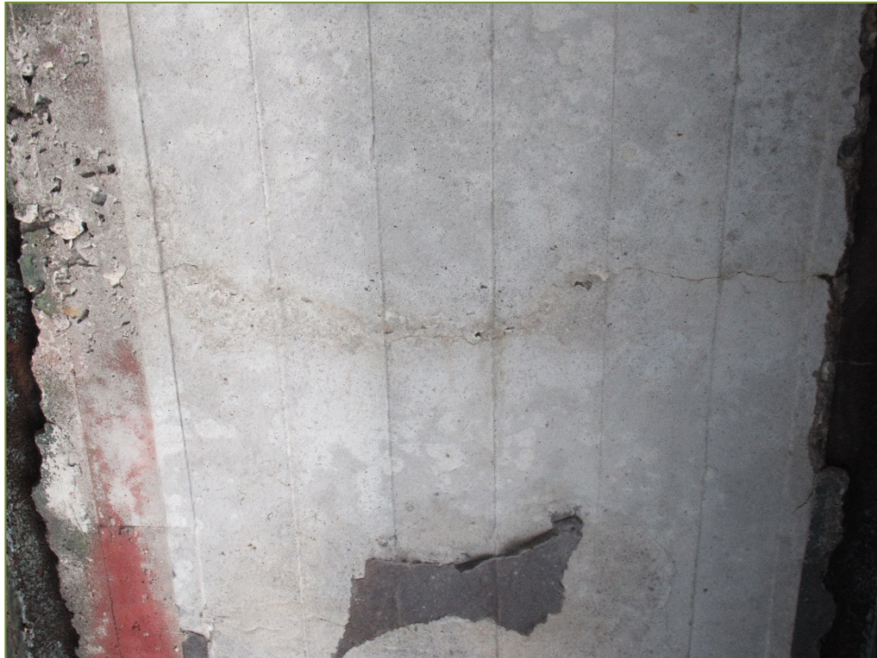
Photo P16 Soffit between West Abutment and Pier between 4 th and 5 th Girder (crack, and honeycombing)
