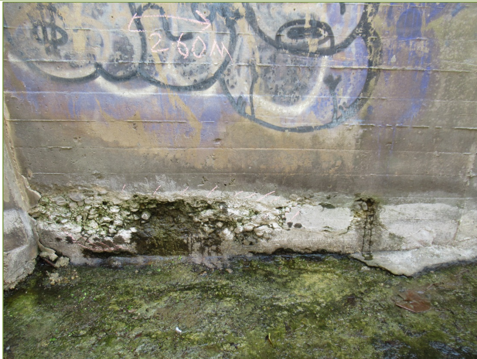
Photo P20 Outlet – South Wall (spall and delamination) note, exposed rebar
