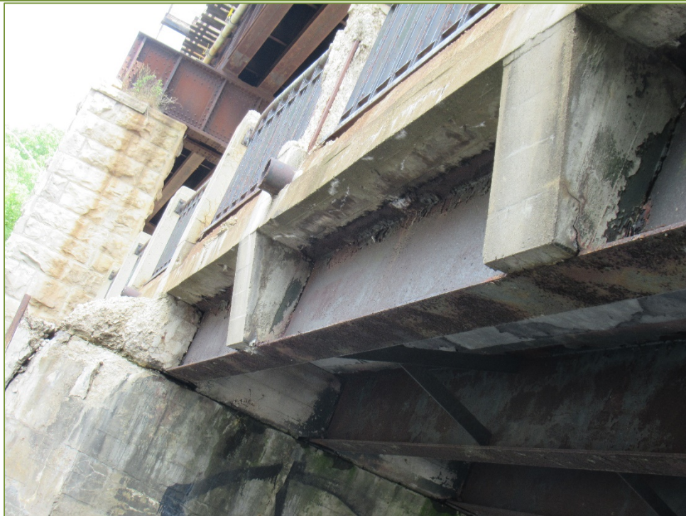
Photo P18 Soffit between West Abutment and Pier, north edge (cracks, and delamination) and Girders (light corrosion)
