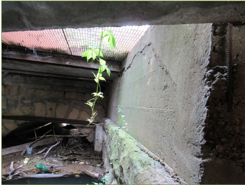
Photo P7 Inlet- West Wall (wide crack, spall, delamination and medium scaling)
