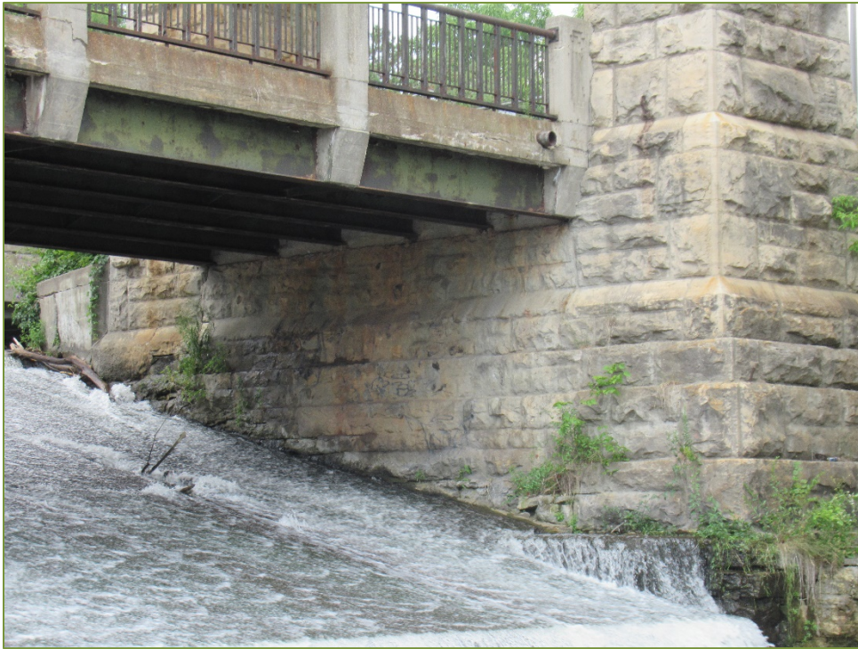
Photo P55 East Abutment – Masonry Wall
