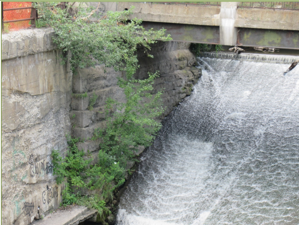
Photo P56 West Abutment – Masonry Wall (cracks, and spall)
