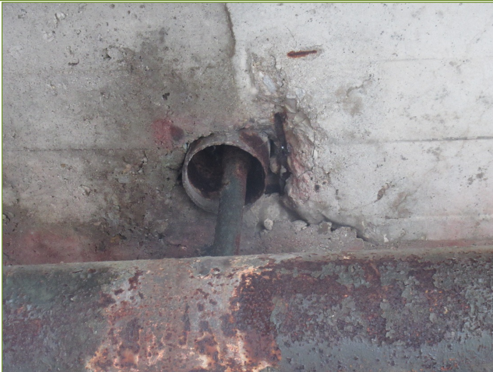
Photo P10 Soffit at West Abutment, south edge (spall, and delamination) note, light corrosion on utility duct
