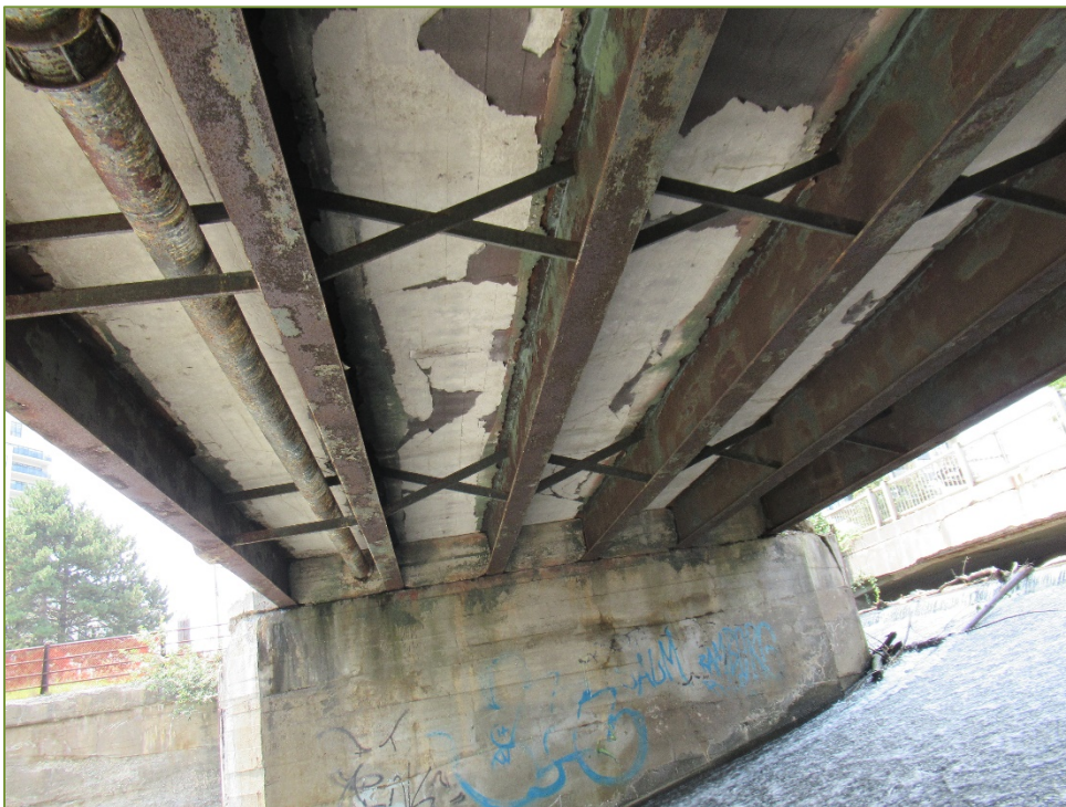
Photo P26 Soffit between Pier and East Abutment (fair condition – cracks, spall, delamination and honeycombing) and Girders (fair condition – light to severe corrosion)
