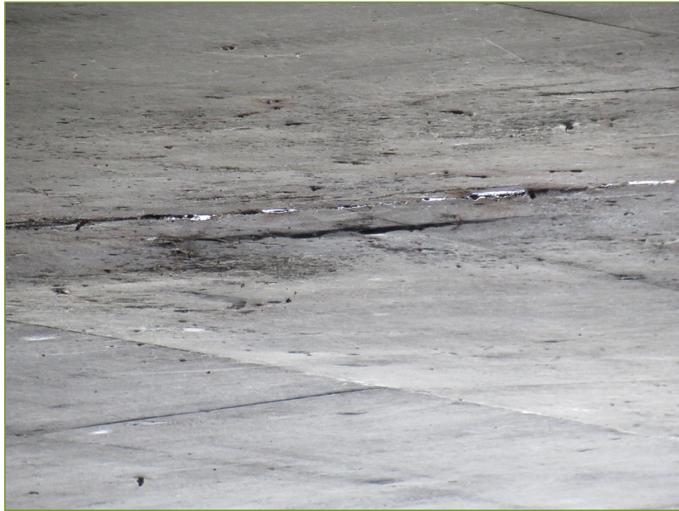
Photo P15 Soffit between East Abutment and Pier (cracks, spall, delamination, and wet area)
