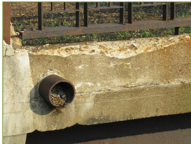
Typical Condition of North Deck Drainage
