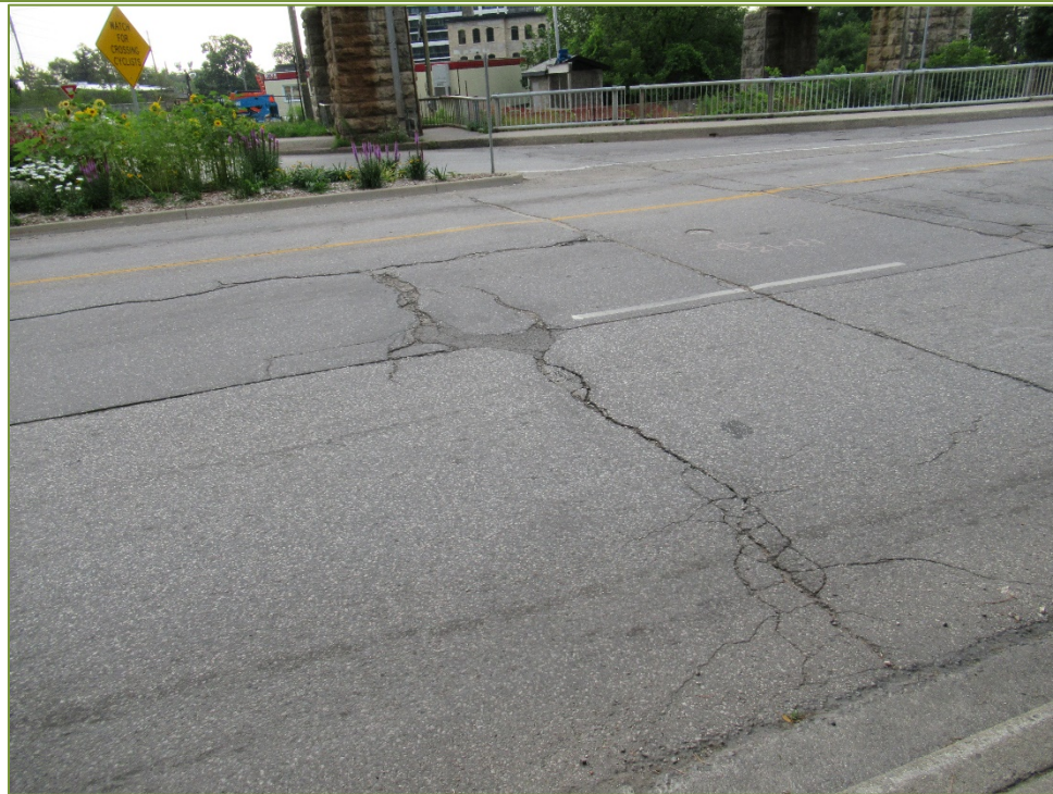
Photo P26 East Approach Wearing Surface (fair condition - unsealed cracks, and pot holes)
