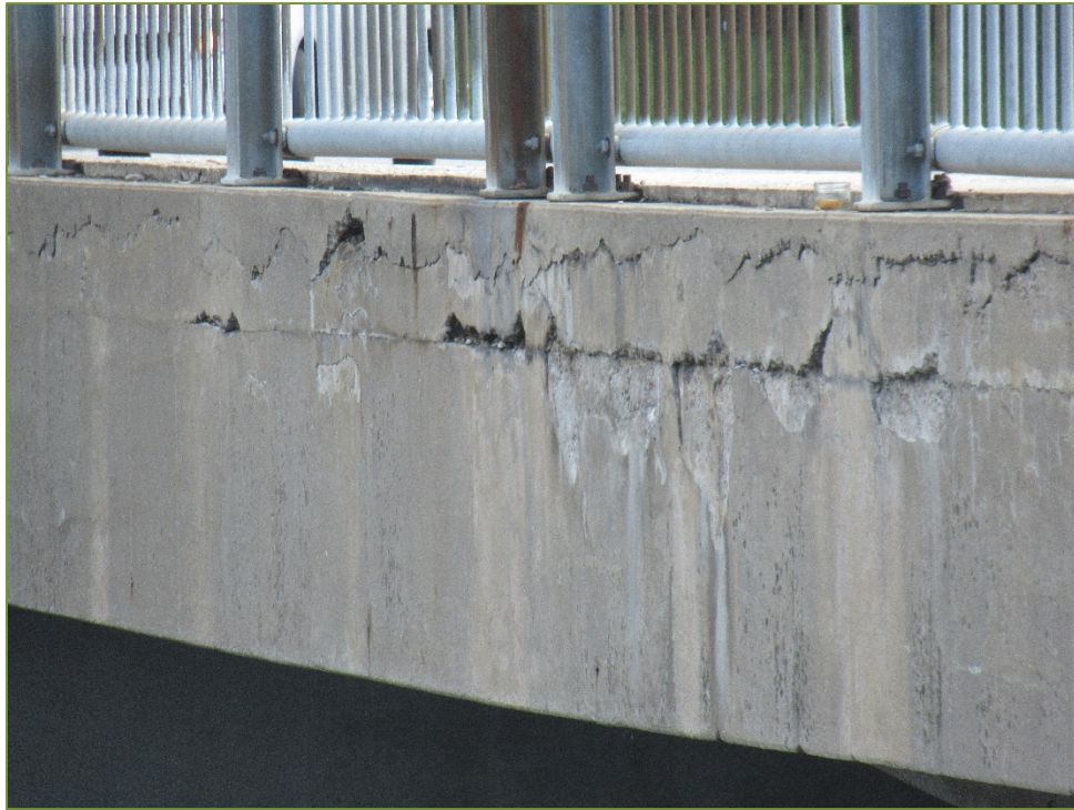
Photo P23 North Elevation – Fascia, east span (wide cracks, spall and delamination)
