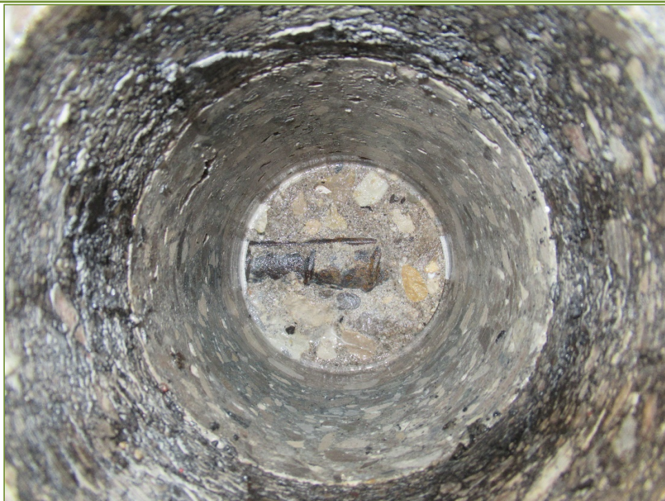
Photo P64 Typical Condition of Inside Core – C5
