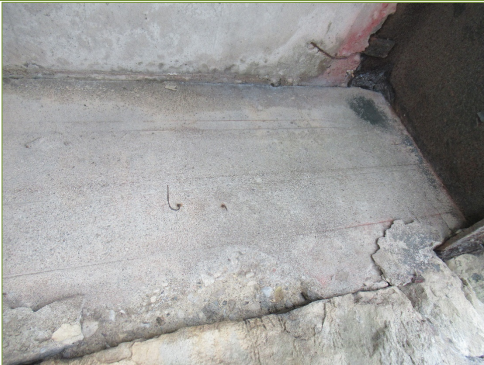
Photo P60 West Diaphragm, north side (spall, delamination, and light scaling)
