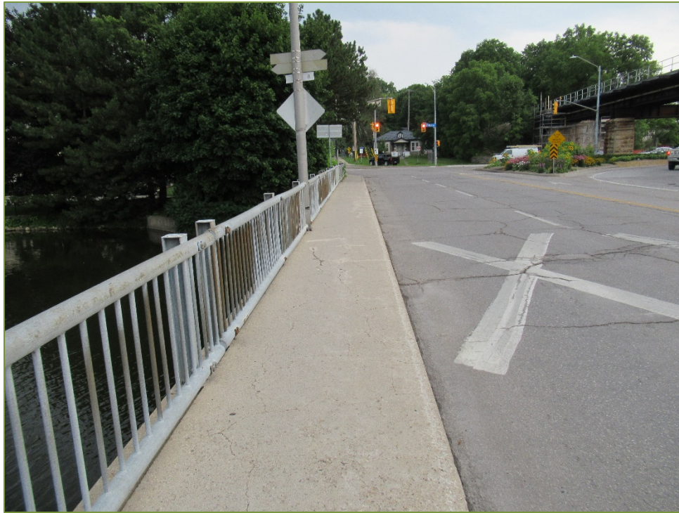
Photo P37 North Sidewalk (cracks, delamination, and medium scaling) and Handrail (light corrosion)
