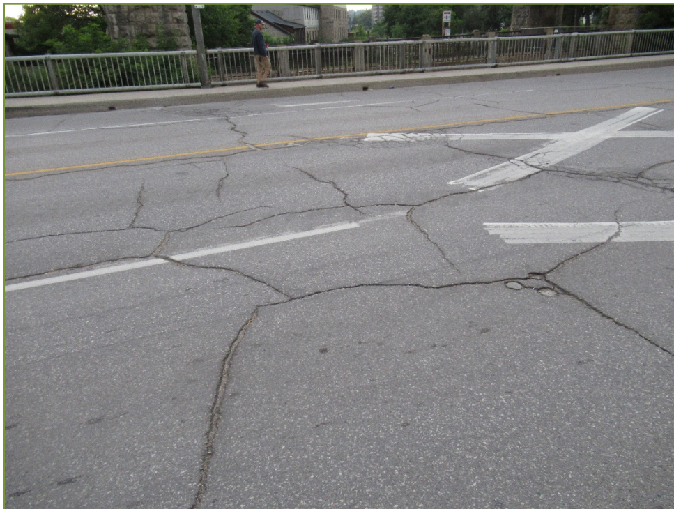
Photo P6 Deck Wearing Surface (unsealed cracks)
