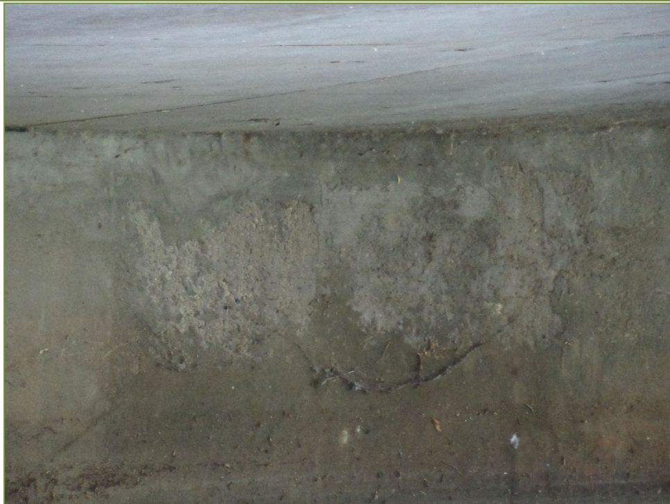
Photo P58 Pier - East Face (light scaling)
