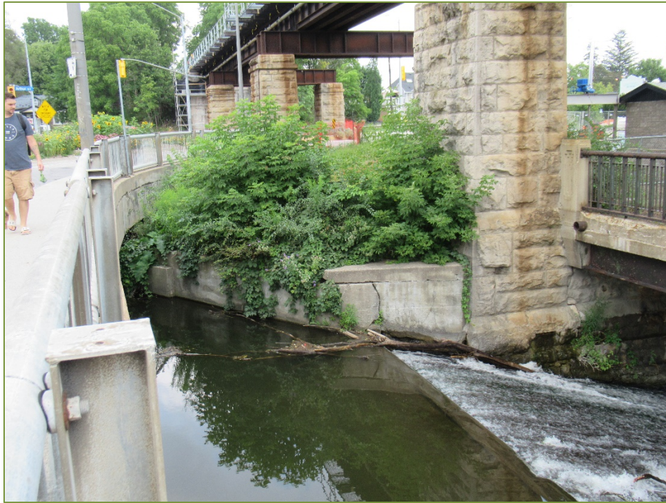
Photo P65 Northeast Retaining Wall (fair to poor condition – wide cracks, spall, and light scaling)
