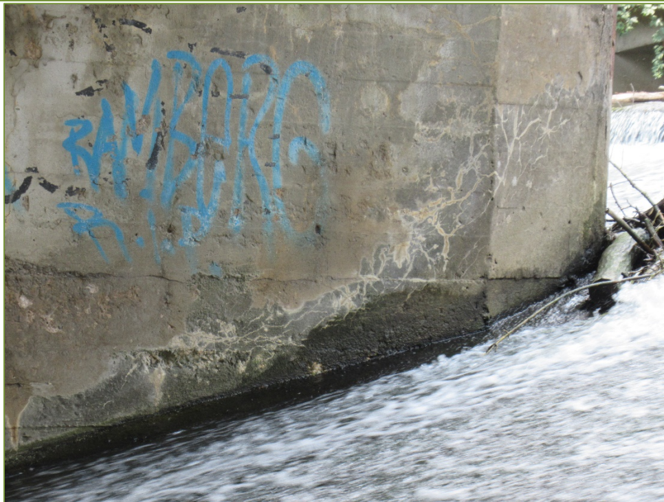
Photo P72 Pier - East Face, north side (cracks, spall, light to medium scaling, and wet area)
