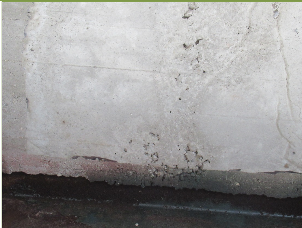
Photo P34 Soffit between at East Abutment (crack and honeycombing)
