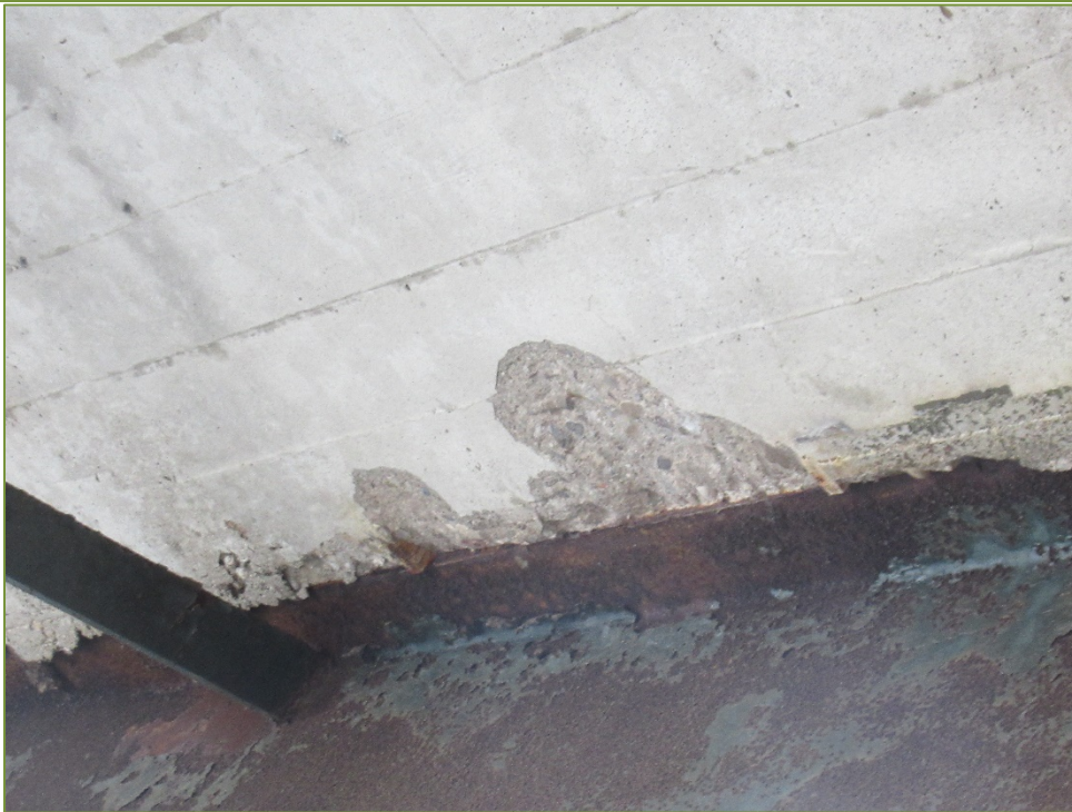
Photo P32 Soffit between Pier and East Abutment, north side (crack, spall, and delamination) and Girders (light corrosion)
