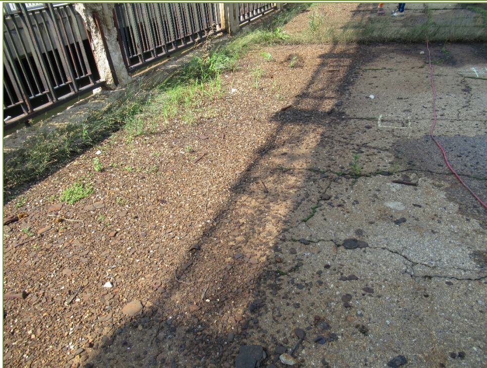
Photo P6 Deck Wearing Surface (unsealed cracks, and raveling) note vegetation growth and debris
