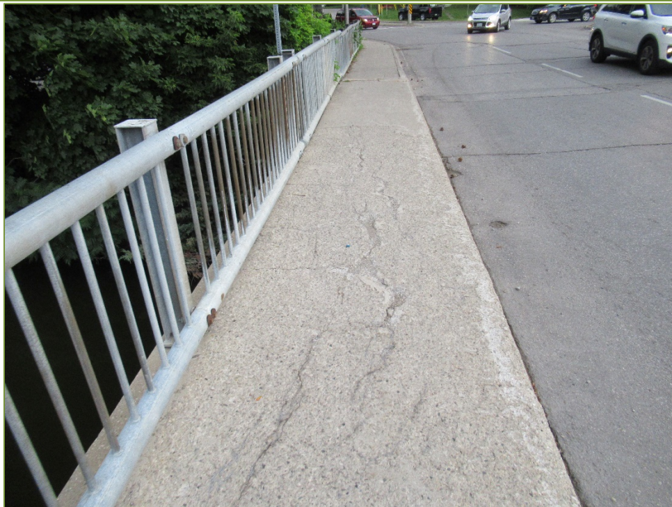
Photo P38 North Sidewalk (cracks, spall, delamination, and severe scaling) and Handrail (light corrosion)
