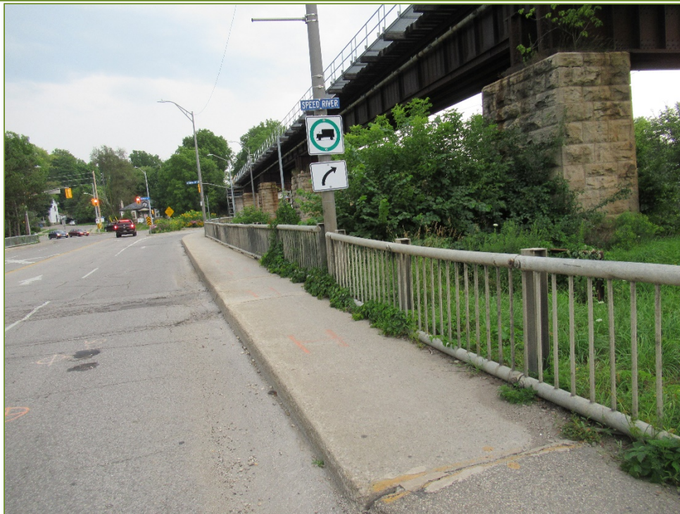
Photo P42 South Sidewalk (fair condition – wide cracks and light to medium scaling) and Handrail (fair condition - light corrosion)
