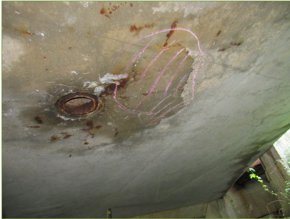
Photo P17 Soffit between East Abutment and Pier, south side (cracks, spall, delamination, and wet area) note, drain is discharging directly onto soffit
