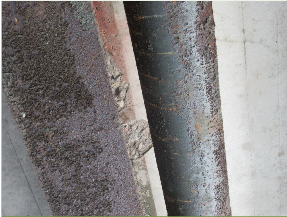
Photo P11 Soffit at West Abutment, south edge (spall, and delamination) and Girder (light corrosion)
