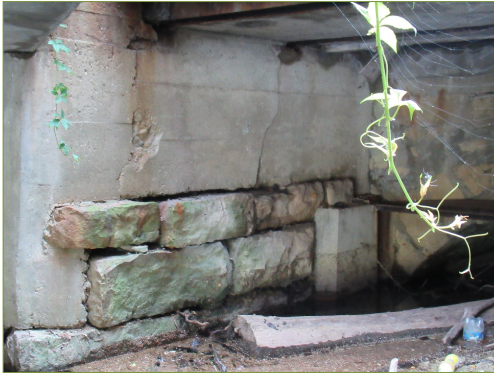
Photo P5 Inlet – East Wall (wide crack, spall, delamination, and light to medium scaling)
