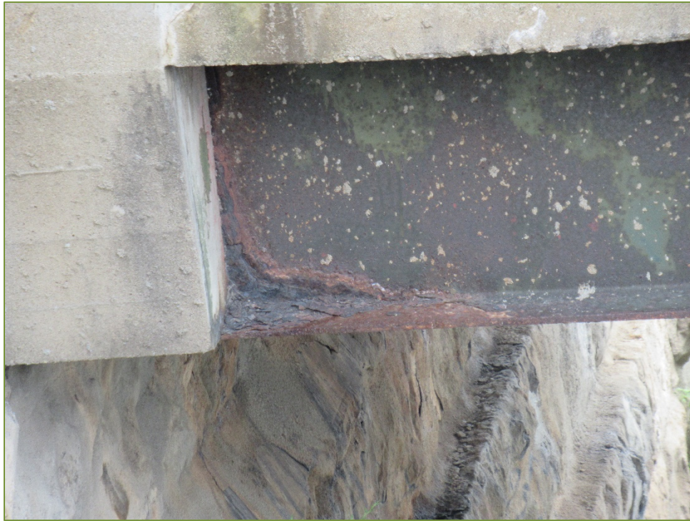
Photo P35 1 st Girder from North at East Abutment (severe corrosion on top flange)
