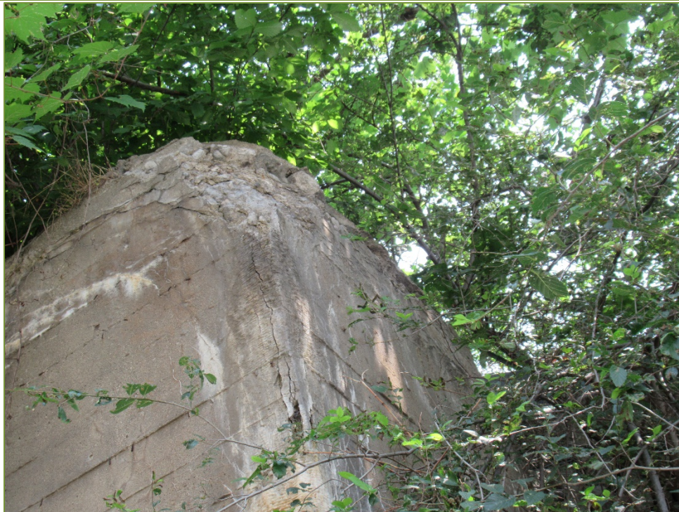
Photo P10 Outlet – West Elevation, South side (cracks, spall, and delamination)
