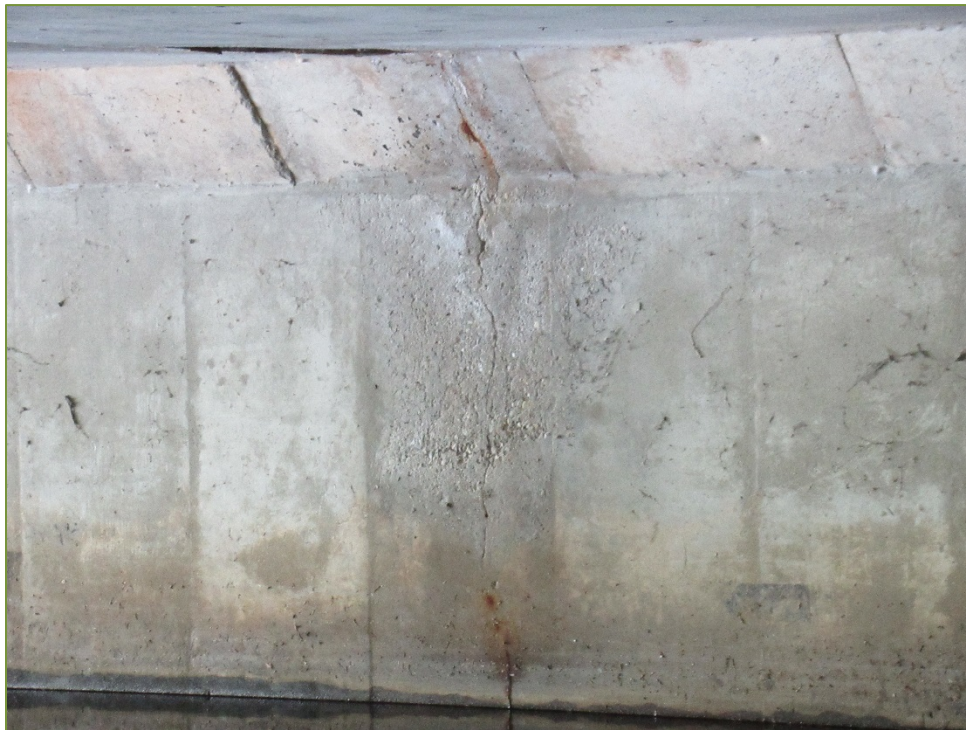
Photo P47 East Abutment (cracks, light to medium scaling, and wet area)
