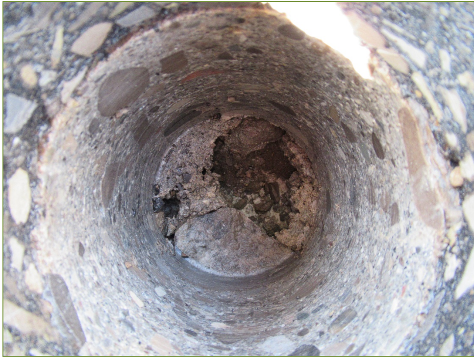
Photo P79 Typical Condition of Inside Core – C7 (East Approach)
