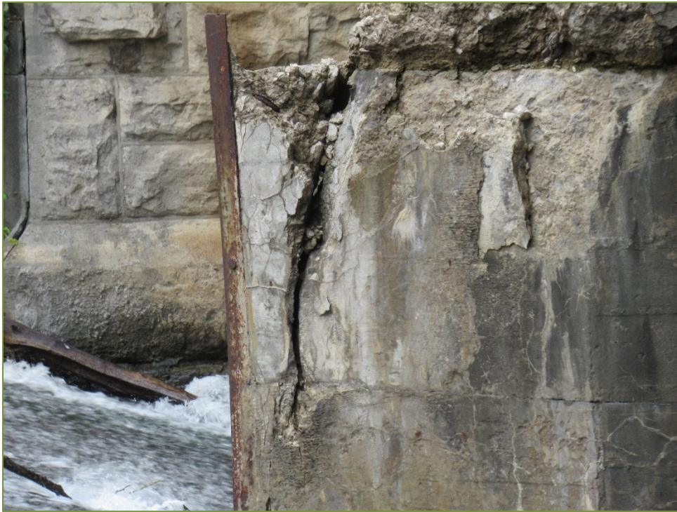
Photo P77 Pier - West Face, north side (cracks, spall, and delamination) note, exposed rebar)
