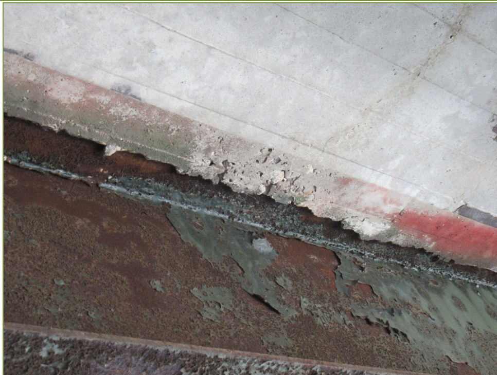
Photo P12 Soffit at West Abutment (honeycombing) and Girder (light corrosion)
