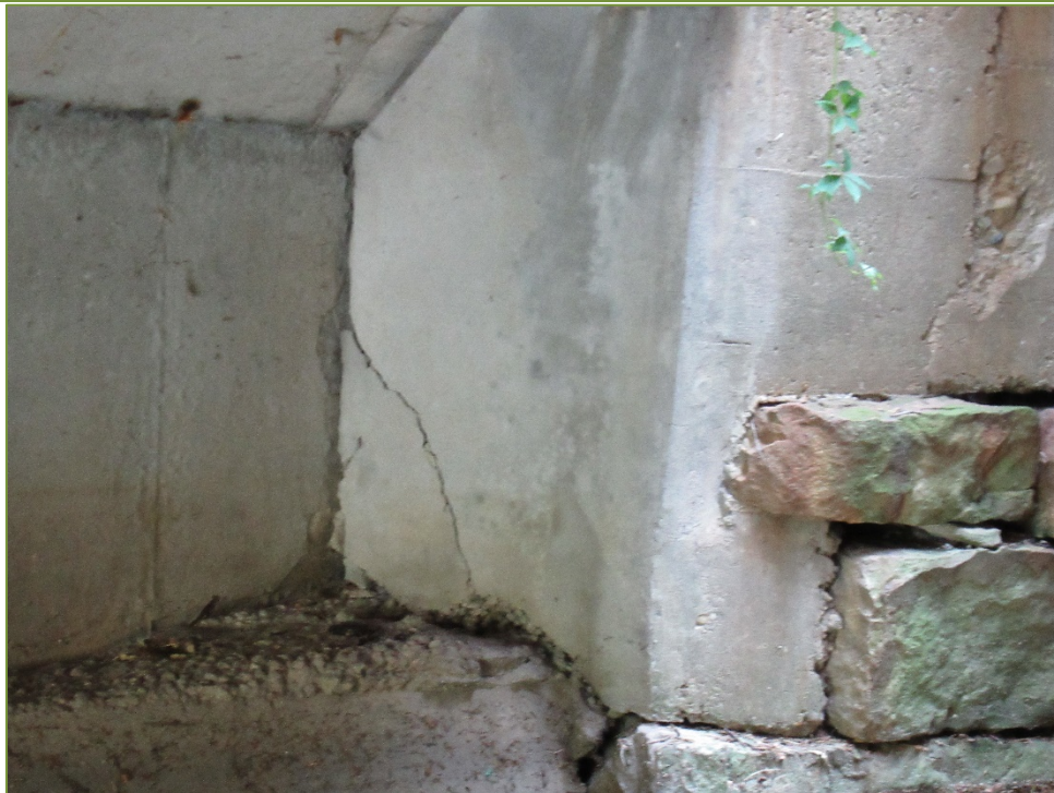
Photo P2 Inlet – North Elevation, East Wall (wide crack)
