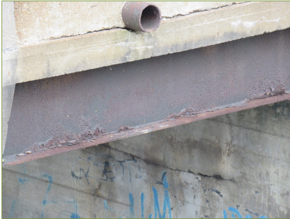
Photo P37 1 st Girder from North at Pier (severe corrosion on top flange)
