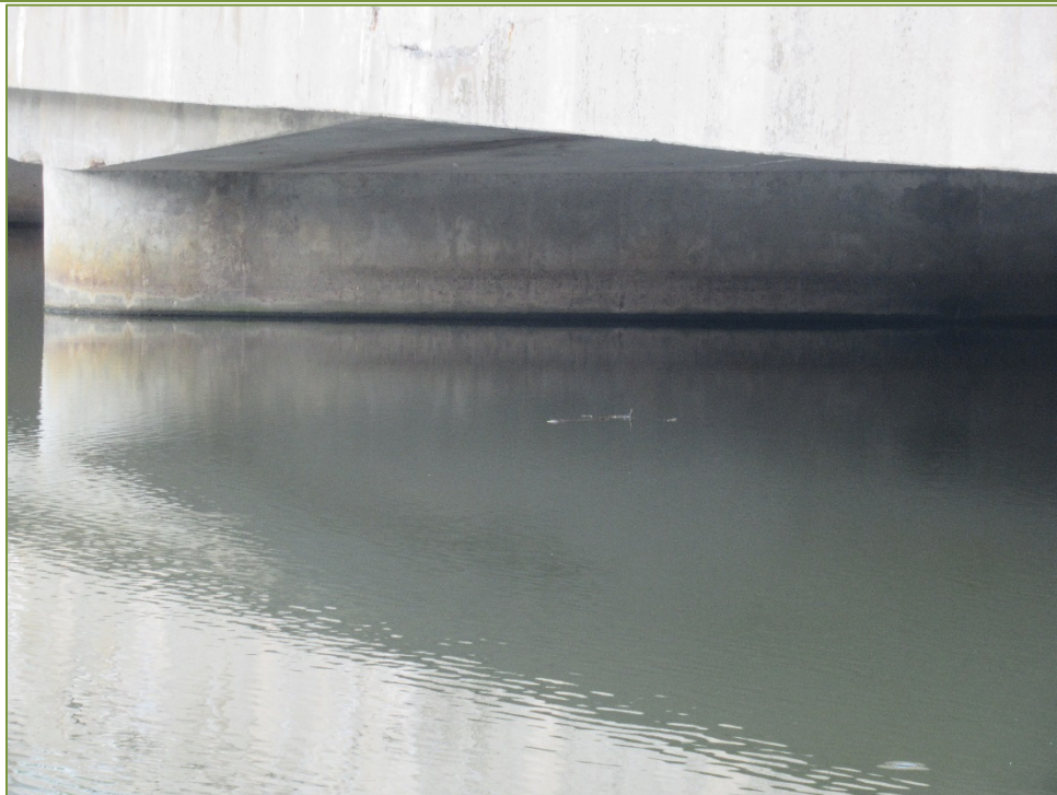
Photo P60 Pier - West Face (cracks, and light scaling)
