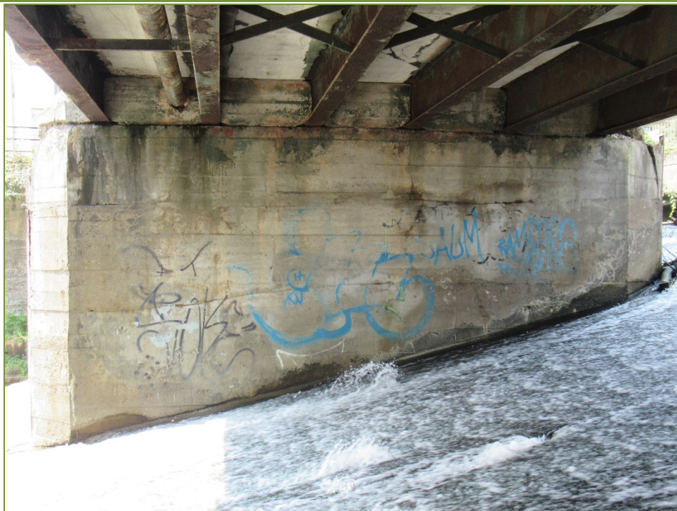
Photo P70 Pier - East Face (fair to poor condition - cracks, spall, delamination, light to medium scaling, and wet area)
