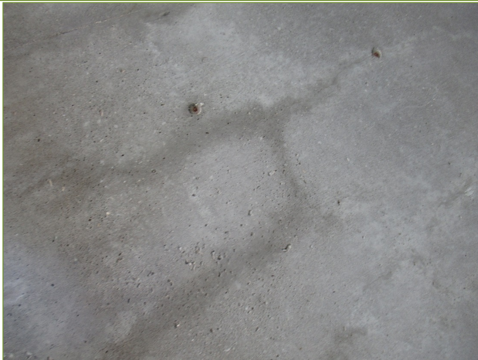
Photo P12 Soffit between East Abutment and Pier (cracks and light scaling)
