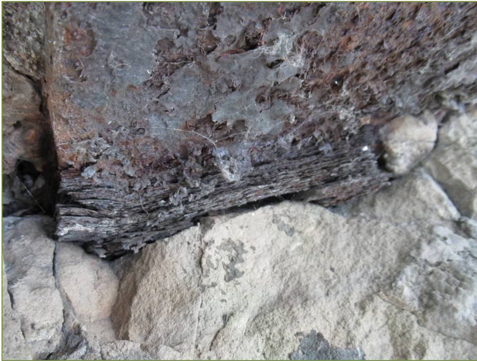
Photo P23 1 st Girder from North at West Abutment (severe corrosion)
