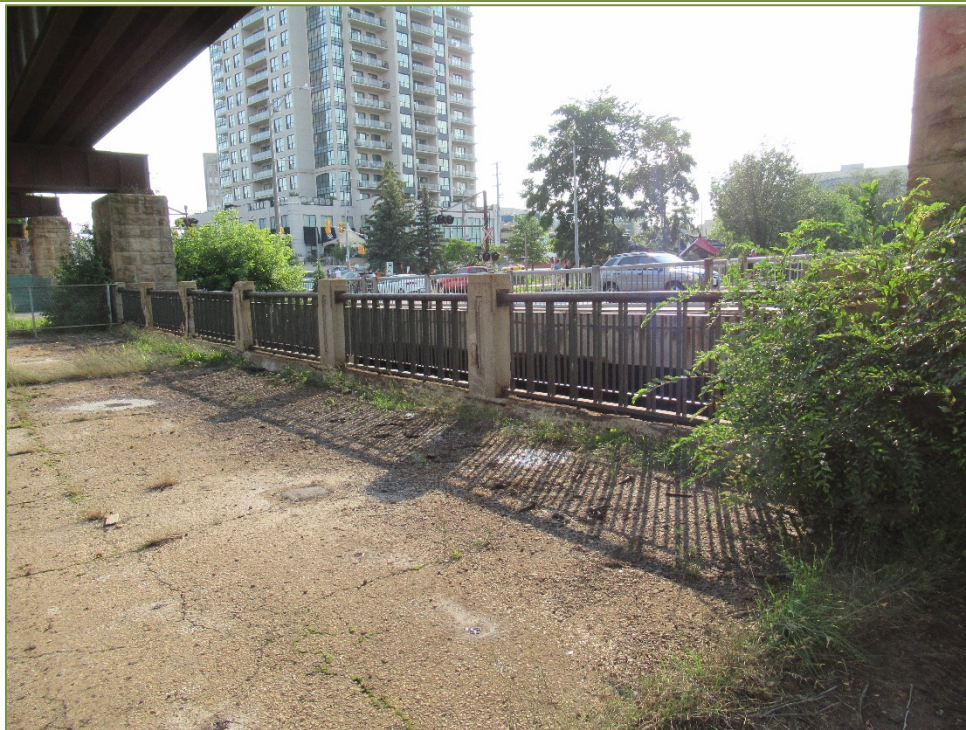
Photo P46 North Curb (poor condition – cracks, spall, delamination, and medium to severe scaling) Concrete Posts (fair to poor condition – cracks, spall, delamination, and light scaling) and Handrail (fair condition – light corrosion)
