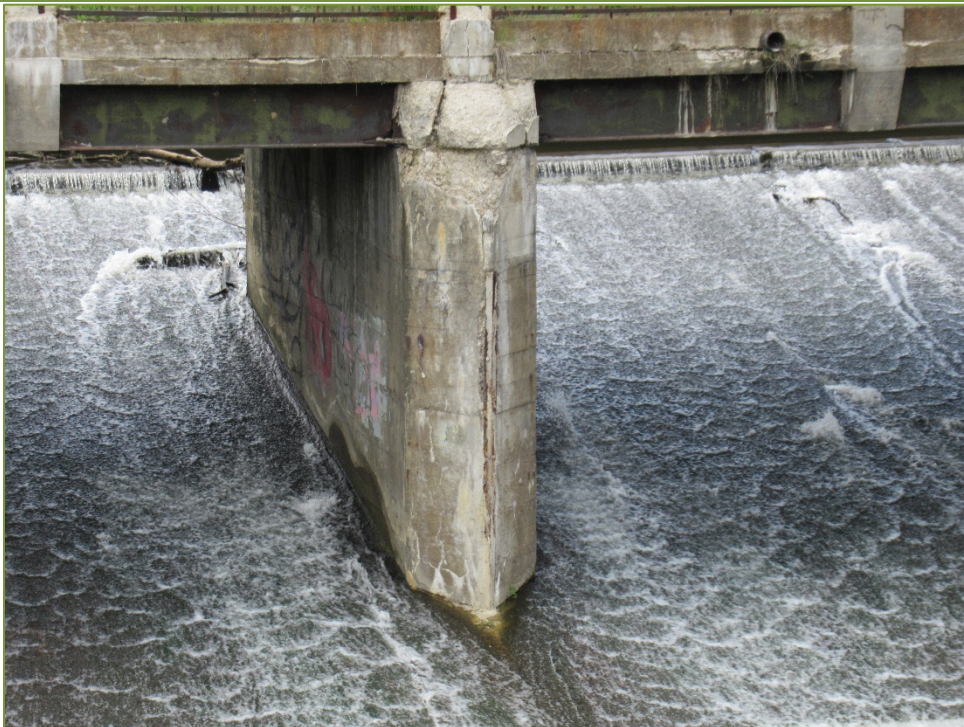
Photo P78 Pier - South Face (cracks, spall, and delamination)
