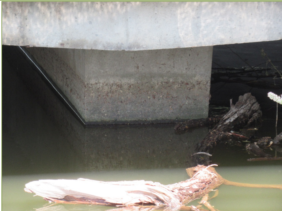
Photo P62 Pier - South Face (medium scaling)
