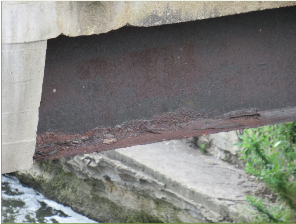
Photo P21 1 st Girder from North at Pier (severe corrosion on flange)
