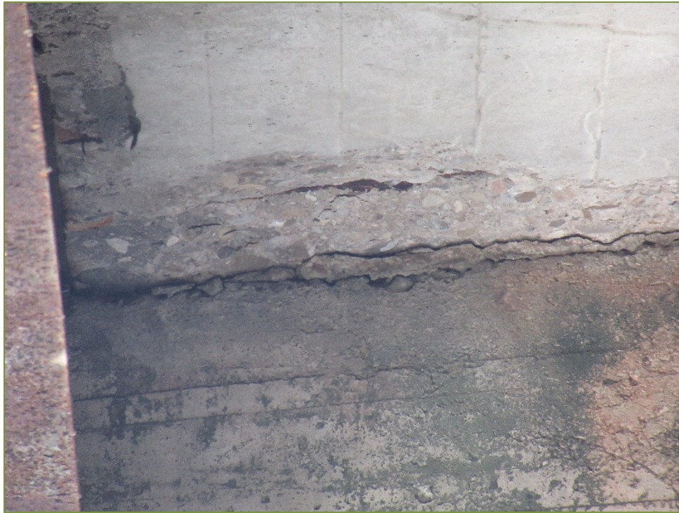
Photo P27 Soffit at Pier, south edge (spall)
