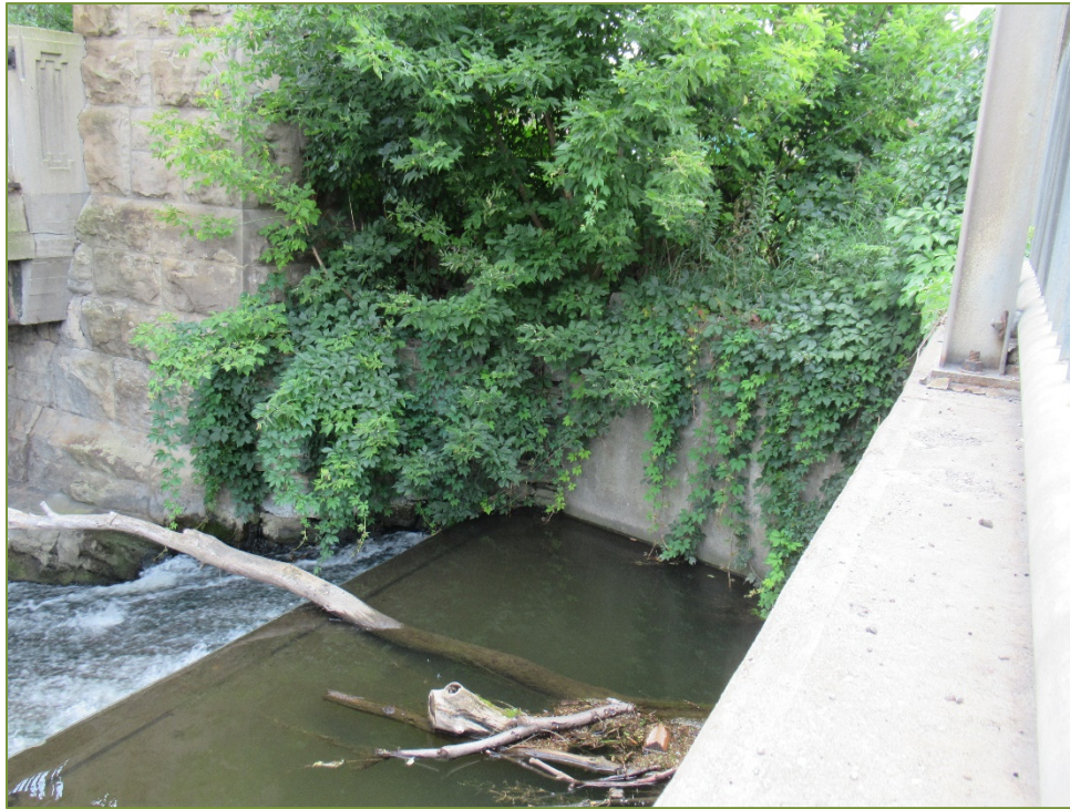
Photo P67 Northwest Retaining Wall (fair to good condition – cracks, and light scaling)
