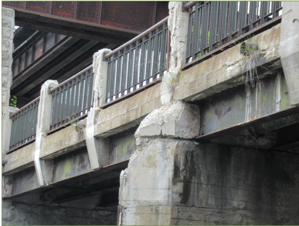
Photo P43 South Elevation – Fascia (cracks, spall, delamination, and light scaling)
