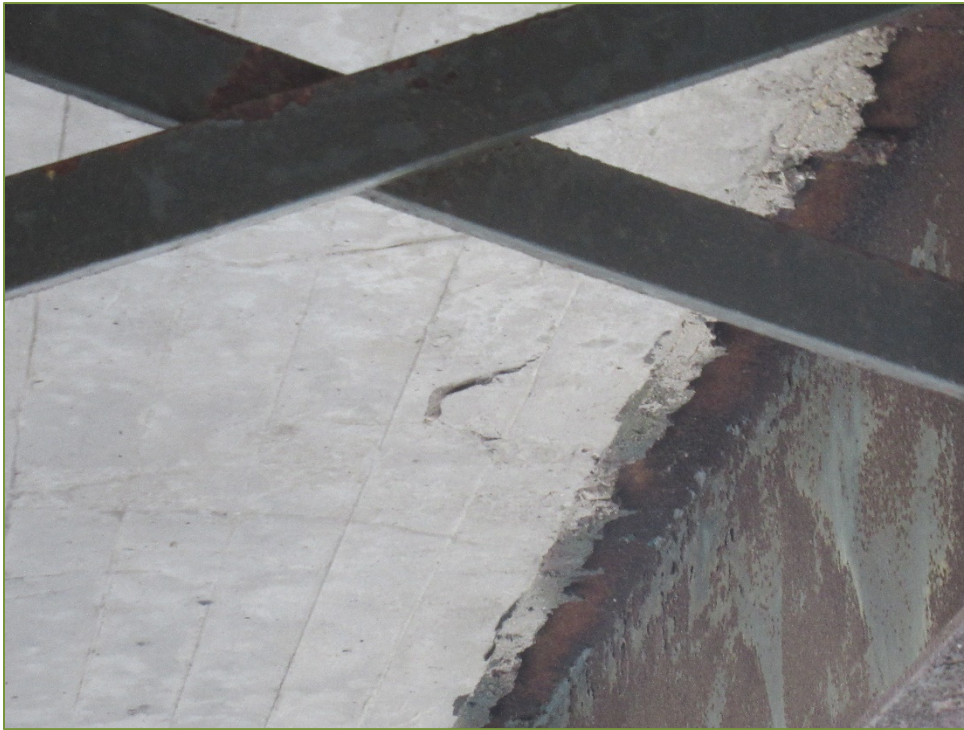
Photo P31 Soffit between Pier and East Abutment between 1 st and 2 nd Girder from North (delamination) and Girders (light corrosion)
