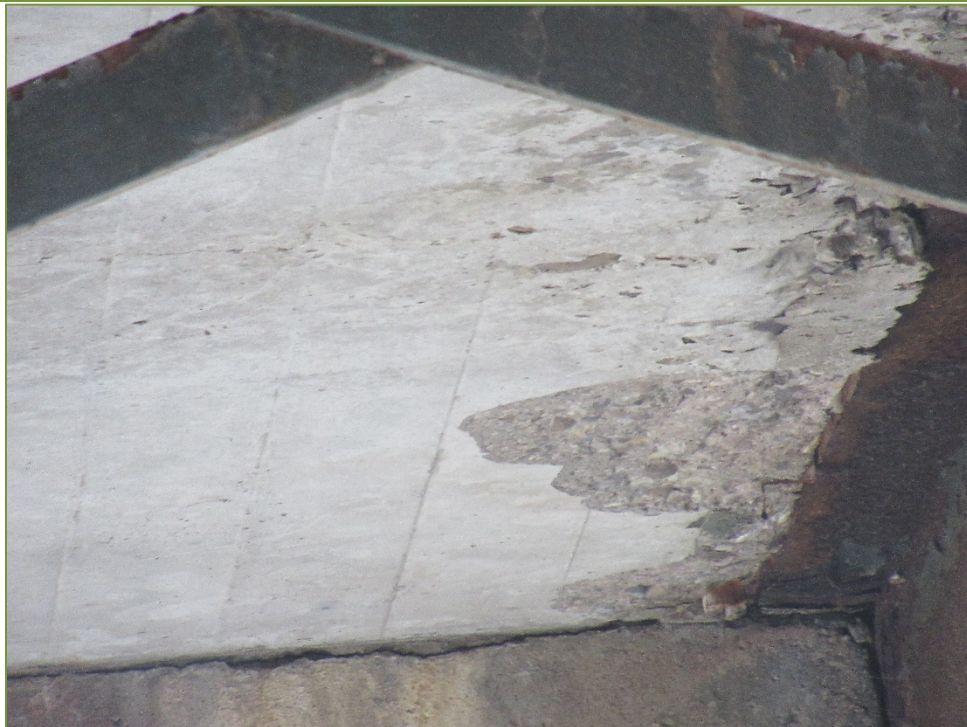
Photo P28 Soffit at Pier, north edge (crack, spall, and delamination)
