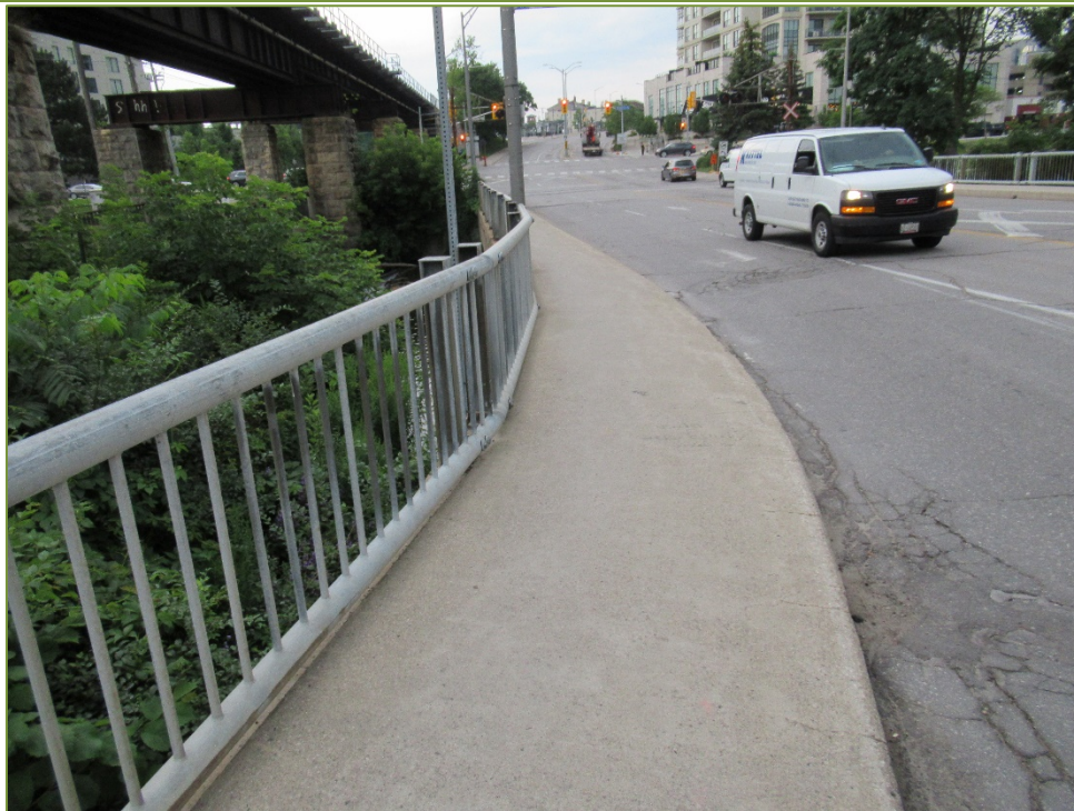
Photo P44 South Sidewalk (cracks and light to medium scaling) and Handrail (light corrosion)
