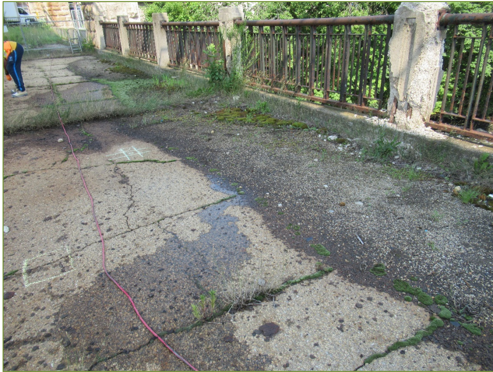
Photo P7 Deck Wearing Surface (unsealed cracks, and raveling) note vegetation growth and debris
