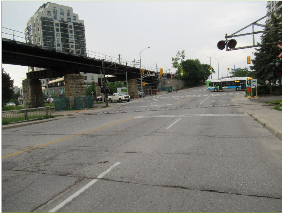
Photo P27 West Approach Wearing Surface (fair to poor condition - unsealed cracks, and pot holes)
