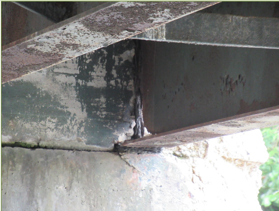
Photo P22 6 th Girder from North at Pier (severe corrosion, and section loss)
