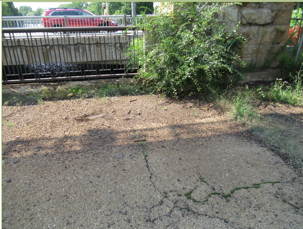
Photo P8 Deck Wearing Surface (unsealed cracks, and raveling) note vegetation growth and debris
