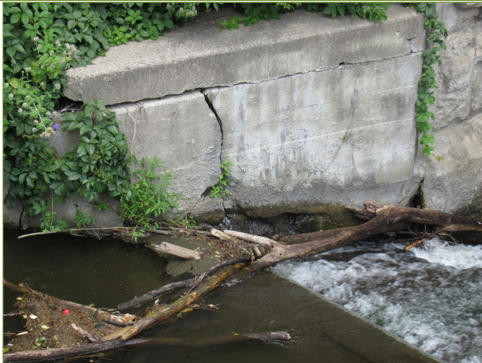
Photo P66 Northeast Retaining Wall (wide cracks and spall)
