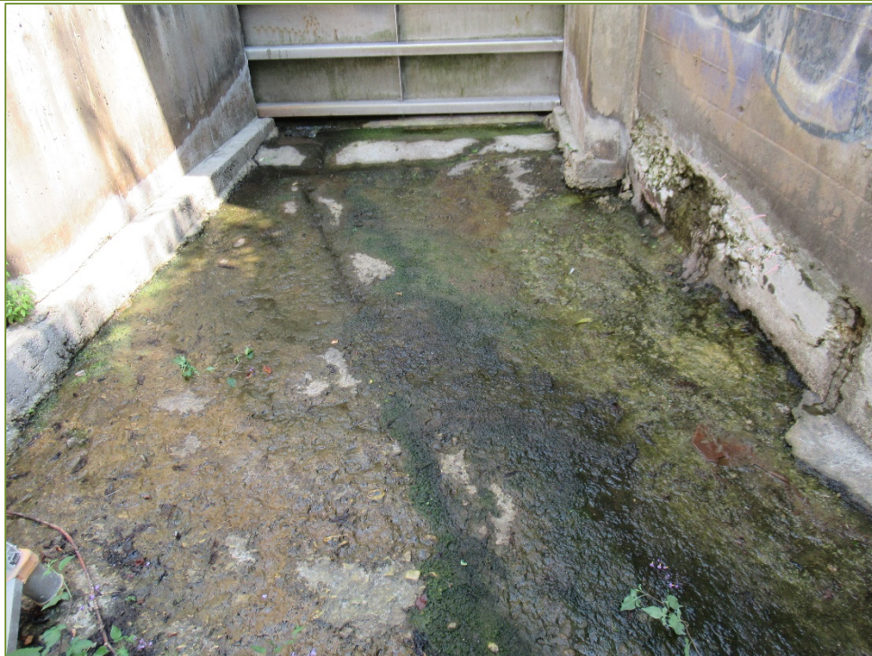
Photo P22 Outlet – Floor (cracks, and medium to severe scaling)
