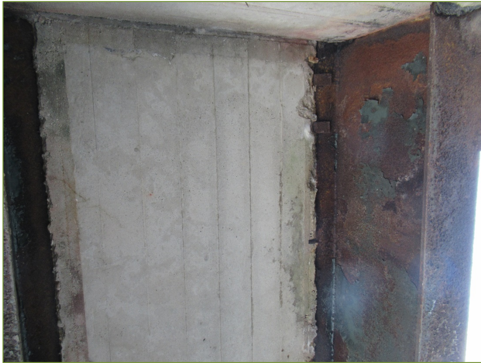
Photo P33 Soffit between at East Abutment (crack, spall, and delamination) and Girders (light to medium corrosion)
