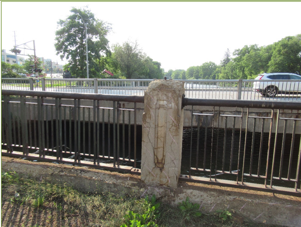
Photo P48 North Curb (cracks, spall, delamination, and medium to severe scaling) Concrete Posts (cracks, spall, delamination, and light scaling) and Handrail (light corrosion)
