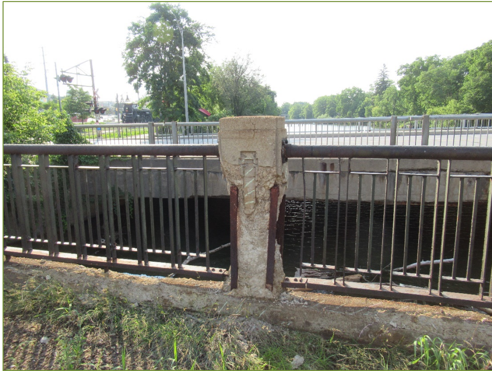
Photo P49 North Curb (cracks, spall, delamination, and medium to severe scaling) Concrete Posts (cracks, spall, delamination, and light scaling) and Handrail (light corrosion)
