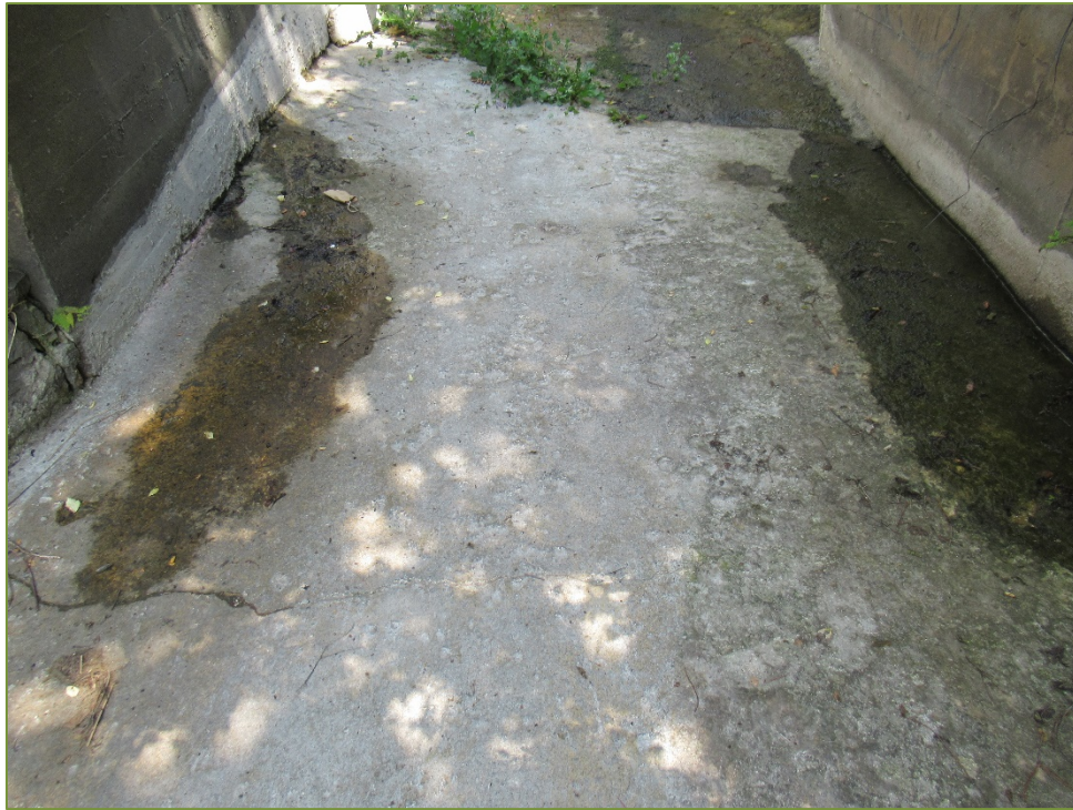
Photo P21 Outlet – Floor (cracks, and medium to severe scaling)
