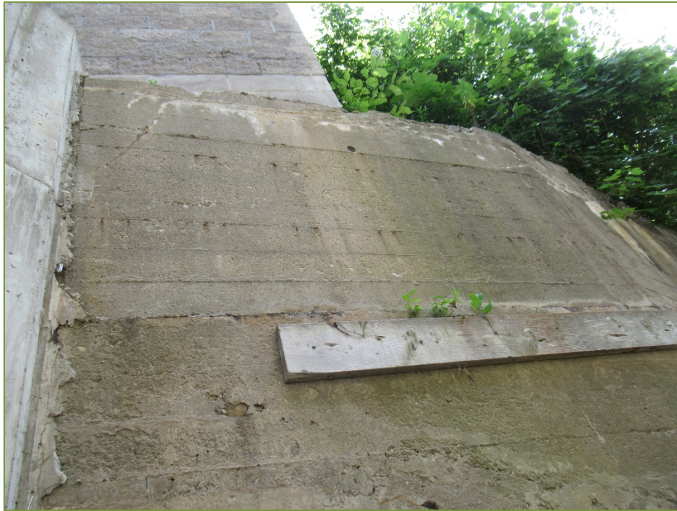
Photo P19 Outlet – South Wall (cracks, spall, delamination, and medium scaling)
