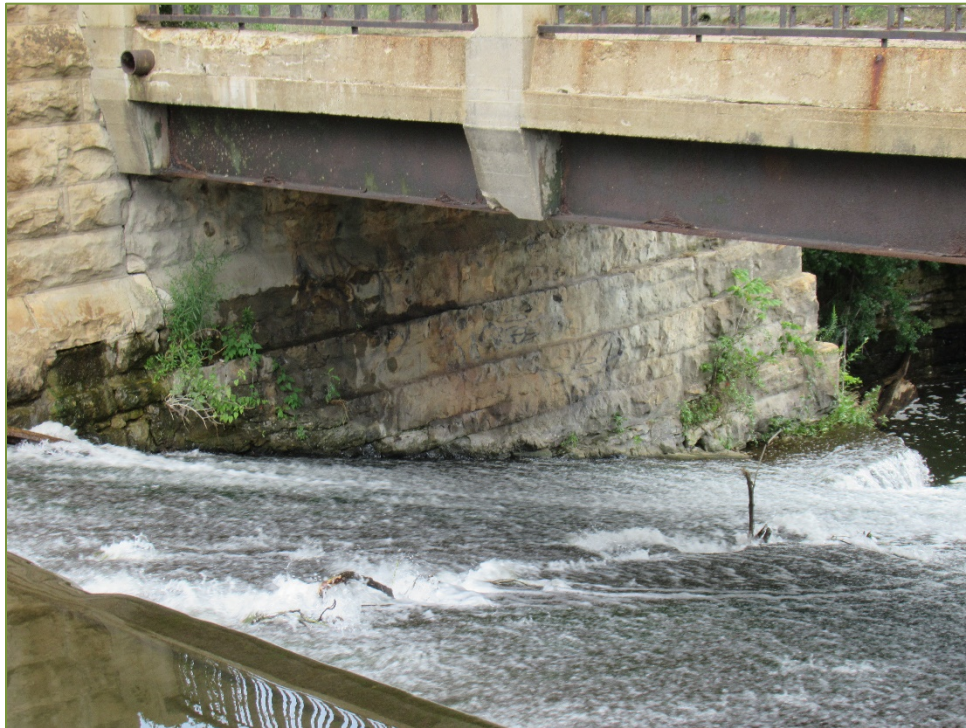
Photo P54 East Abutment – Masonry Wall (cracks, spall and wet area)
