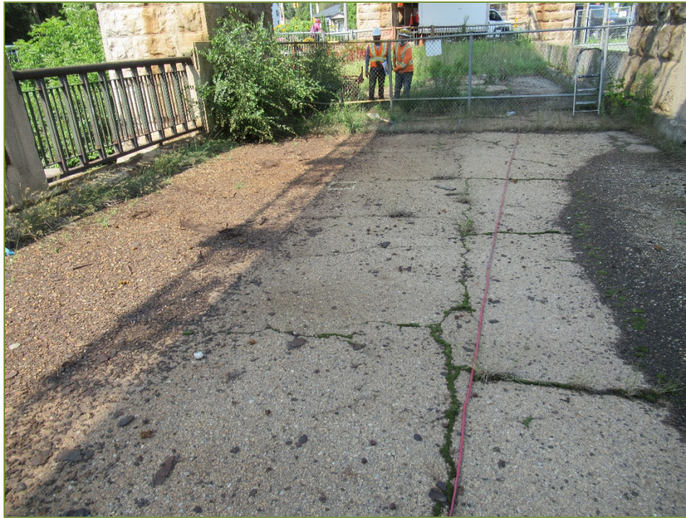
Photo P5 Deck Wearing Surface (poor condition – unsealed cracks, and raveling) note vegetation growth and debris
