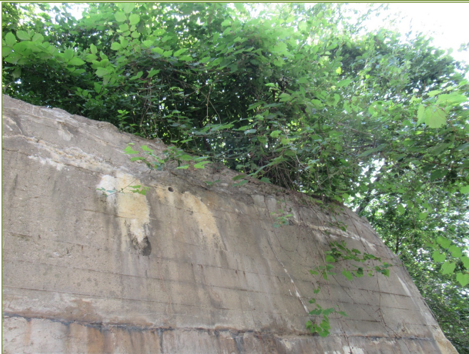
Photo P18 Outlet – South Wall (cracks, spall, delamination and medium scaling)
