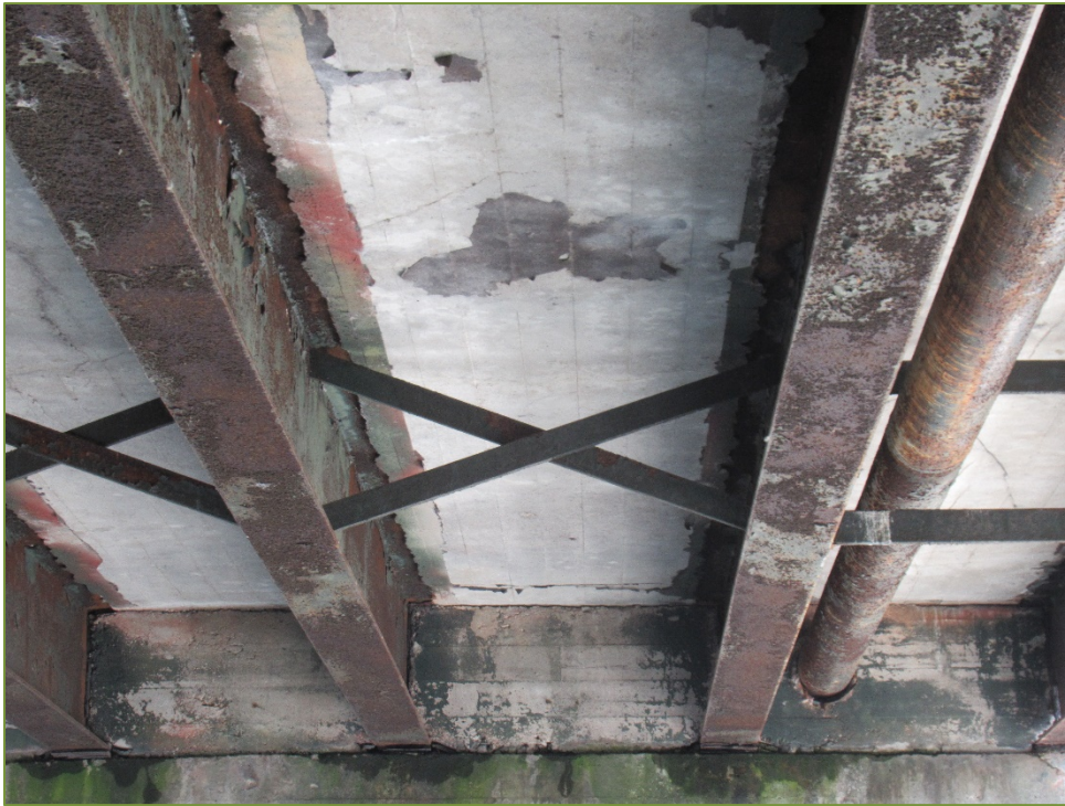
Photo P19 Soffit at Pier (cracks) and Girders (light corrosion)
