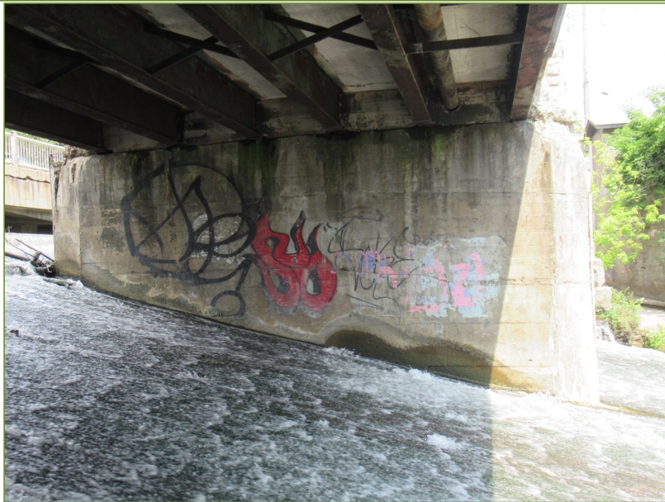
Photo P74 Pier - West Face (fair to poor condition - cracks, spall, delamination, light to medium scaling, and wet area)
