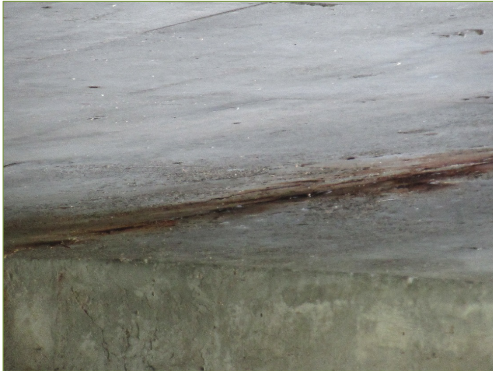
Photo P14 Soffit at Pier (cracks, spall, delamination, and wet area)
