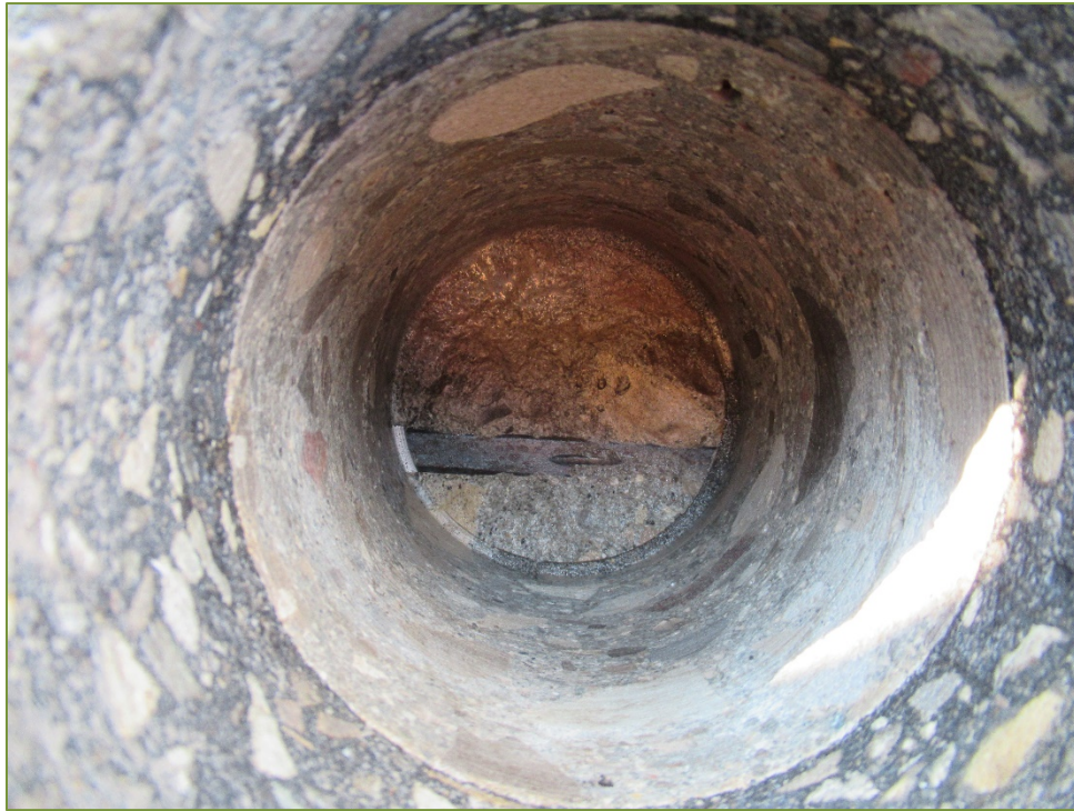
Photo P81 Typical Condition of Inside Core – C2
