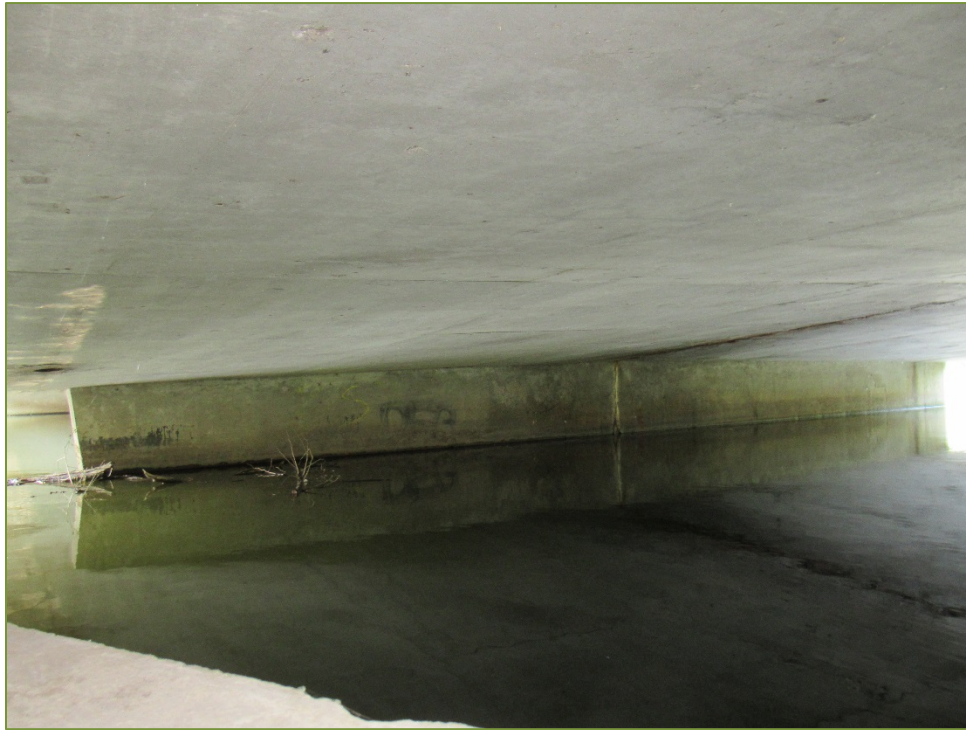
Photo P57 Pier - East Face (fair to good condition - crack and light scaling)
