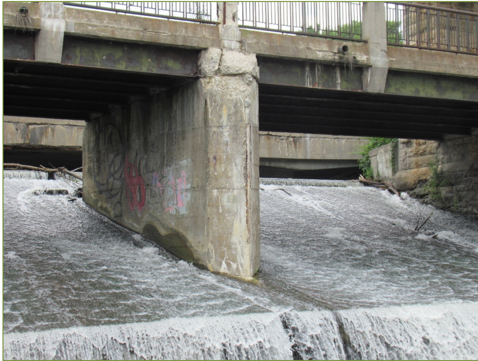
Photo P73 Pier – East Face, south side (cracks, spall, delamination, light to medium scaling, and wet area)
