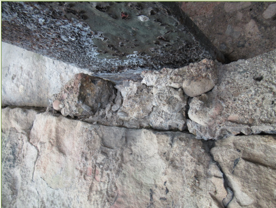
Photo P24 2 nd Girder from North at West Abutment (severe corrosion)
