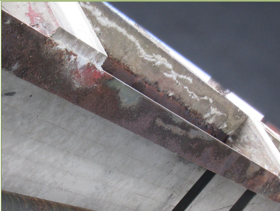
Photo P20 Soffit between West Abutment and Pier, south edge (cracks, and delamination) and Girders (light corrosion)
