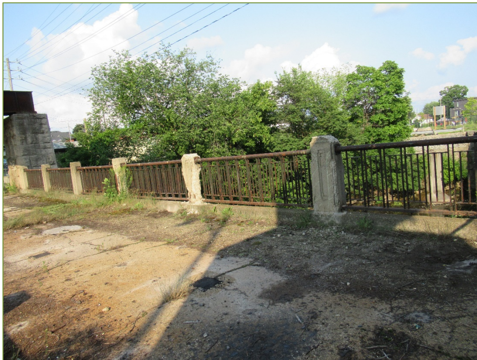
Photo P50 South Curb (fair condition – cracks, spall, delamination, and medium scaling) Concrete Posts (fair to poor condition – cracks, spall, delamination, and light scaling) and Handrail (fair condition – light corrosion)
