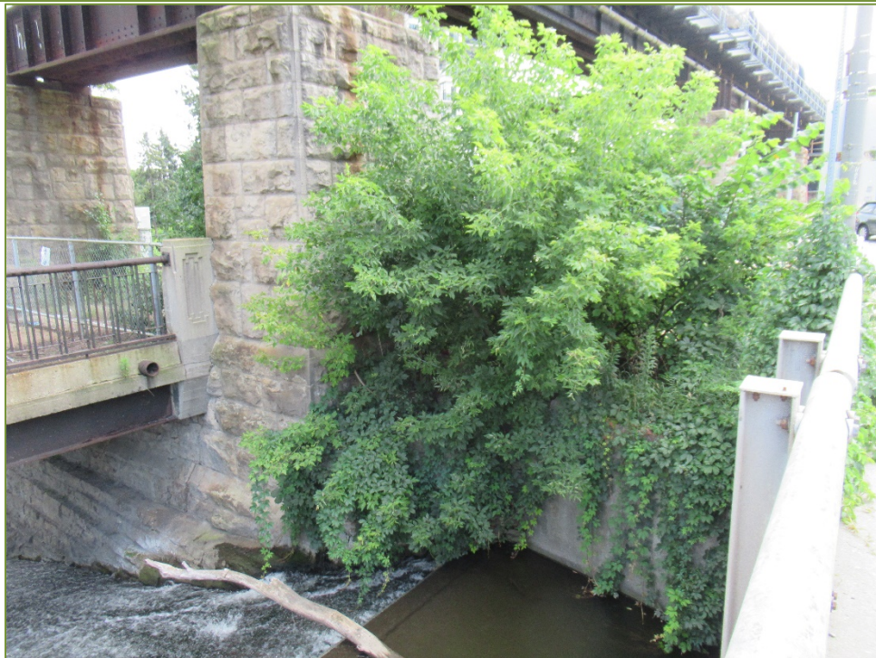
Photo P62 Northwest Wingwall – Masonry Wall
