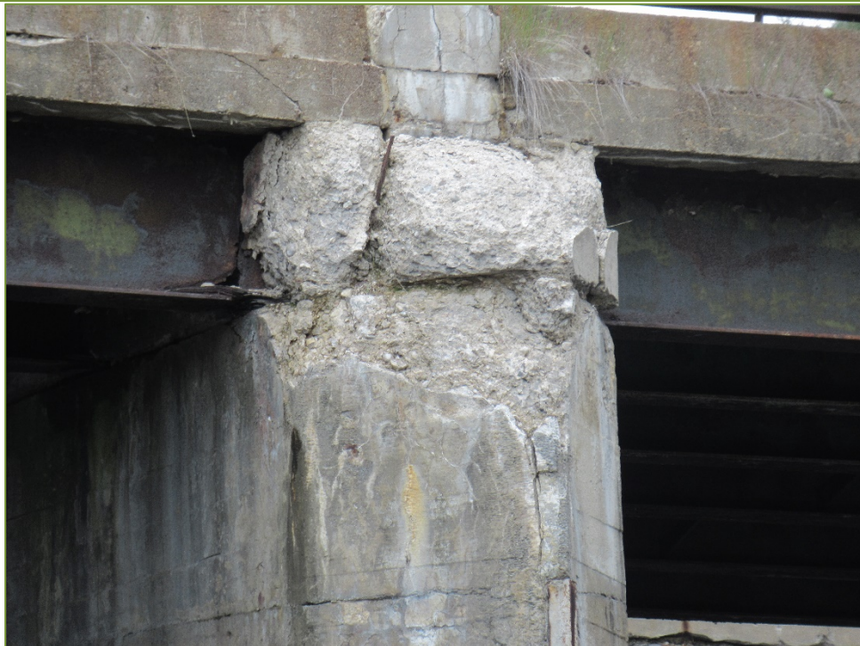
Photo P76 Pier - West Face, south side (cracks, spall, and delamination)
