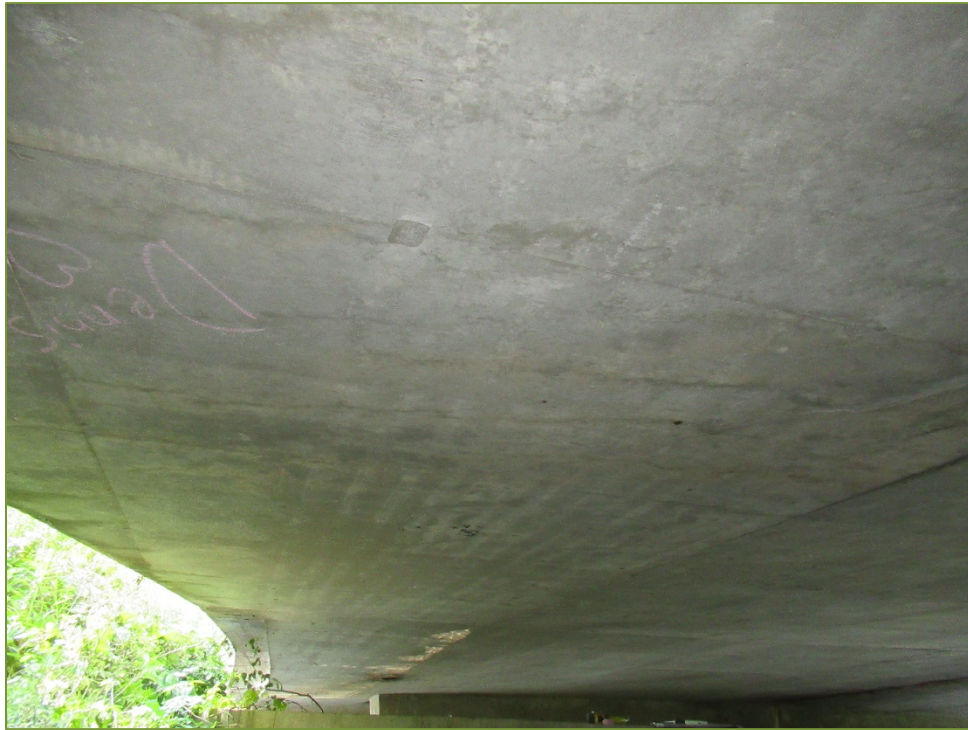
Photo P11 Soffit between East Abutment and Pier (fair condition – cracks, spall, delamination, light scaling, and wet area)
