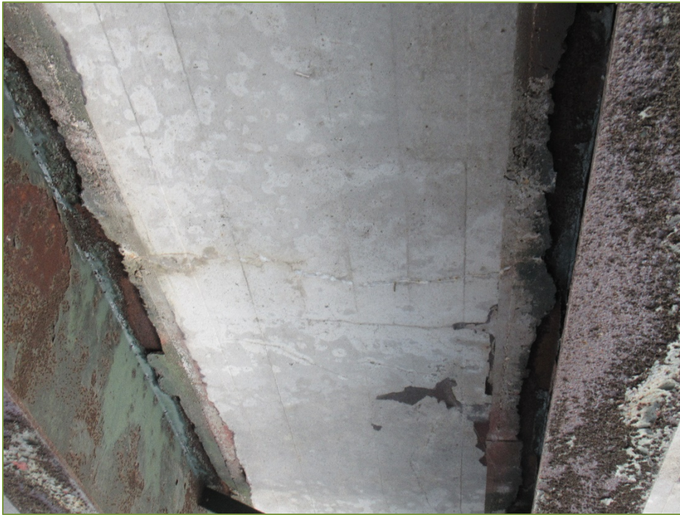
Photo P13 Soffit at West Abutment between 3 rd and 4 th Girder from North (cracks) and Girders (light corrosion)
