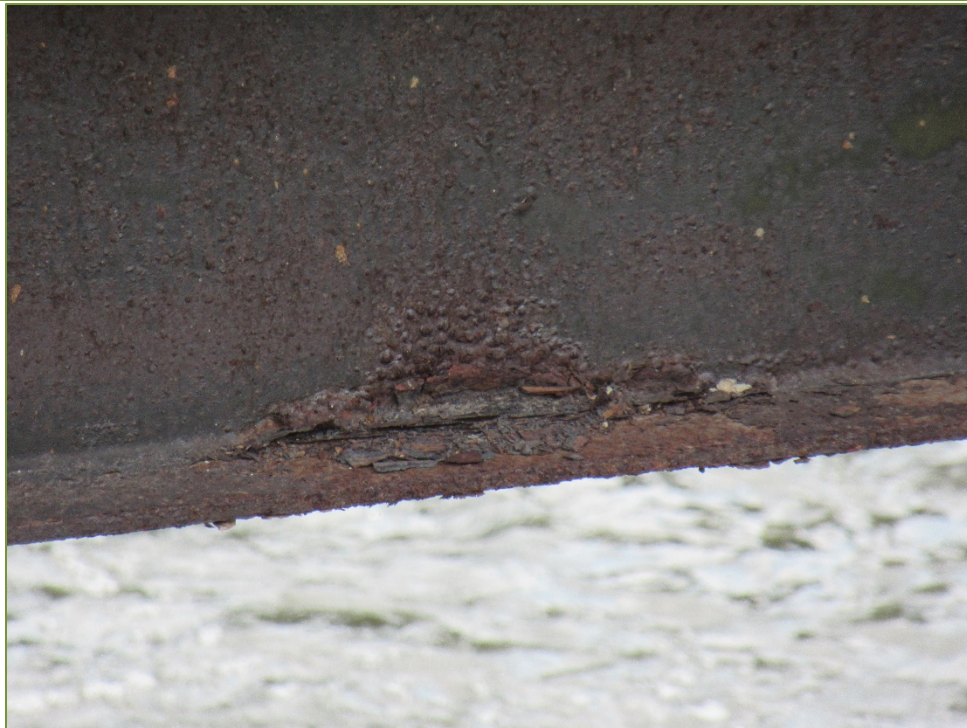
Photo P36 1 st Girder from North between Pier and East Abutment (severe corrosion on top flange)
