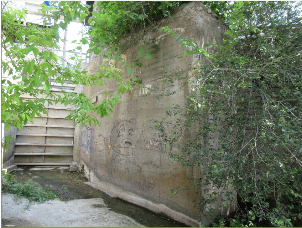
Photo P17 Outlet – South Wall (cracks, spall, delamination, light to medium scaling, and wet area)
