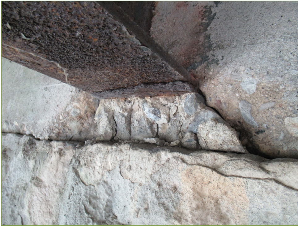
Photo P25 4 th Girder from North at West Abutment (severe corrosion)
