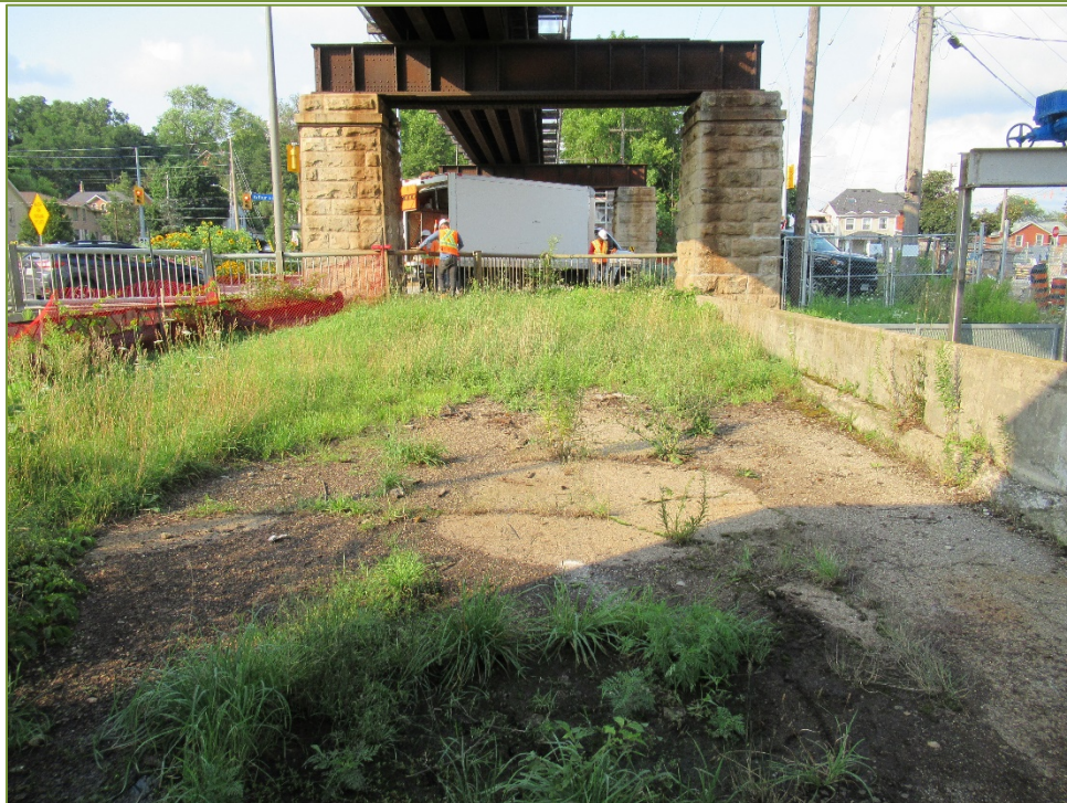
Photo P44 East Approach Wearing Surface (fair condition – unsealed cracks, and raveling) note, vegetation growth
