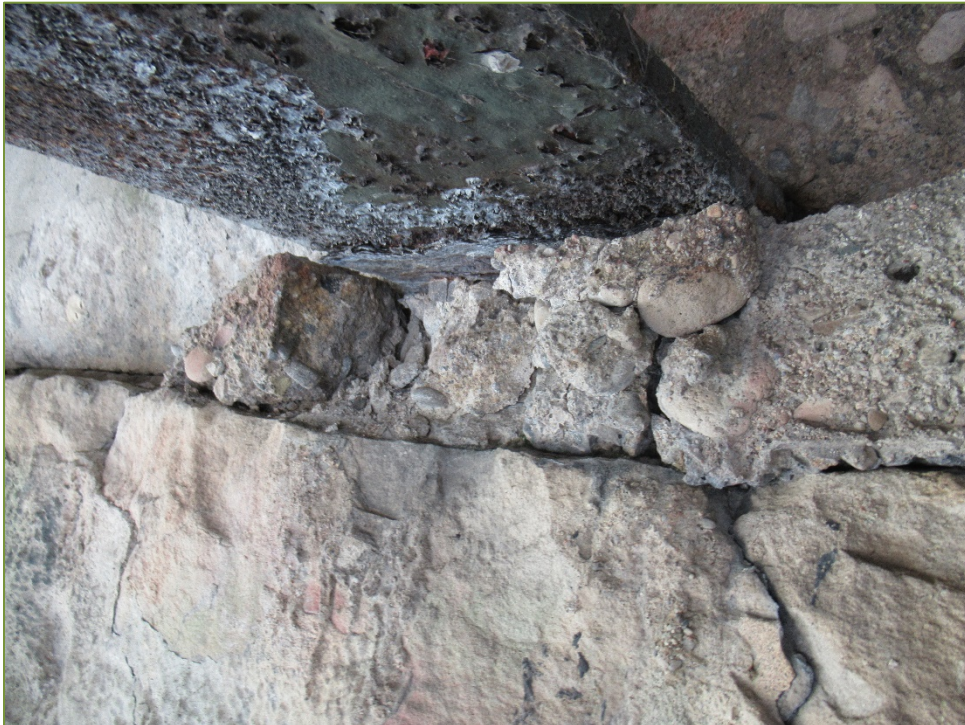
Photo P58 West Abutment – Masonry Wall (spall)
