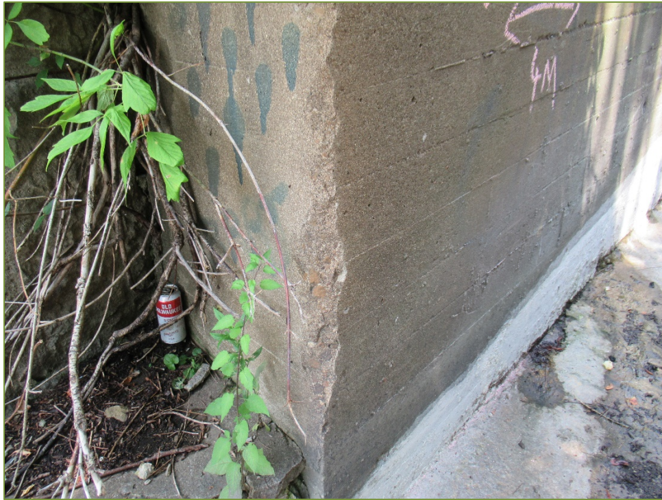
Photo P15 Outlet – North Wall, old structure (spall)
