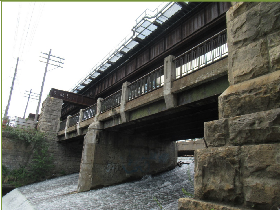
Photo P42 South Elevation – Fascia (cracks, spall, delamination, and light scaling)
