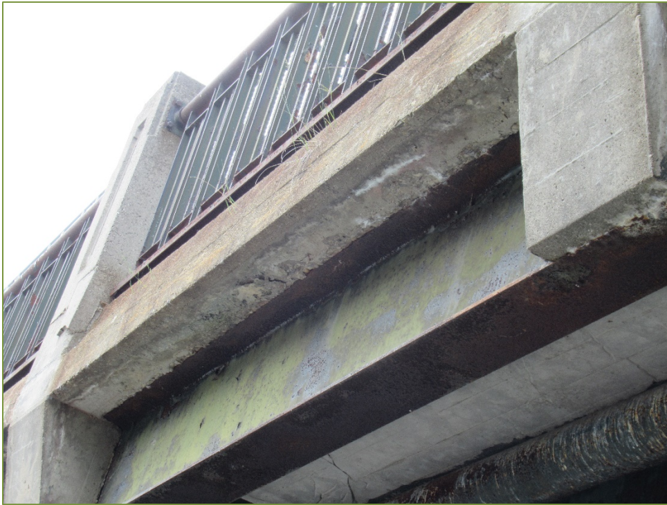
Photo P29 Soffit between Pier and East Abutment, south edge (crack, spall and delamination) and Girders (light corrosion)
