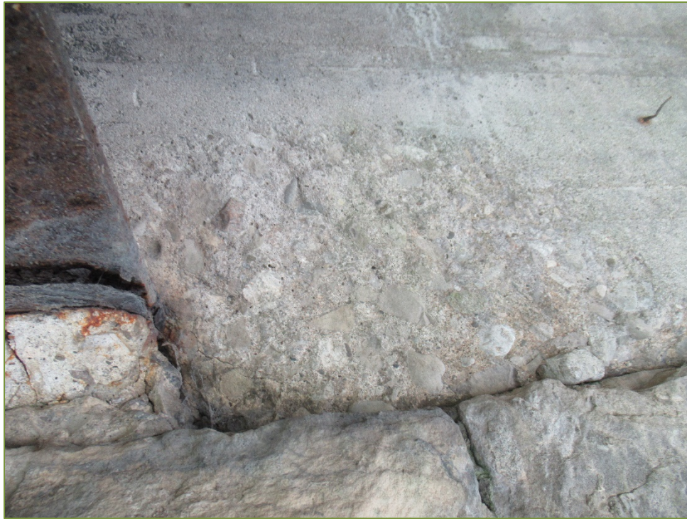
Photo P61 West Diaphragm (spall)
