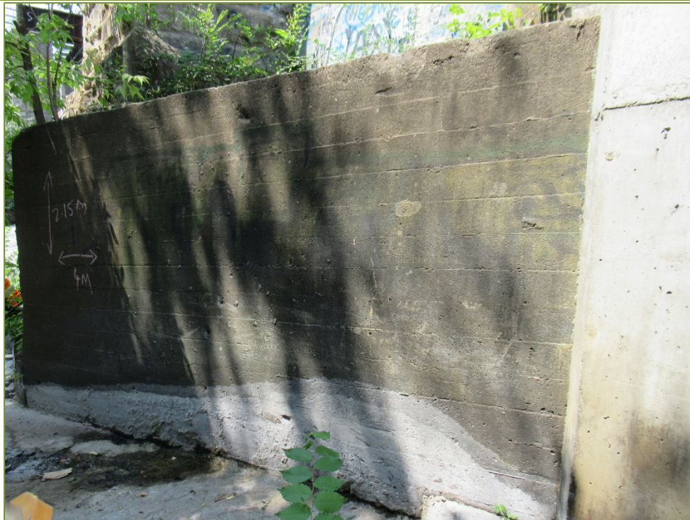
Photo P14 Outlet – North Wall, old structure (crack, spall, delamination, and light scaling)
