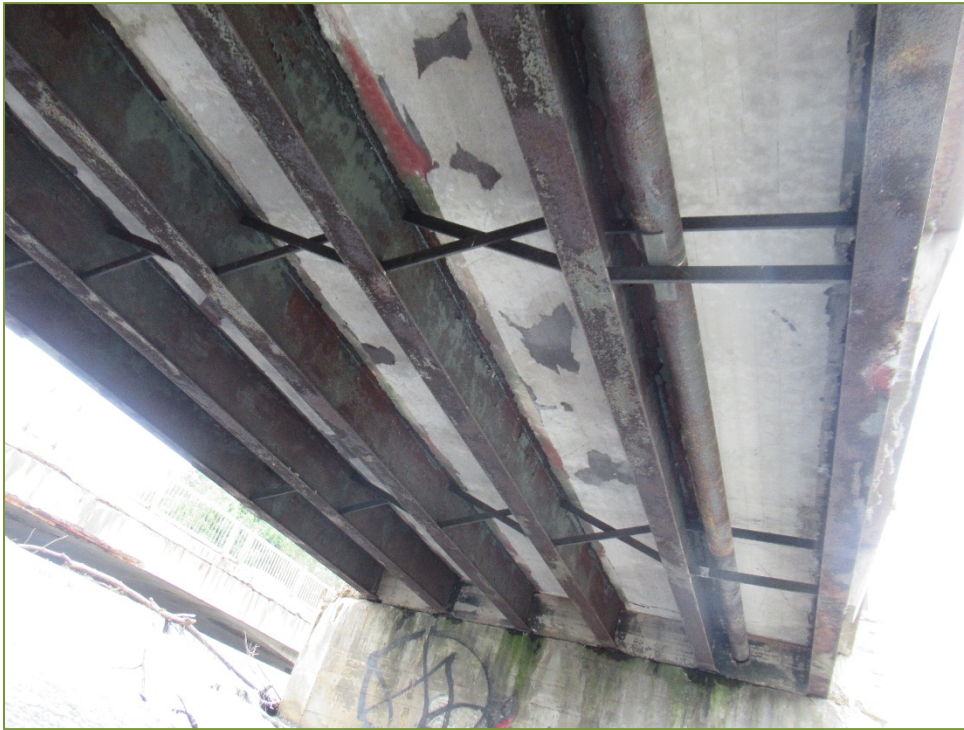
Photo P9 Soffit between West Abutment and Pier, looking east (fair condition – cracks, spall, delamination and light scaling) and Girders (fair condition – light to severe corrosion)
