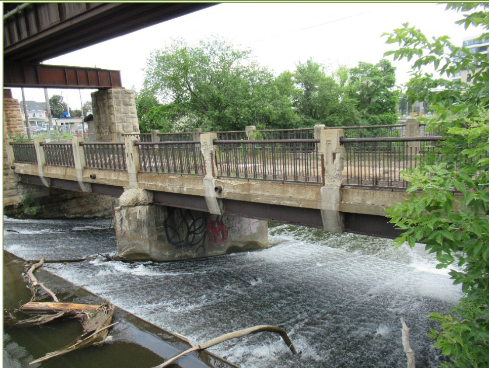
Photo P40 North Elevation – Fascia (cracks, spall, delamination, and light scaling)
