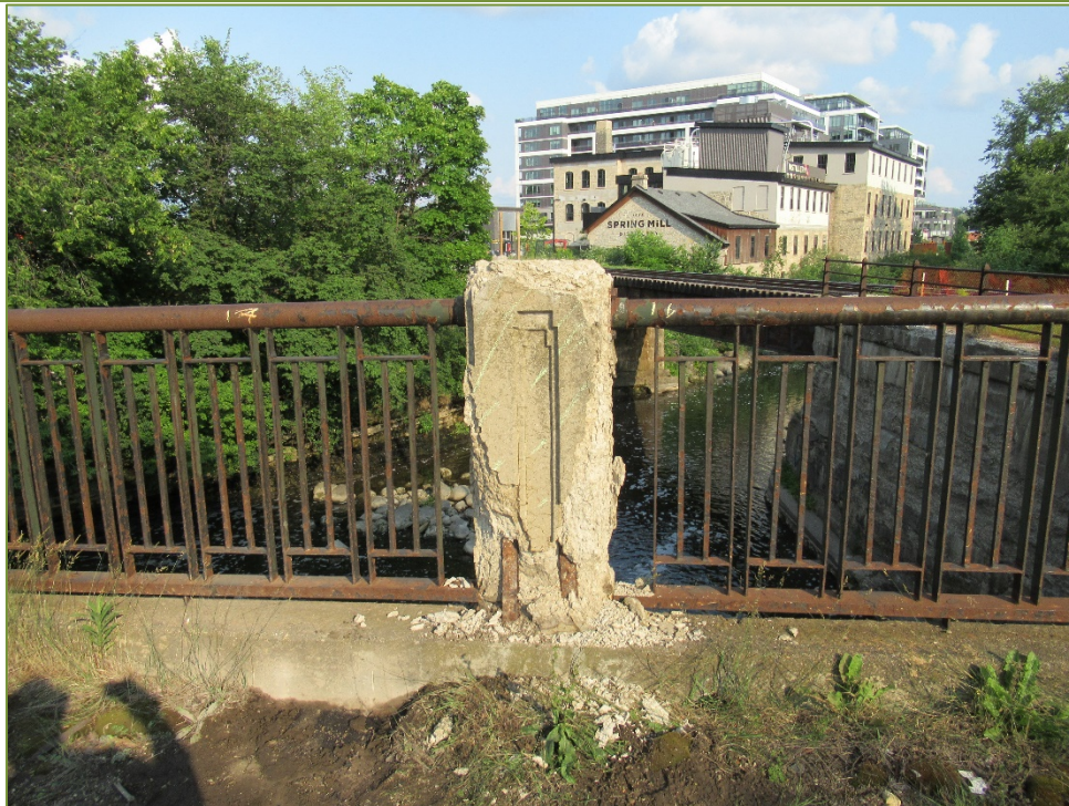
Photo P52 South Curb (medium scaling) Concrete Posts (cracks, spall, delamination, and light scaling) and Handrail (light corrosion)
