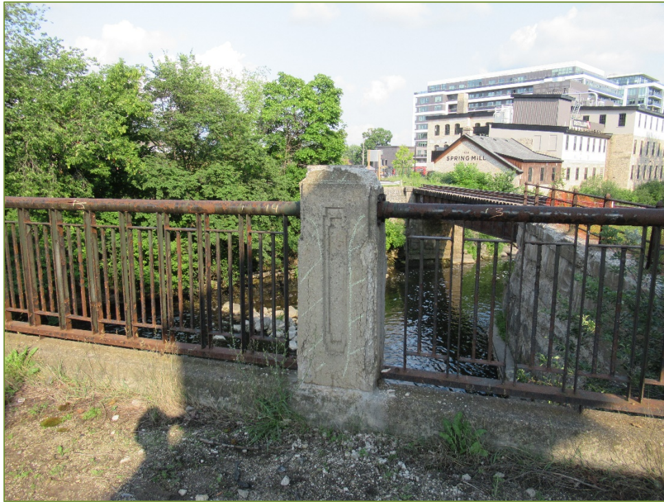
Photo P51 South Curb (medium scaling) Concrete Posts (cracks, spall, delamination, and light scaling) and Handrail (light corrosion)
