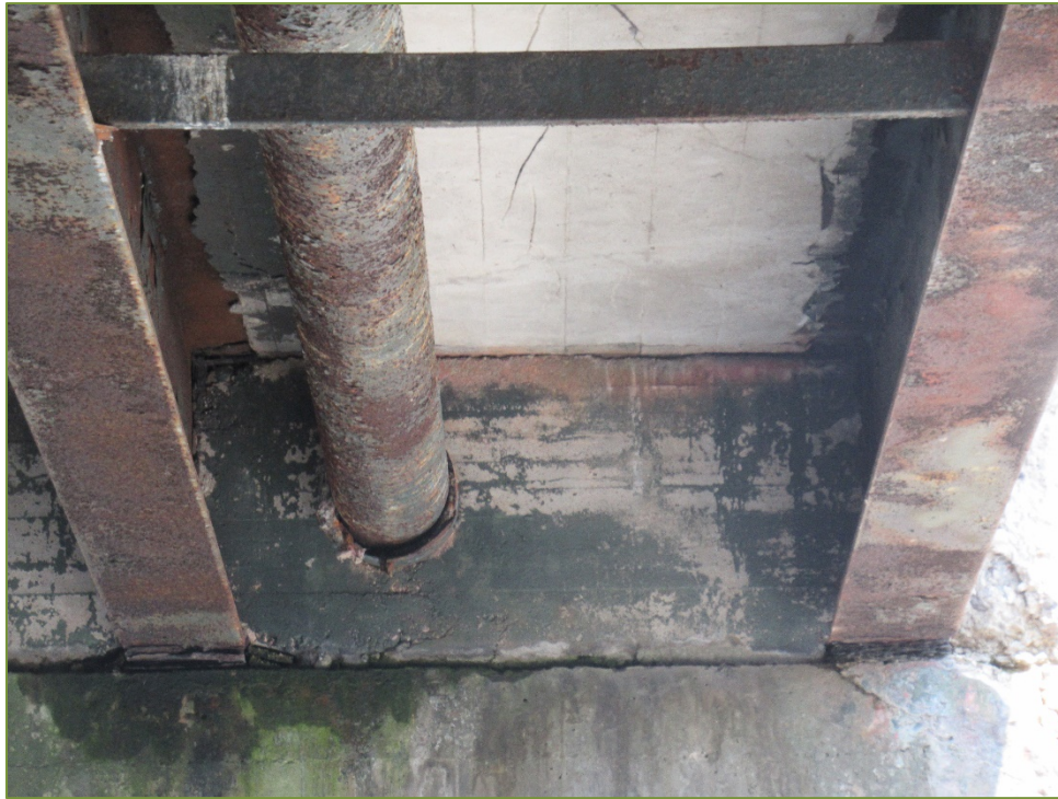
Photo P39 Typical Diaphragm at Pier – West Face (spall and honeycombing)
