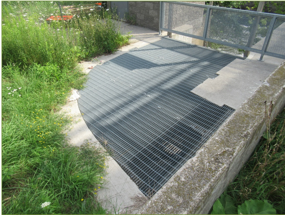
Photo P11 Outlet – Top Surface (cracks, spall, and medium scaling)
