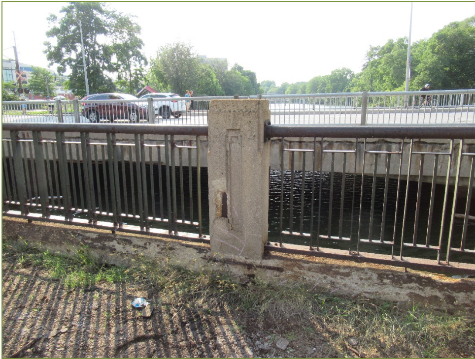
Photo P47 North Curb (cracks, spall, delamination, and medium to severe scaling) Concrete Posts (cracks, spall, delamination, and light scaling) and Handrail (light corrosion)
