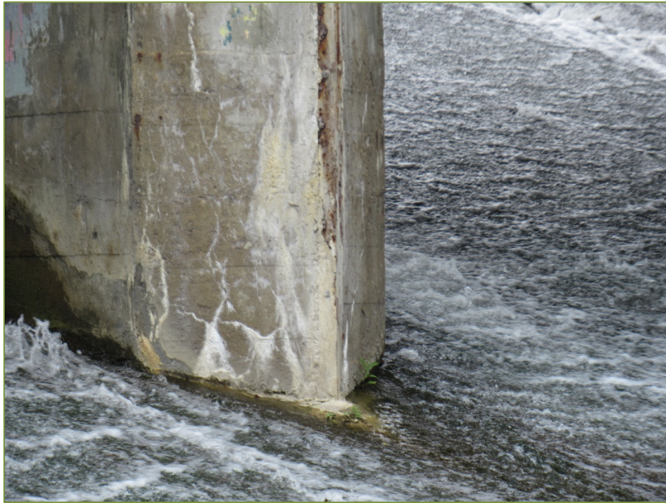
Photo P75 Pier - West Face, south side (cracks)
