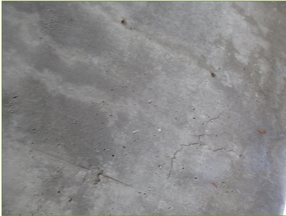
Photo P13 Soffit between East Abutment and Pier (cracks, delamination, and wet area)
