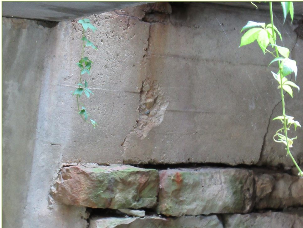
Photo P6 Inlet- East Wall, North side (wide crack, spall, delamination, and light to medium scaling)
