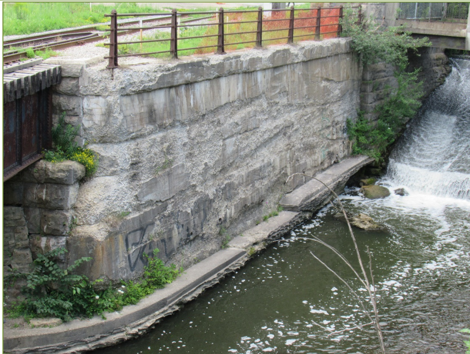
Photo P68 Southwest Retaining Wall (spall and severe scaling)
