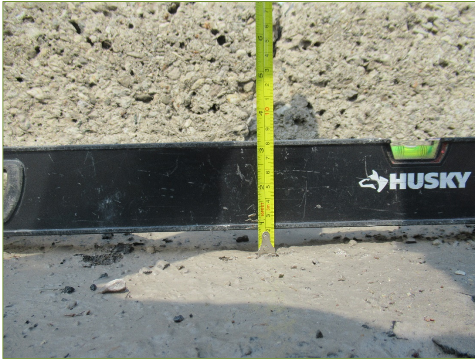
Photo P35 West Joint (settlement)
