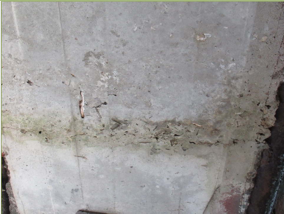
Photo P14 Soffit at West Abutment between 2 nd and 3 rd Girder from North (cracks, honeycombing, and wet area)
