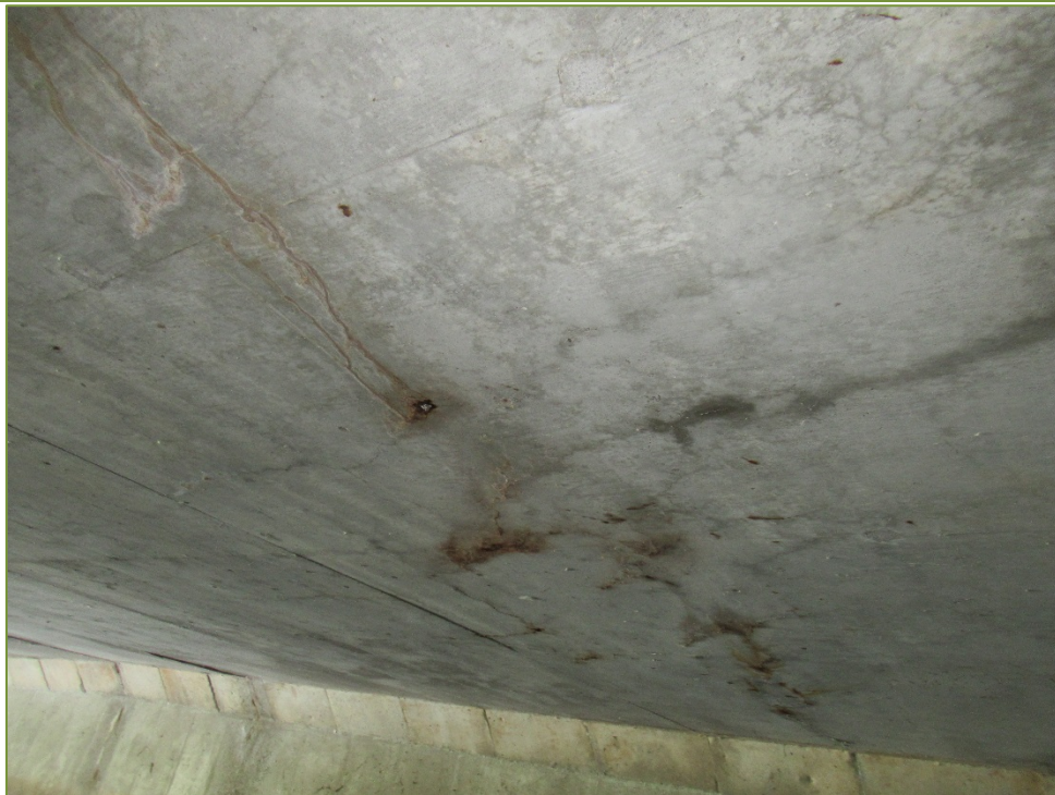
Photo P18 Soffit between East Abutment and Pier (cracks and wet area)
