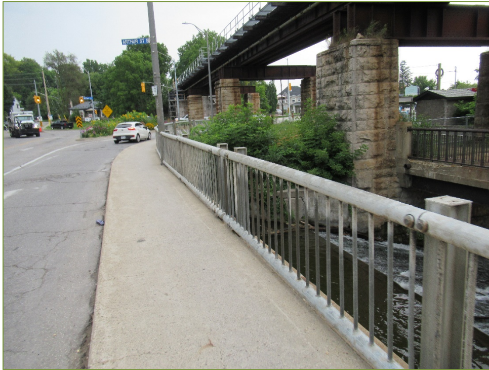
Photo P45 South Sidewalk (cracks and light to medium scaling) and Handrail (light corrosion)
