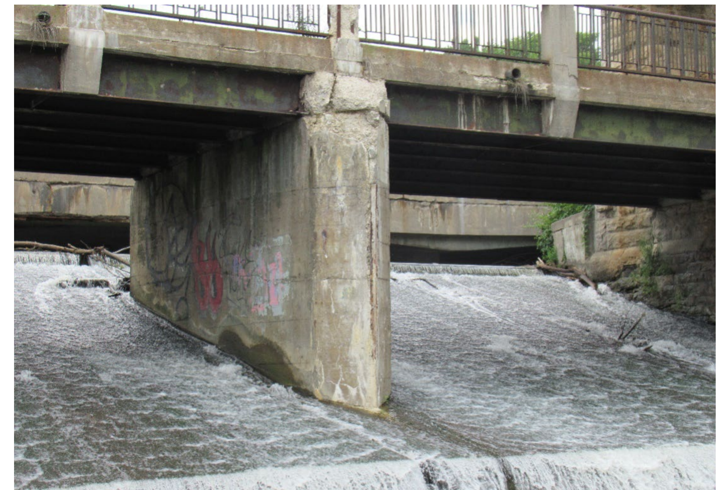
The spillway forms a weir to control the Speed River elevation, previously used for the now-removed Allan's Mill.
