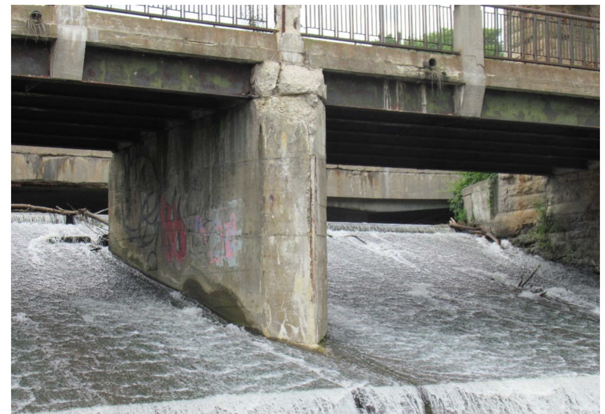
23b) The spillway forms a weir to control the Speed River elevation, previously used for the now-removed Allan's Mill.
