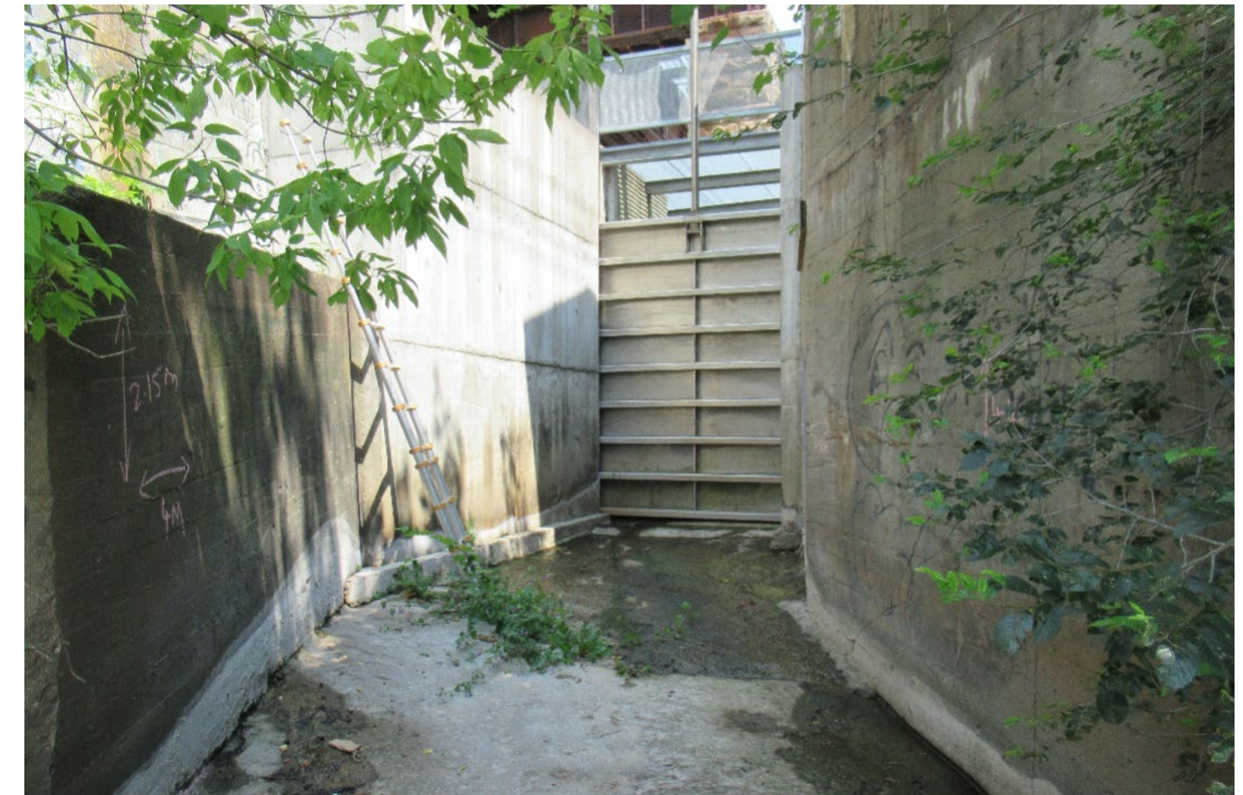
The sluiceway is a concrete channel with a metal gate to carry excess water.
