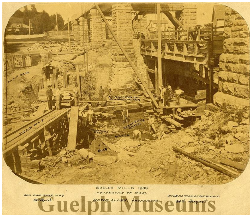
Figure 14: Foundation of dam/spillway and new Allan's Bridge in 1869 (Guelph Museums, n.d.)
