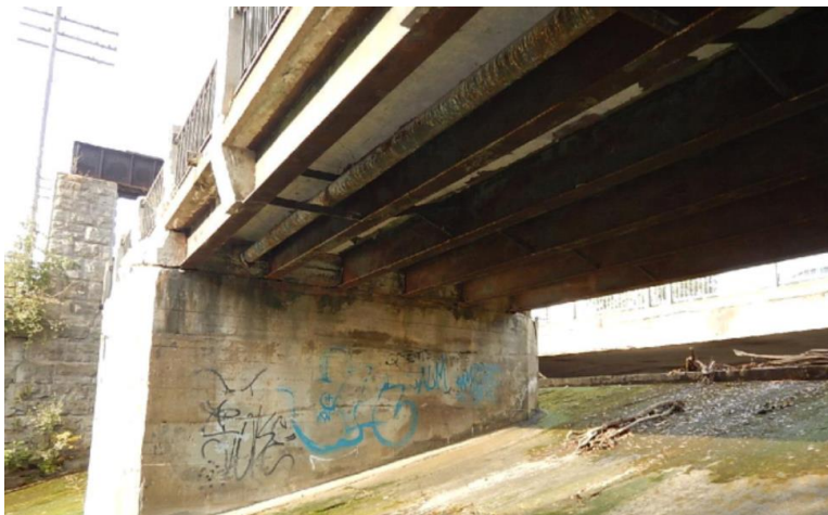
Figure 37: Soffit and girders on underside of Allan's Bridge (OSIM, 2018a)
