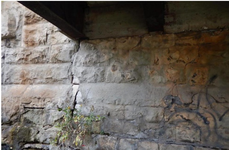
Figure 35: Limestone pier walls supporting the Allan's Bridge superstructure (OSIM, 2018a)
