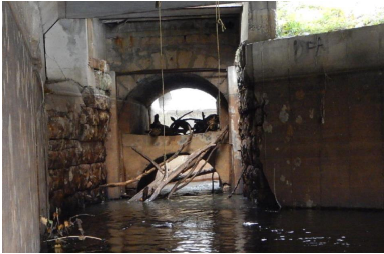
Figure 44: Sluiceway inlet, featuring large and small arches (OSIM, 2018b)
