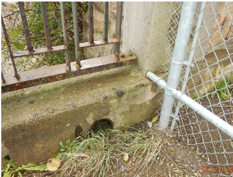
Figure 39: Southwest drain on Allan's Bridge (OSIM, 2018a)
