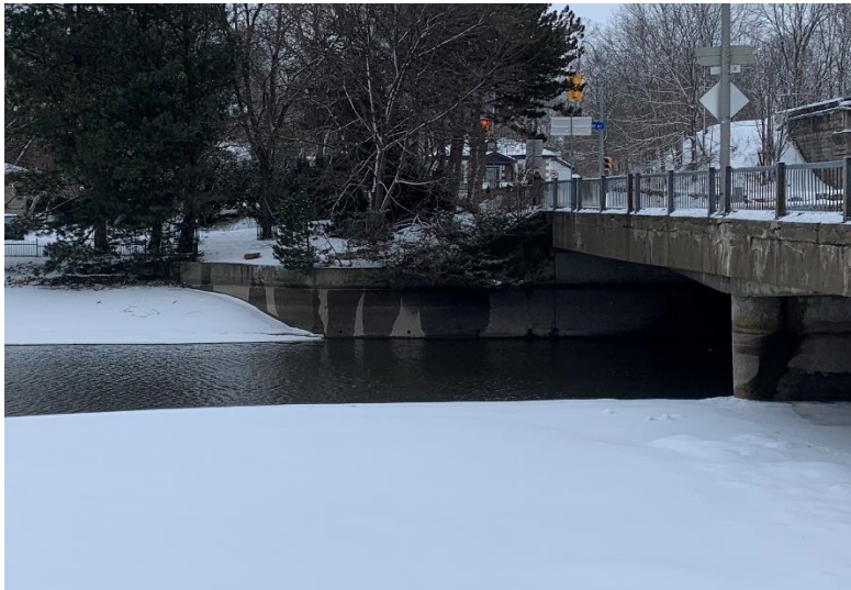
Figure 30: Macdonell Street Bridge northwest abutment wall, wingwall, and embankment, looking northeast (ASI 2022)
