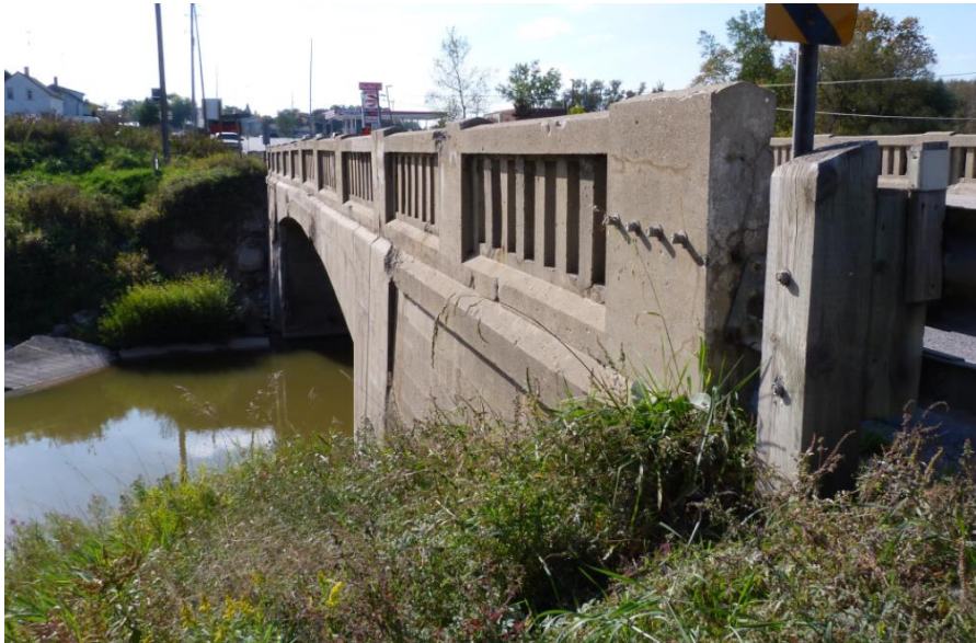
Figure 67: CR-109 West Bridge over Conestogo River in Wellington County, built in 1931 and featuring original concrete balustrade railing (Holth, 2021)
