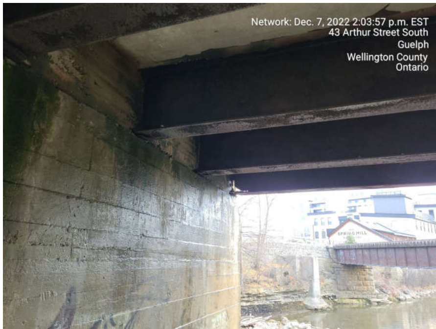
Southwest girder ends shoing section loss at the flange
