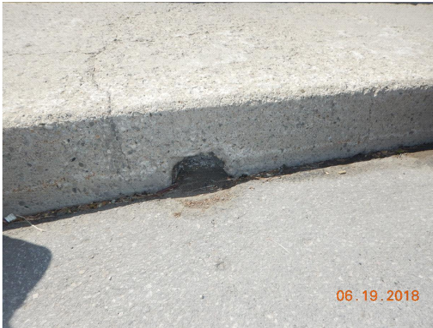
Plugged curb drains
