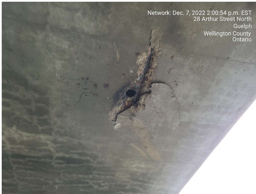
Drainage system outlet showing spalls
