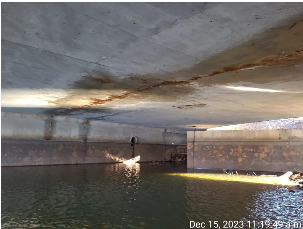
Photograph: 14 East span soffit showing wide crack w/ efflorescence, rust and moisture staining along centerline
