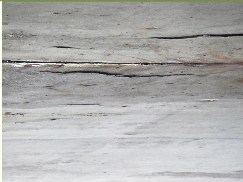
Photo P16 Soffit between East Abutment and Pier (cracks, spall, delamination, and wet area)
