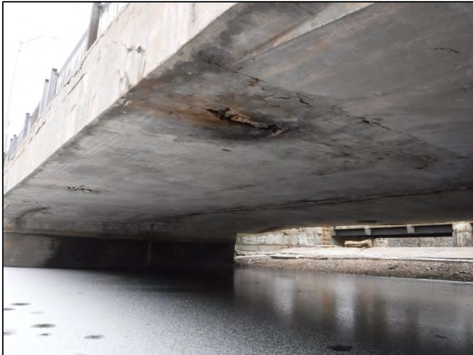
Photo 14: Spall with Exposed Corroded Reinforcing Steel and Delaminated Concrete on Soffit, West End of West Span
