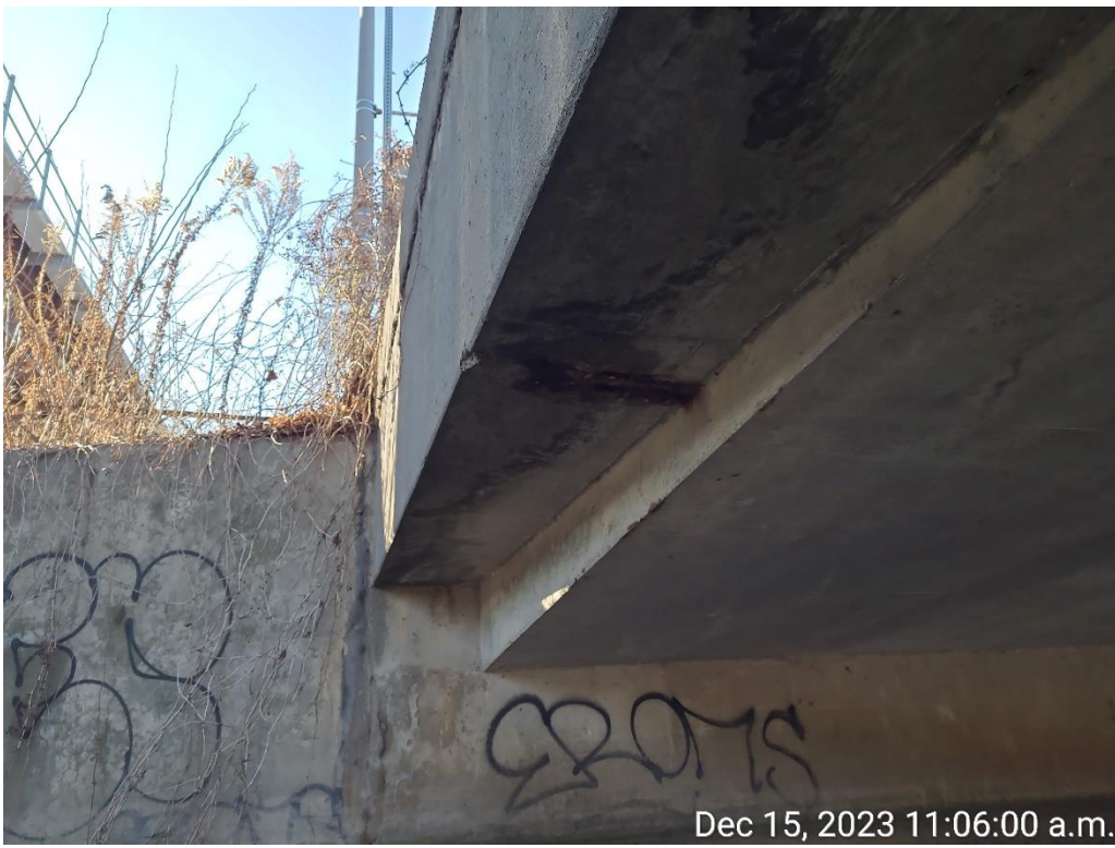
Photograph 6: Underside of southwest fascia showing delamination, spalls and exposed corroded rebar
