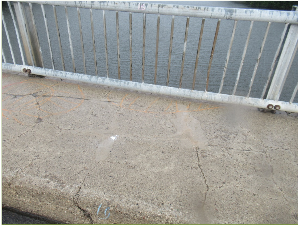
Photo P41 North Sidewalk (cracks, spall, delamination, and severe scaling) and Handrail (light corrosion)
