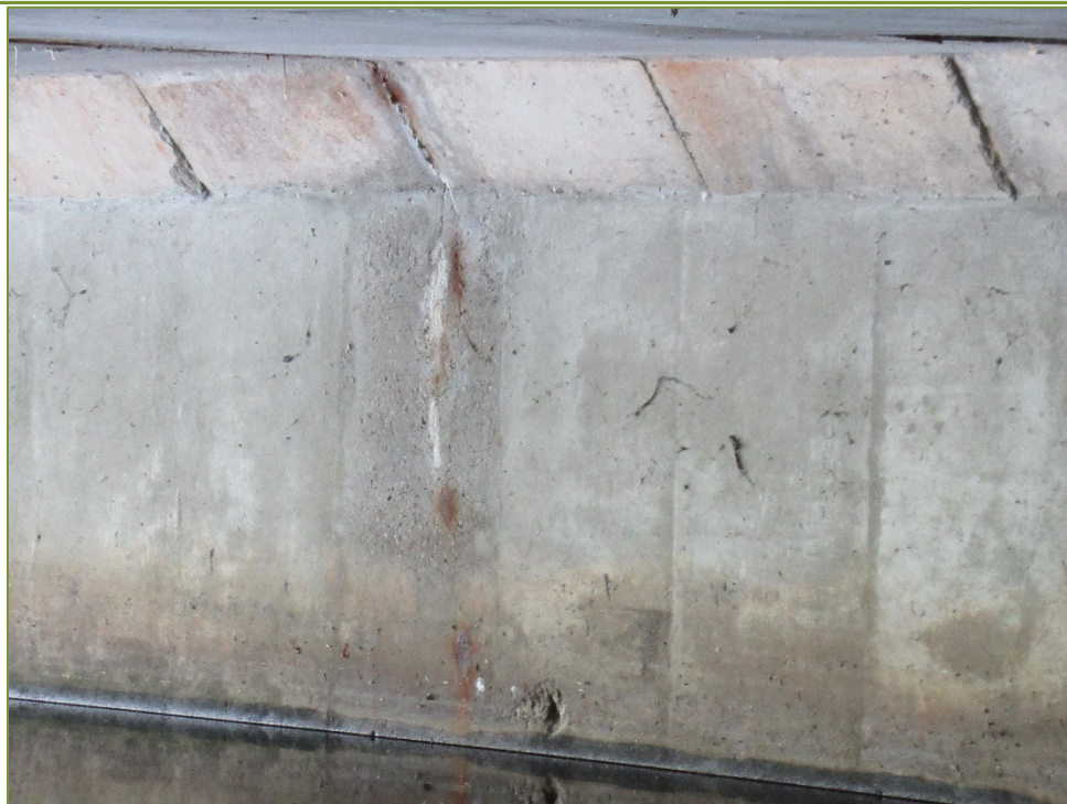
Photo P48 East Abutment (cracks, spall, light to medium scaling, and wet area)
