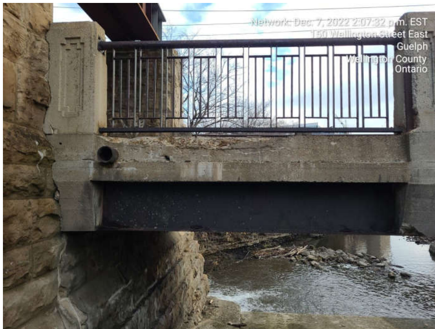
Deck drain and spalls on soffit exterior
