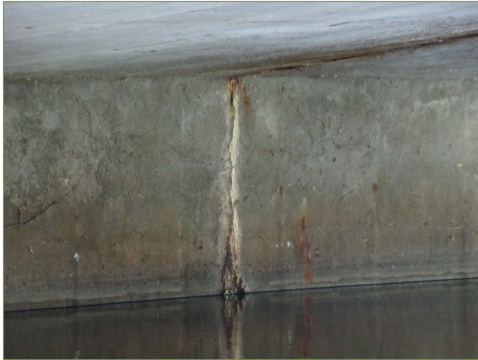
Photo P59 Pier - East Face (cracks, spall, and wet area)
