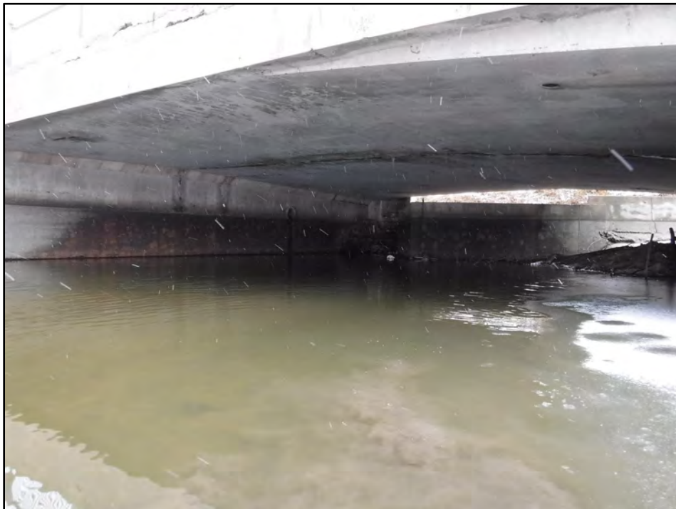
Photo 16: Wide Longitudinal Crack with Damp Staining, Full Length of East Span Soffit
