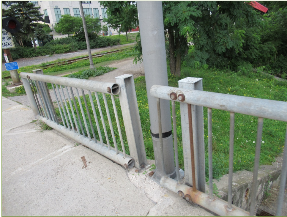
Photo P39 North Handrail (light corrosion)
