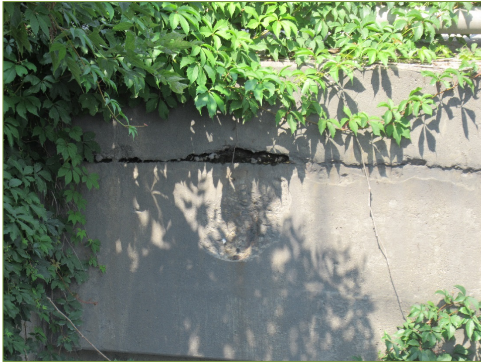
Photo P25 South Elevation – Fascia (wide cracks and spall)
