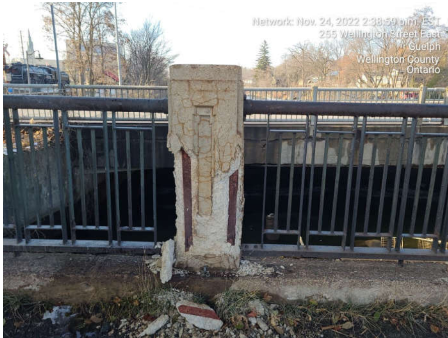
Severe spalls and exposed corroded steel on barrier posts
