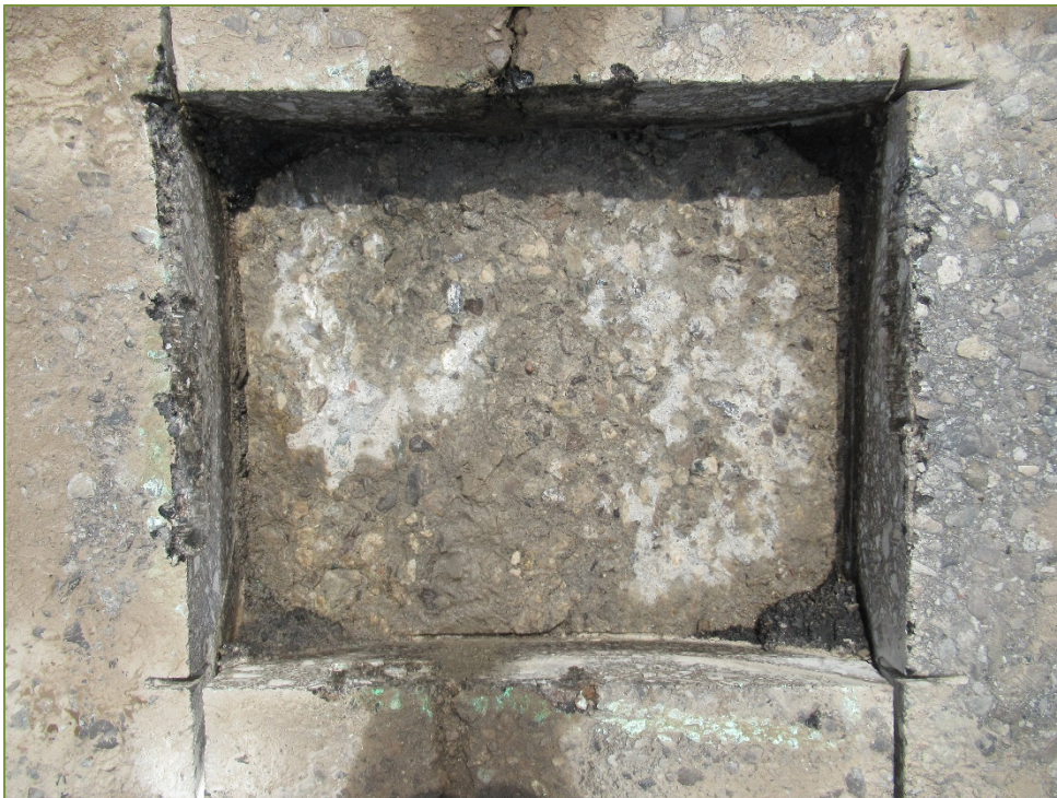
Photo S8 – Sawn Sample SS8 (medium scaling)
