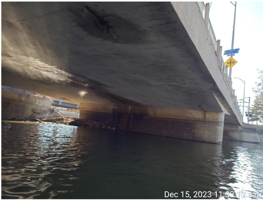
Photograph 20: East span deck soffit showing wide longitudinal crack along centerline
