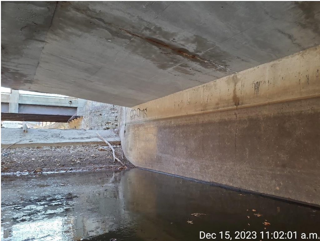
Photograph 5: Wide crack with rust staining and efflorescence continuing into north abutment
