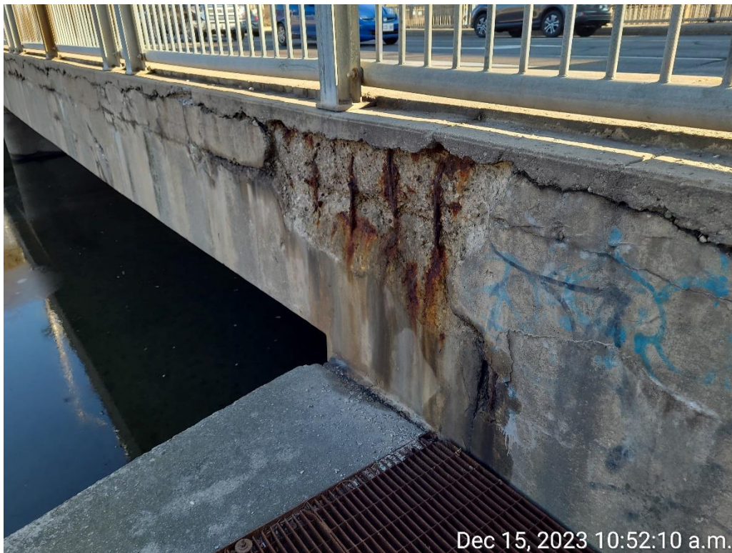
Photograph 2: North soffit exterior showing severe delamination and exposed corroded rebar
