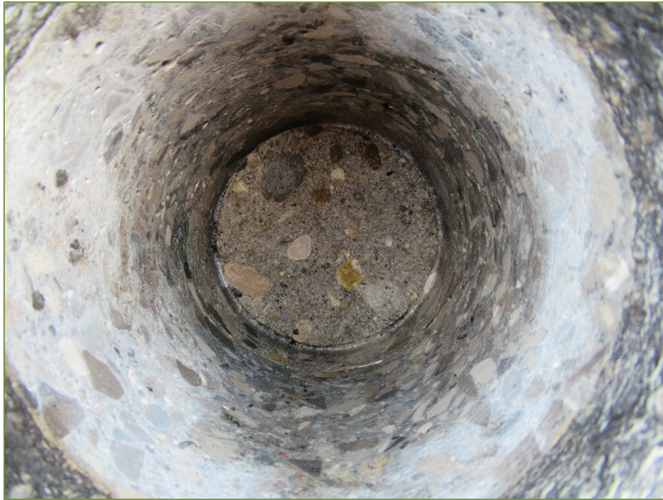
Photo P69 Typical Condition of Inside Core – C10
