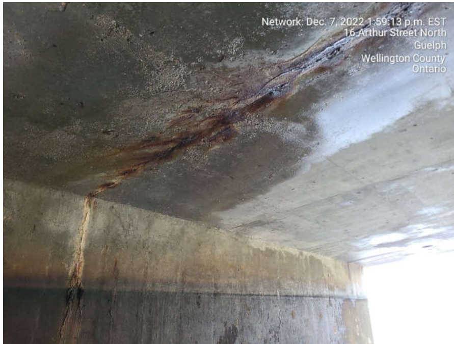
Medium full length crack with rust stains showing on east abutment wall and soffit
