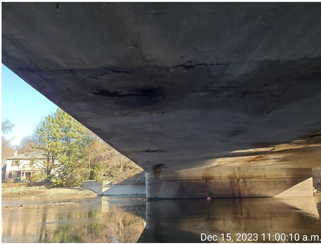
Photograph 4: Northwest deck drain hole showing delamination and spalls
