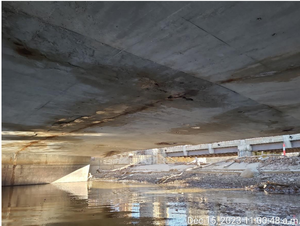
Photograph 3: West span soffit interior showing longitudinal wide crack along centerline
