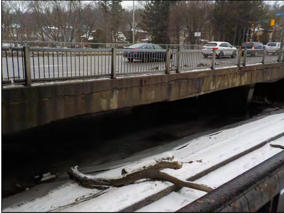
Photo 13: Wide Cracks and Delaminated Concrete on South Soffit Fascia
