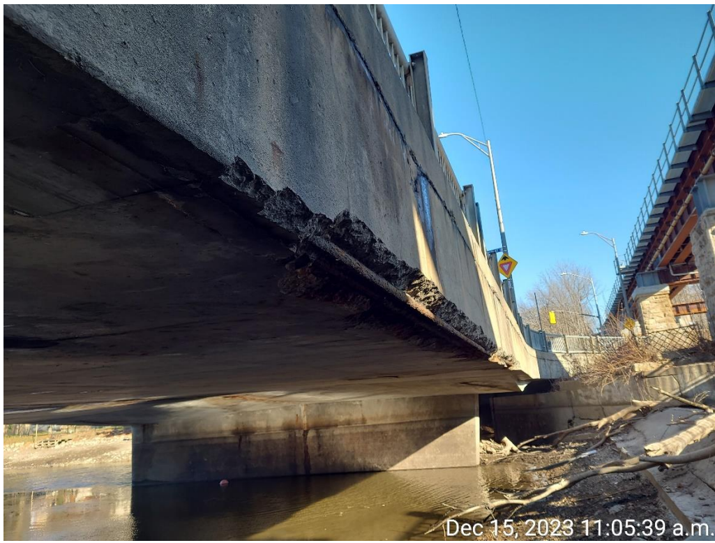
Photograph 8: South fascia showing severe spalls and exposed corroded rebar
