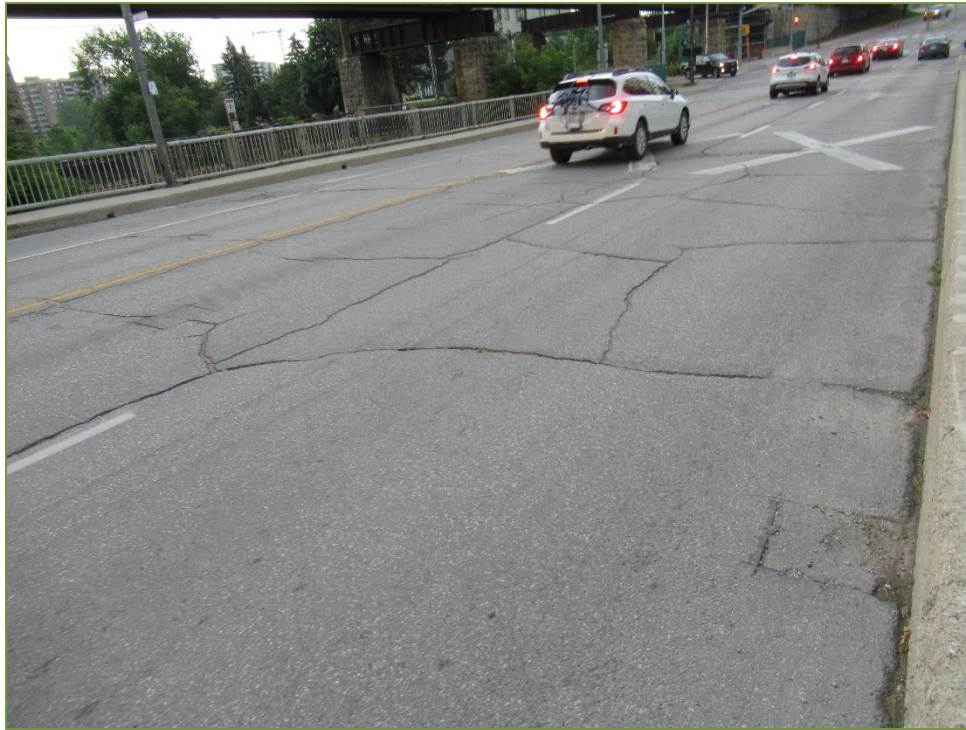
Photo P5 Deck Wearing Surface (fair to poor condition – unsealed cracks, alligator cracks, pot holes, ravelling and rutting)
