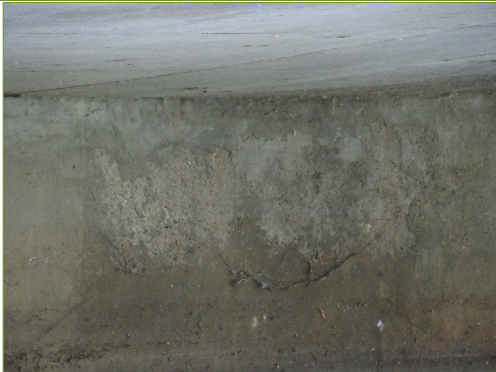
Photo P58 Pier - East Face (light scaling)
