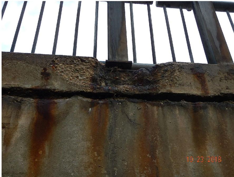
Southeast exterior soffit, spall at post base
