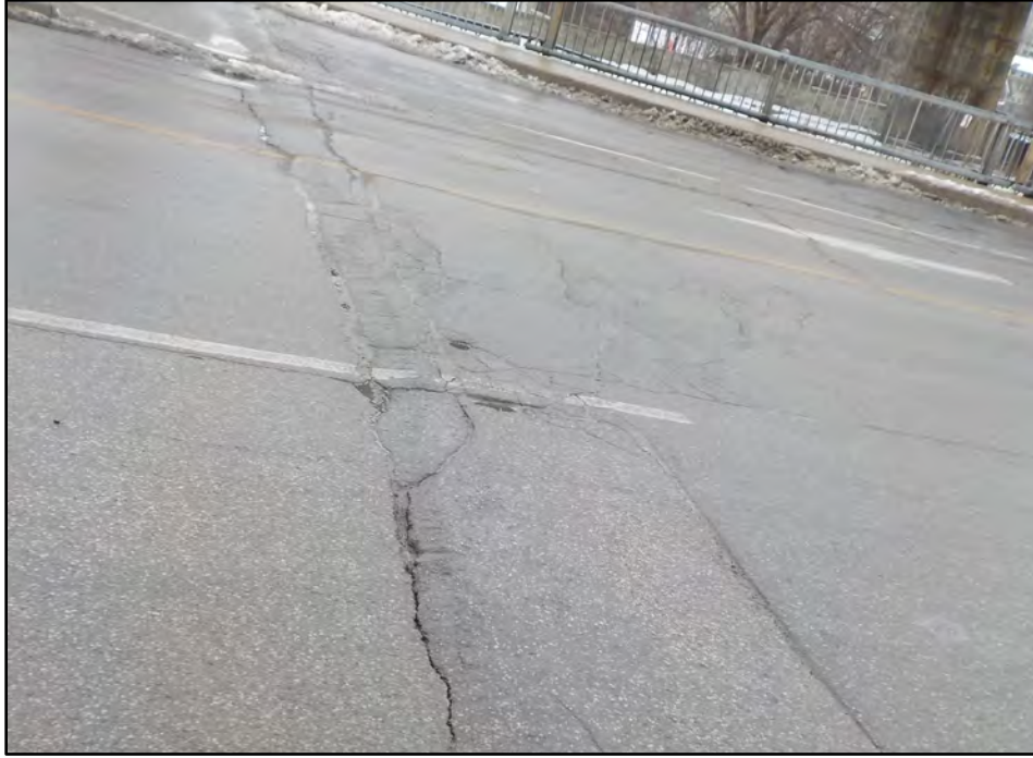
Photo 7: Wide Transverse Cracks and Bump Transition at East End of Deck
