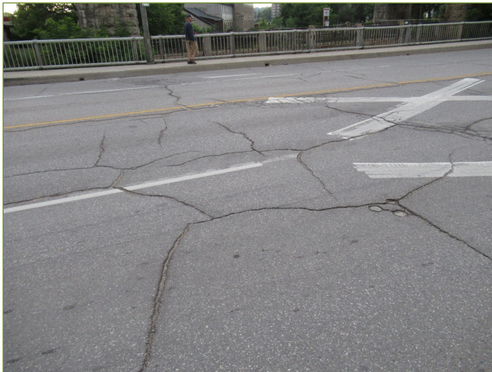
Photo P6 Deck Wearing Surface (unsealed cracks)
