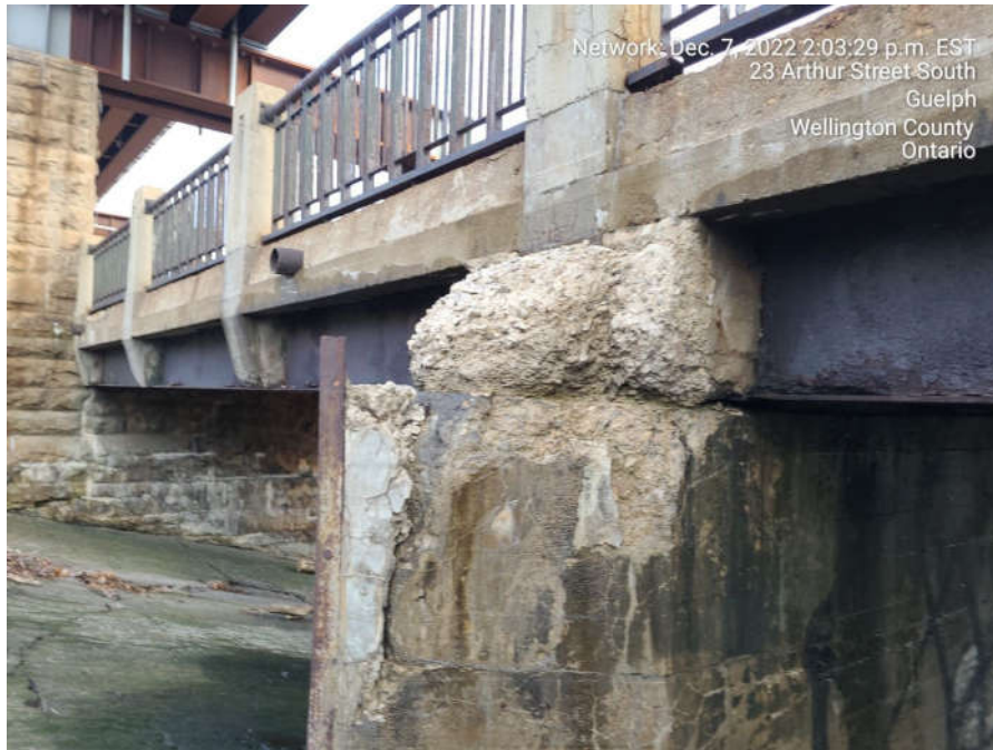
Very severe deterioration of concrete on top of pier cap, north side of structure
