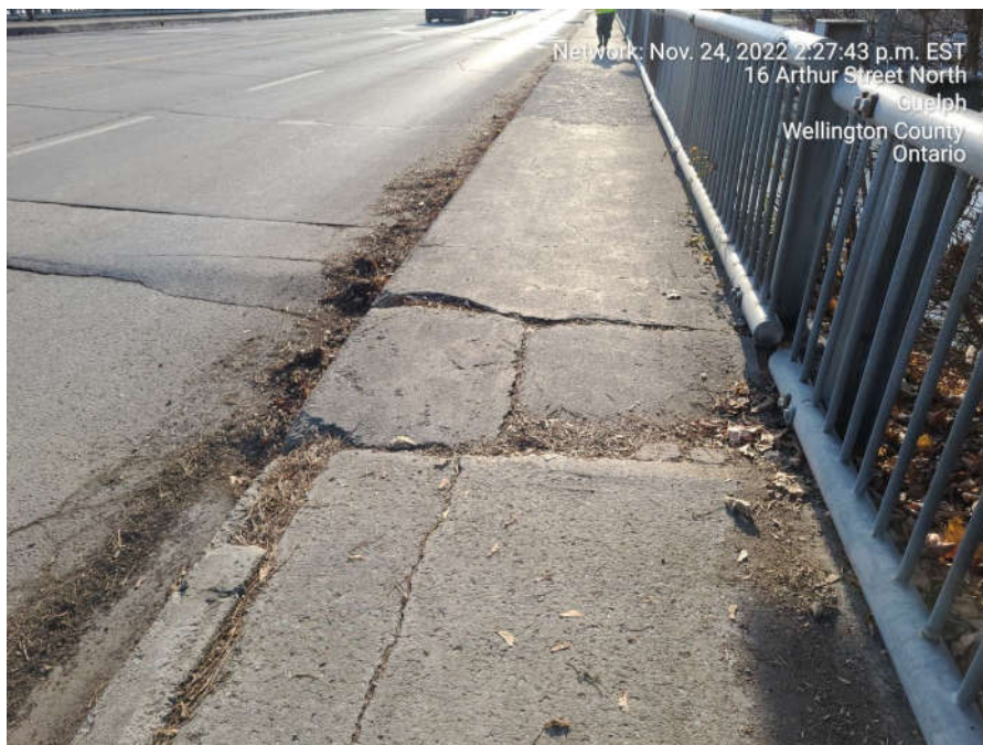
North sidewalk show wide cracks and settlement
