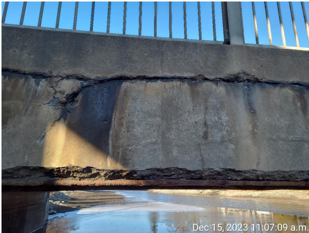
Photograph 7: South fascia showing severe spalls and exposed corroded rebar
