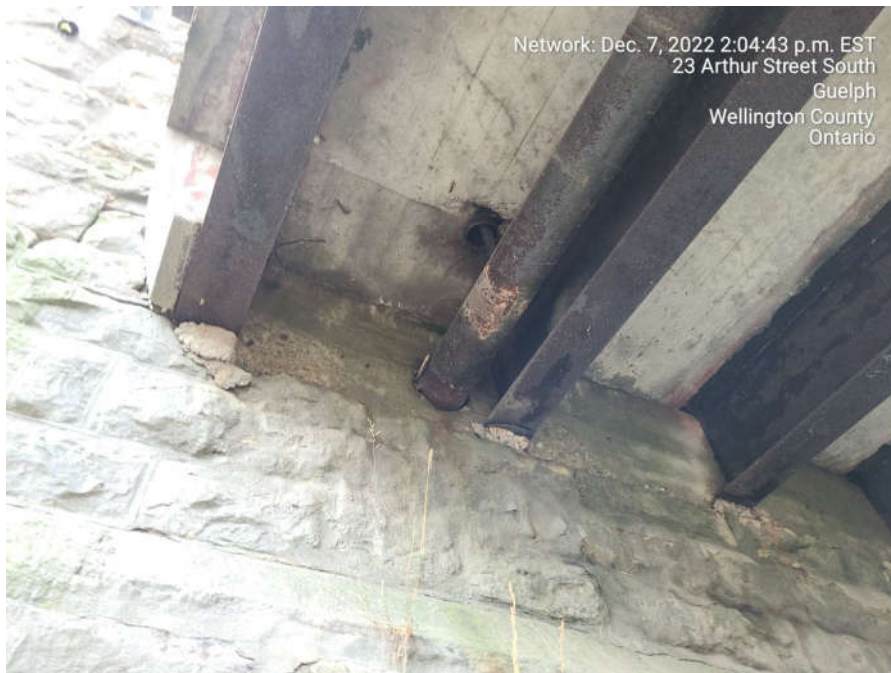
Medium to severe corrosion on deck drains
