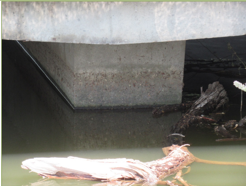
Photo P62 Pier - South Face (medium scaling)
