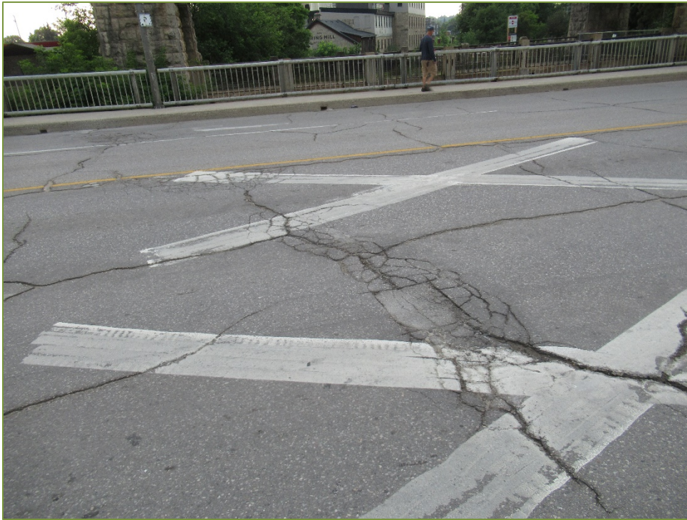
Photo P7 Deck Wearing Surface (unsealed cracks, alligator cracks)
