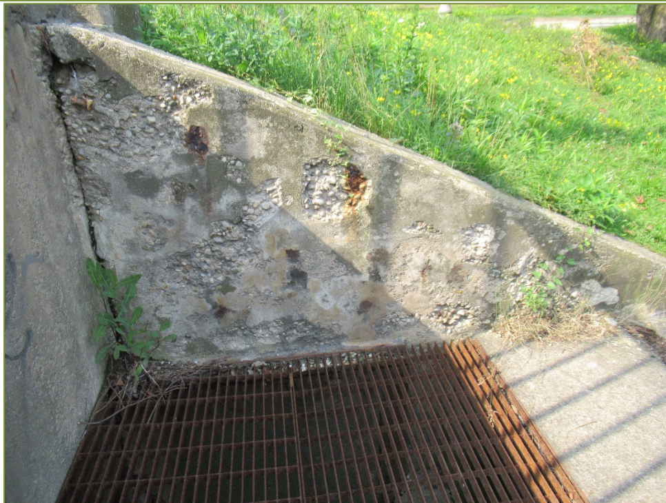
Photo P54 Northwest Retaining Wall (severe scaling)
