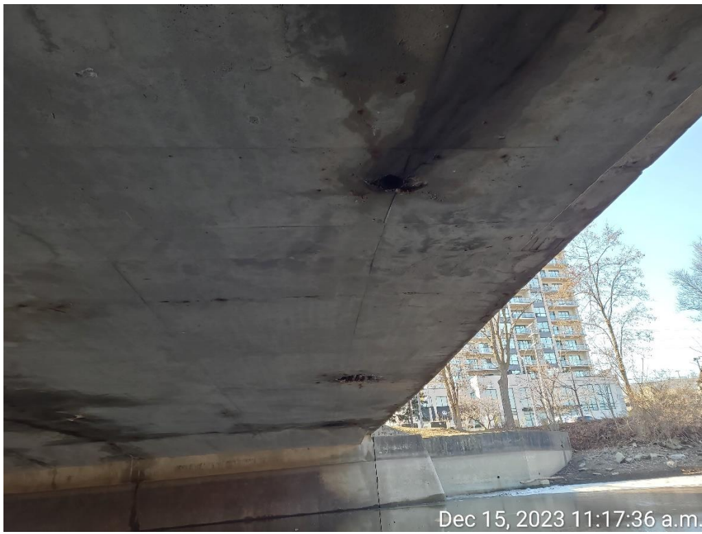
Photograph 12: Northeast drain on west span showing delamination and moisture staining around opening
