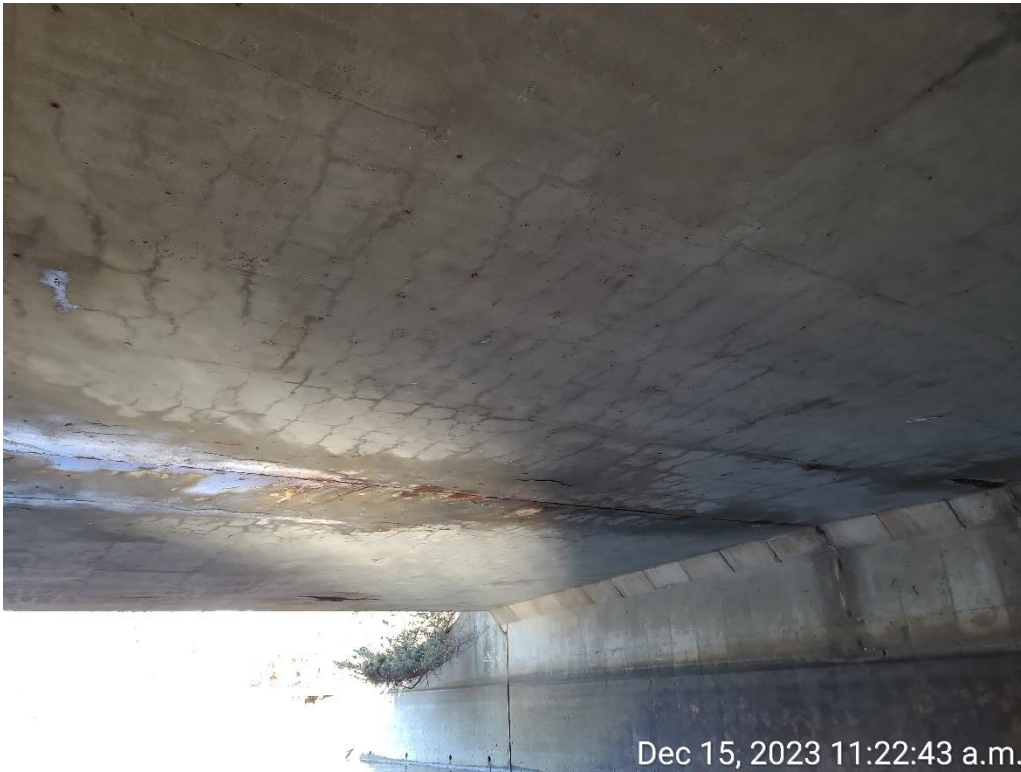
Photograph 17: East span soffit showing pattern cracking near midspan
