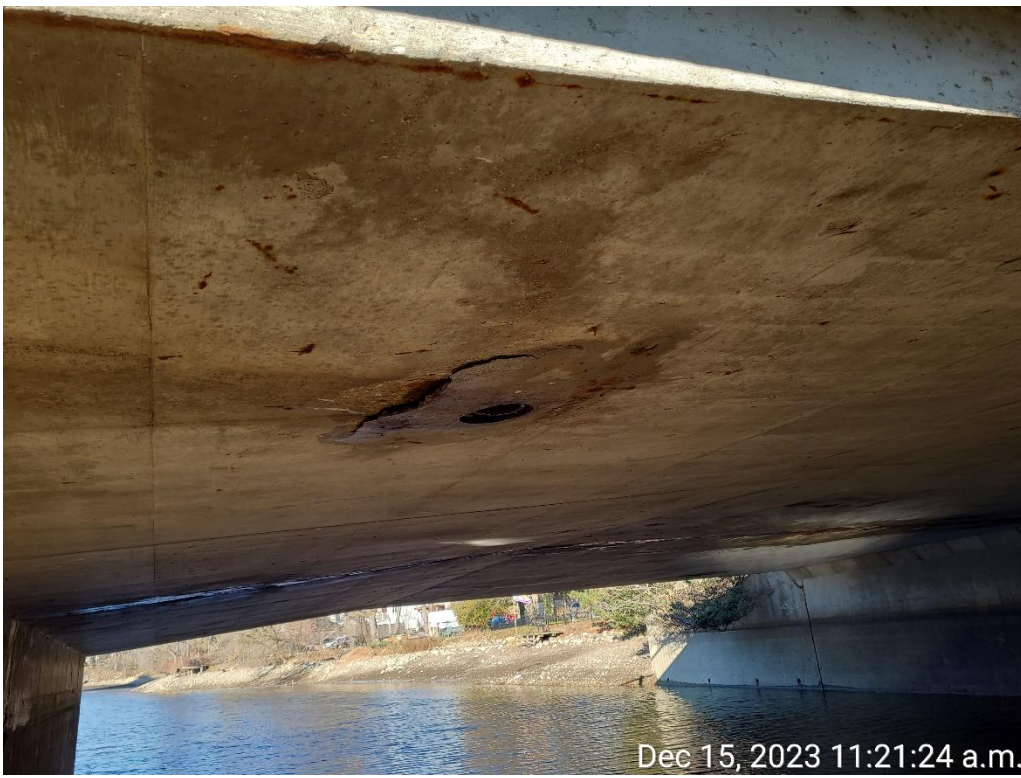
Photograph 18: Southwest deck drain on east span showing delamination around opening
