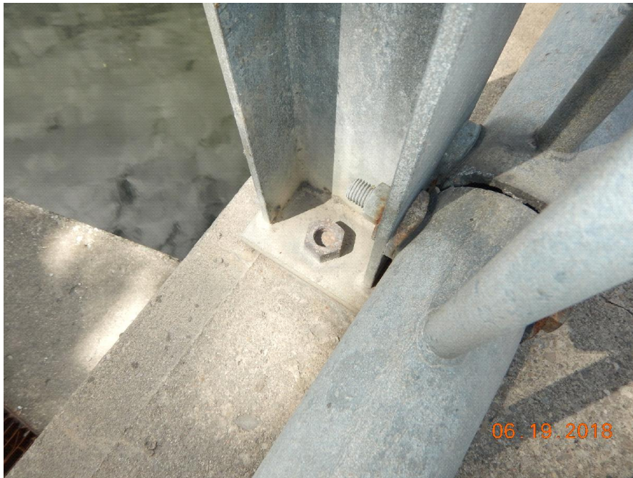
Insufficient bolt length on northwest railing
