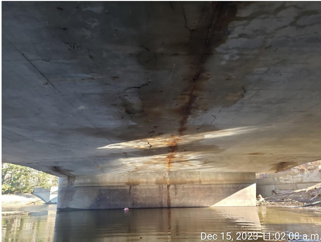
Photograph 11: Centerline wide cracking w/ efflorescence and rut staining along western span deck soffit
