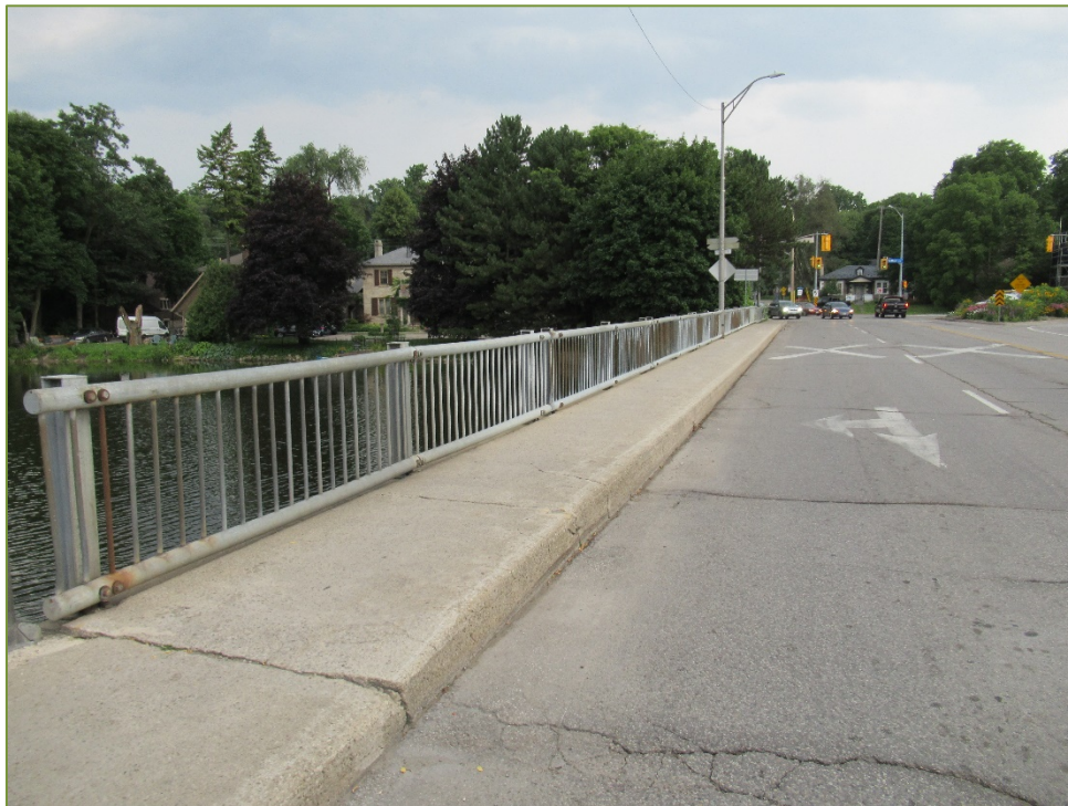
Photo P36 North Sidewalk (fair to poor condition - cracks, spall, delamination, and light to severe scaling) and Handrail (fair condition - light corrosion)
