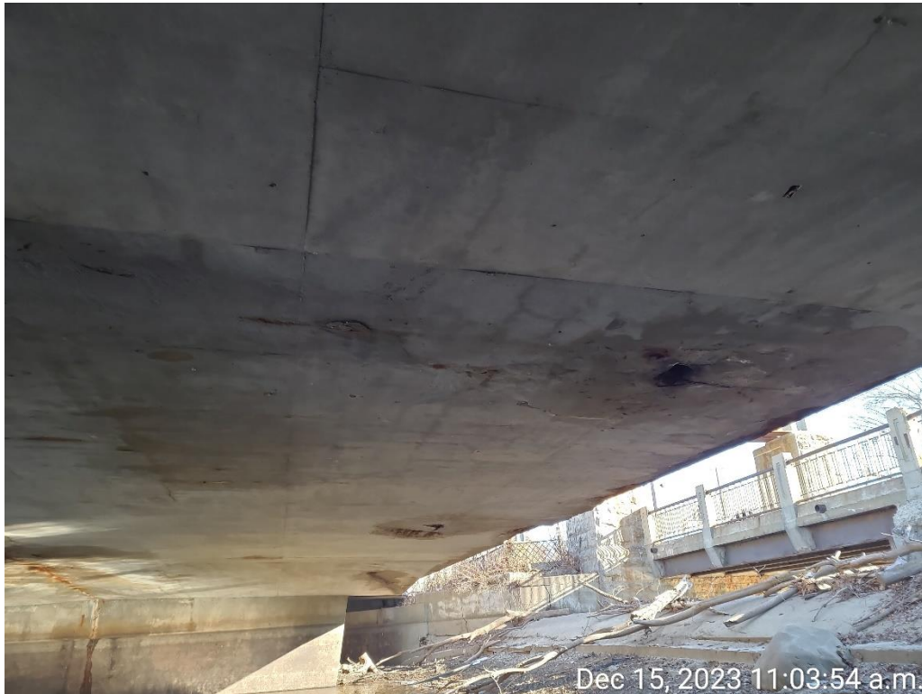
Photograph 13: Southwest drain hole showing spalls around opening
