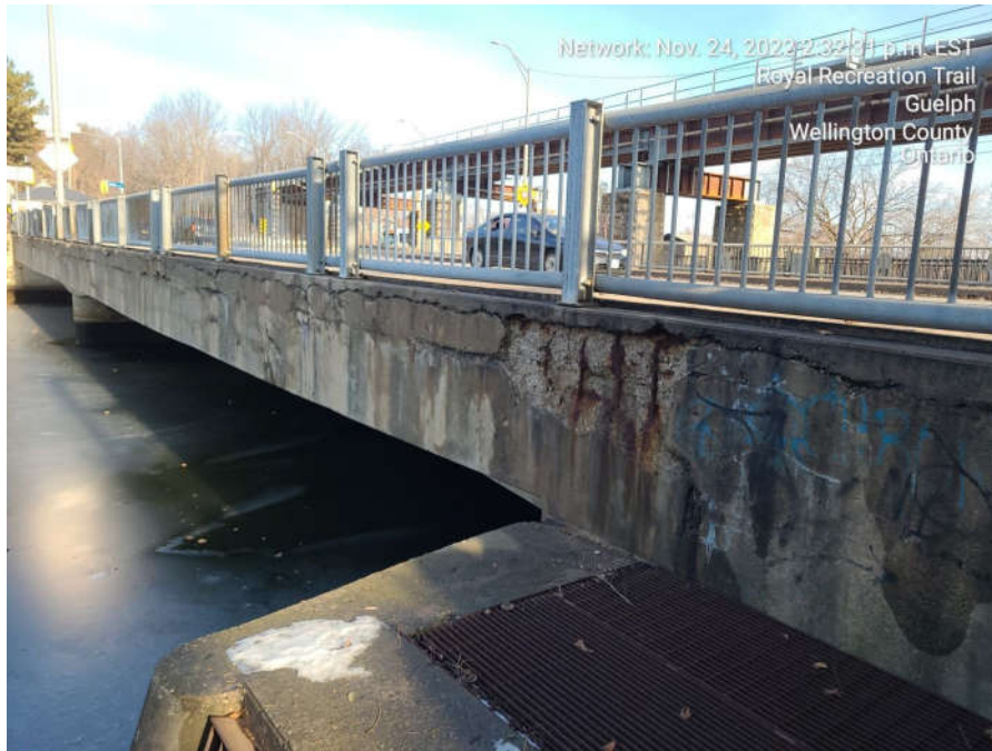
North soffit exterior shows severe delamination and exposed corroded rebar throughout
