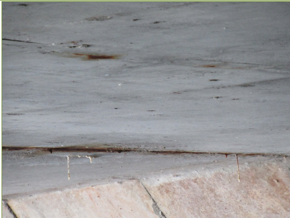
Photo P20 Soffit at East Abutment (cracks, and spall)
