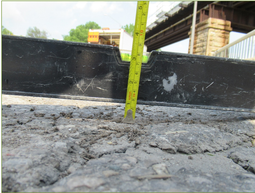
Photo P9 Deck Wearing Surface at East Abutment, south side (rutting)
