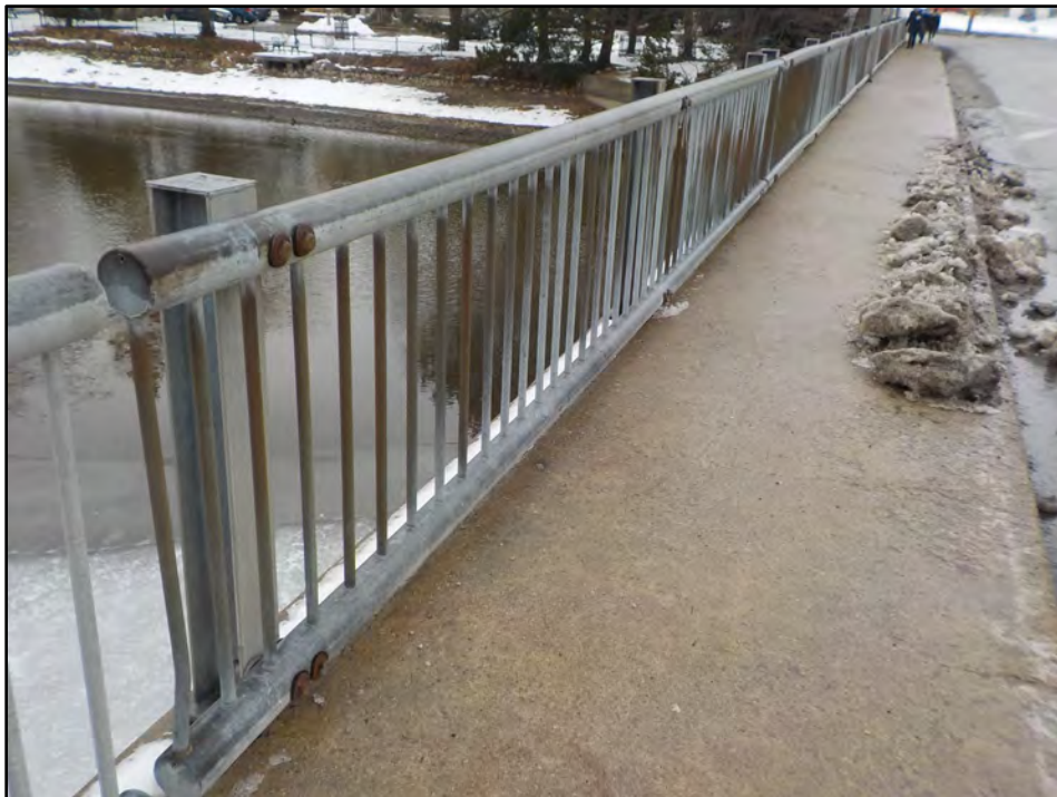
Photo 10: Light to Localized Moderate Corrosion on Steel Barrier
