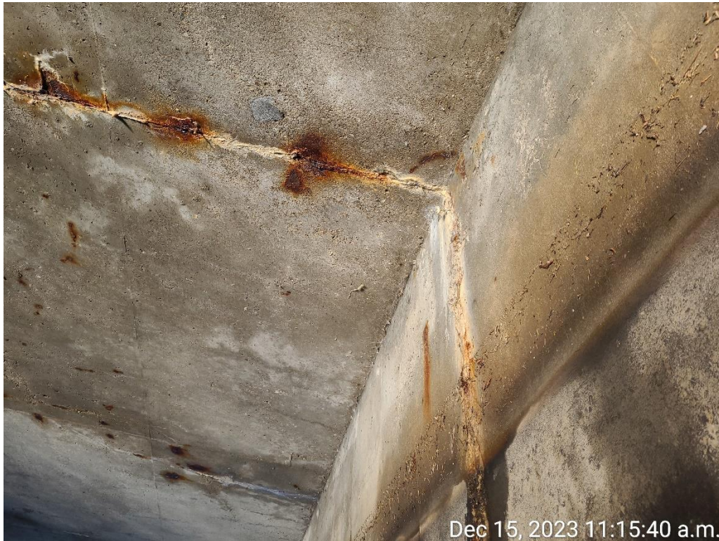
Photograph 15: East span centerline crack continue into east abutment wall
