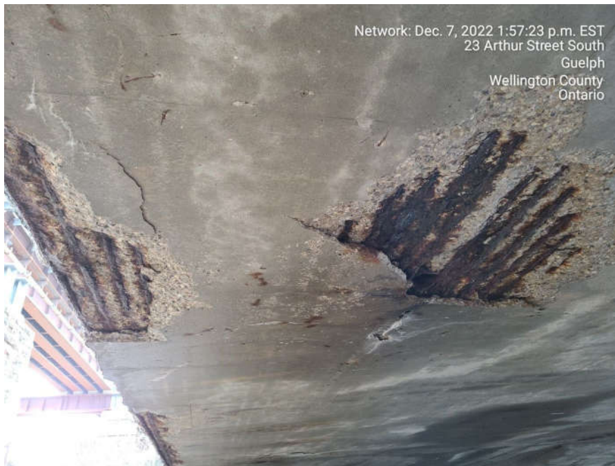
South soffit exterior and interior showing spalls and exposed corroded rebars
