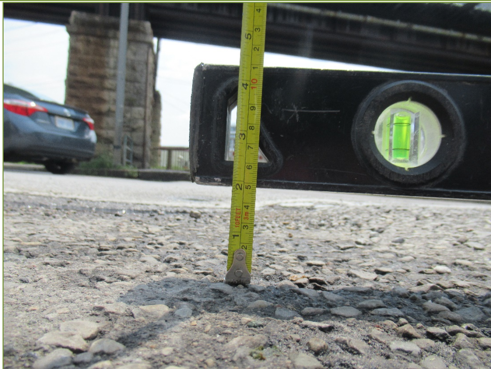
Photo P34 East Joint (settlement)
