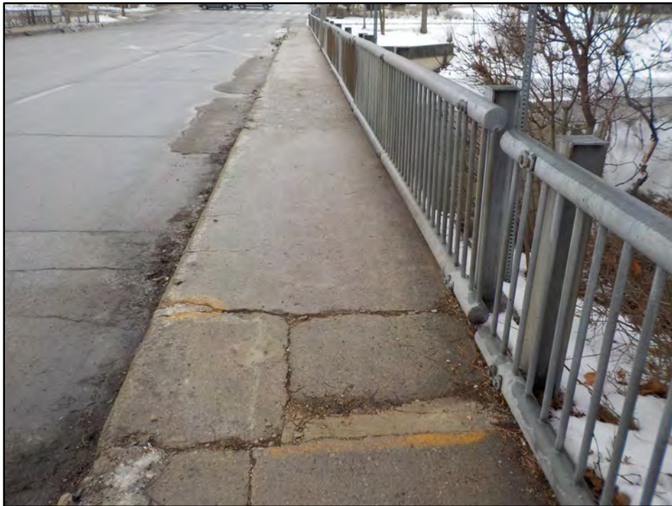
Photo 8: Wide Cracks on North Sidewalk at East End of Deck
