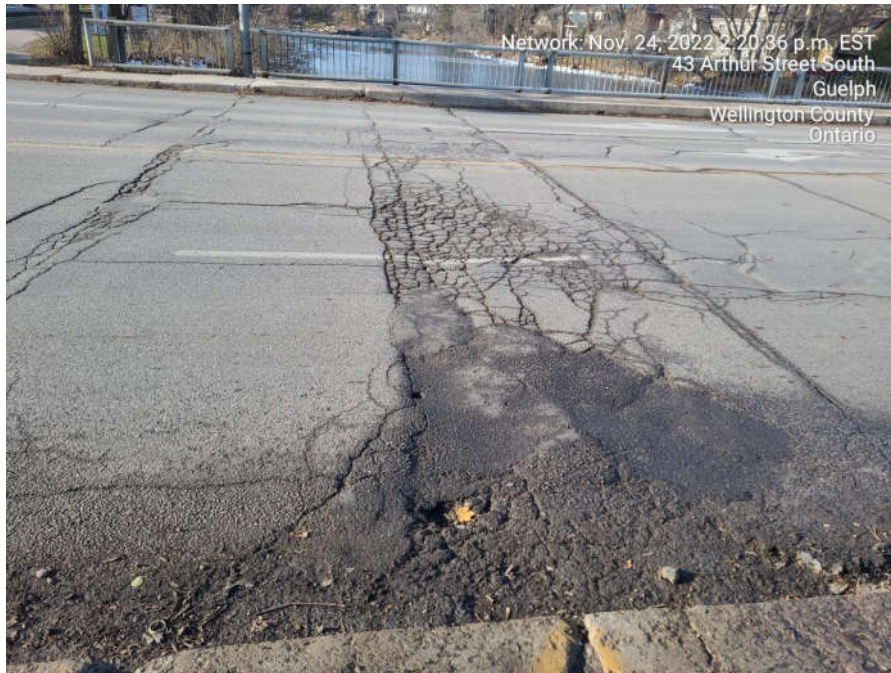
Severe alligator cracking and severe transverse and longitudinal cracks throughout wearing surface
