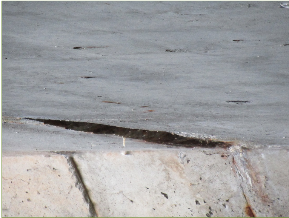
Photo P21 Soffit at East Abutment (cracks, and spall)
