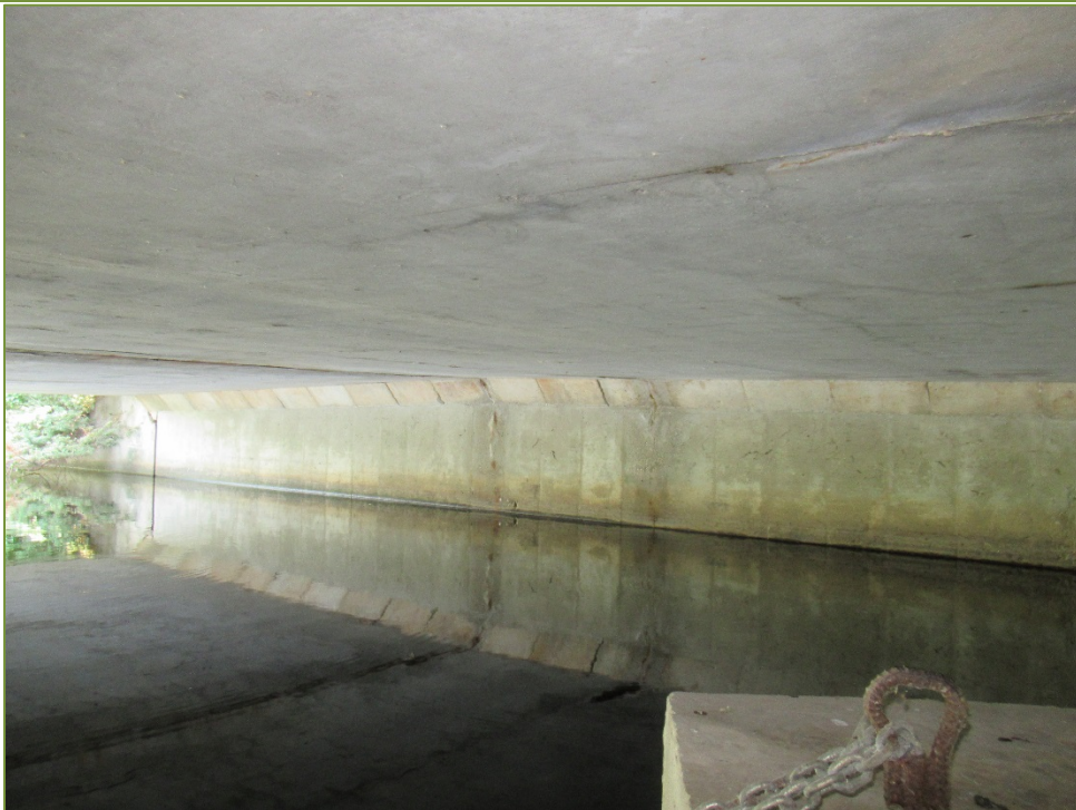
Photo P46 East Abutment (fair condition – cracks, spall, light to medium scaling, and wet area)
