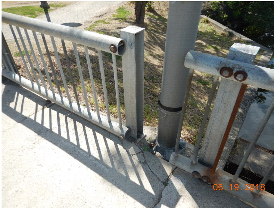
Northwest railing, missing end cap
