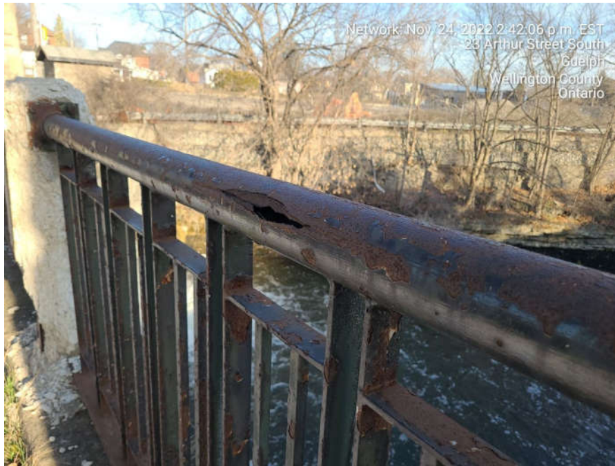
South barrier showing section loss on top rail
