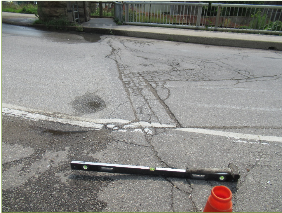
Photo P33 East Joint (settlement and water ponding)
