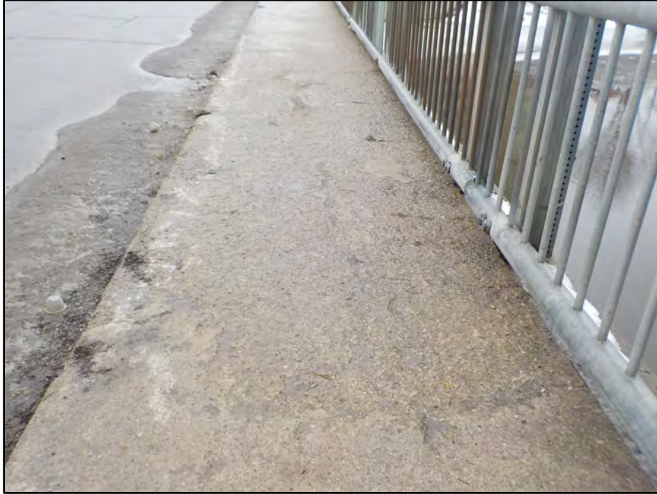
Photo 9: Light to Moderate Scaling on North Sidewalk
