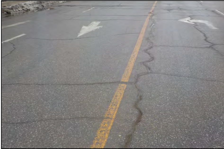
Photo 11: Wide Transverse and Longitudinal Cracks on Deck Wearing Surface
