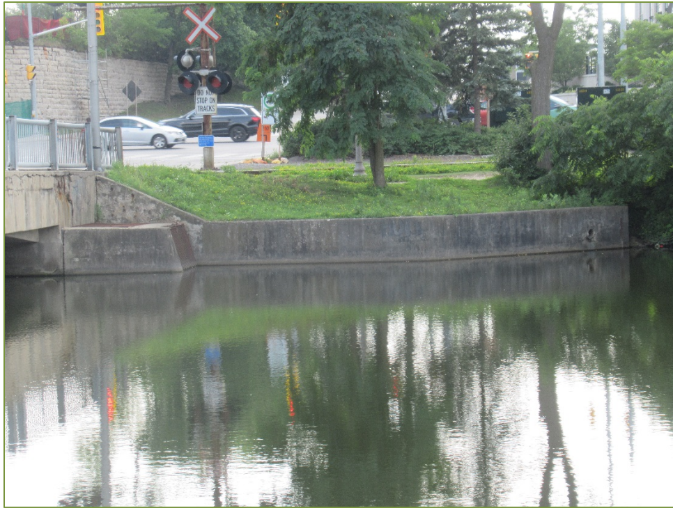
Photo P53 Northwest Retaining Wall (fair condition – cracks, spall and light to severe scaling)
