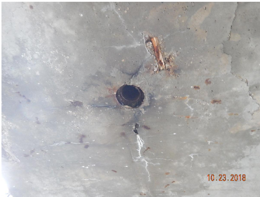
Typical deck drain in soffit
