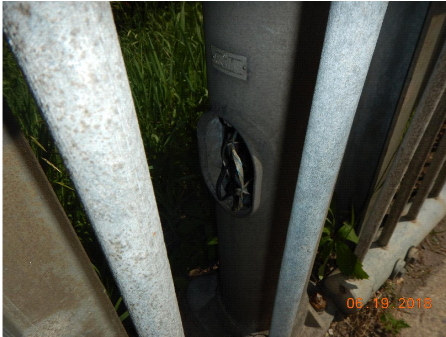
Southwest light post, missing electrical cover
