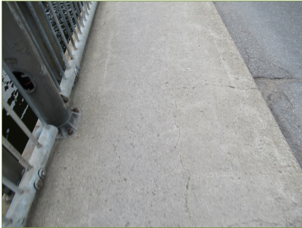
Photo P43 South Sidewalk (wide cracks and light to medium scaling) and Handrail (light corrosion)
