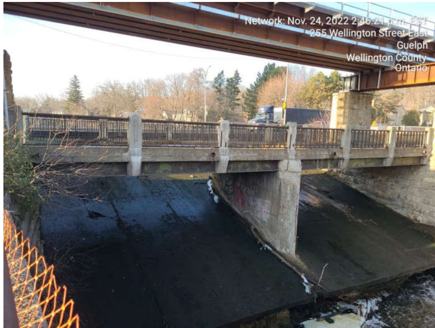
South elevation, showing possible undermining under southeast foundation
