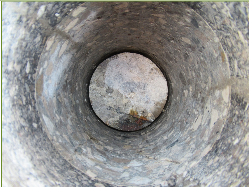
Photo P68 Typical Condition of Inside Core – C9
