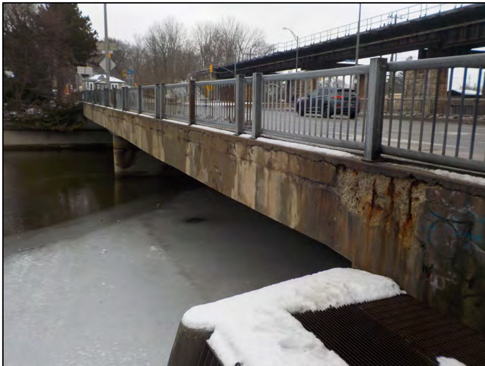
Photo 12: Medium Cracks and Large Spall with Exposed Corroded Reinforcing Steel on North Soffit Fascia
