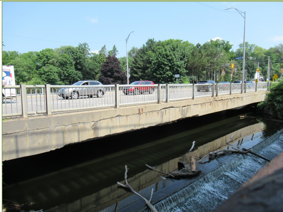
Photo P24 South Elevation – Fascia (wide cracks, spall and delamination)
