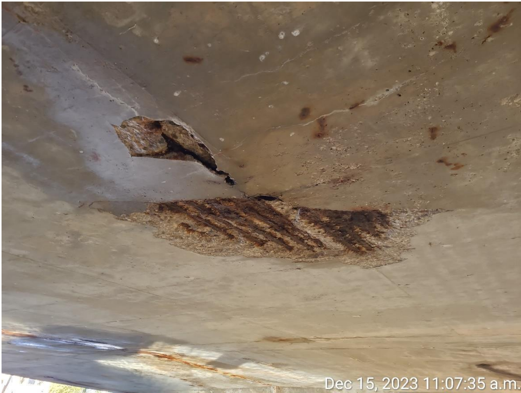
Photograph 9: South soffit interior showing spalls and exposed corroded rebars
