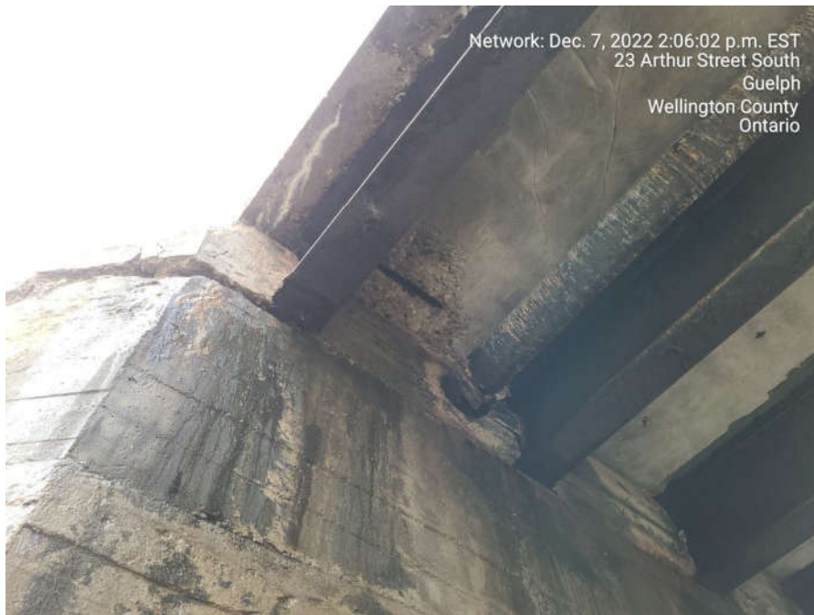
Spalls and exposed corroded rebar on soffit interior on east abutment
