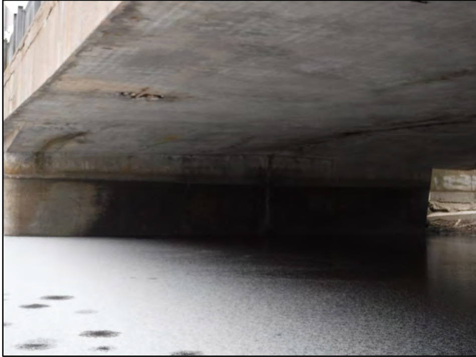
Photo 15: Spall with Exposed Corroded Reinforcing Steel and Delaminated Concrete on Soffit, Center of West Span
