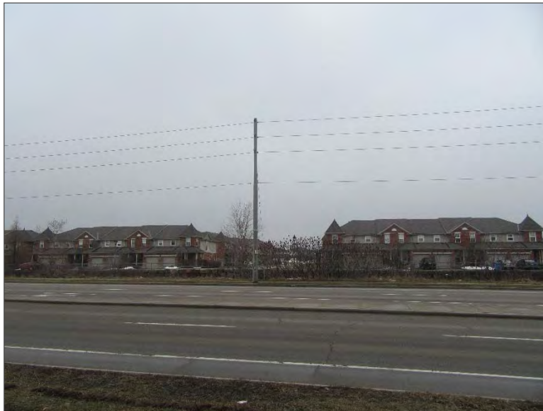
Photo 6 – Adjacent properties southwest of the Site.
