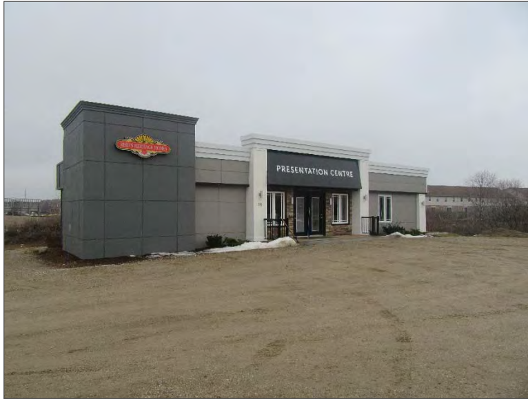
Photo 1 – General view of the Temporary Sales Centre (northeast elevation and partial southeast elevation).
