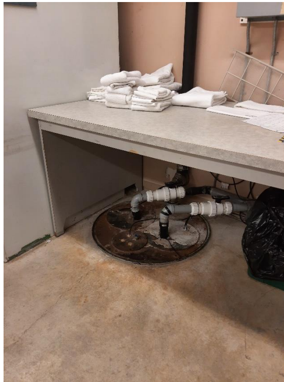
Photograph No. 6 – A sump pump located in the laundry room in the basement of Days Inn.
