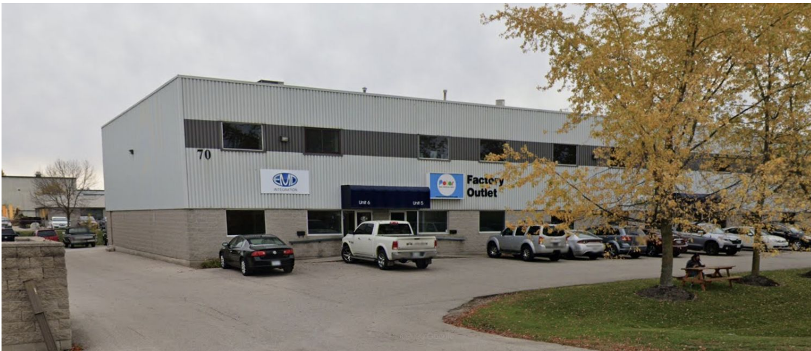
Street view of Subject Site.
