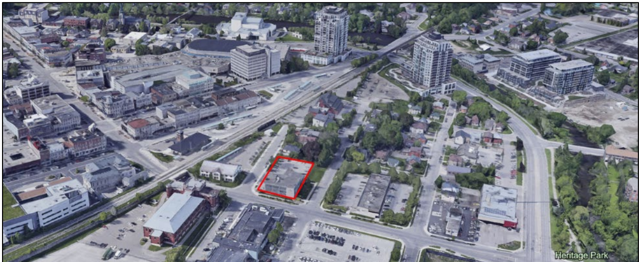
Figure 1: Aerial Image of Subject Property (Source: Google Earth)
