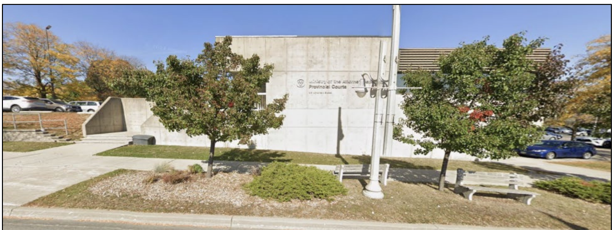
Figure 10: Ministry of Attorney Provincial Courts Building East of the Subject Property (Source: Google Streetview)
