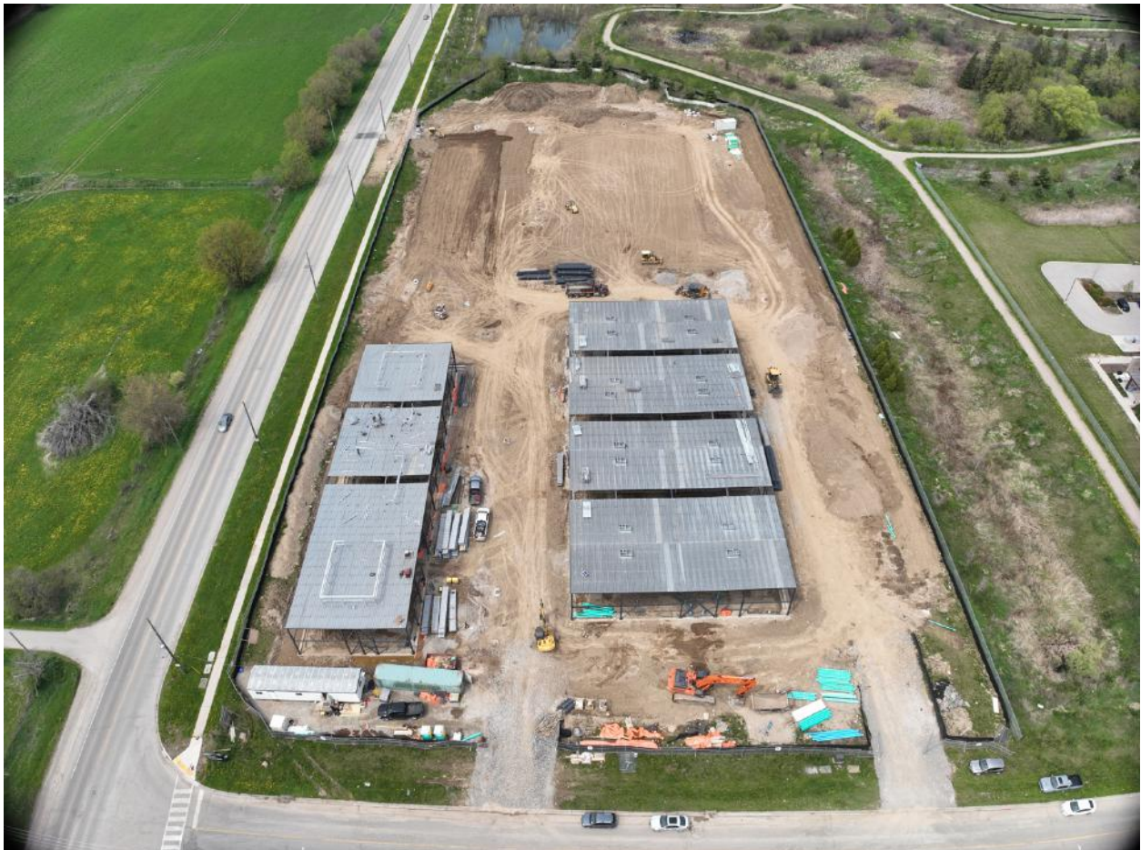
Figure 2 – Aerial Photo of site currently under construction (July 2023)
