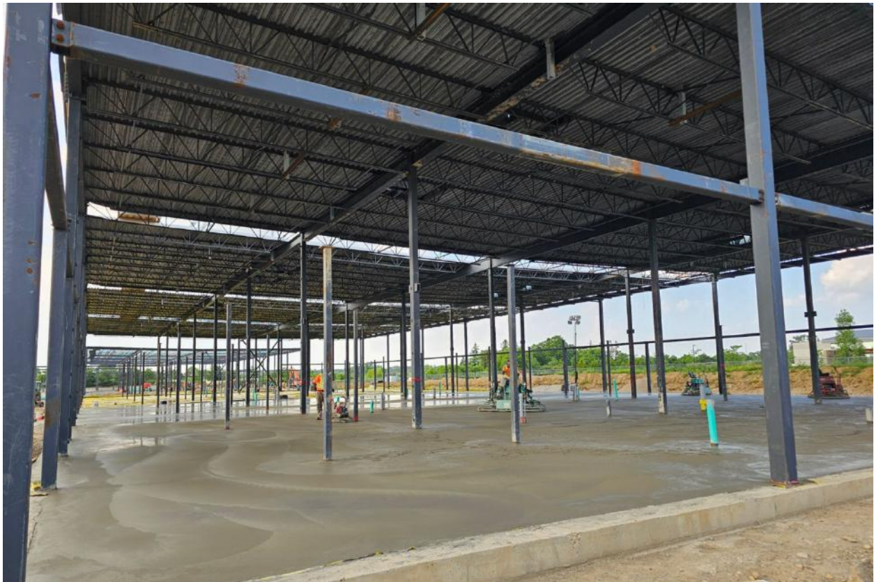
Figure 6 – Building Under Construction
