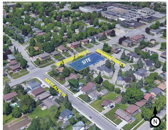
Image 1: Aerial View of the Project Site and Surroundings (courtesy of Google™ Earth)
