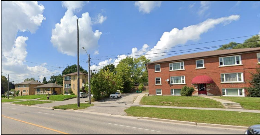
Figure 6. Medium Density Residential uses, looking north of Speedvale Avenue East. Source: Google Streetview
