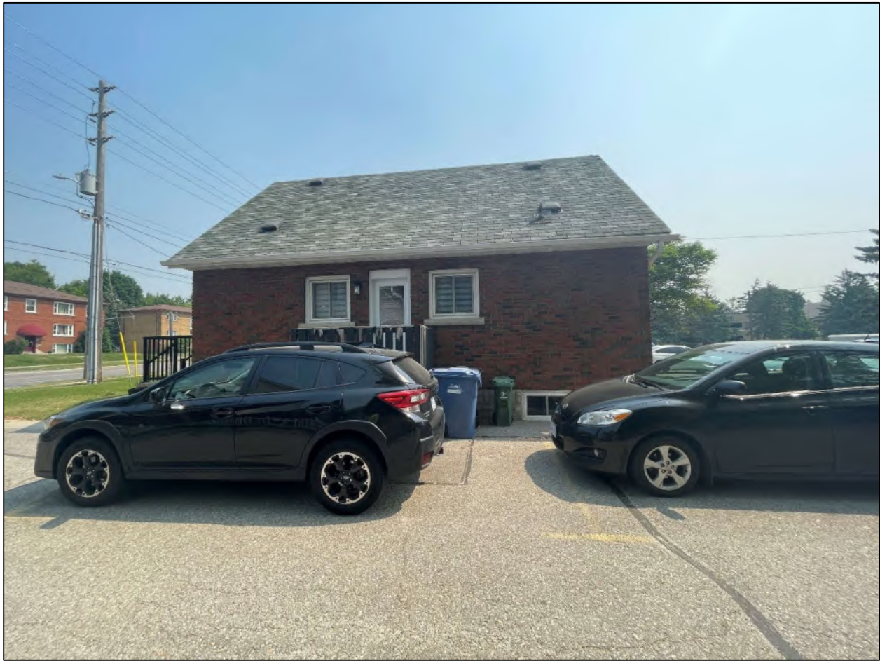
Figure 9 View of southwest elevation of 309 Speedvale Avenue East, facing northeast.
