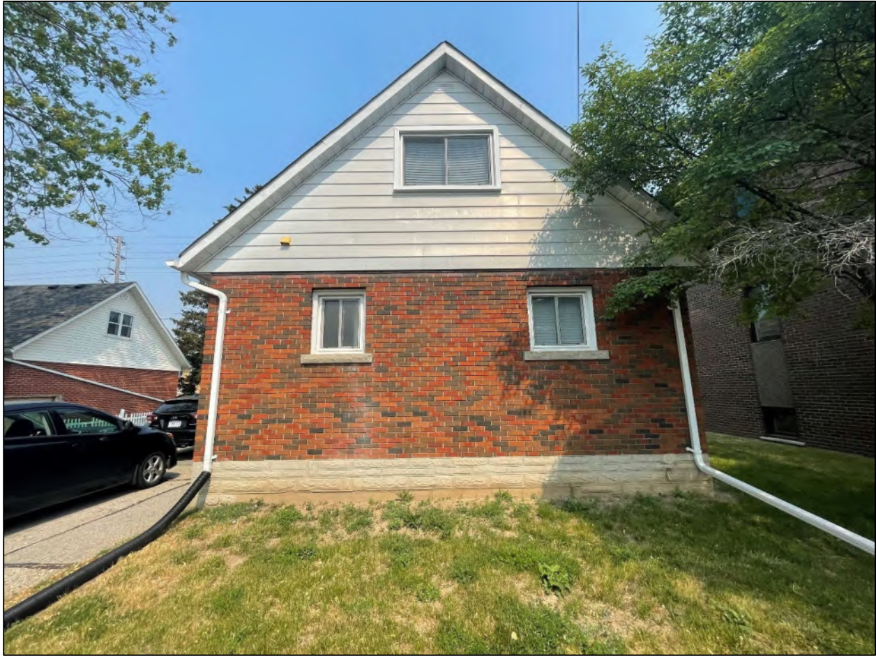
Figure 6 View of southeast elevation of 309 Speedvale Avenue East, facing northwest.
