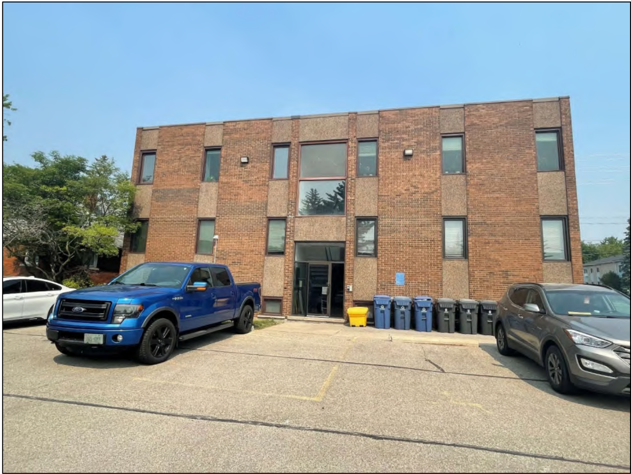
Figure 19 View of the southeast elevation and secondary entrance of 317 Speedvale Avenue East, facing northwest and showing waste bin storage location.
