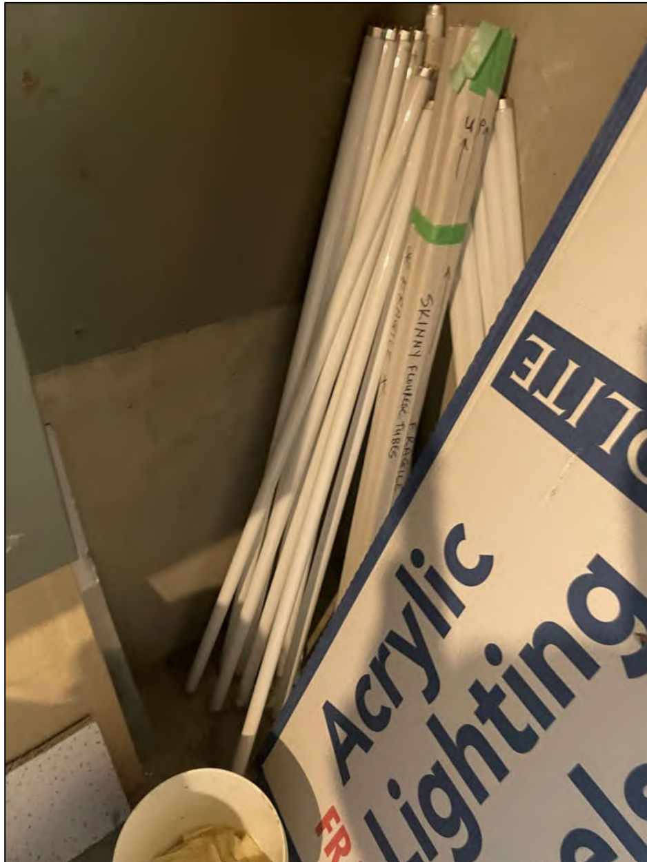
Figure 26 View of storage of additional fluorescent lighting tubes in the front right corner of the mechanical room in the basement of 317 Speedvale Avenue East.
