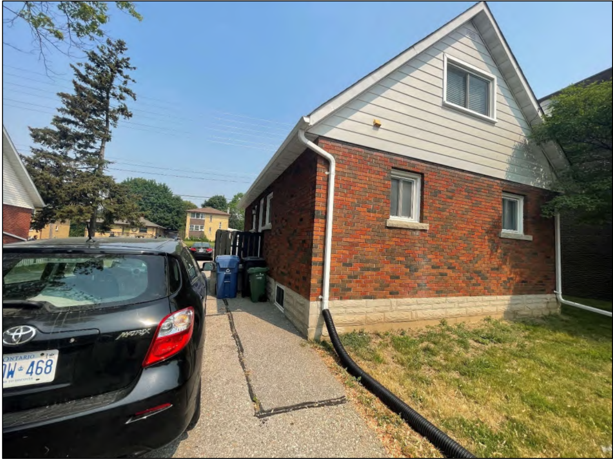
Figure 7 View of southwest elevation of 309 Speedvale Avenue East, facing northwest.
