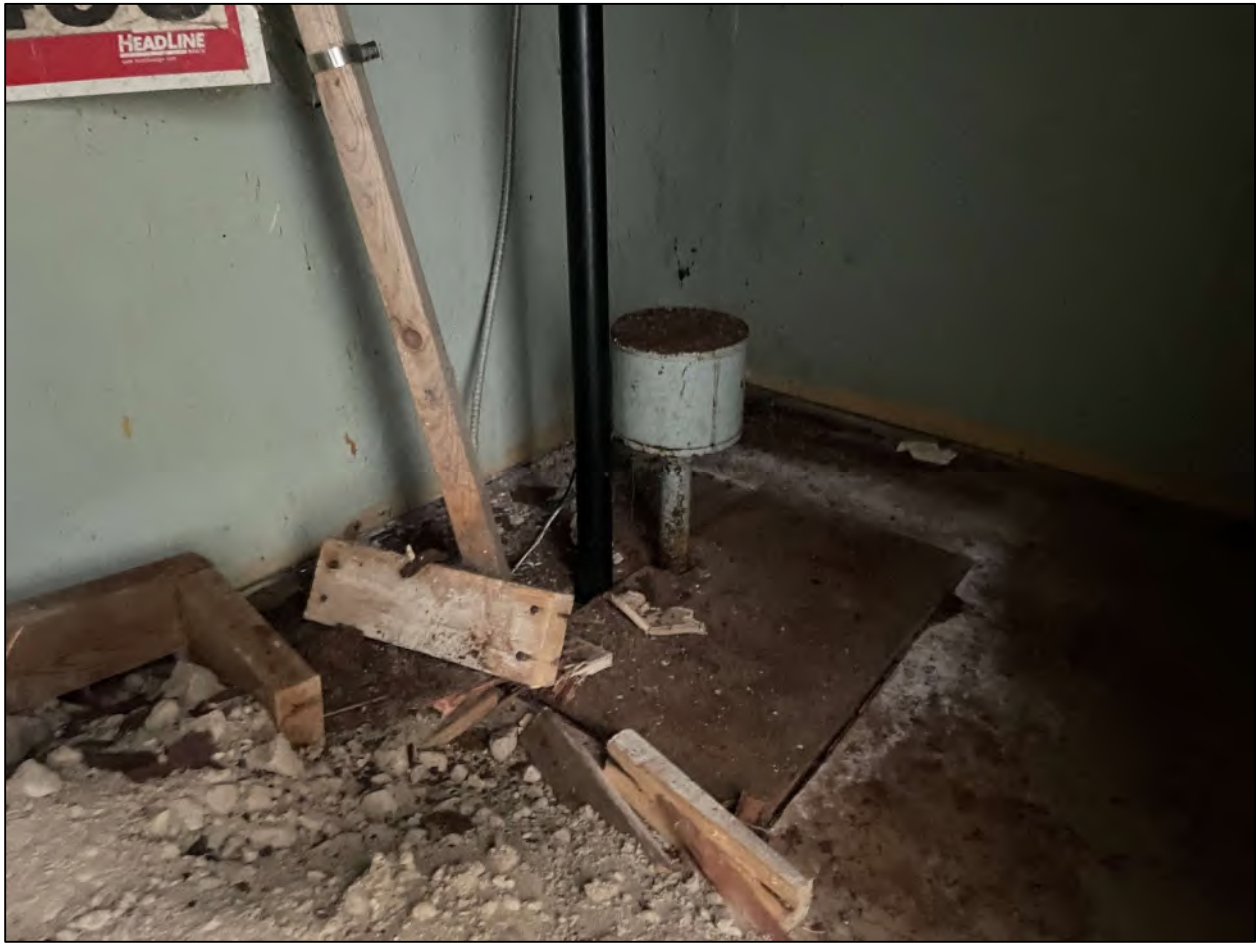
Figure 27 View of the sump in the basement of 317 Speedvale Avenue East.
