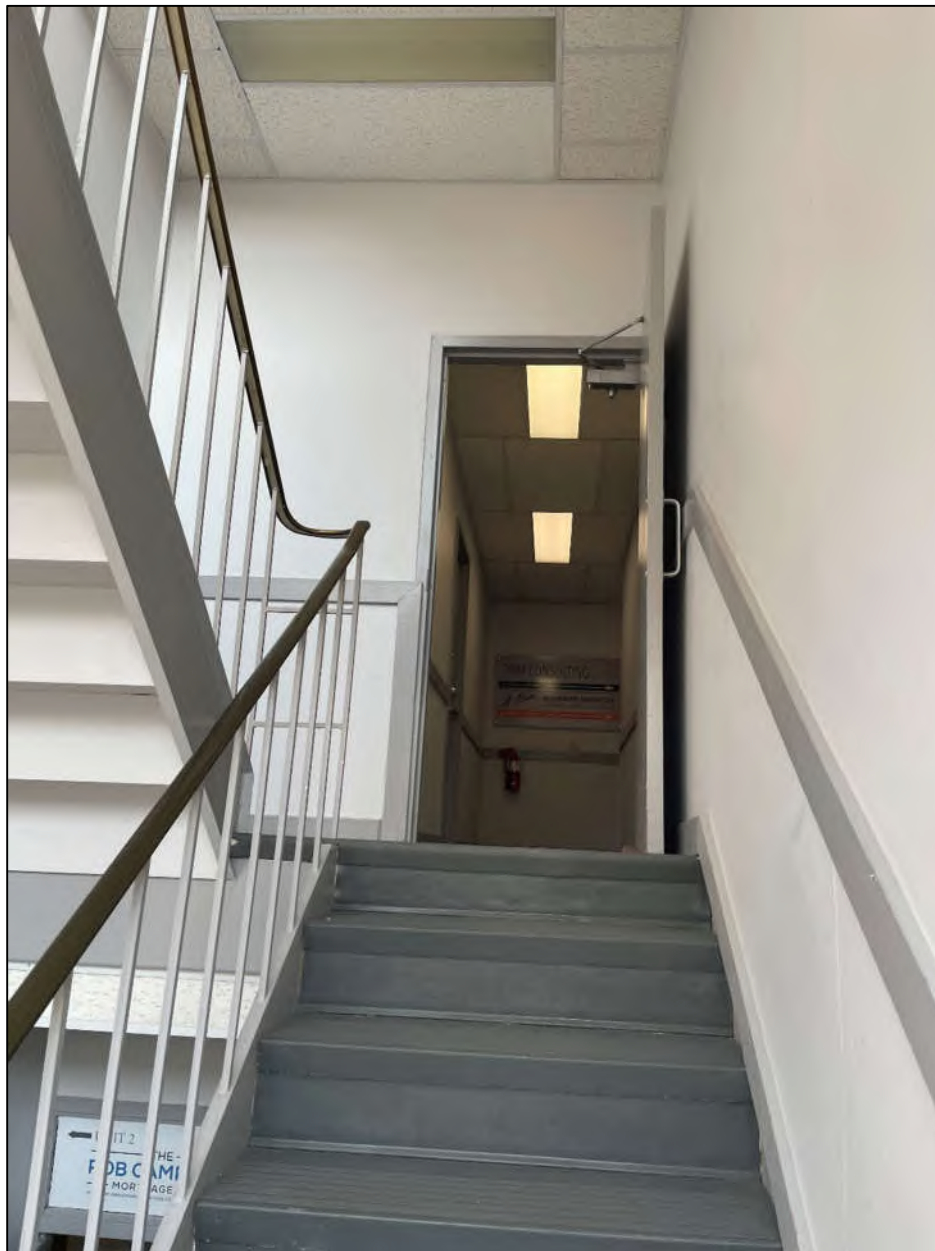
Figure 28 View of the southeast stairwell in 317 Speedvale Avenue East.
