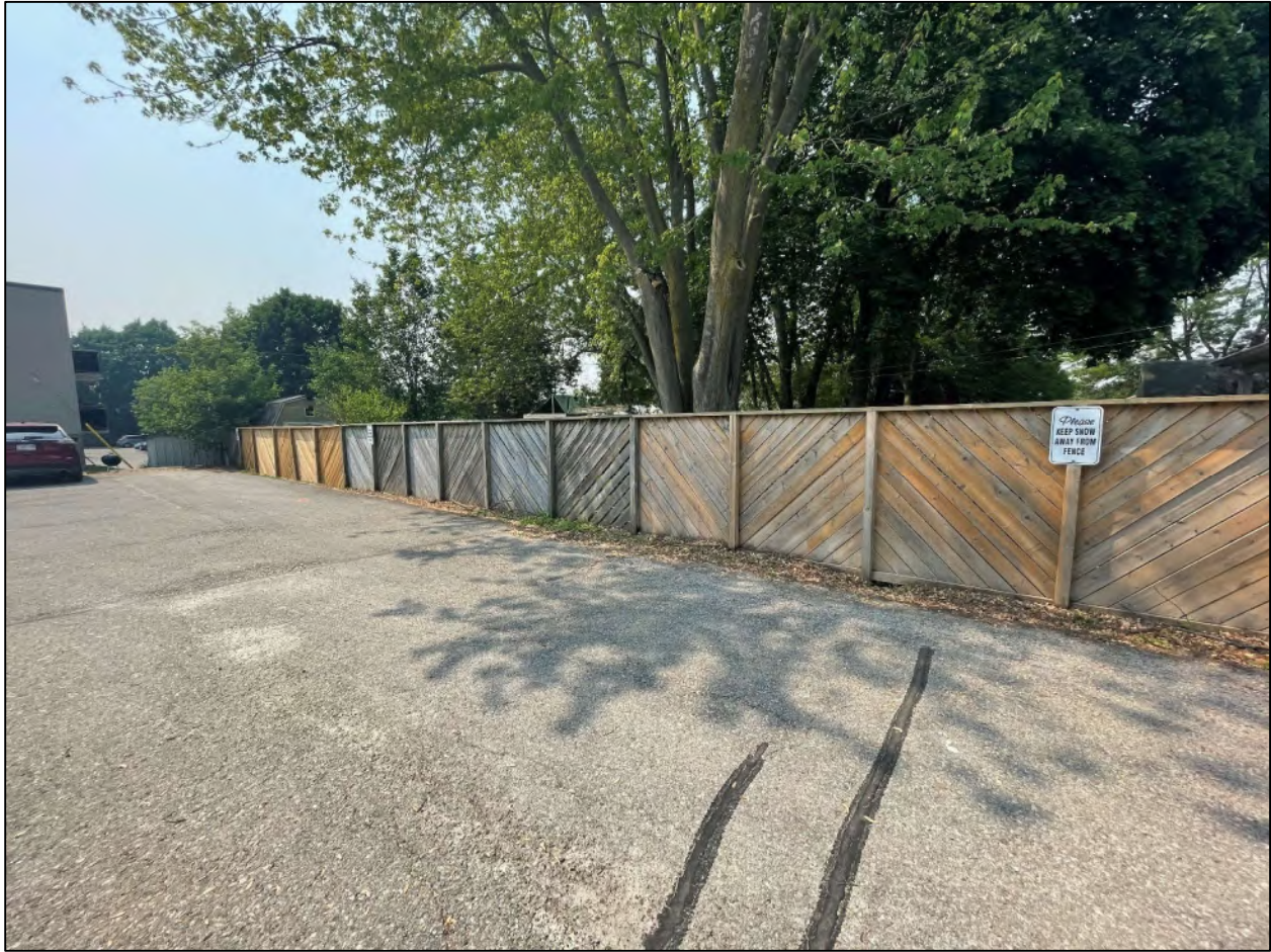
Figure 22 View of the parking lot and fence along the property boundary of 303 and 309 Speedvale Avenue East and located on the south side of the parking area behind 317 Speedvale Avenue East, facing south.
