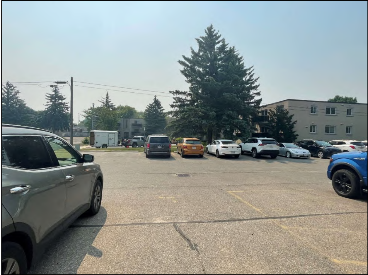
Figure 21 View of the parking lot and one of the catch basins located on the southeast side of 317 Speedvale Avenue East, facing southeast. Overhead lines running parallel to the property boundary are also visible.
