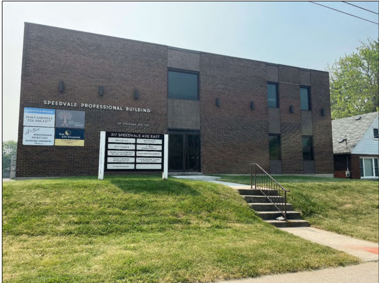
Figure 16 View of the northwest elevation and main entrance of 317 Speedvale Avenue East, facing southeast.
