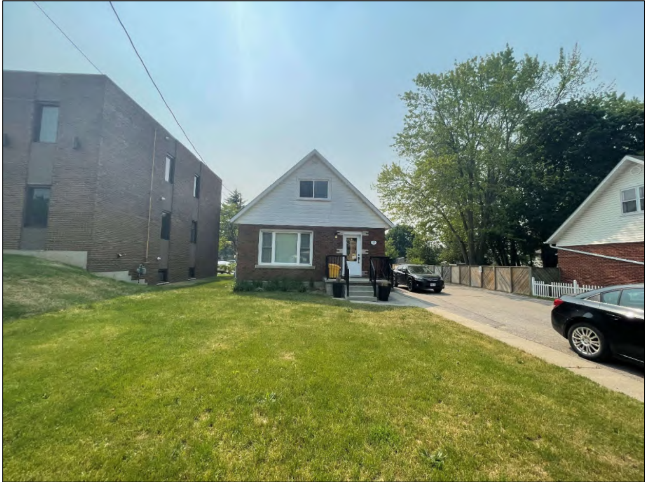
Figure 4 View of 309 Speedvale Avenue East, facing southeast.
