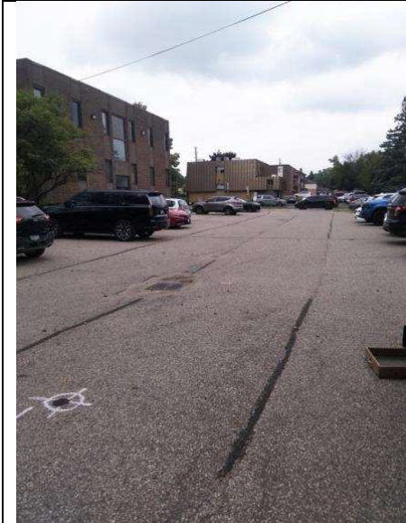
IMAGE 1 PARKING LOT OVERVIEW
