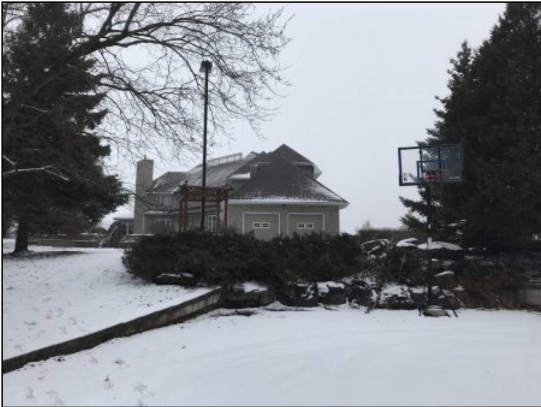
View of the residential building, facing northeast in 2018
