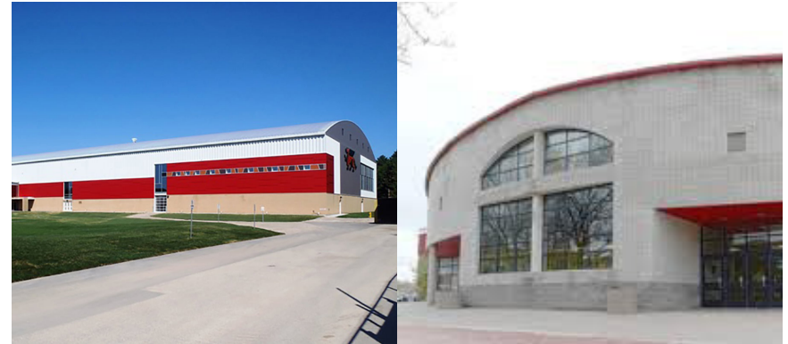
Fig.16: Gryphon Field House Fig.17: Gryphon Centre
