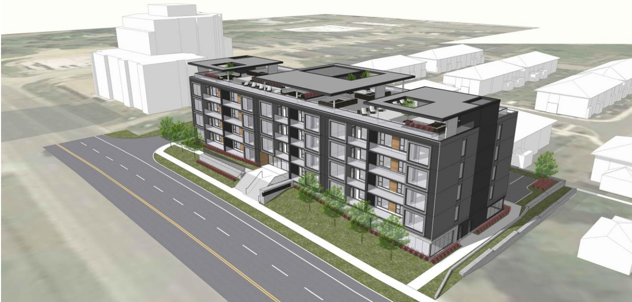
Figure 2: View from Gordon Street looking south.
