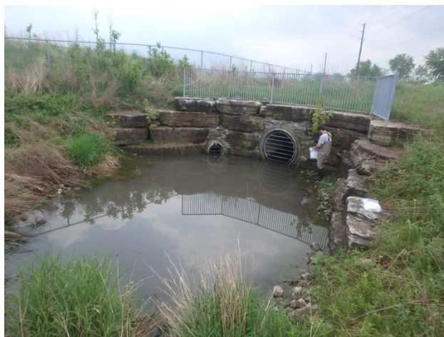
Pond 4: Pond inlet HC-P2(05), backwater conditions
