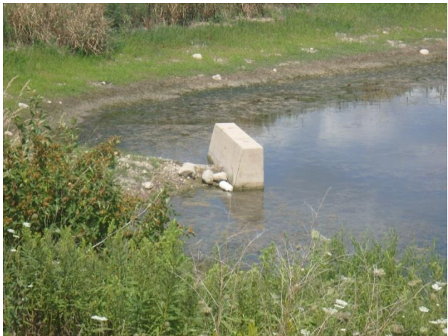
Pond 1: Main cell, exposed outlet structure
