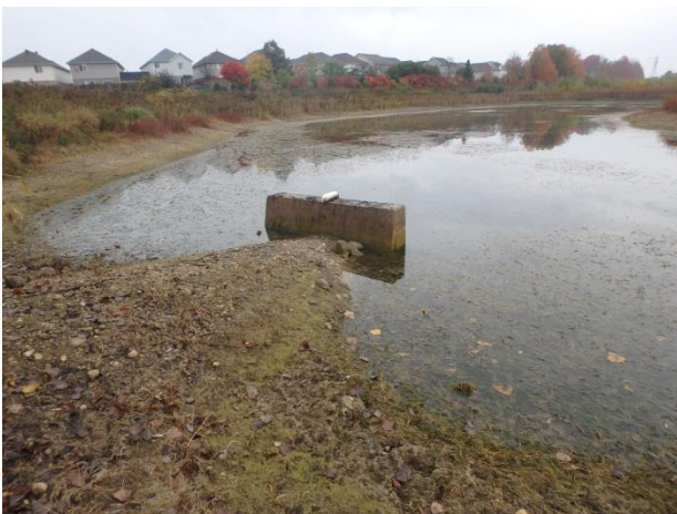
Pond 1: HC-P1(07) Outlet not flowing
