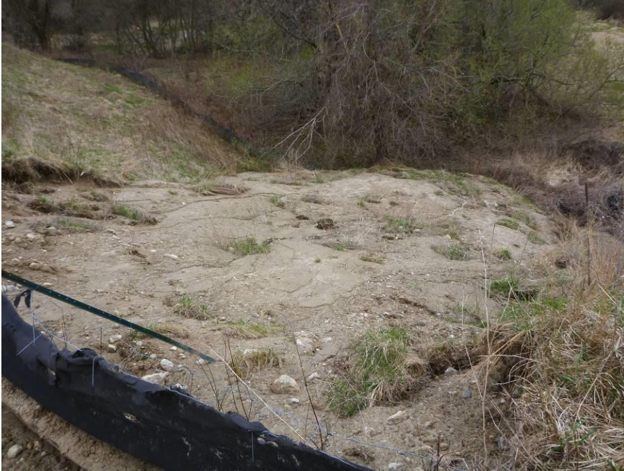
Photo 3: Material migration at most eastern failure location
