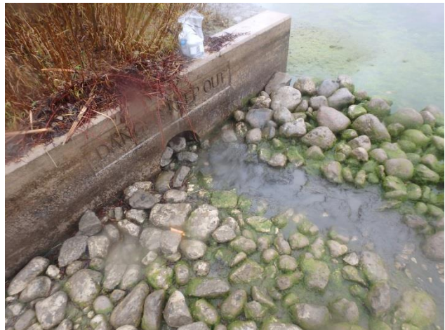
Pond 2: HC-P2(07) Outlet not flowing
