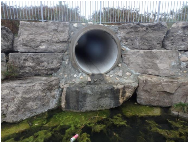
Pond 1: HC-P1(04) not flowing at pond
