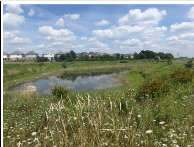
Figure 4-7: Low water levels observed in the main cell of Pond 1. (8/9/2016)
