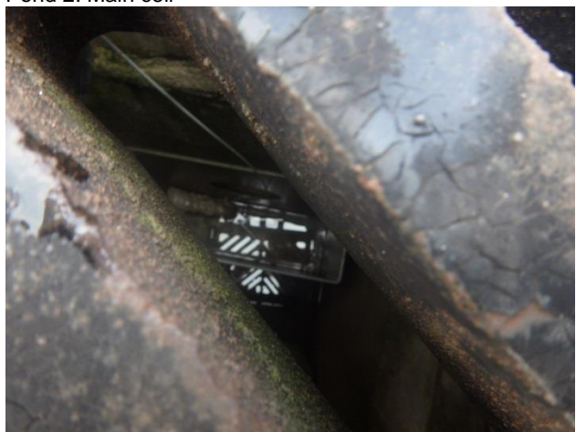
Pond 2: HC-P1(07) outlet not flowing
