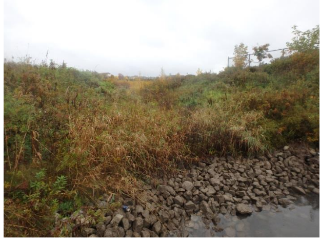
Pond 2: HC-P2(06) Inlet swale not flowing
