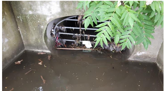
Pond 2: Inlet HC-P2(04), backwater conditions
