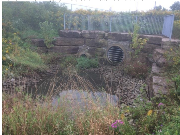
Pond 4: Pond inlet HC-P2(05), backwater conditions
