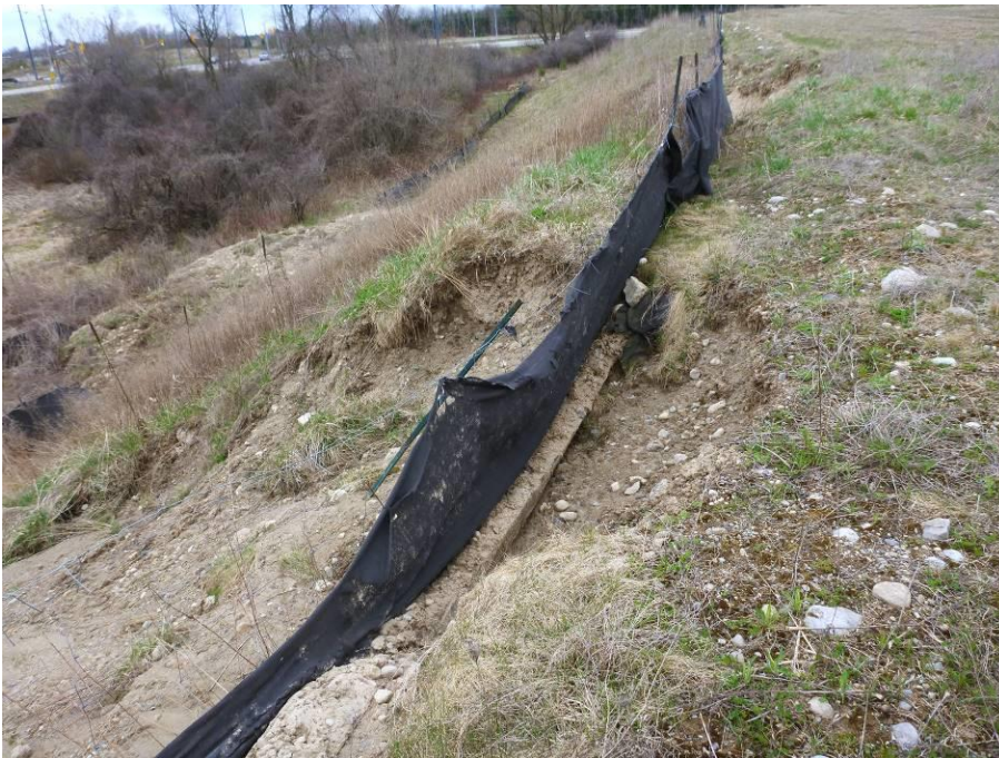
Photo 2: Failure at top of slope, closest to east side
