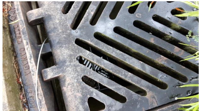
Pond 2: HC-P2(07) outlet not flowing
