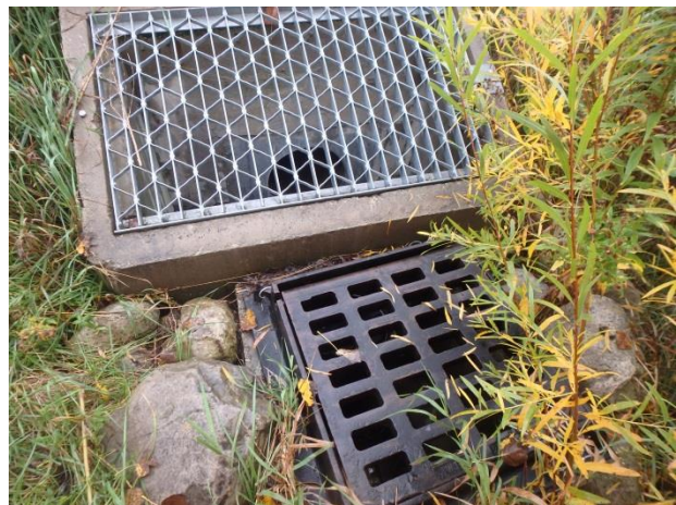
Pond 1: HC-P1(07) Outlet not flowing
