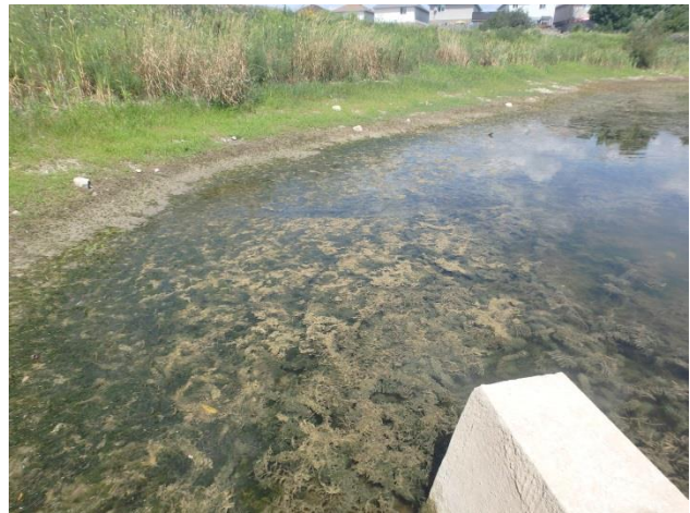
Pond 1: Main cell, low water level looking from outlet structure. Vegetation starting to grow on exposed pond bottom.
