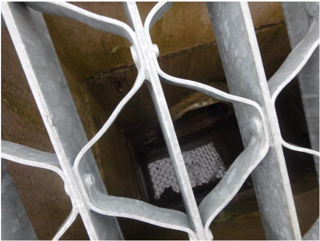
Pond 4: HC-P2(07) outlet not flowing
