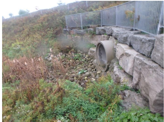
Pond 1: HC-P1(04) with no water at swale culvert
