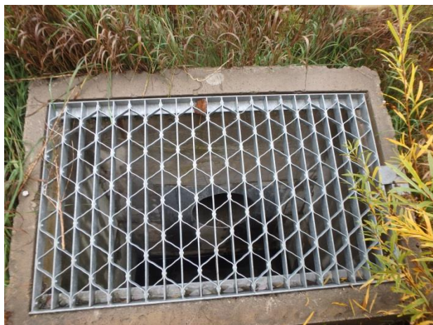
Pond 1: HC-P1(07) Outlet not flowing
