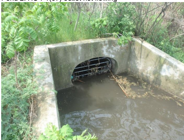
Pond 2: HC-P2(04) inlet, backwater conditions
