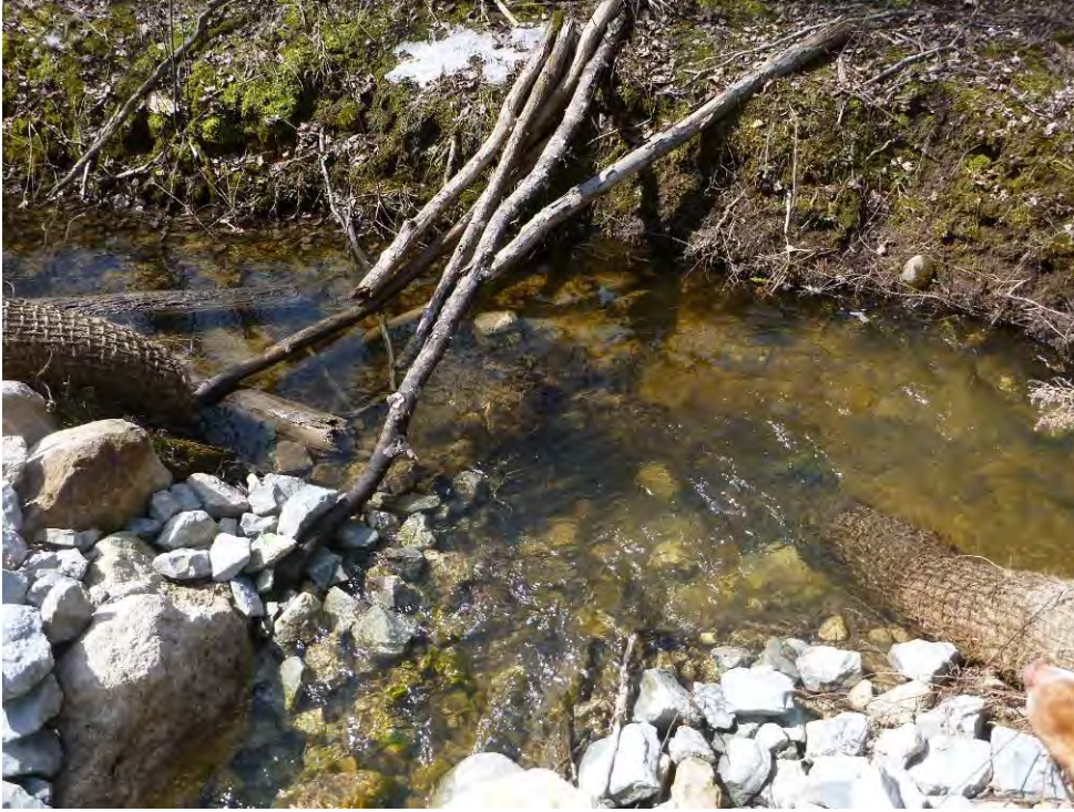
Photo 3: Water flows within SWM Pond 4 cooling trench, coir log and bank undermining
