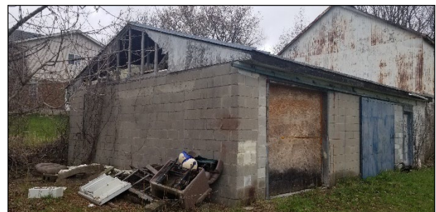
Photos 9 & 10: Views of concrete block wall sections on main barn (left) and addition (right) (source: MHBC, 2022)
