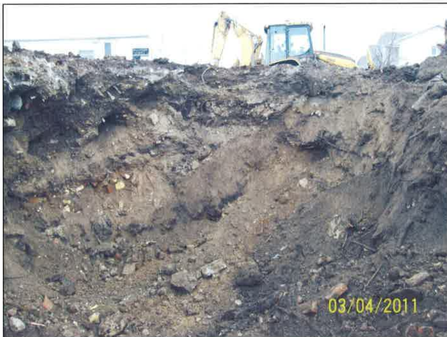
Photo 8 - Northeast area of excavation. Note bricks and debris.
