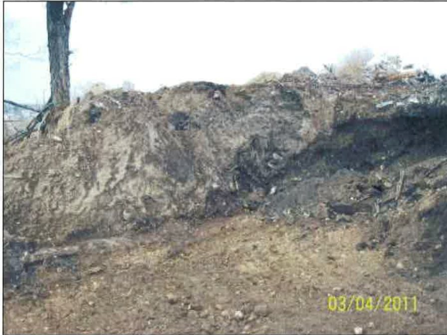
Photo 9 - West side wall of the excavation.
