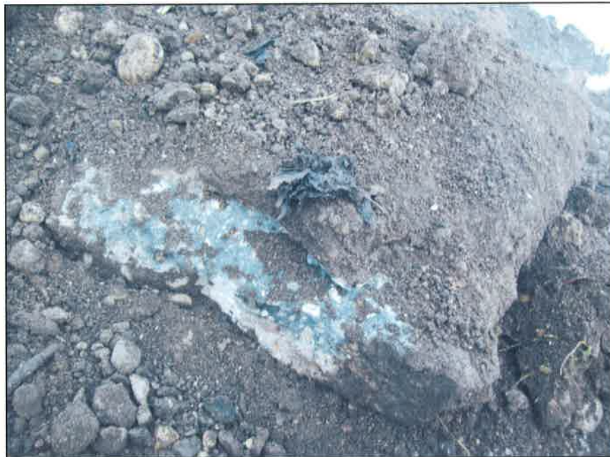
Photo 4 - Buried concrete in TH-12.
