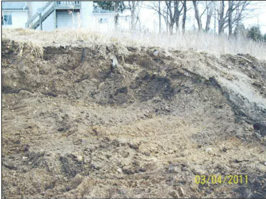
Photo 7 - Native silt till along east of excavation.
