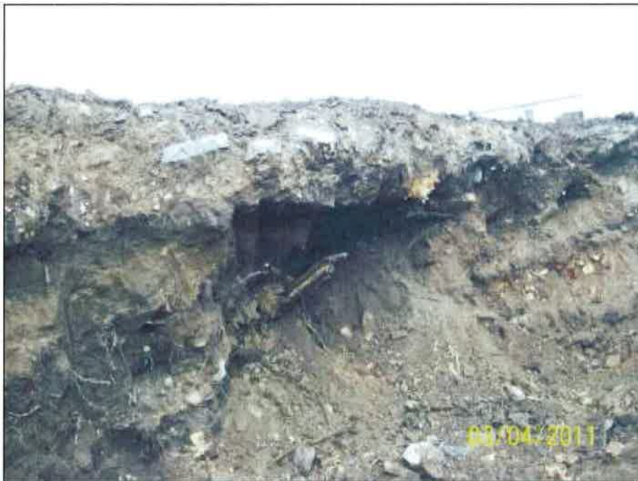
Photo 10 - Northwest wall of excavation.
