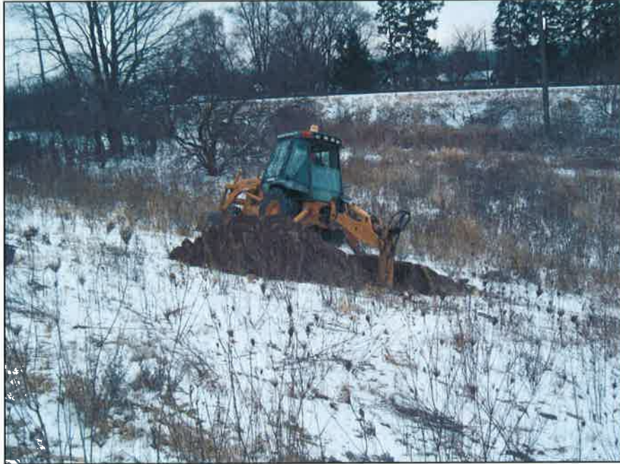
Photo 1 - Excavating testhole TH-10.
