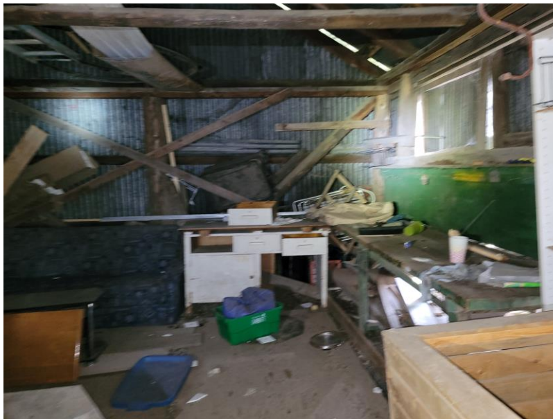
Photograph 6: View inside of the 20 Cityview Dr. N. storage shed.
