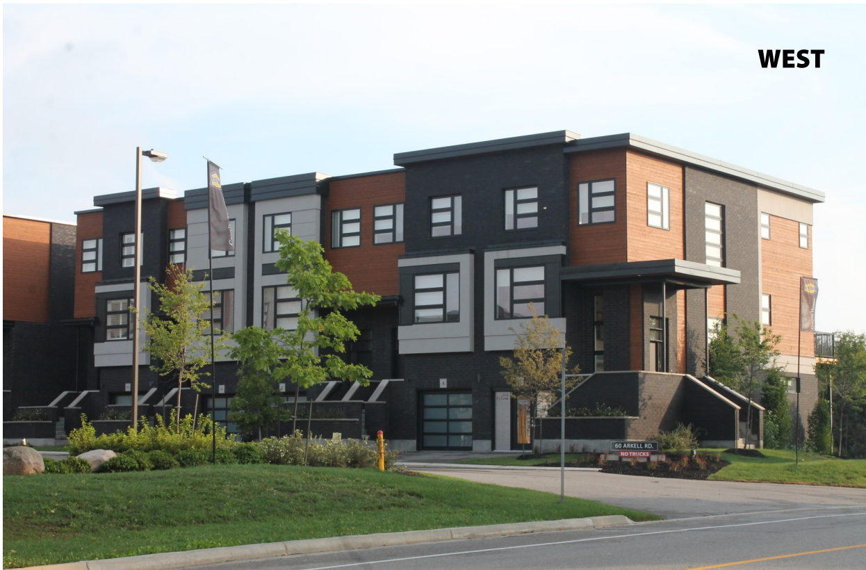
A LARGE MULTI—RESIDENTIAL DEVELOPMENT IS LOCATED FURTHER WEST OF THE SUBJECT LANDS NEAR THE INTERSECTION OF ARKELL ROAD AND GORDON STREET
