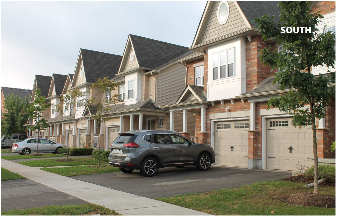
THE SUBDIVISION SOUTH OF THE SUBJECT LANDS INCLUDES A RANGE OF UNIT TYPES, SCHOOLS, PARKS AND TRAILS.
