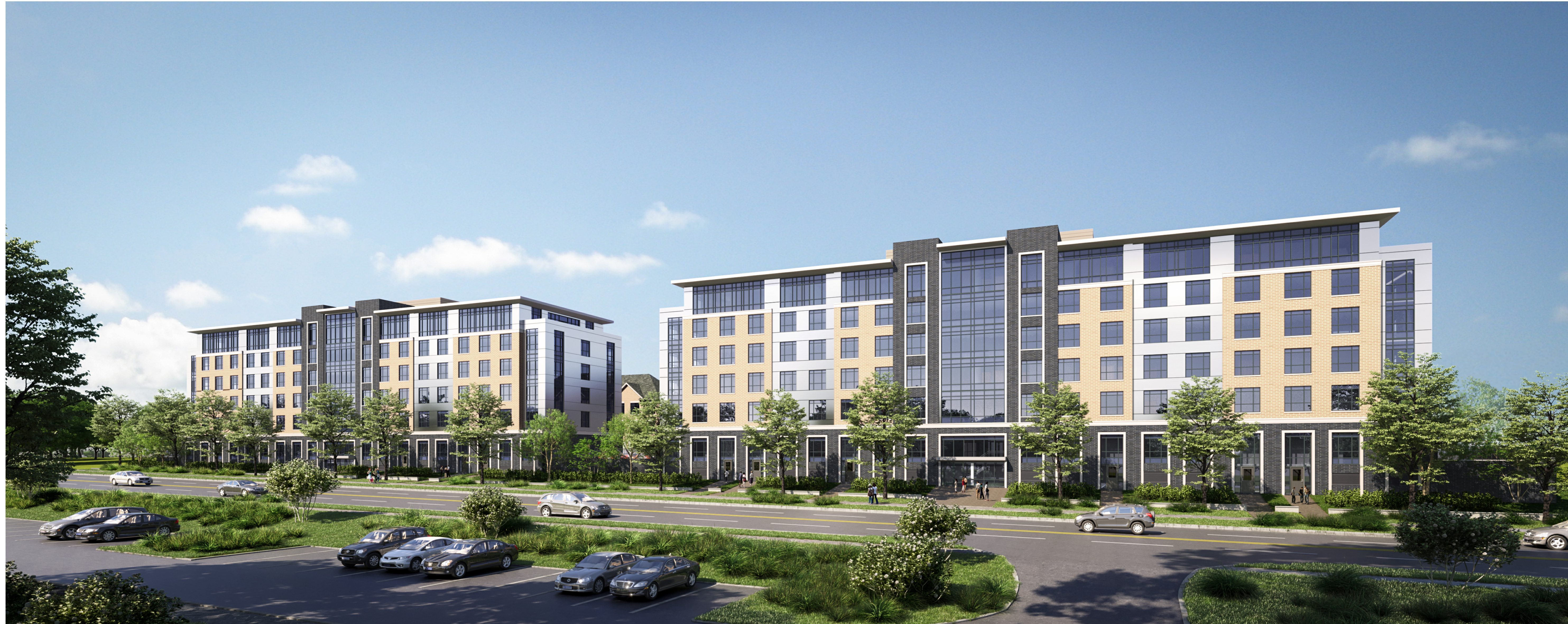
APARTMENT BUILDINGS VIEW FROM GORDON STREET
