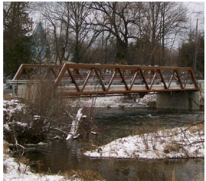
Figure 12: New steel truss bridge constructed with welded connections to mimic previous structure
