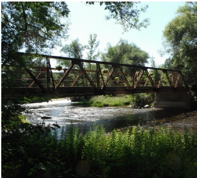
Figure 11: Historic steel truss bridge at the end of its useful life requiring replacement
