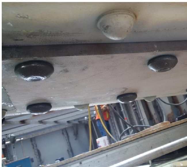
Figure 7: As viewed from the surface, bolts used adjacent to existing rivets to mimic the appearance of rivets
