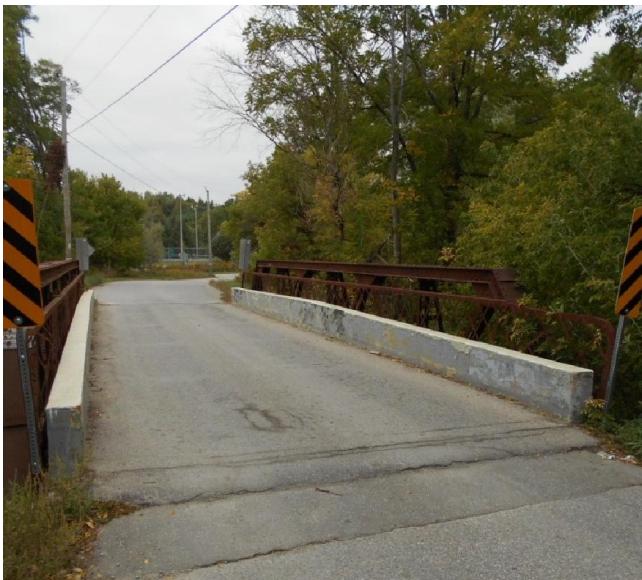
Figure 9: Similar truss bridge with FRP deck, where the steel trusses carry only their own weight
