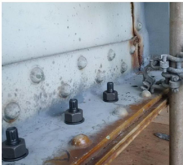
Figure 8: As viewed from the opposite side, these bolts resemble a typical threaded bolt and nut assembly
