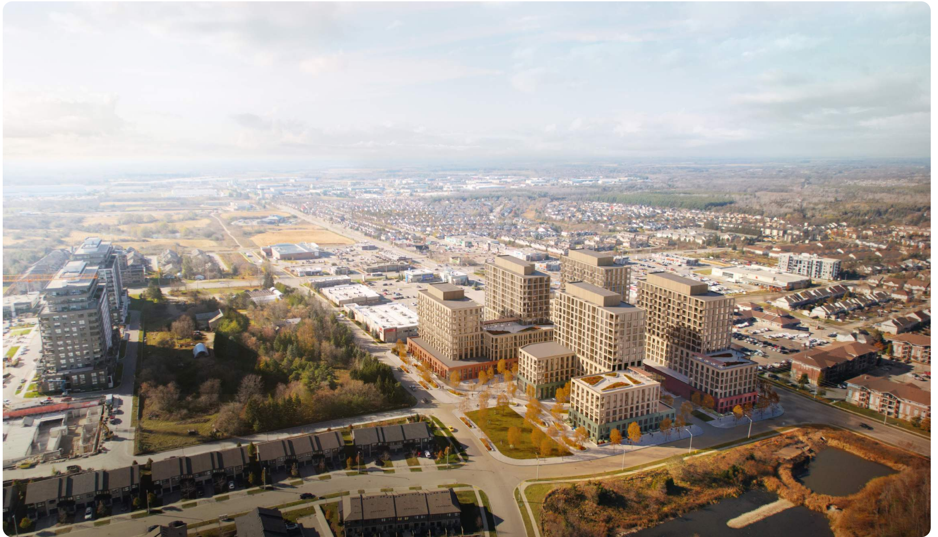
Bird's Eye View Looking Northwest toward Subject Site, (Rendering provided by SvN Architects + Planners)
